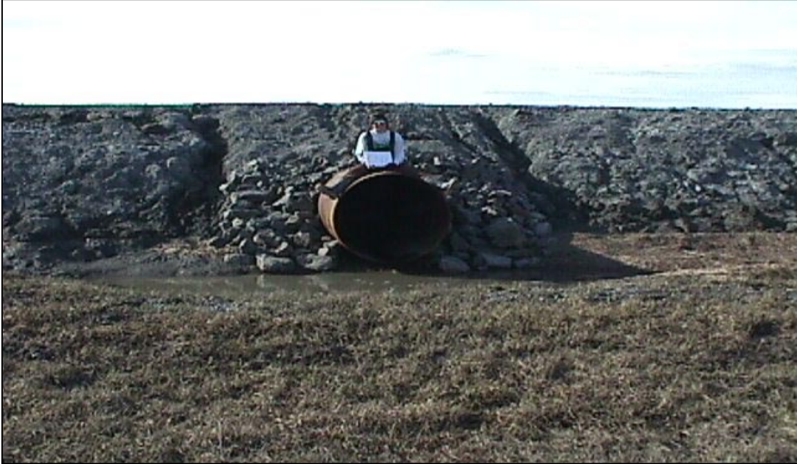
CN-6: Looking south at the north end of the culvert. (6/18/00)
