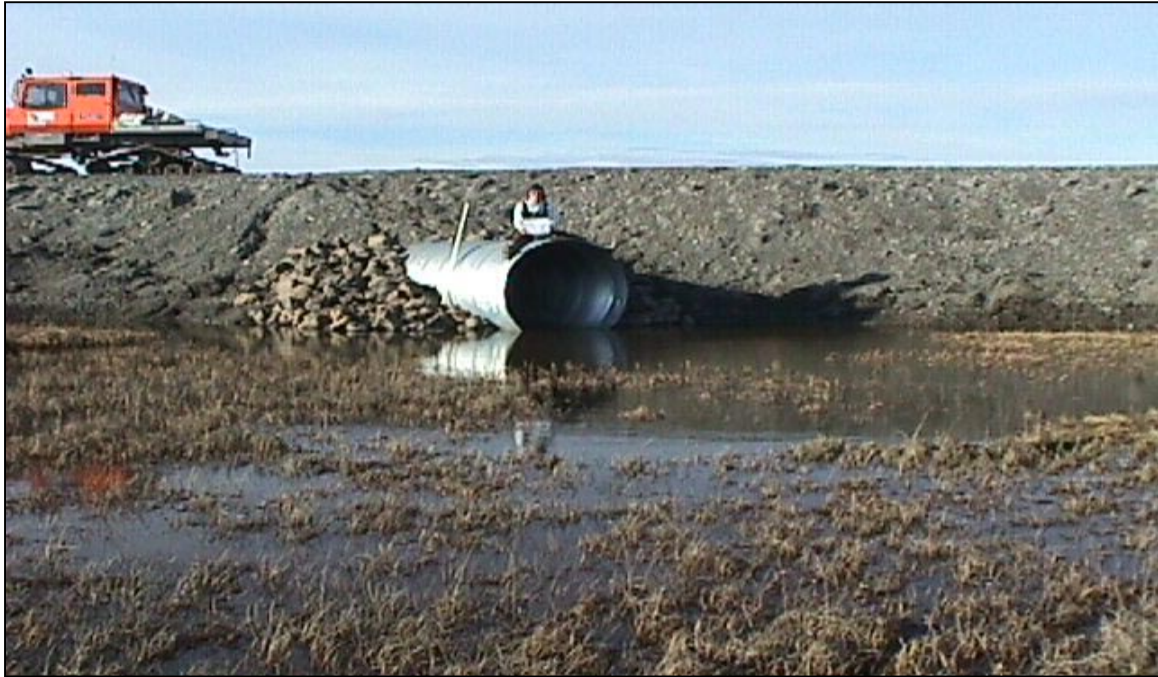
CN-12: Looking south at the north end of the culvert. (6/18/00)
