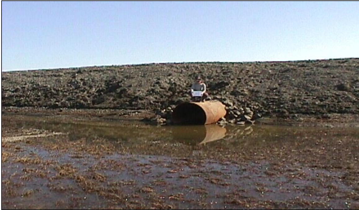
CN-23: Looking south at the north end of the culvert. (6/15/00)
