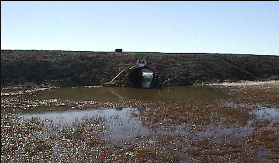
CN-15: Looking south at the north end of the culvert. (6/17/00)
