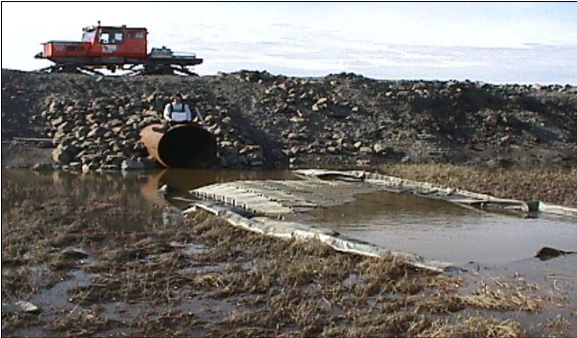
CN-5: Looking south at the north end of the culvert. (6/18/00)
