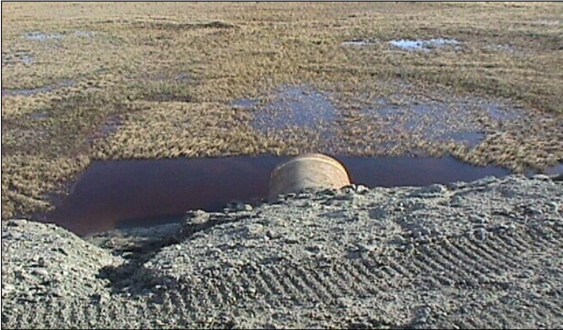
CN-10: Looking north at the north end of the culvert. (6/18/00)
