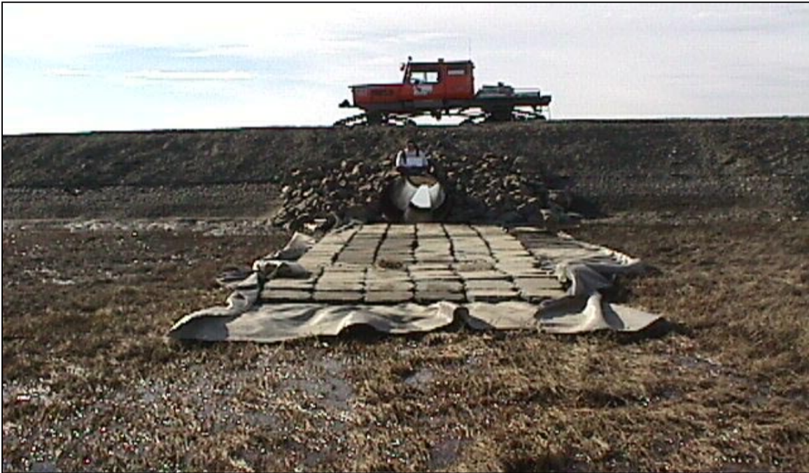
CN-4: Looking south at the north end of the culvert. (6/18/00)
