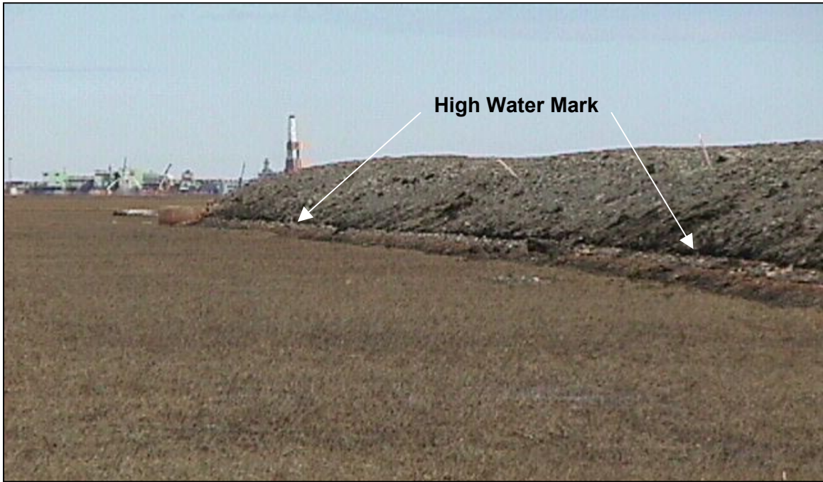
Photo 1: Looking east along the north side of the embankment on the road to CD-2 near culvert CN-24. (6/15/00)
