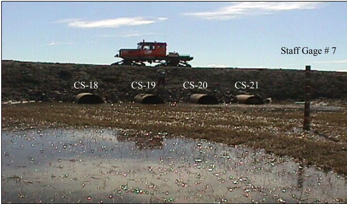
CN-18, CN-19, CN-20, CN-21: Looking south at the north end of the culverts. Staff gage #7 is on the right side of the picture. (6/19/00)
