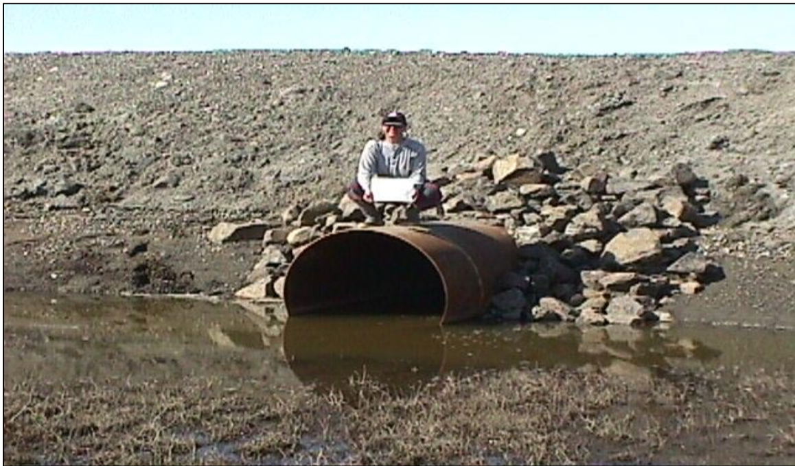
CS-23: Looking north at the south end of the culvert. (6/15/00)
