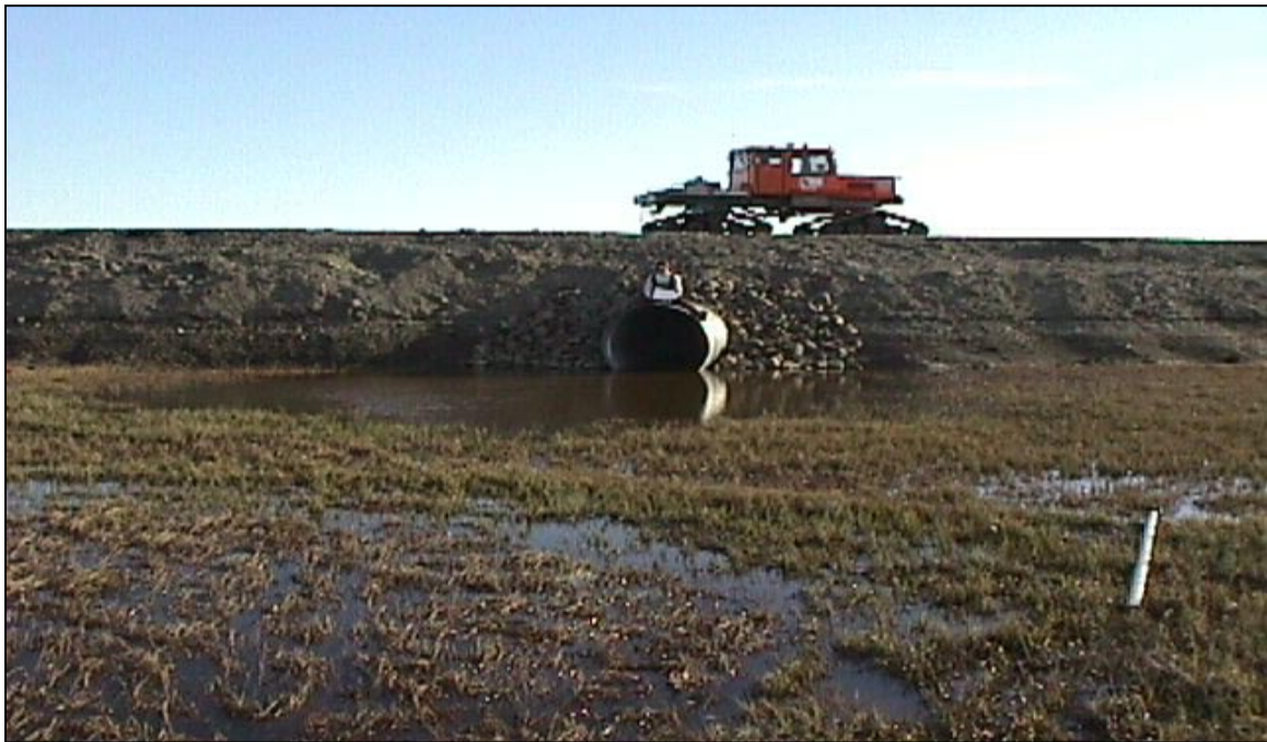
CS-11: Looking north at the south end of the culvert. (6/18/00)
