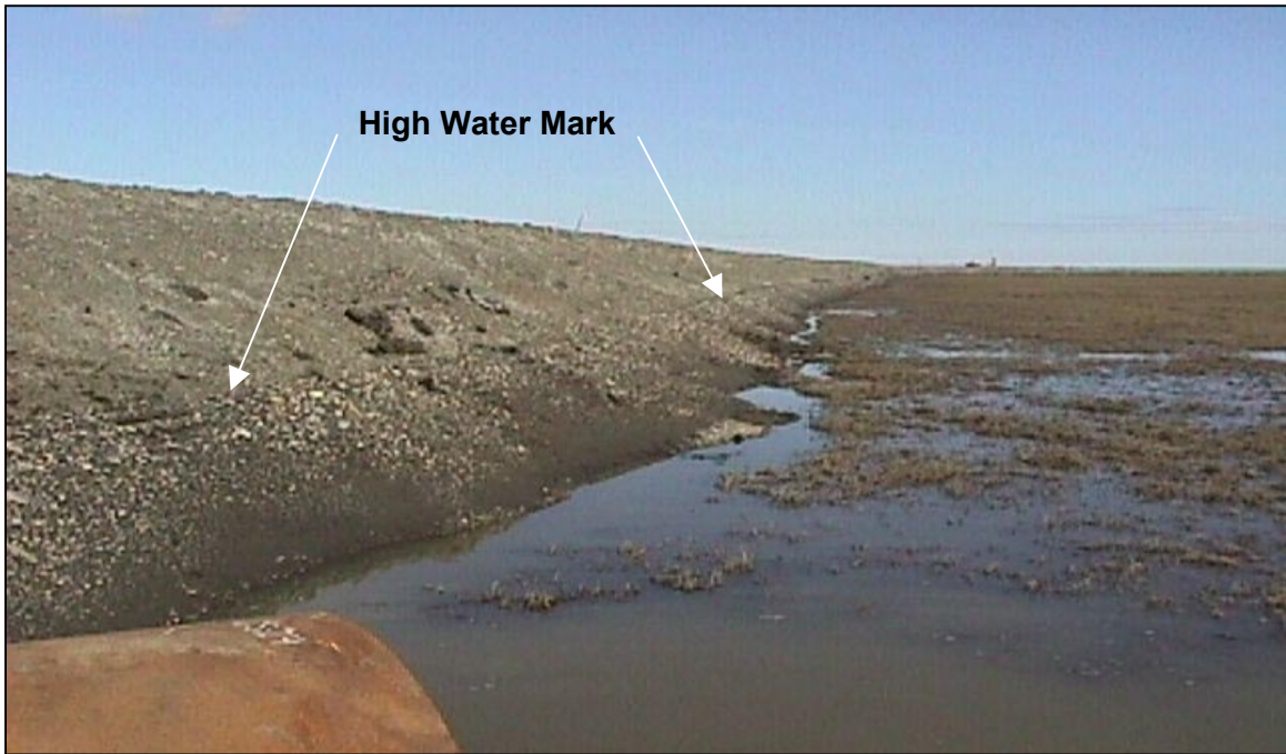
Photo 2: Looking east along the south side of the embankment on the road to CD-2 near culvert CS-24. (6/15/00)
