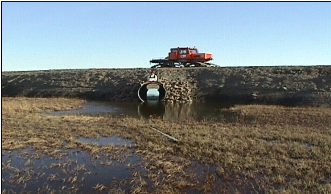
CS-12: Looking north at the south end of the culvert. (6/18/00)
