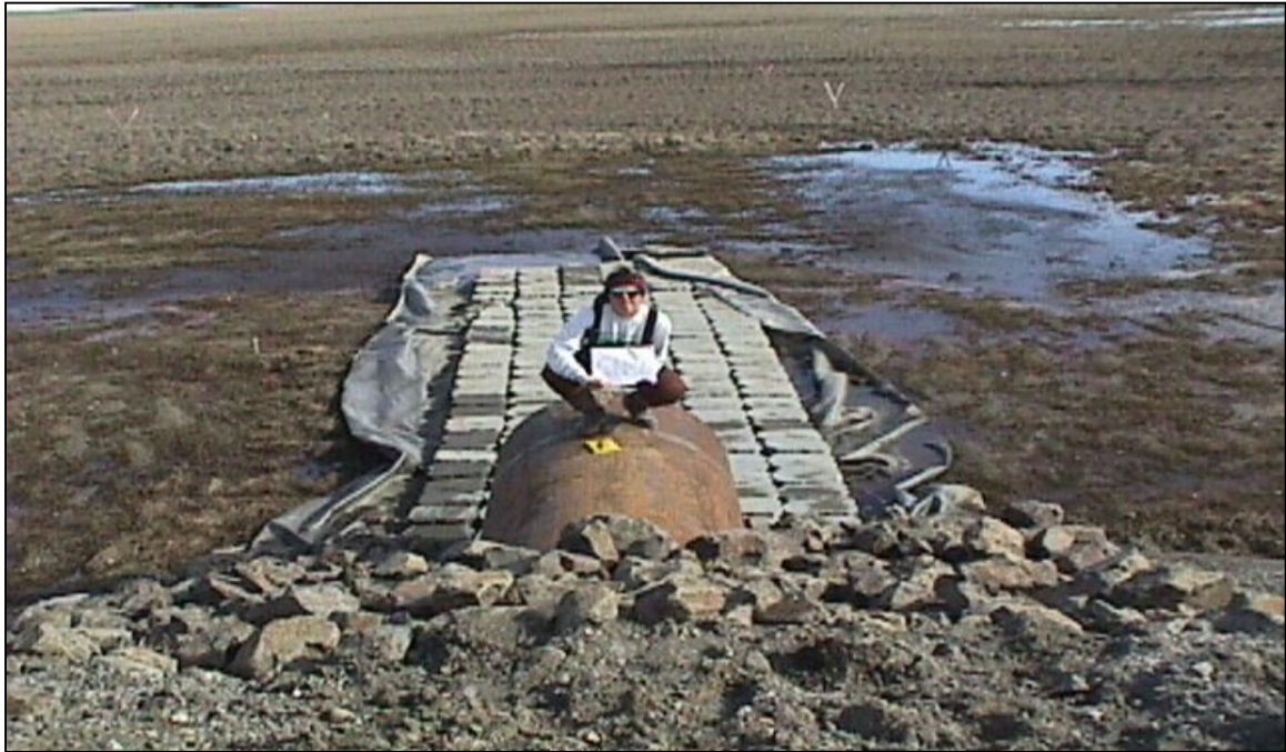
CN-1: Looking north at the north end of the culvert. (6/18/00)
