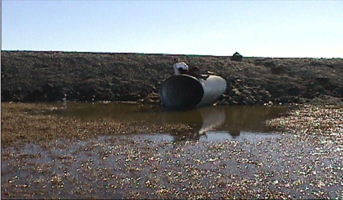
CN-14: Looking south at the north end of the culvert. (6/17/00)
