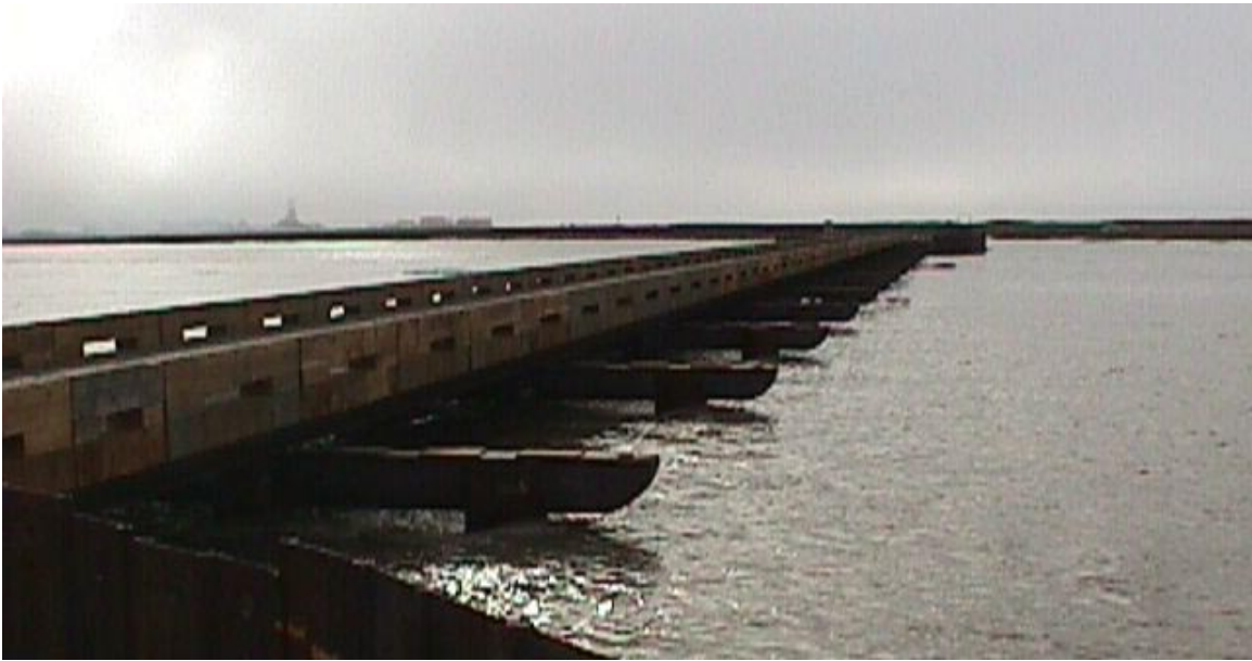
Up-stream side of the Large (East) Bridge taken from the West abutment on the CD-2 access road looking Northeast, on 12-Jun-00.
