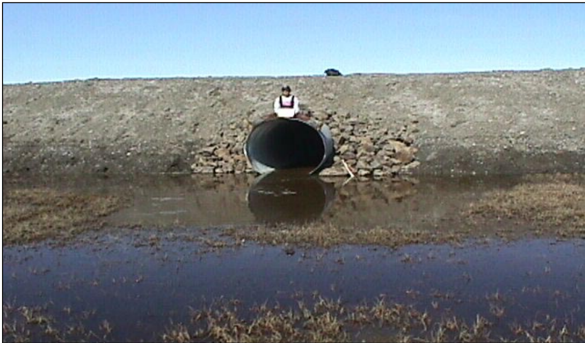
CS-16: Looking north at the south end of the culvert. (6/17/00)
