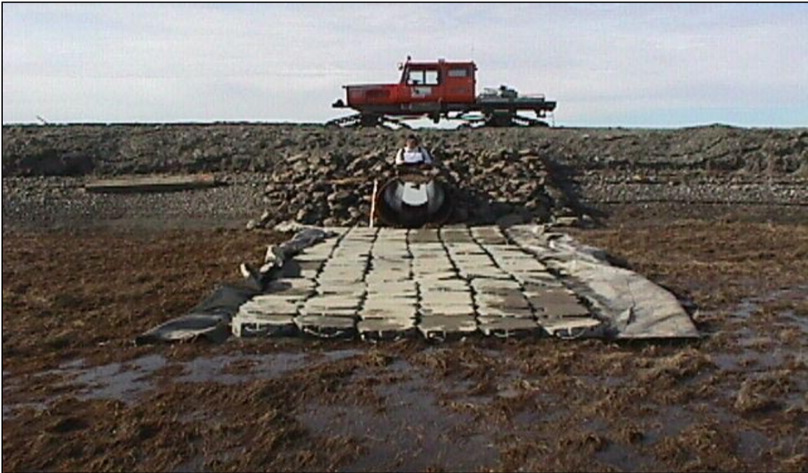
CN-2: Looking south at the north end of the culvert. (6/18/00)
