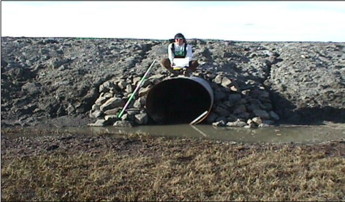
CN-8: Looking south at the north end of the culvert. (6/18/00)
