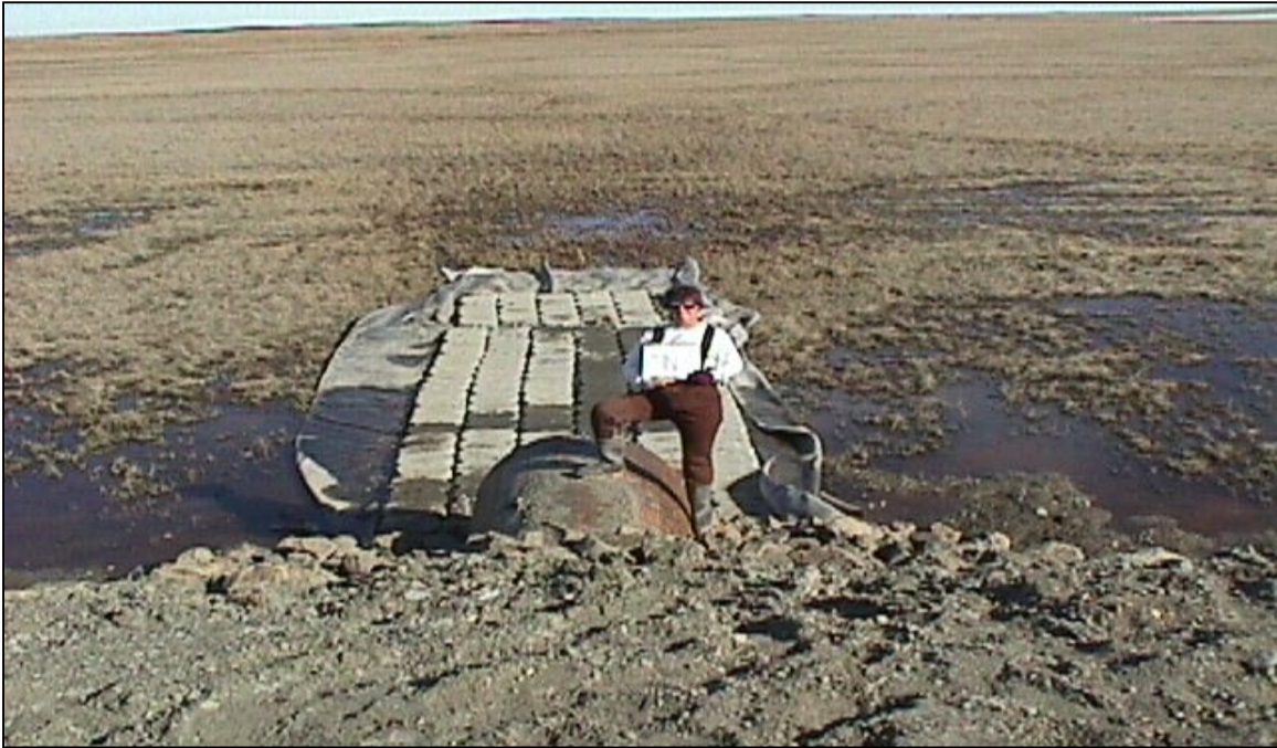
CN-4: Looking north at the north end of the culvert. (6/18/00)
