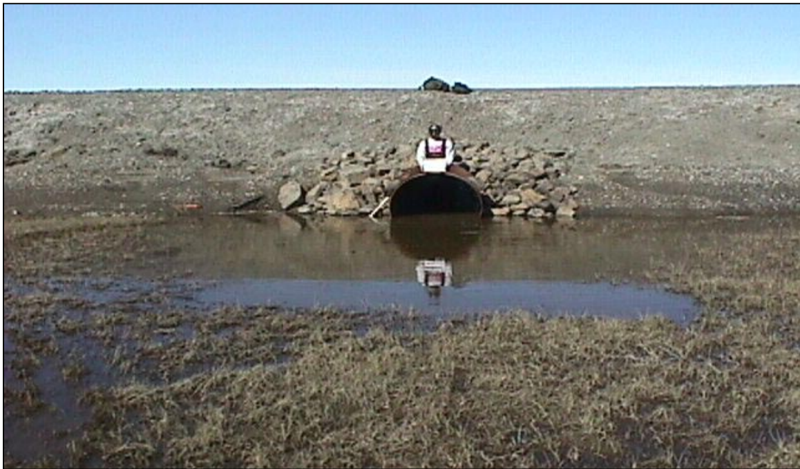
CS-17: Looking north at the south end of the culvert. (6/17/00)
