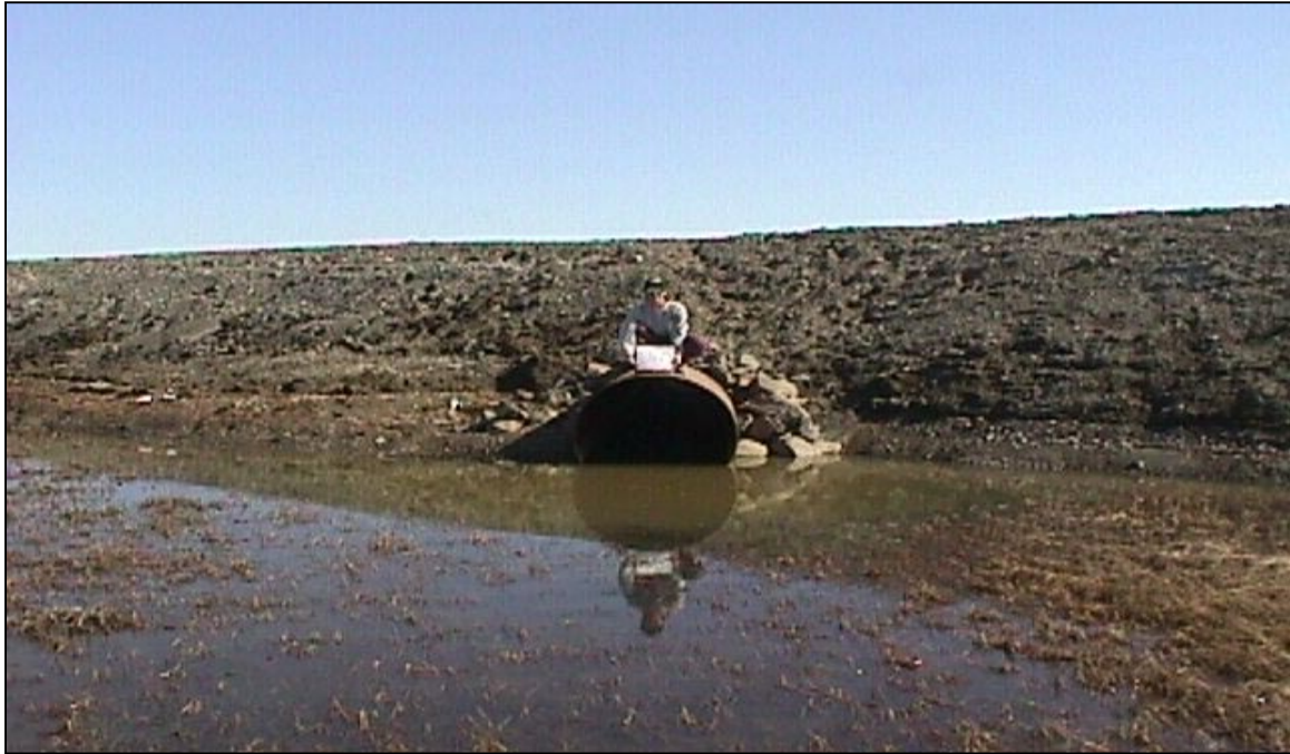
CN-24: Looking south at the north end of the culvert. (6/15/00)
