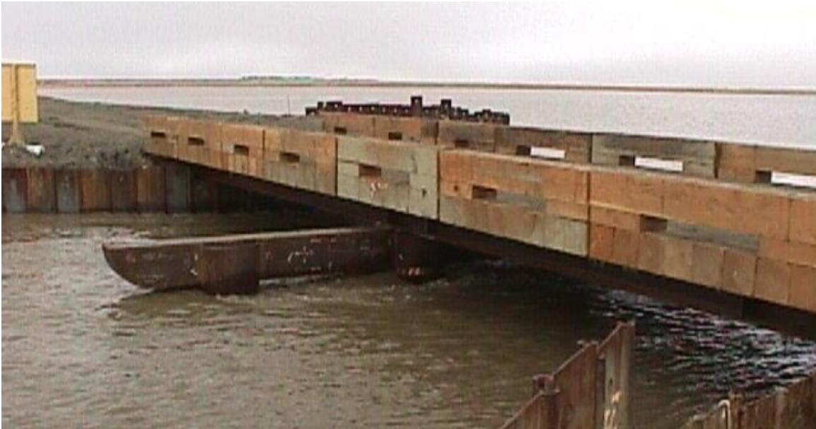
Up-stream side of the Small (West) Bridge taken from the East abutment on the CD-2 access road looking Northwest, on 12-Jun-00.
