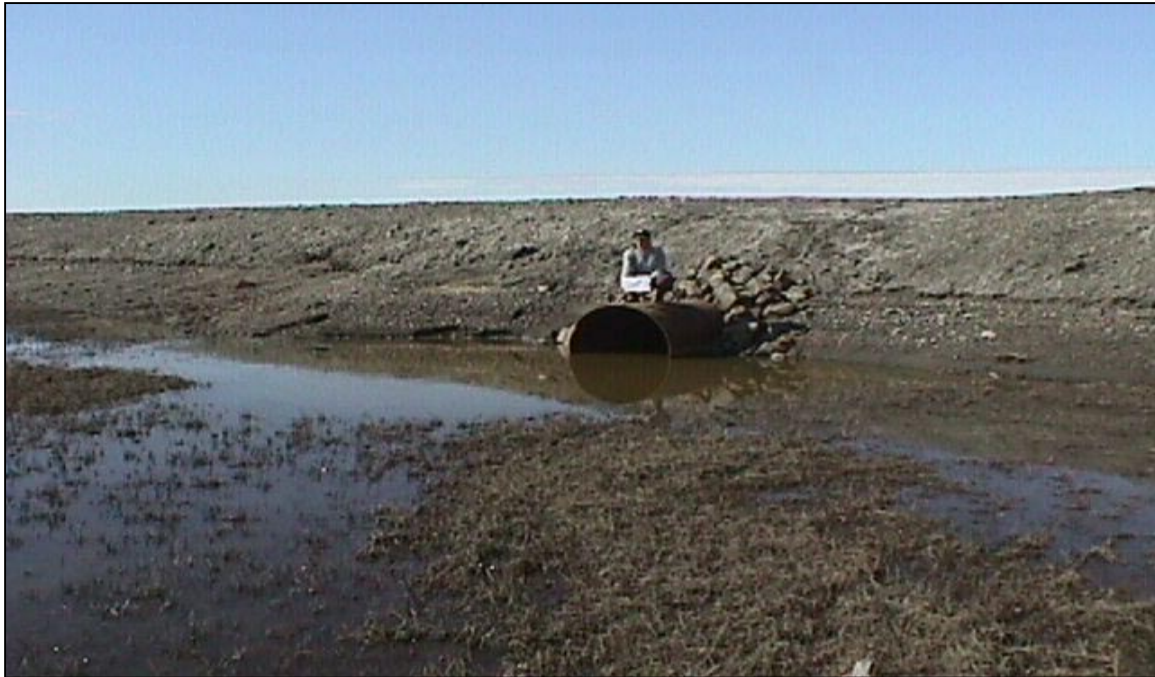
CS-22: Looking north at the south end of the culvert. (6/15/00)
