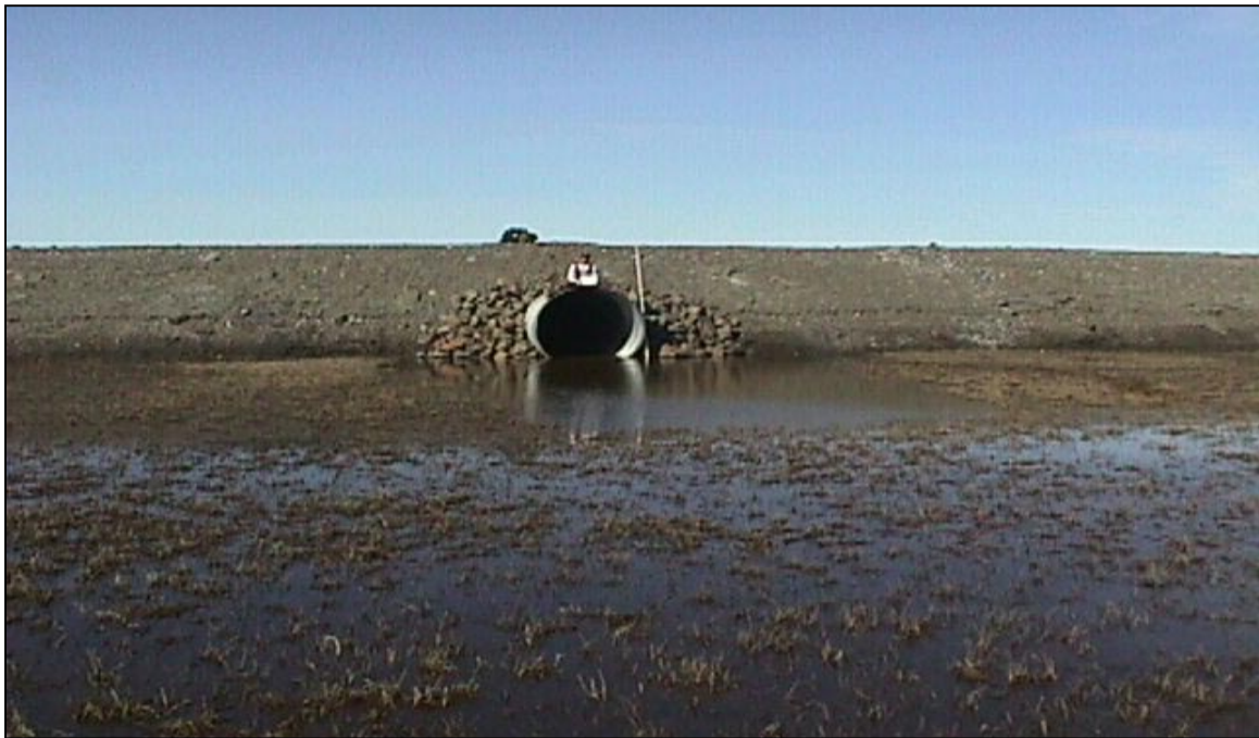
CS-13: Looking north at the south end of the culvert. (6/17/00)
