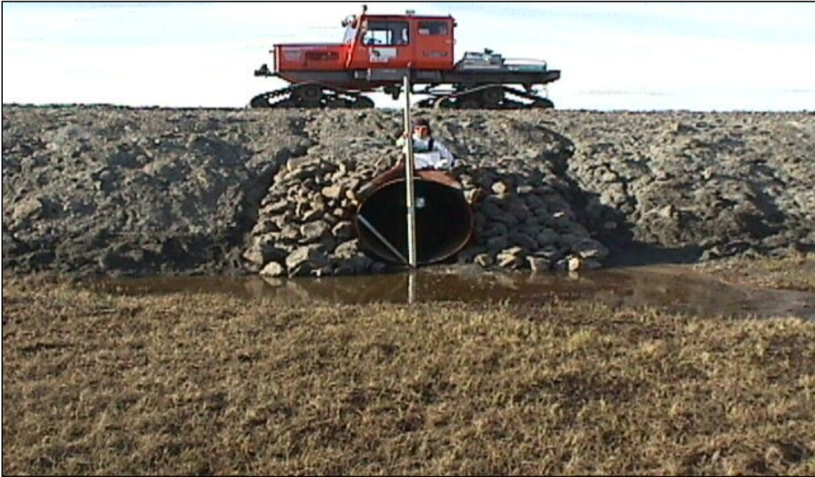
CN-9: Looking south at the north end of the culvert. (6/18/00)
