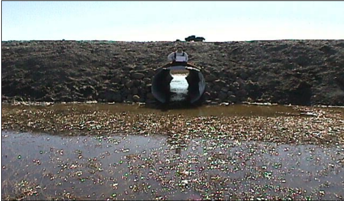
CN-16: Looking south at the north end of the culvert. (6/17/00)
