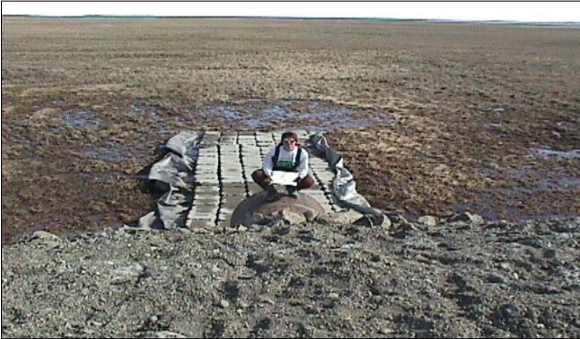
CN-2: Looking north at the north end of the culvert. (6/18/00)
