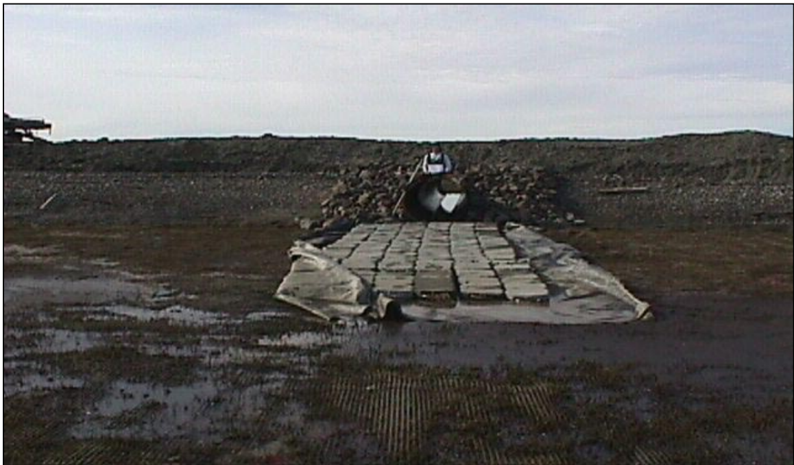
CN-1: Looking south at the north end of the culvert. (6/18/00)
