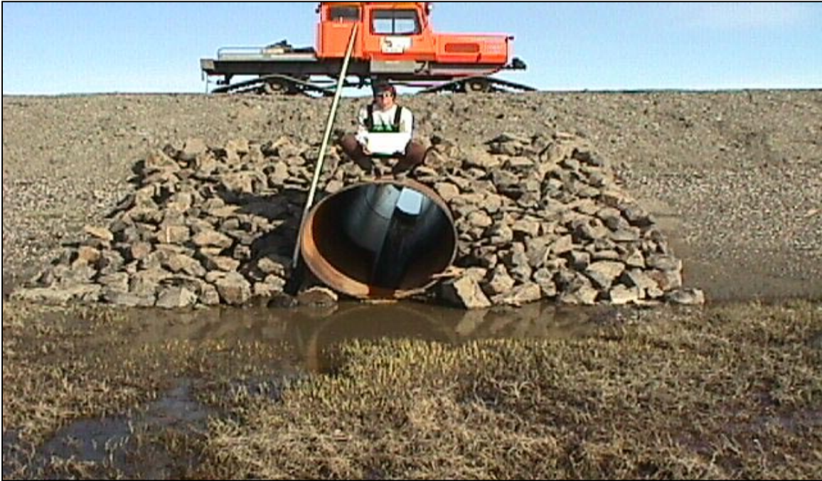
CS-4: Looking north at the south end of the culvert. (6/18/00)
