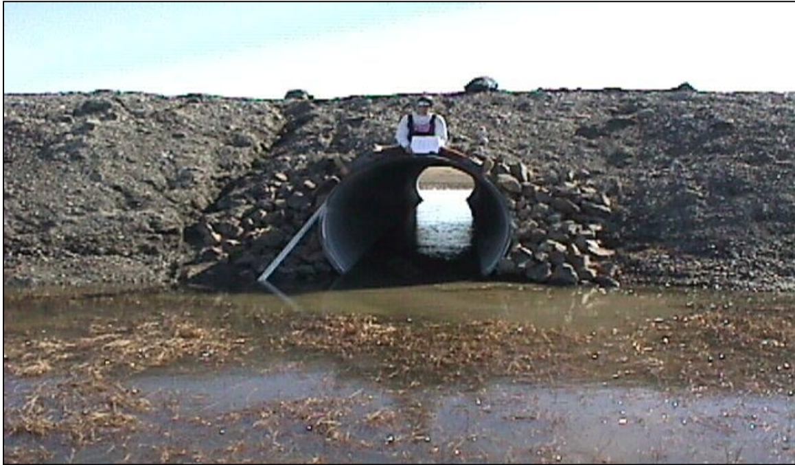
CN-13: Looking south at the north end of the culvert. (6/17/00)
