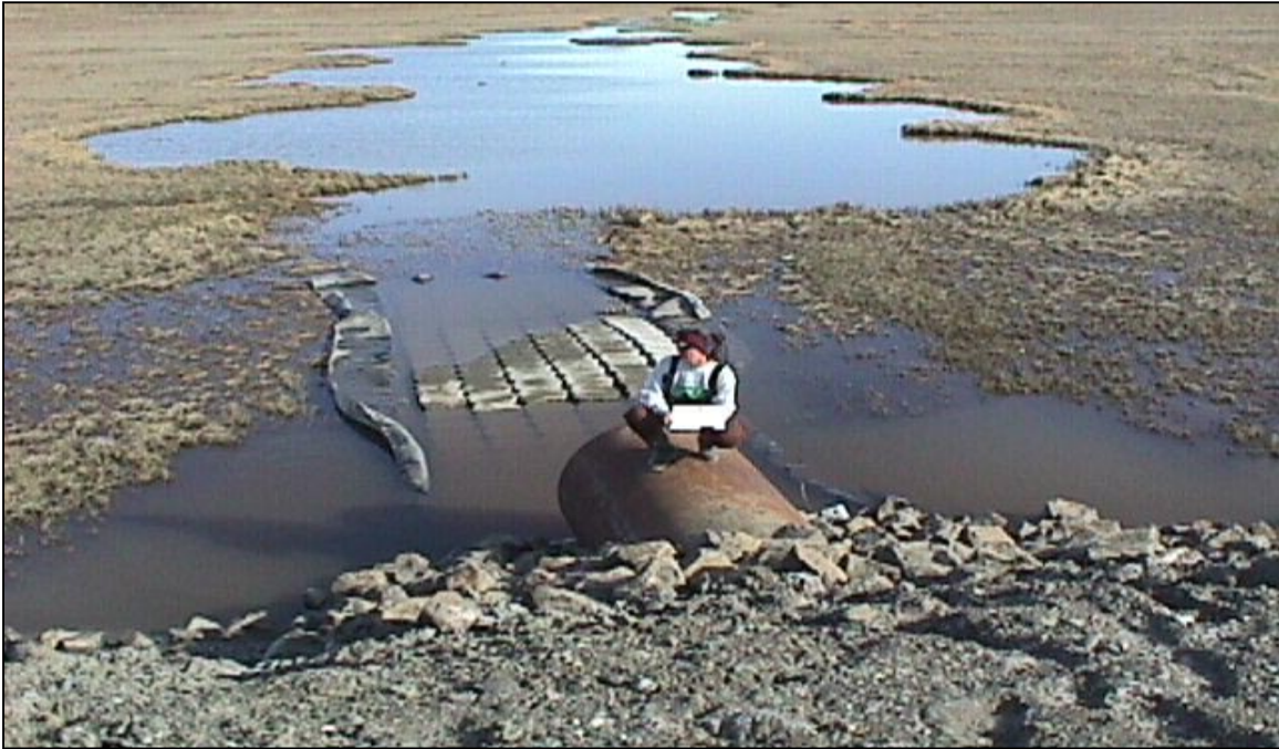
CN-5: Looking north at the north end of the culvert. (6/18/00)
