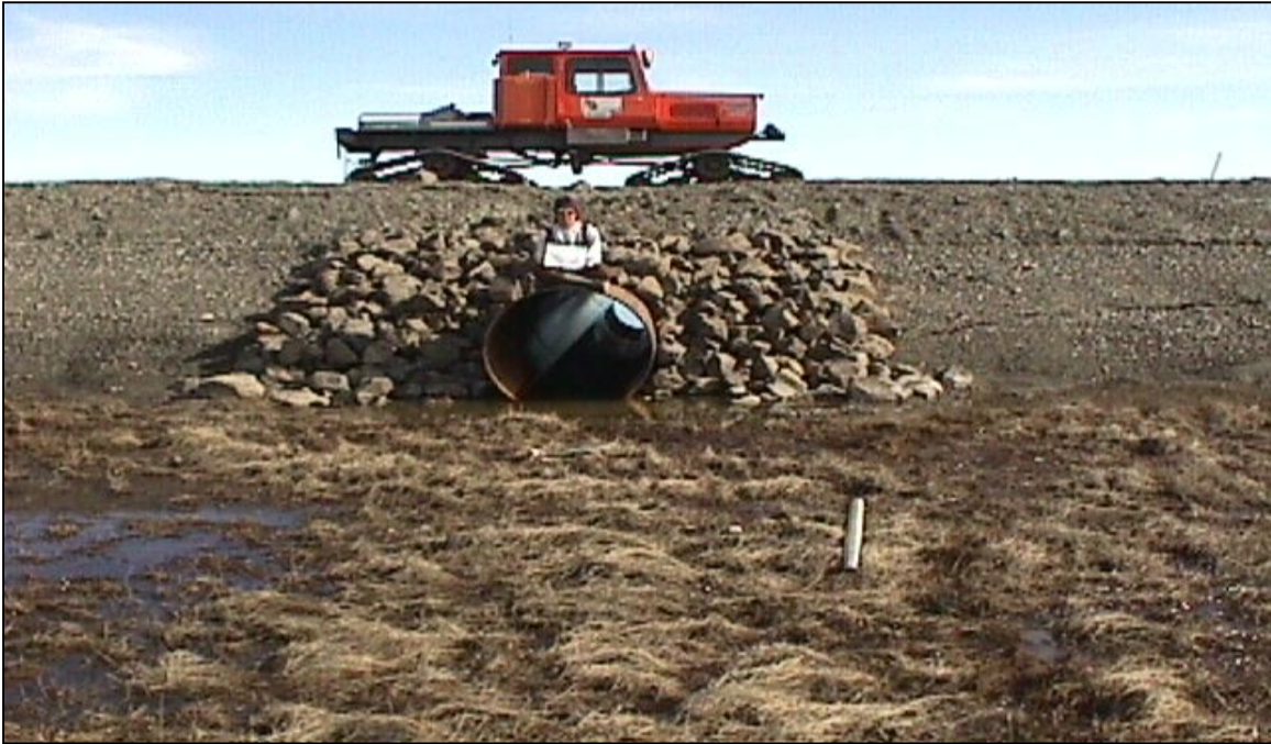
CS-2: Looking north at the south end of the culvert. (6/18/00)
