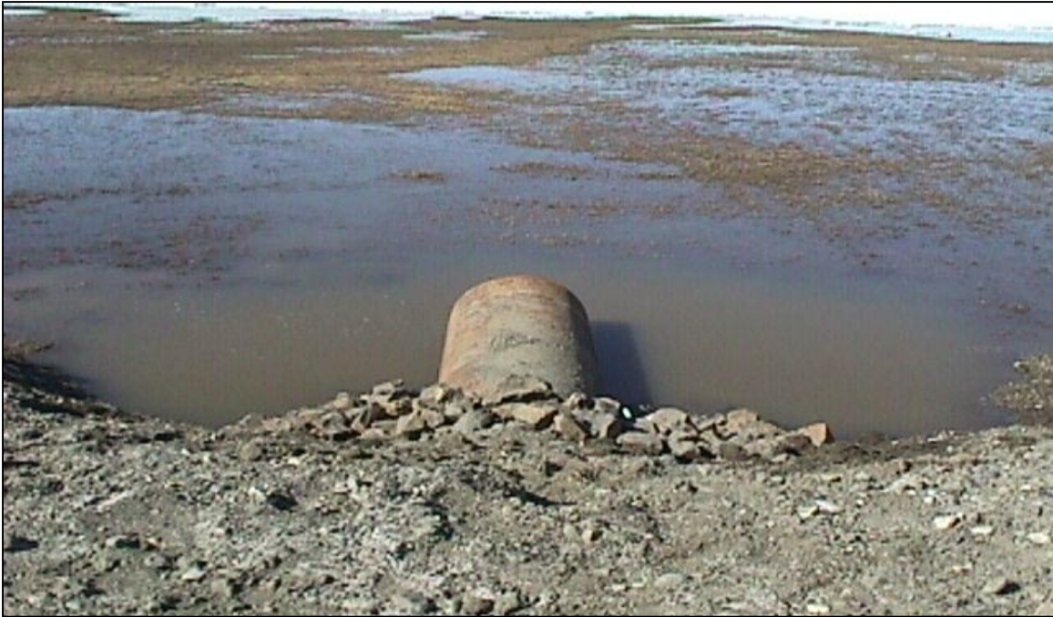
CN-22: Looking north at the north end of the culvert. (6/15/00)
