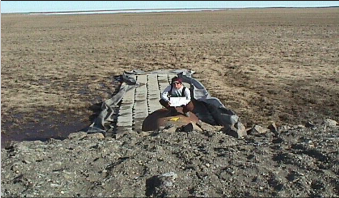
CN-3: Looking north at the north end of the culvert. (6/18/00)
