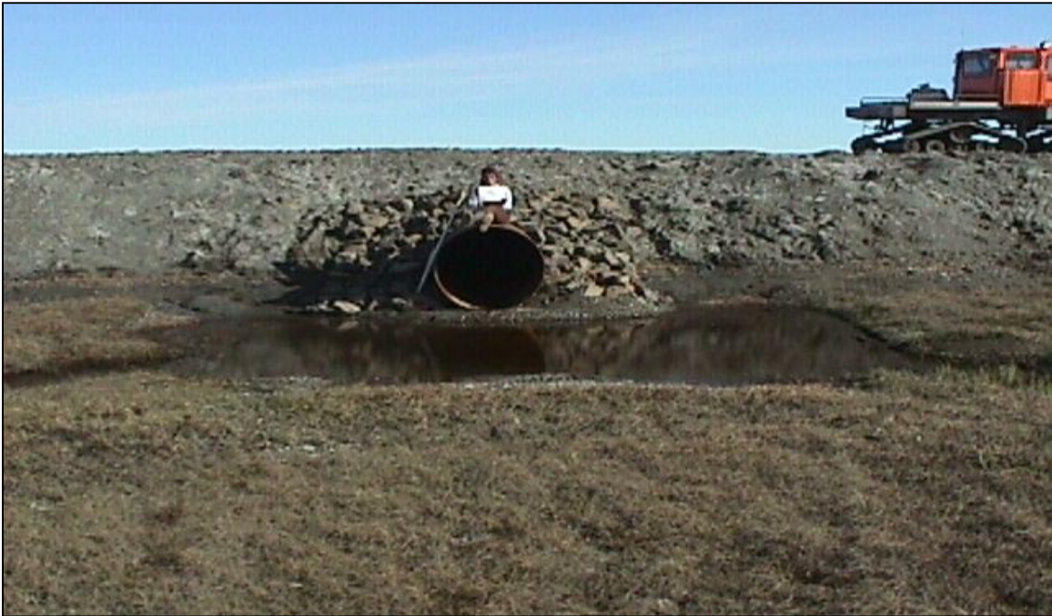
CS-6: Looking north at the south end of the culvert. (6/18/00)
