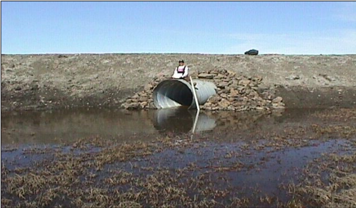
CS-15: Looking north at the south end of the culvert. (6/17/00)
