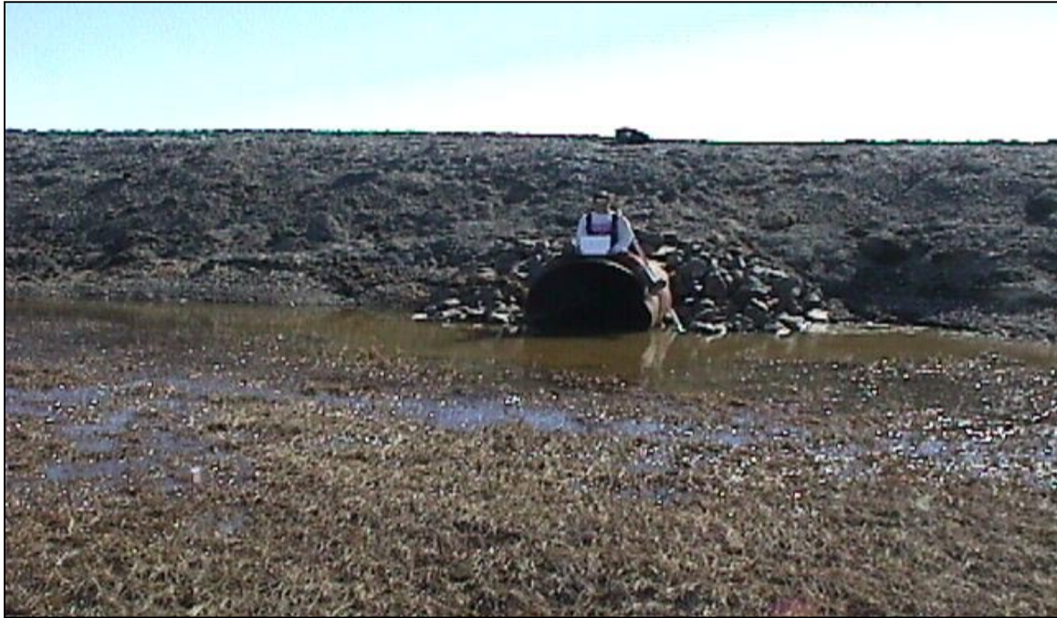
CN-17: Looking south at the north end of the culvert. (6/17/00)
