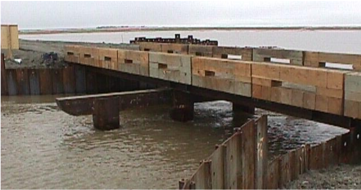
Up-stream side of the Small (West) Bridge taken from the East abutment on the CD-2 access road looking Northwest, on 10-Jun-00.
