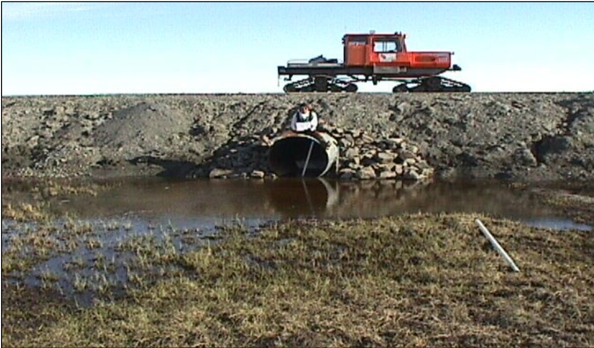
CS-9: Looking north at the south end of the culvert. (6/18/00)
