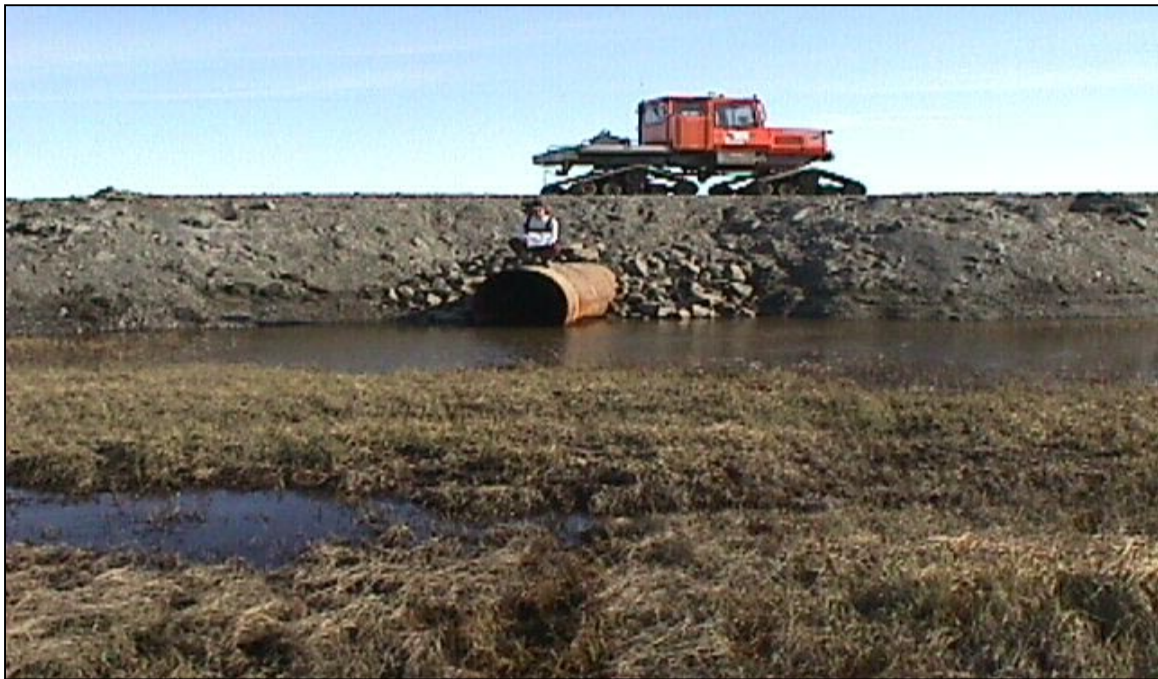
CS-7: Looking north at the south end of the culvert. (6/18/00)
