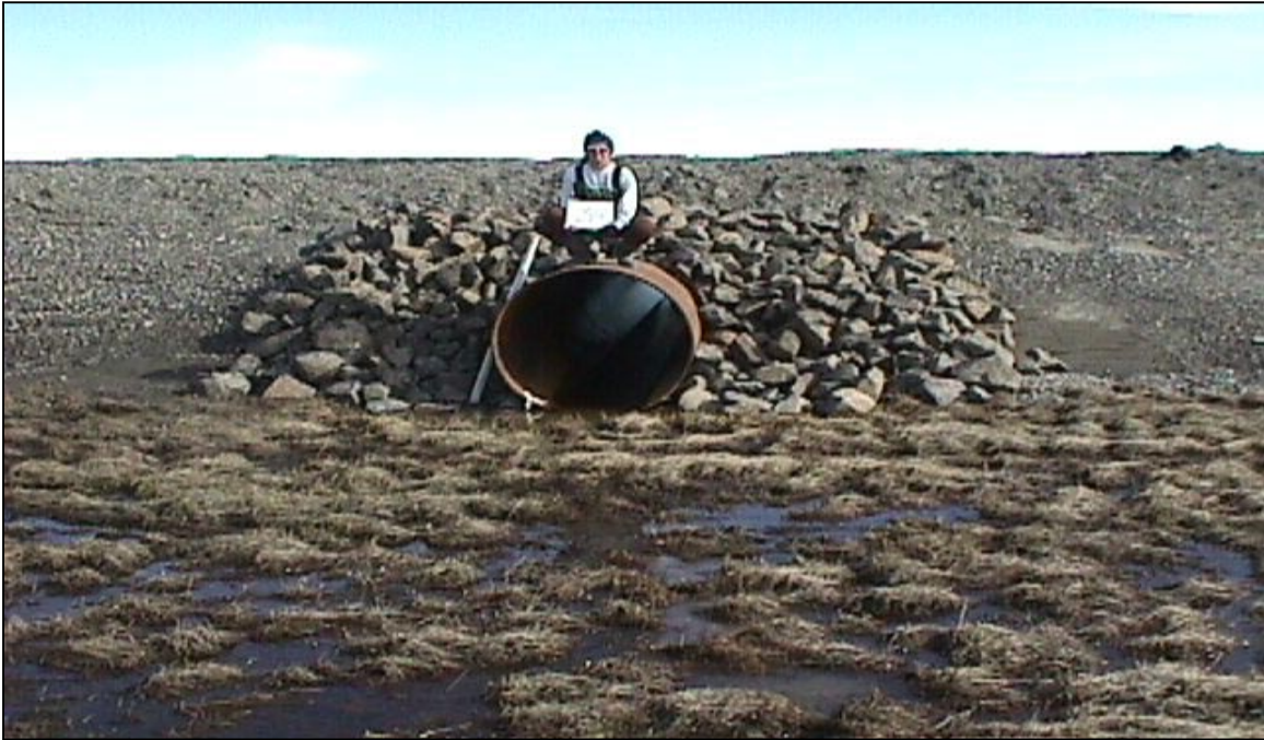
CS-1: Looking north at the south end of the culvert. (6/18/00)
