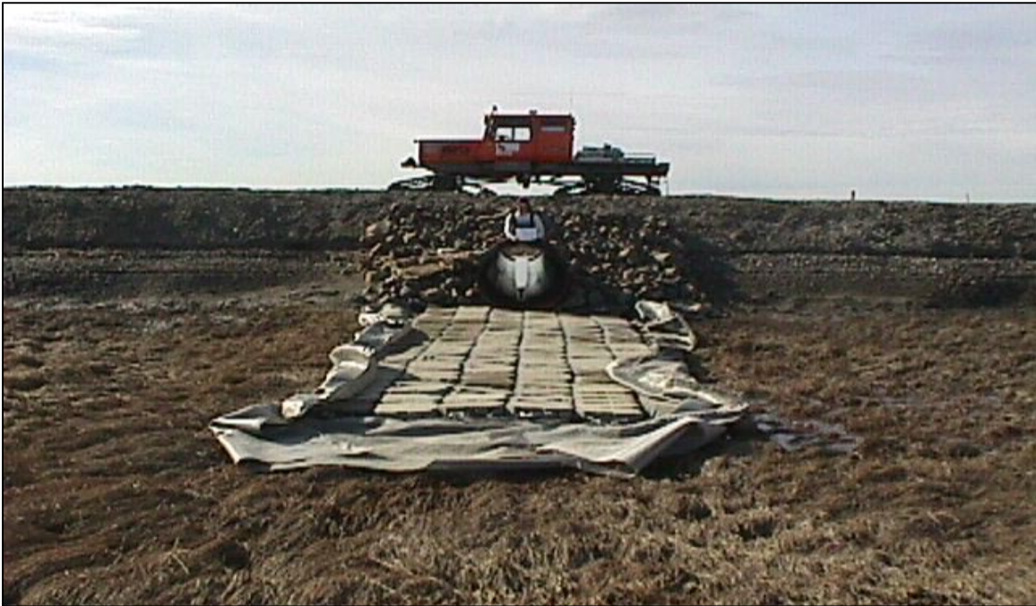
CN-3: Looking south at the north end of the culvert. (6/18/00)
