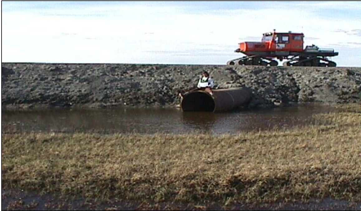
CN-7: Looking south at the north end of the culvert. (6/18/00)
