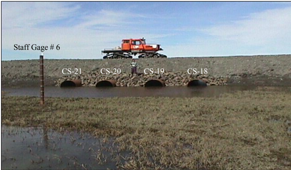
CS-21, CS-20, CS-19, CS-18: Looking north at the south end of the culverts. Staff gage #6 is on the left side of the picture. (6/19/00)
