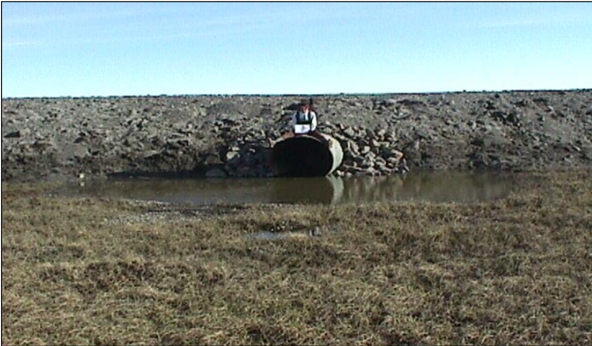
CS-8: Looking north at the south end of the culvert. (6/18/00)
