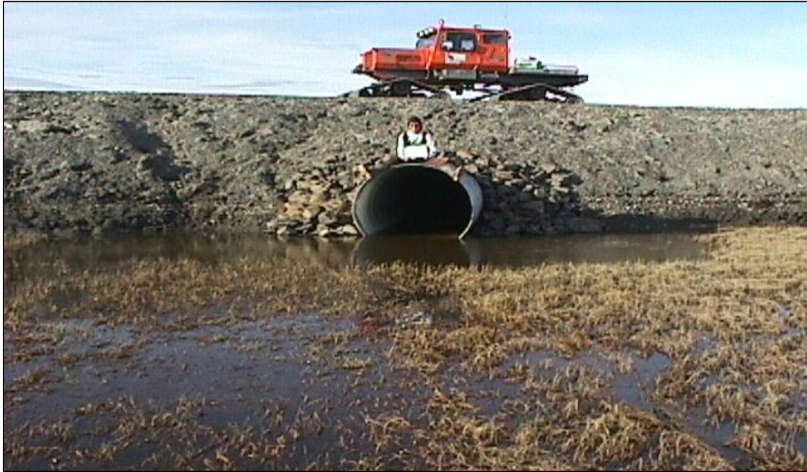
CN-11: Looking south at the north end of the culvert. (6/18/00)
