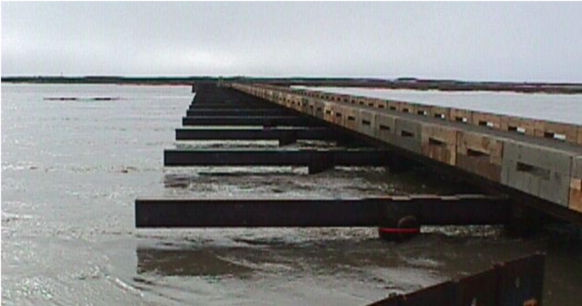
Down-stream side of the Large (East) Bridge taken from the West abutment on the CD-2 access road looking East, on 12-Jun-00.
