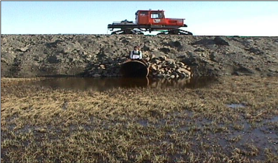
CS-10: Looking north at the south end of the culvert. (6/18/00)
