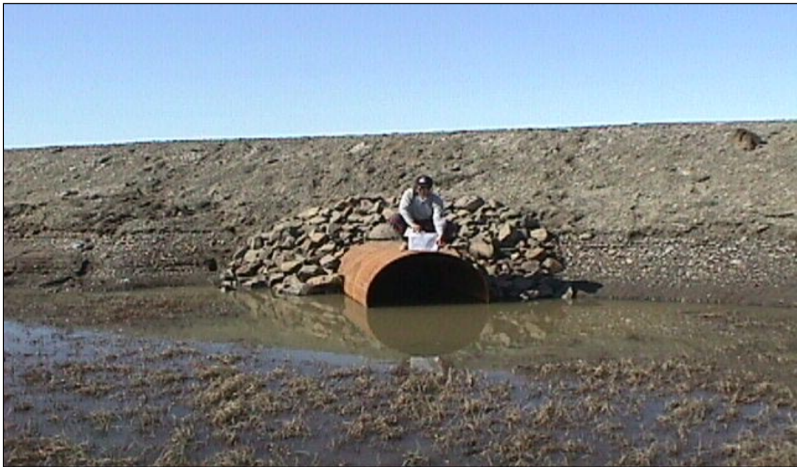
CN-24: Looking north at the south end of the culvert. (6/15/00)
