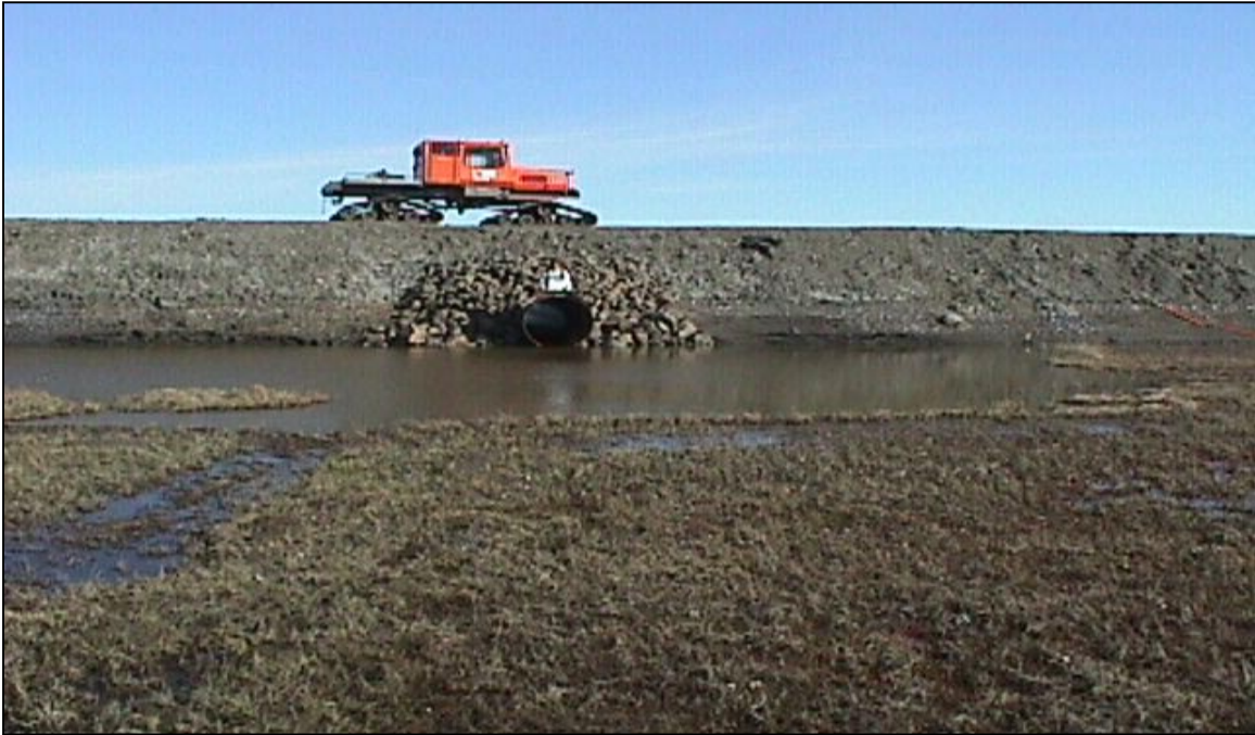
CS-5: Looking north at the south end of the culvert. (6/18/00)
