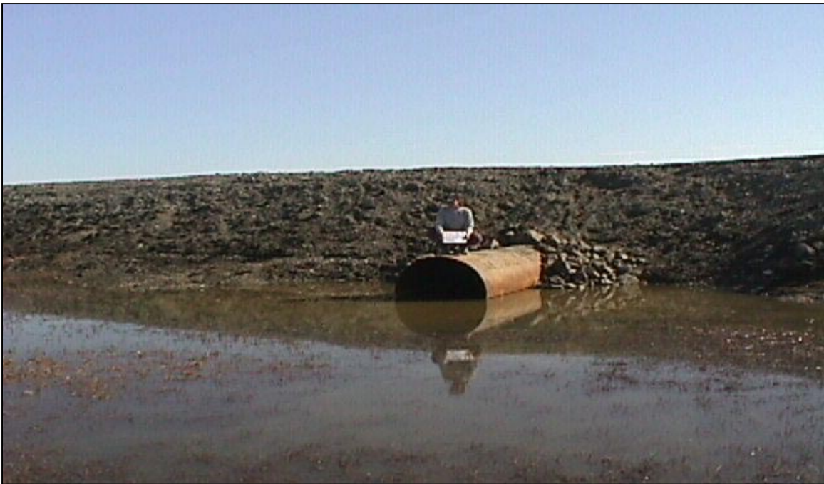
CN-22: Looking south at the north end of the culvert. (6/15/00)
