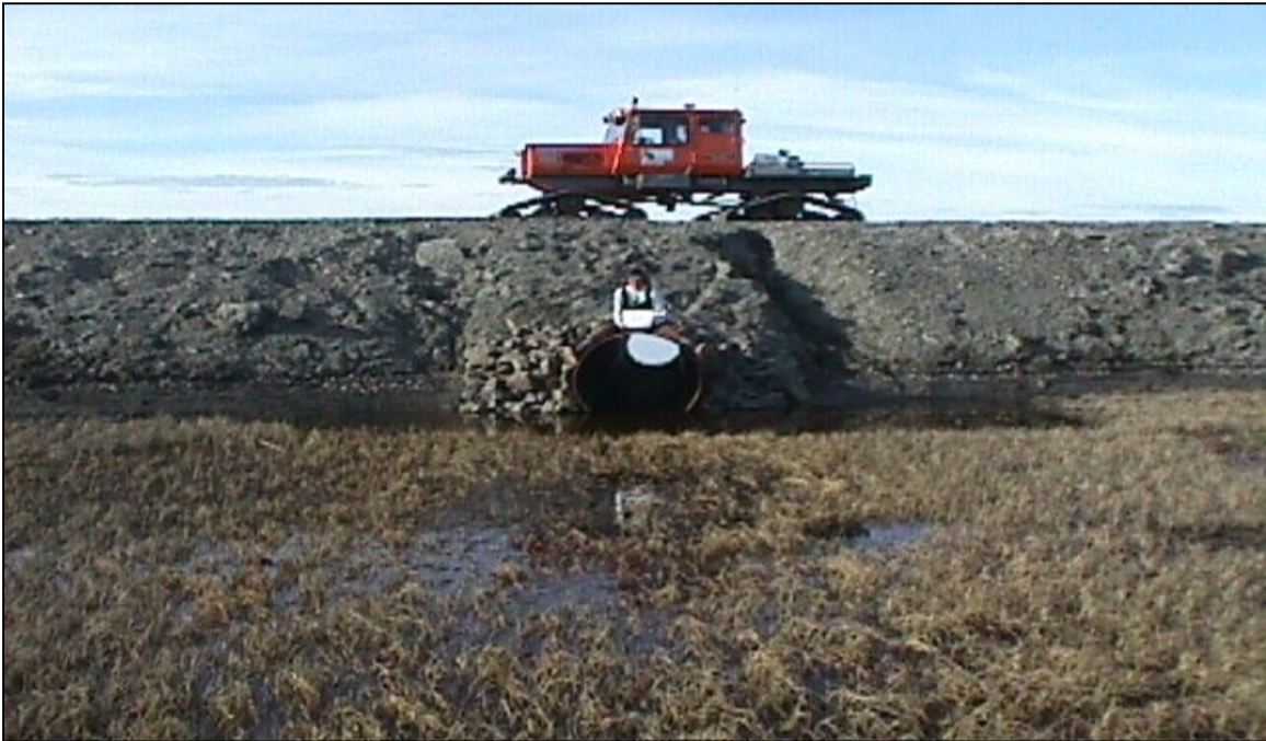
CN-10: Looking south at the north end of the culvert. (6/18/00)
