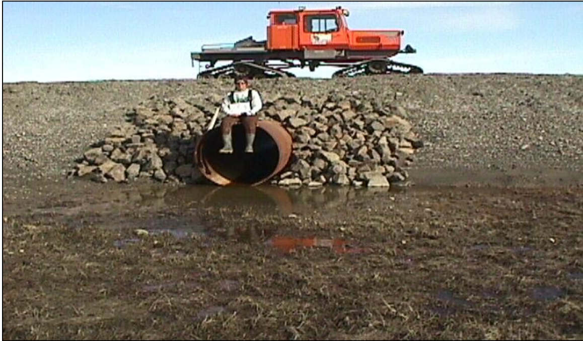
CS-3: Looking north at the south end of the culvert. (6/18/00)
