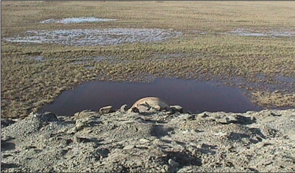
CS-10: Looking south at the south end of the culvert. (6/18/00)
