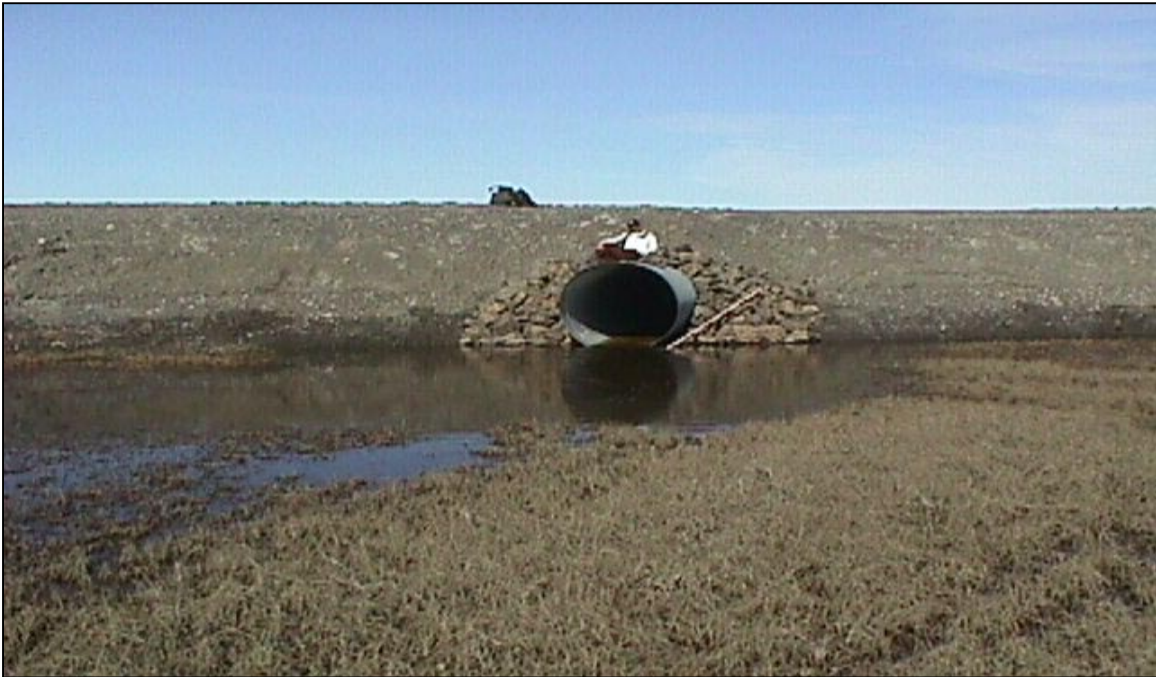
CS-14: Looking north at the south end of the culvert. (6/17/00)
