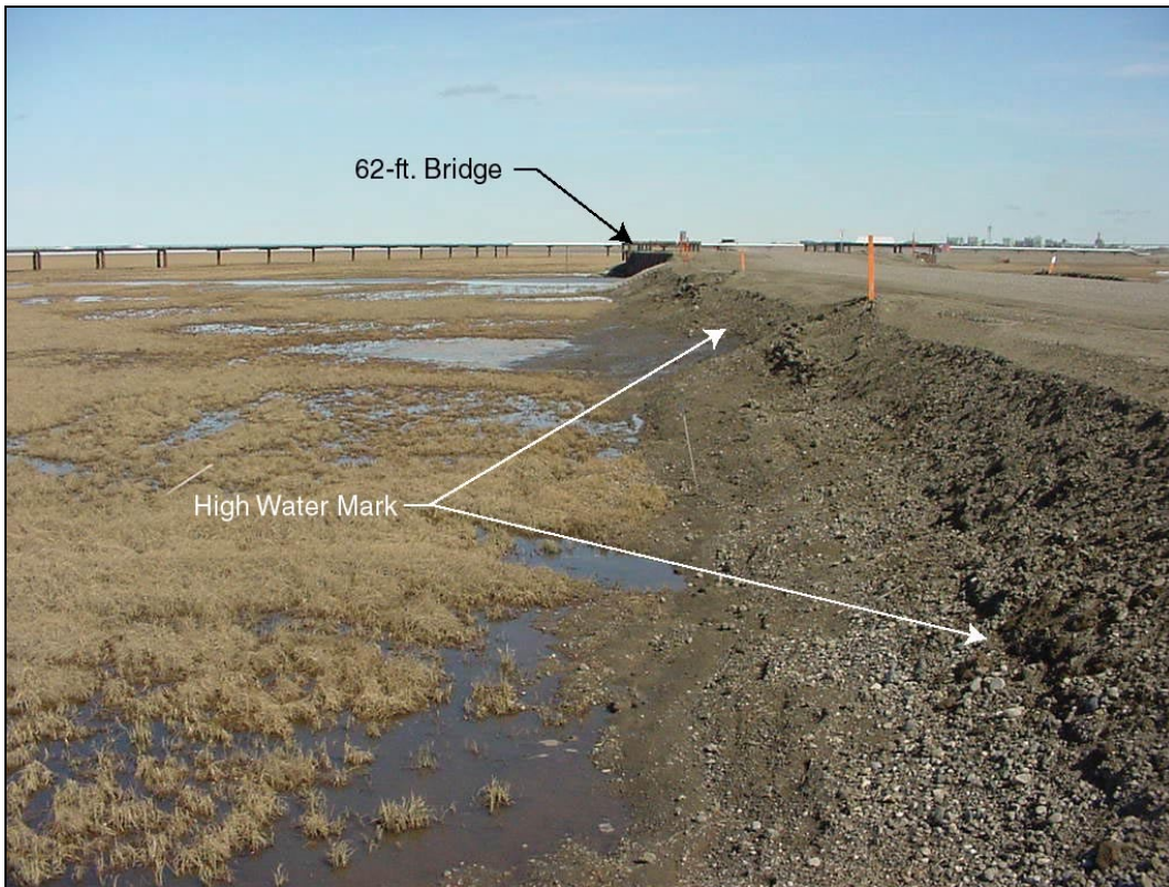
Photo 4-7 Facing east from Culvert #04 along the north side of the CD-2 access road. Photo taken June 16, 2001.
