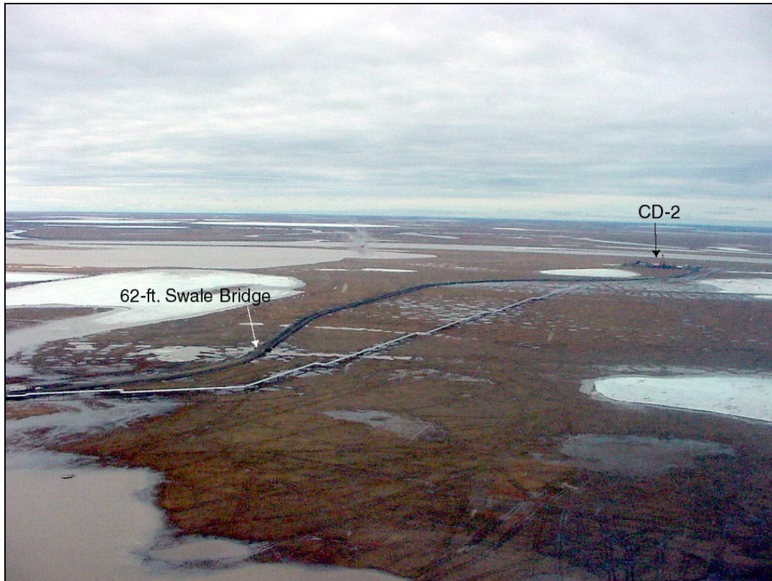
Photo 2-3 b Flooding Conditions at Alpine June 14, 2001, looking west.
