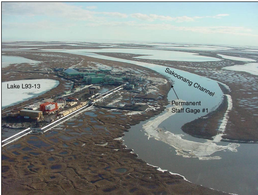
Photo 2-1 b Flooding Conditions at Alpine June 11, 2001, looking north at CD-1.
