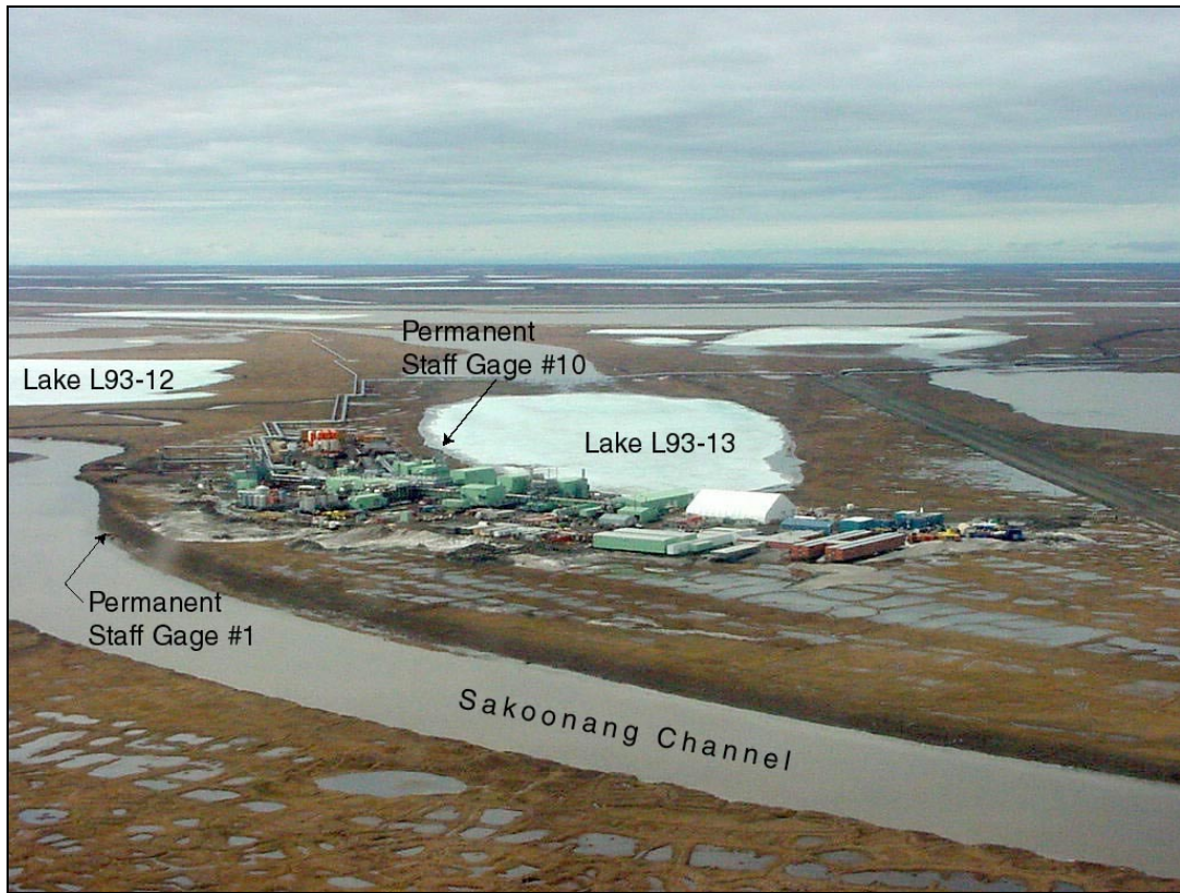
Photo 2-3 a Flooding Conditions at Alpine June 14, 2001, looking southwest.
