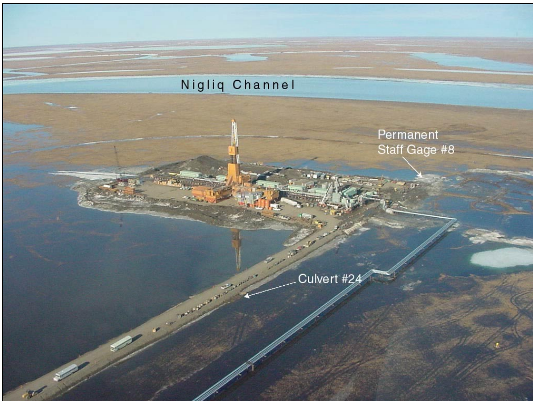
Photo 2-1 f Flooding Conditions at Alpine June 11, 2001, looking southwest at CD-2.
