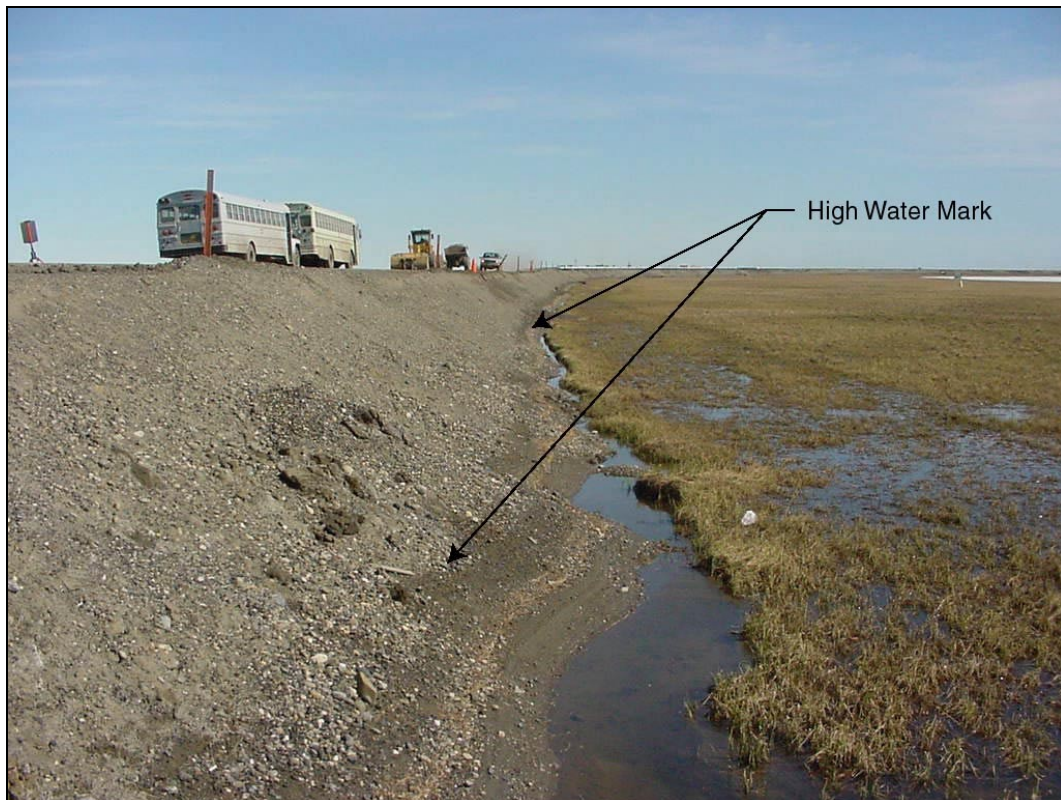
Photo 4-2 Facing east from Culvert #24 along the south side of the CD-2 access road. Photo taken June 16, 2001.
