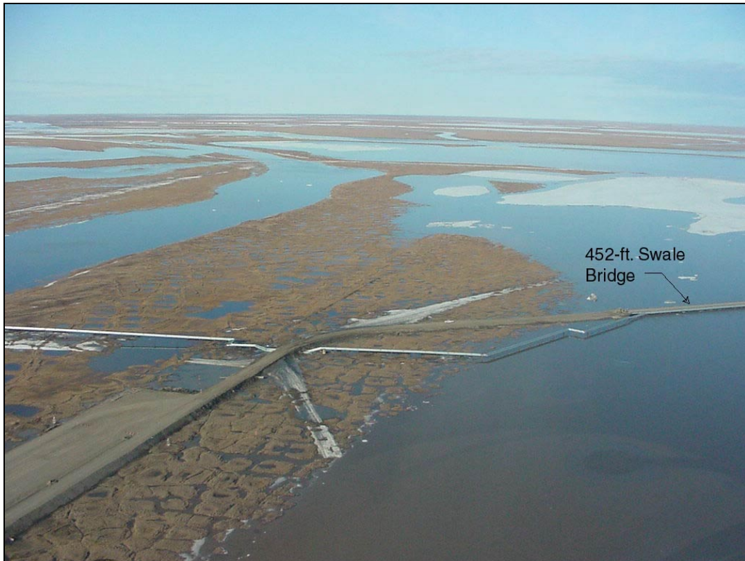
Photo 2-1 c Flooding Conditions at Alpine June 11, 2001, looking south-southwest at the end of the airstrip.
