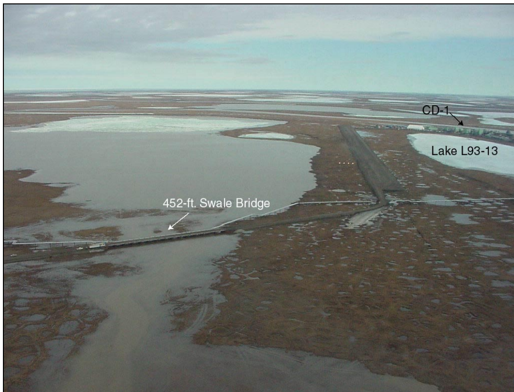
Photo 2-3 d Flooding Conditions at Alpine June 14, 2001, looking northeast at the 452-ft. swale bridge and airstrip.
