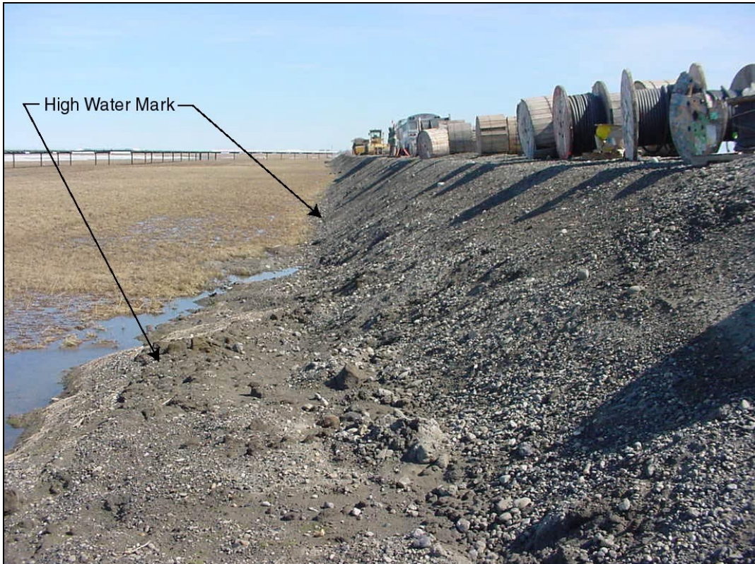
Photo 4-1 Facing east from Culvert #24 along the north side of the CD-2 access road. Photo taken June 16, 2001.
