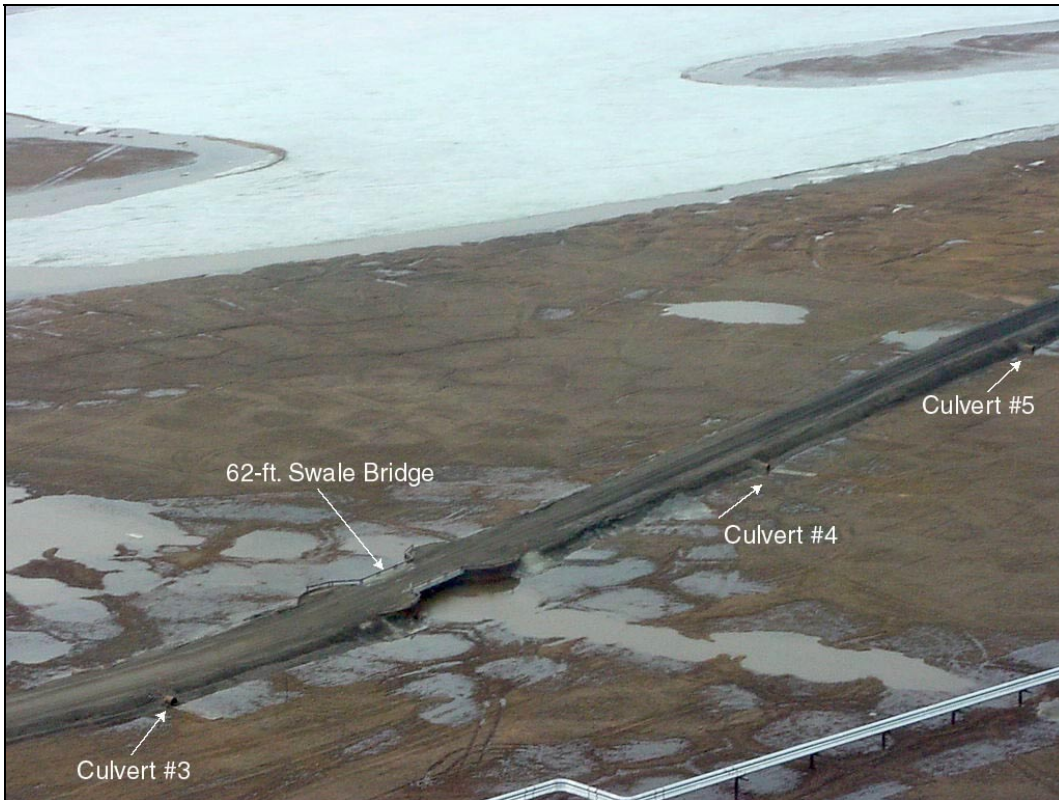
Photo 2-3 c Flooding Conditions at Alpine June 14, 2001, looking southwest at the 62-ft. swale bridge.
