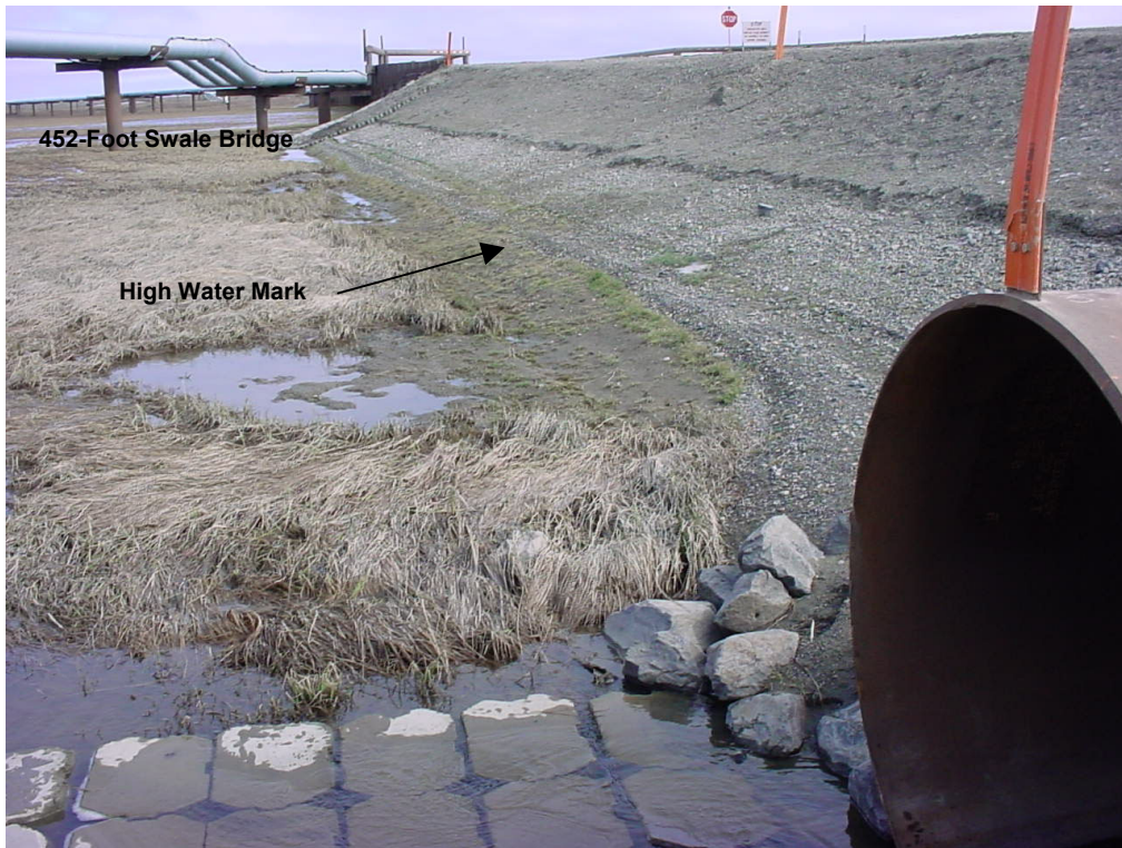
Photo 5-3 Looking east on the north side of the CD-2 access road from Culvert # 24. 13 June 2003
