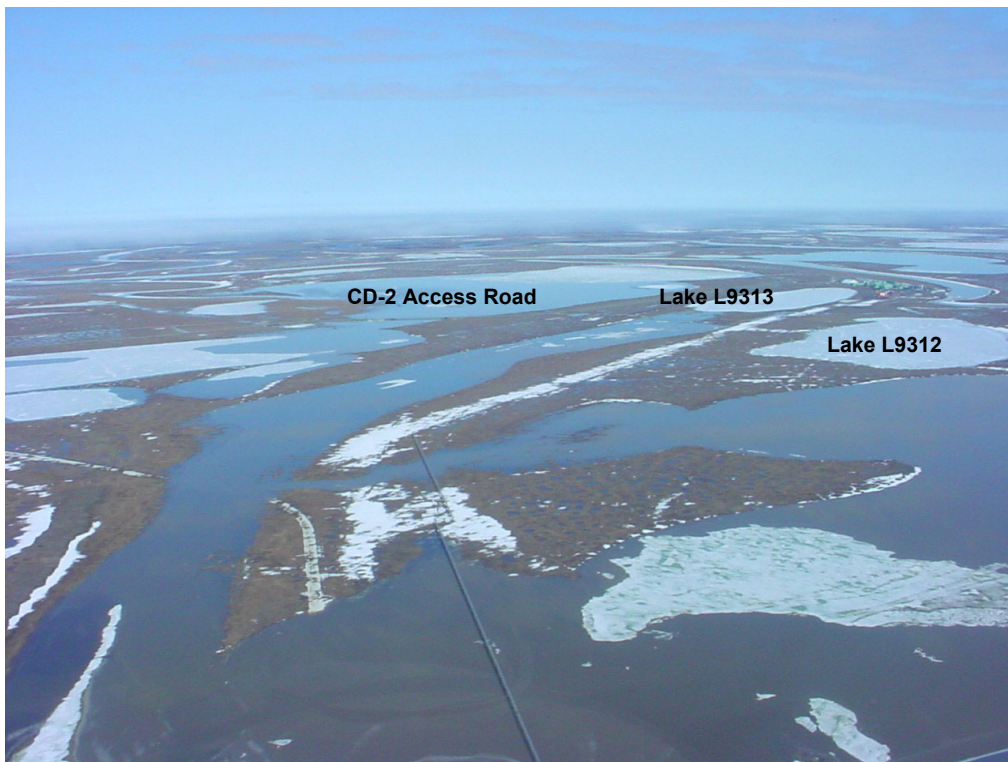
Photo 3-4 Flooding conditions at Alpine approximately 12 hours after peak flood stage. View looking north. Note that Lake L9312 is not receiving recharge from breakup flood flows.
