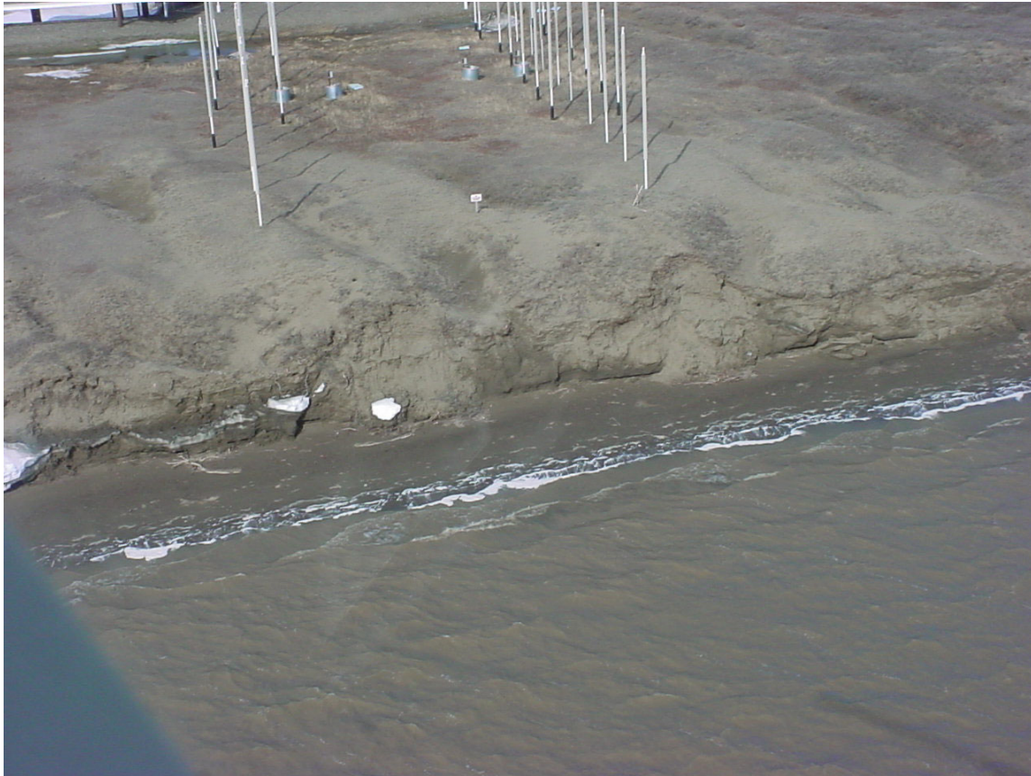
Figure 3 – Colville River HDD west bank
