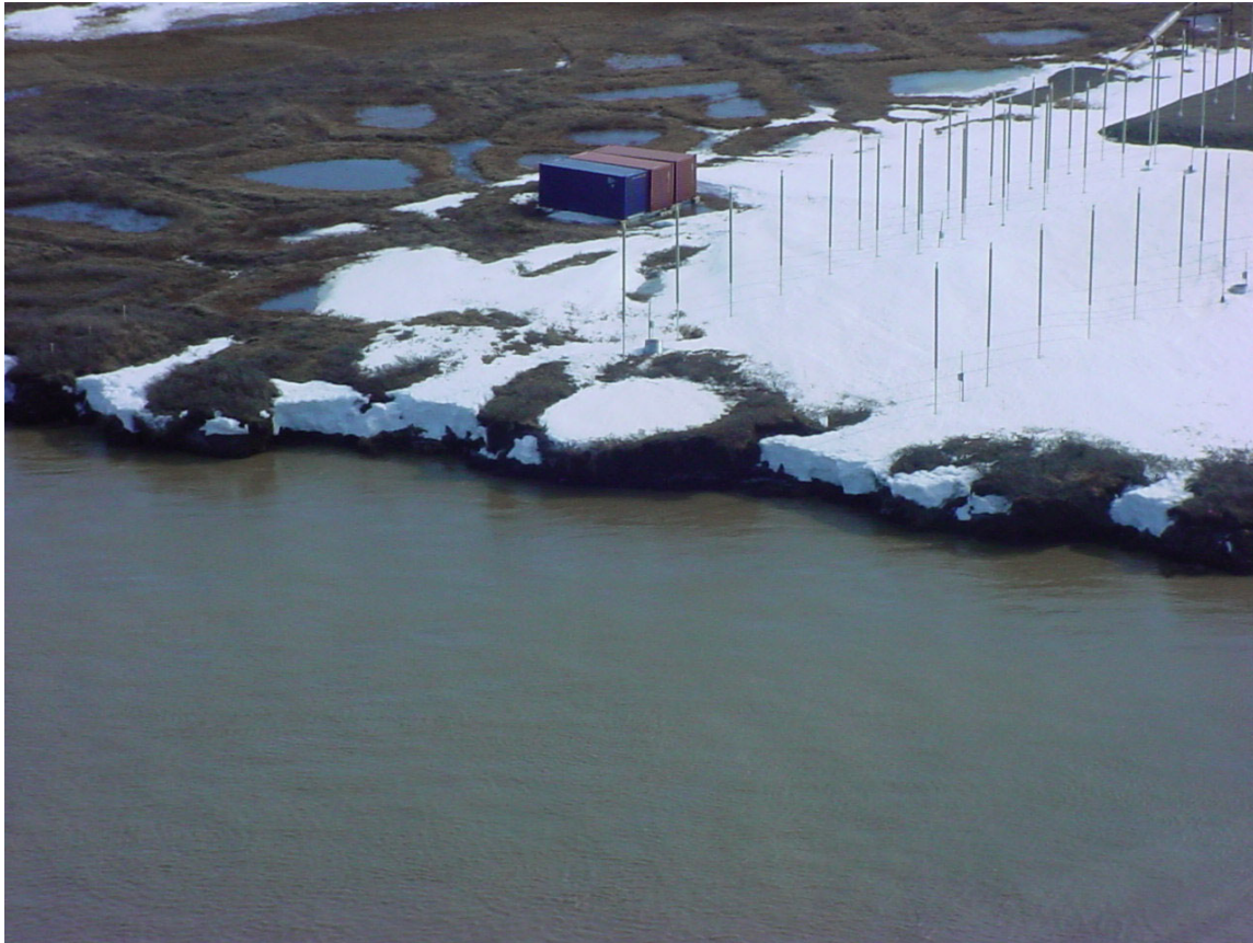
Figure 4 – Colville River HDD east bank
