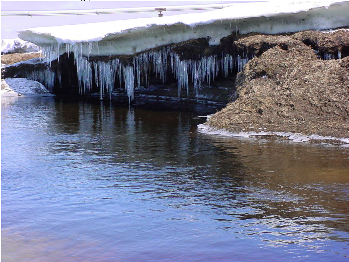
Figure 22 – Erosive damage resulting from flow directed toward the bank by a trench cut through the ice bridge, Kachemach River east bank
