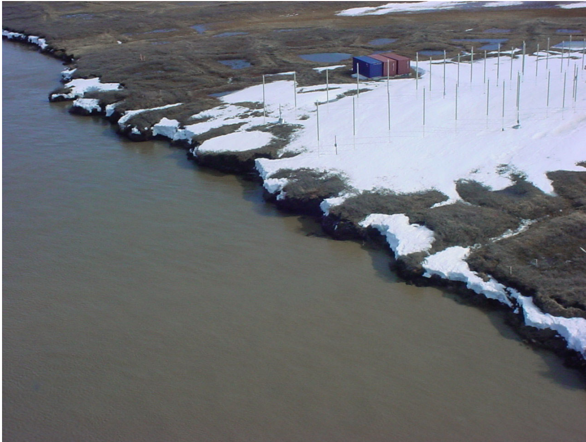
Figure 5 – Colville River HDD east bank
