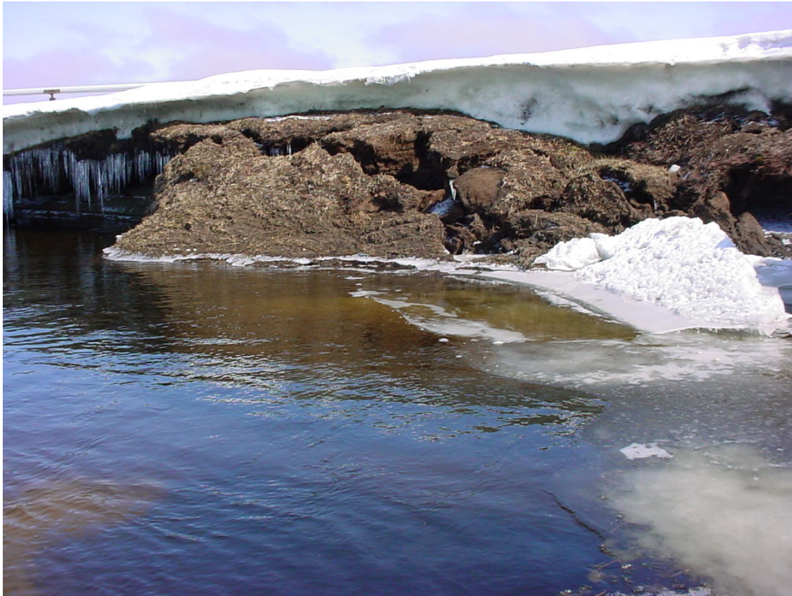
Figure 21 – Erosive damage resulting from flow directed toward the bank by a trench cut through the ice bridge, Kachemach River east bank
