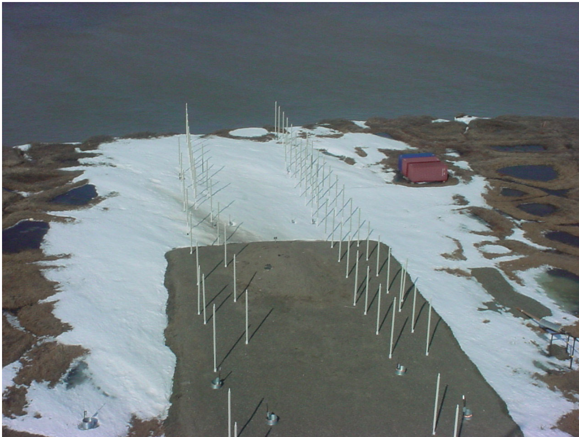
Figure 6 – Colville River HDD east bank
