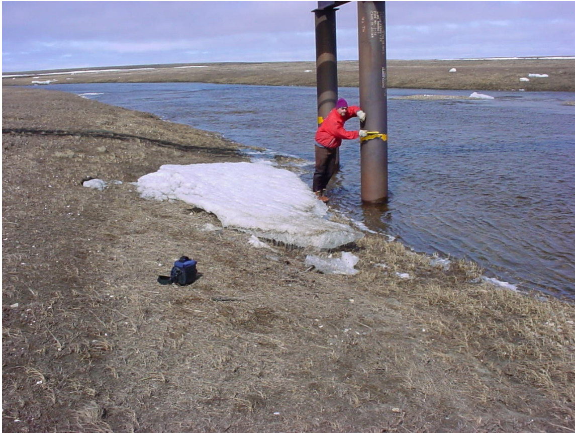
Figure 29 – Approximate high water mark on VSM 2047, Miluveach River looking downstream
