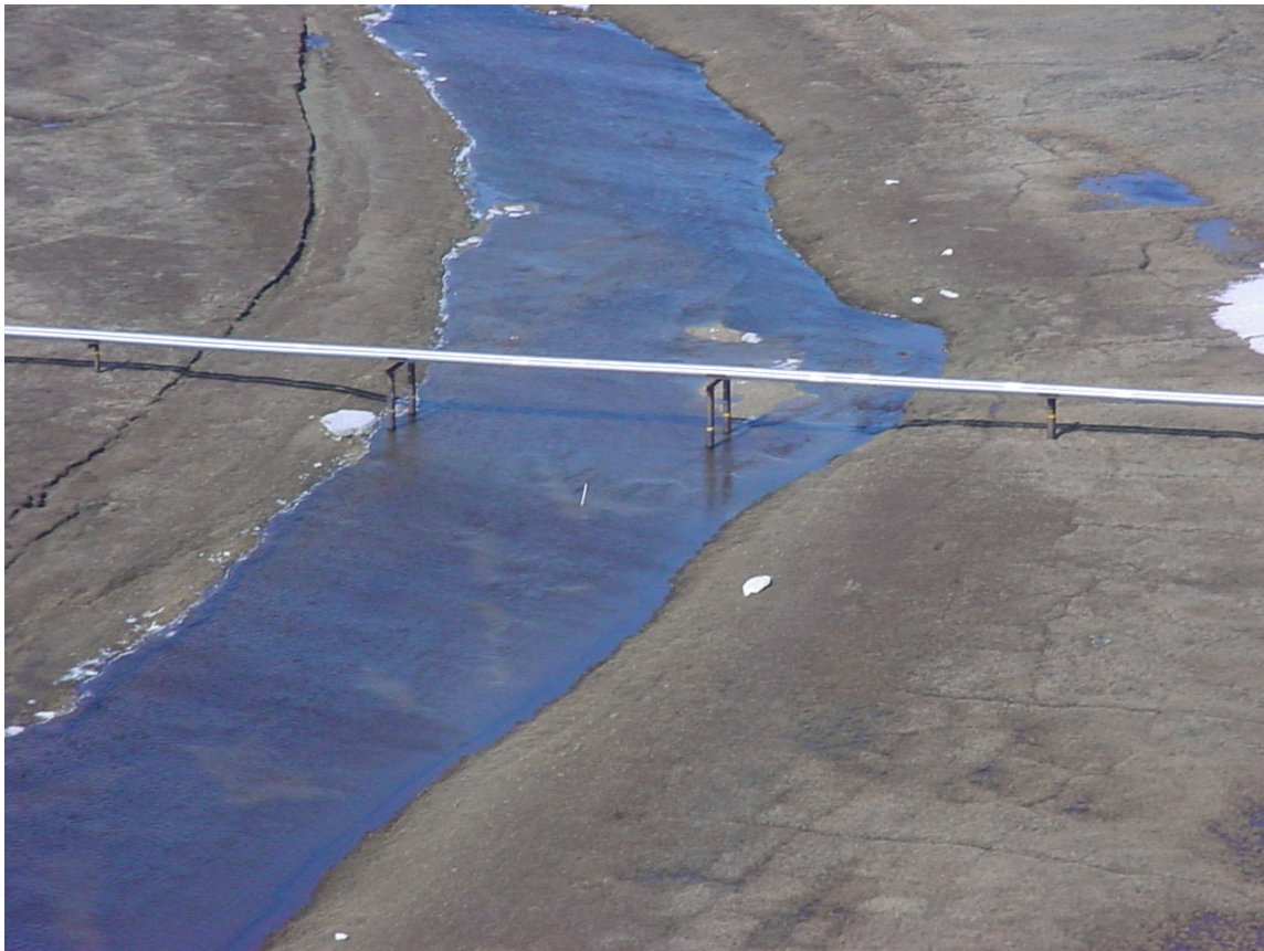
Figure 26 – Miluveach River pipeline crossing looking downstream
