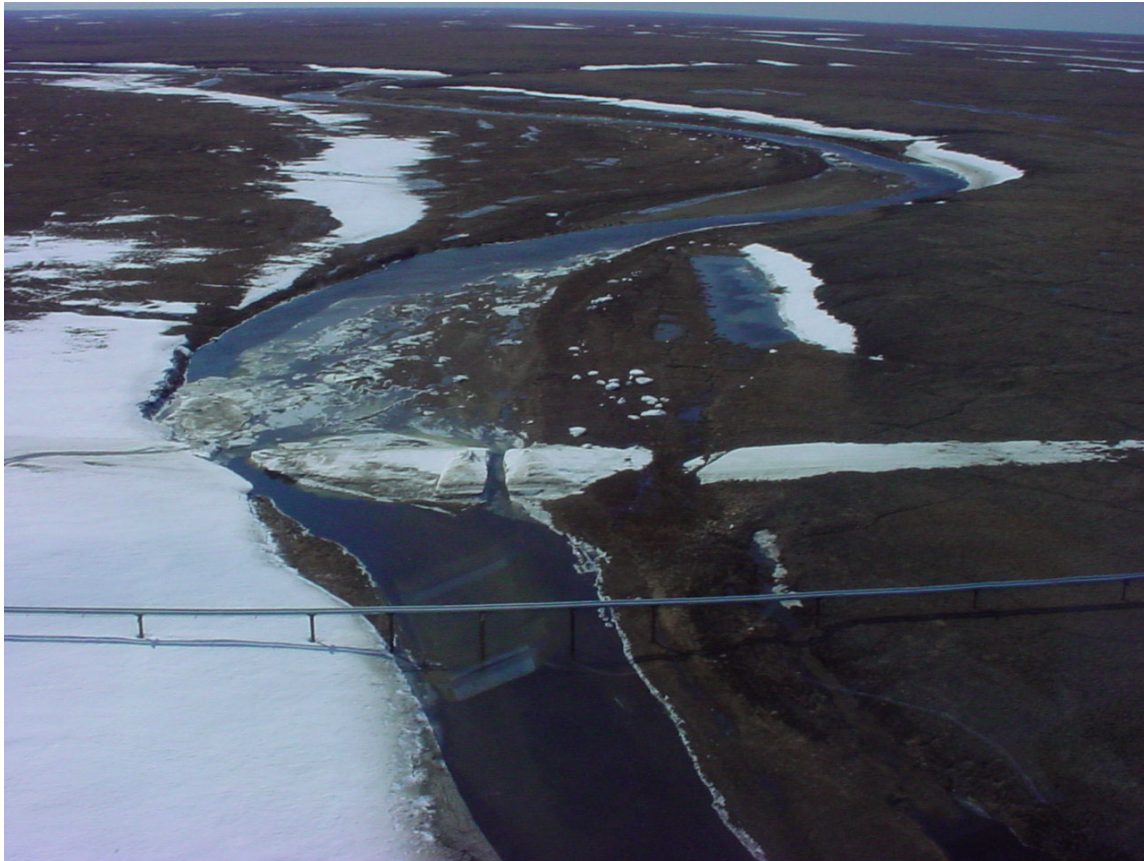
Figure 15 – Kachemach River pipeline crossing looking upstream
