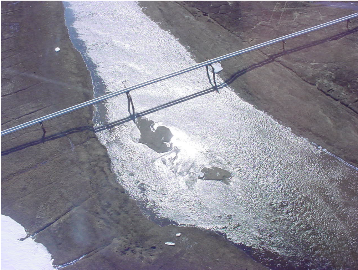
Figure 27 – Miluveach River pipeline crossing looking upstream
