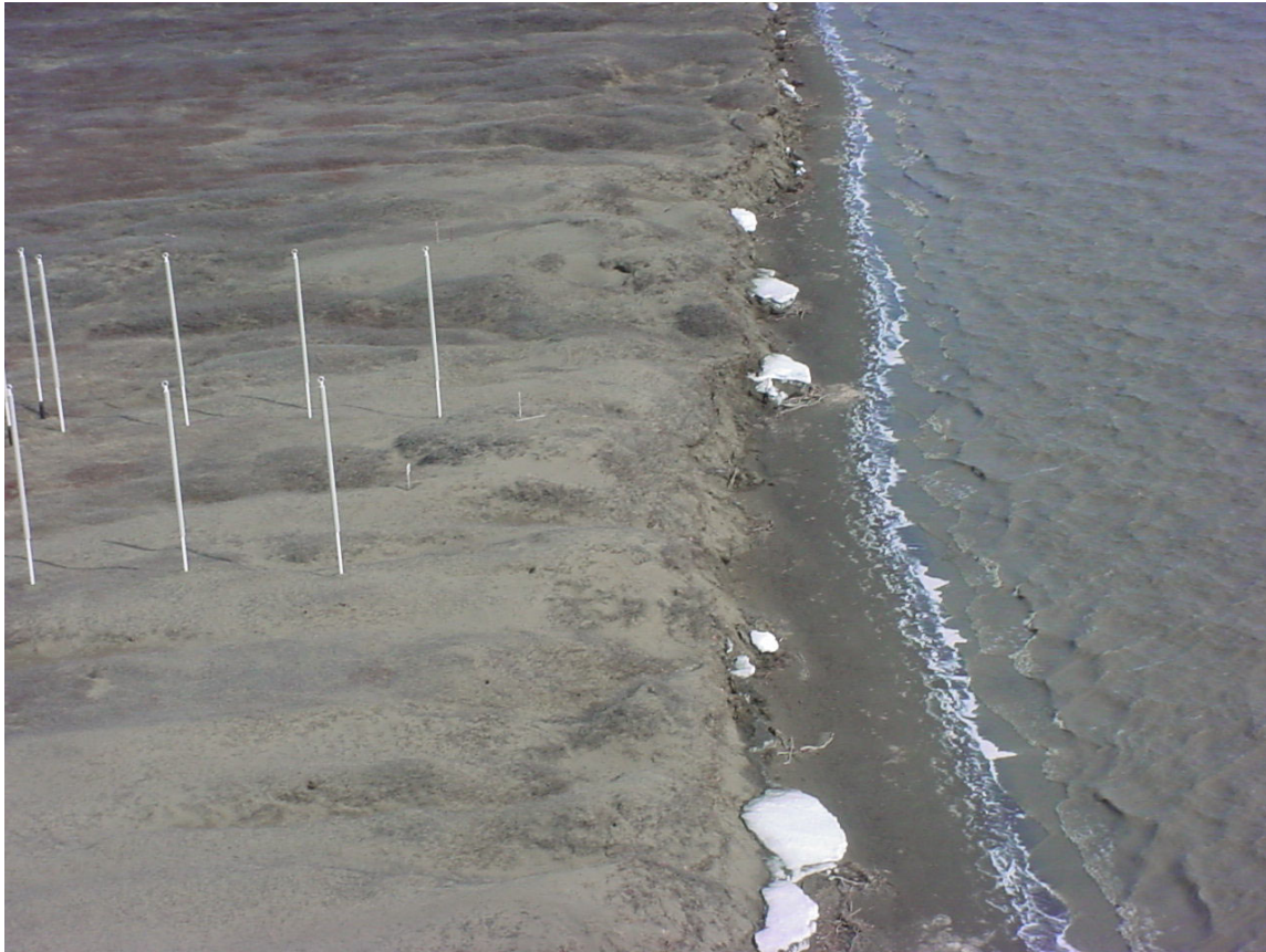
Figure 2 – Colville River HDD west bank
