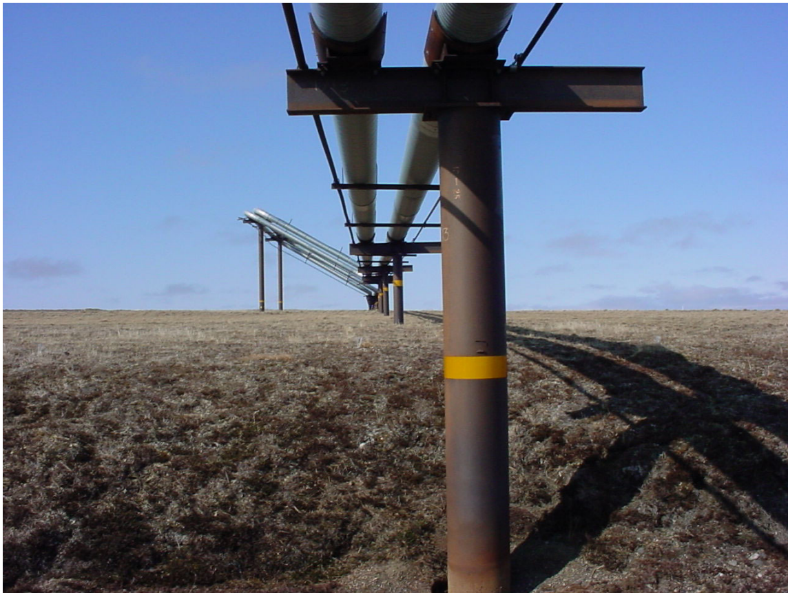
Figure 18 – VSM alignment and vertical loop, Kachemach River west bank
