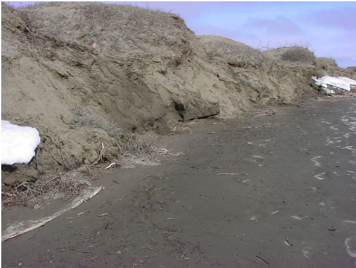
Figure 8 – Colville River HDD west bank - along pipeline alignment
