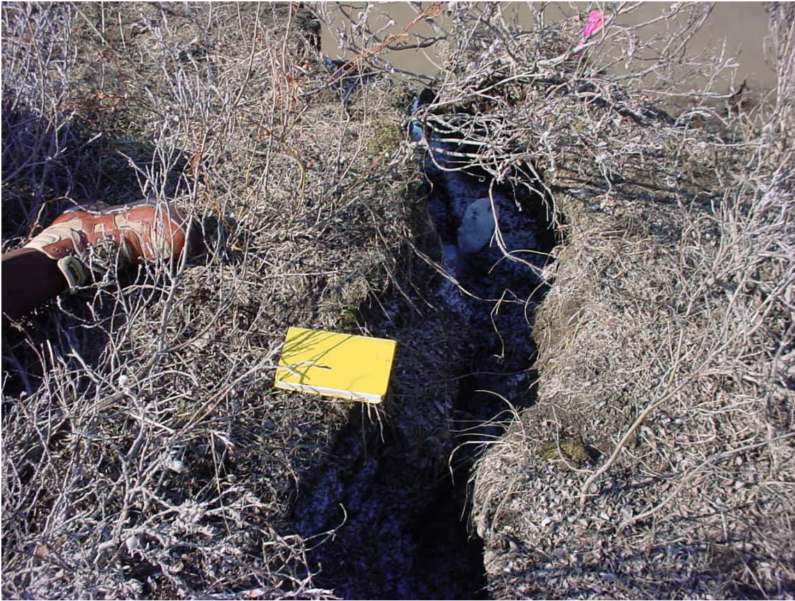
Figure 11 – Colville River HDD east bank, cracking along the top of the bank
