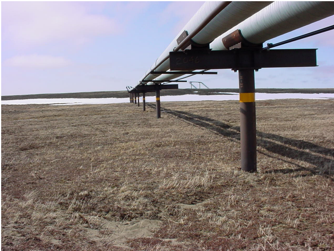
Figure 30 – VSM alignment and vertical loop, Miluveach River west bank
