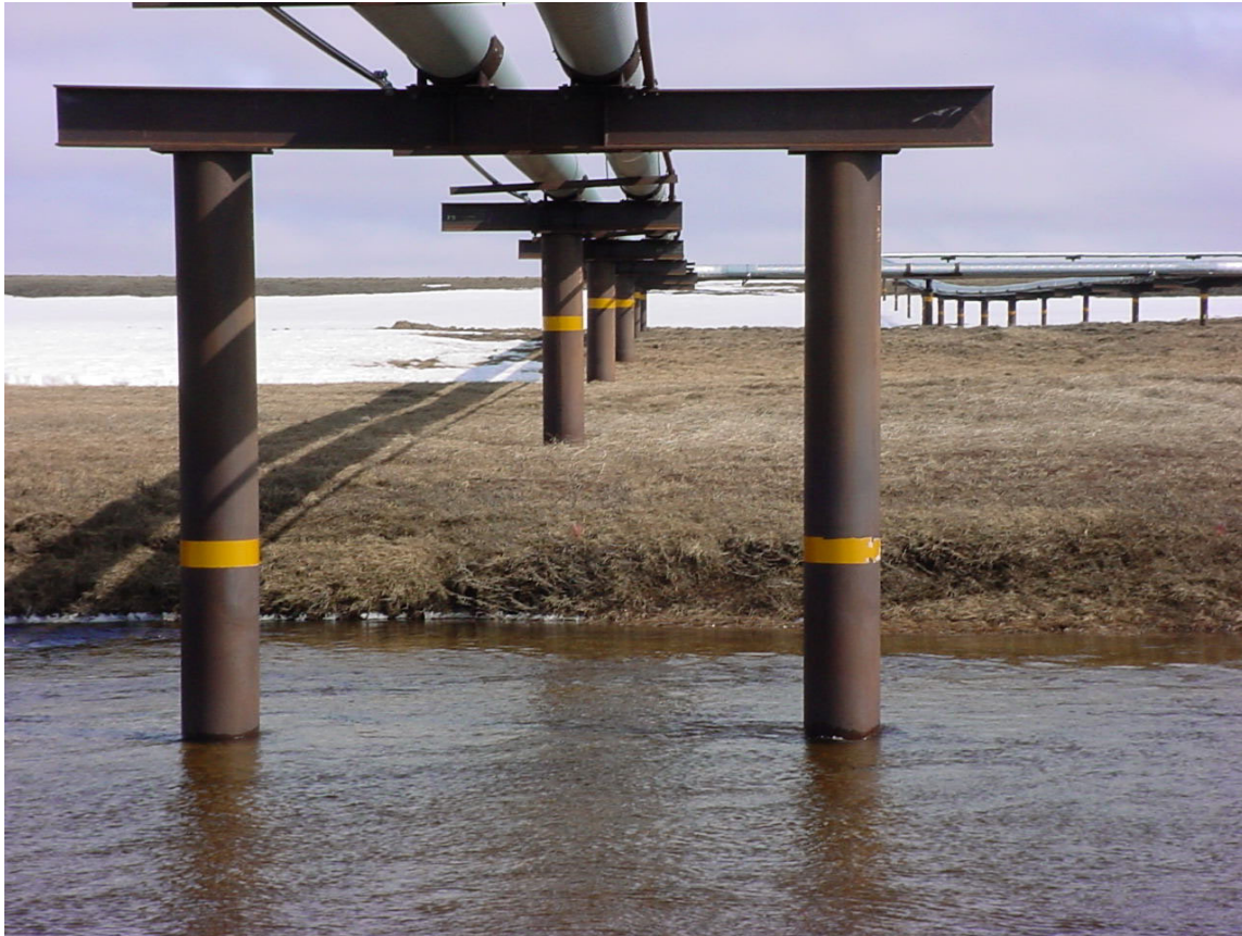
Figure 31 – VSM alignment and horizontal loop, Miluveach River east bank
