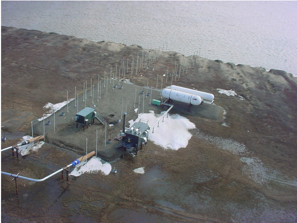
Figure 1 – Colville River HDD west bank
