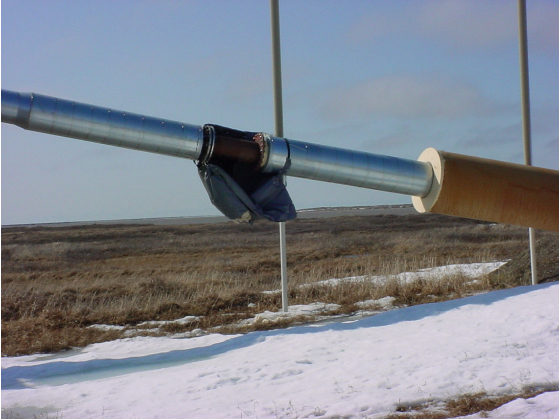
Figure 12 – Colville River HDD east bank, loose pipeline insulation jacket
