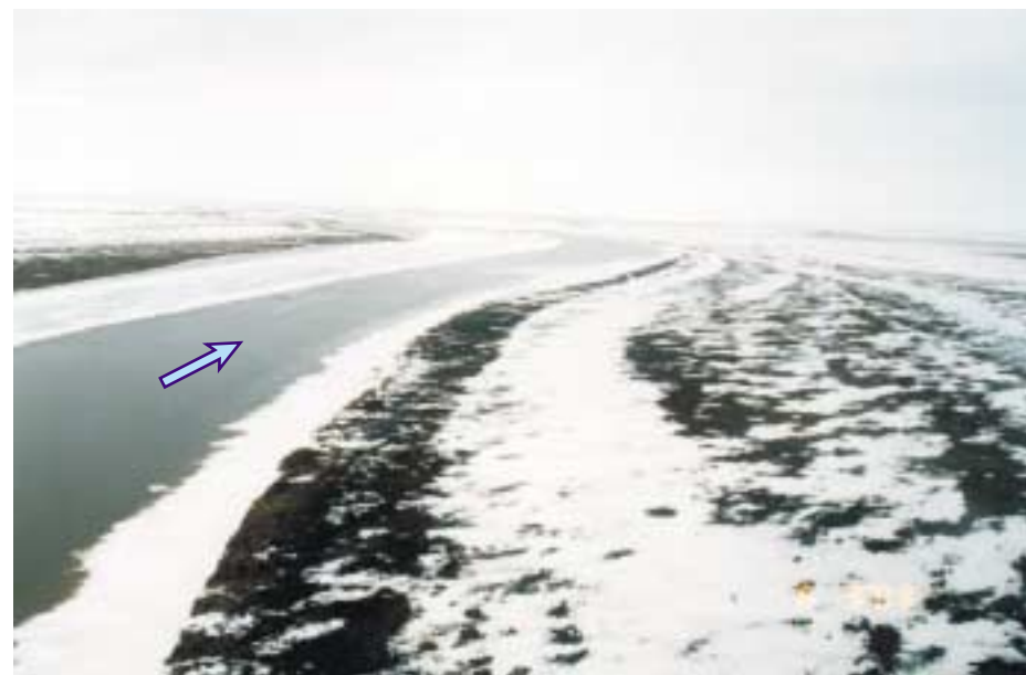
2. Close up of east floodplain.
