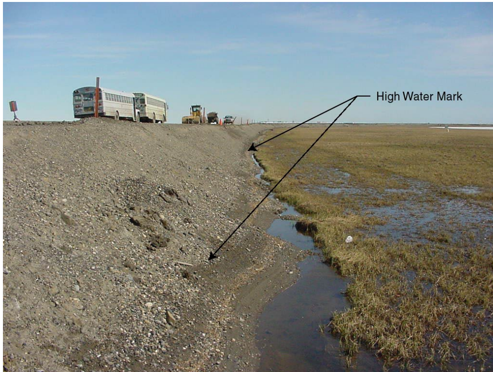
Photo 6 Facing east from Culvert #24 along the south side of the CD-2 access road. (6/16/01)
