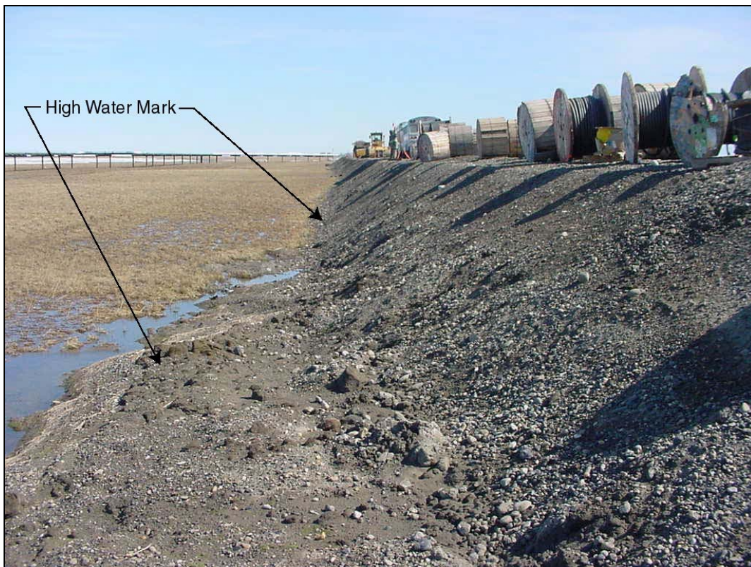
Photo 5 Facing east from Culvert #24 along the north side of the CD-2 access road. (6/16/01)
