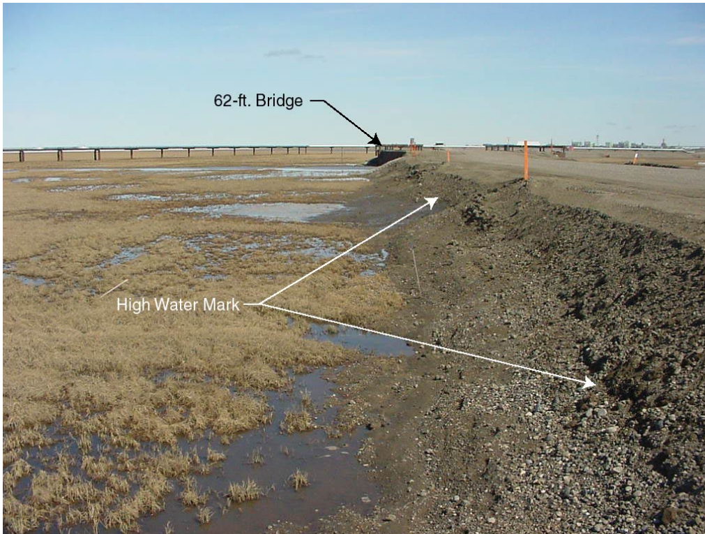
Photo 11 Facing east from Culvert #04 along the north side of the CD-2 access road. (6/15/01)
