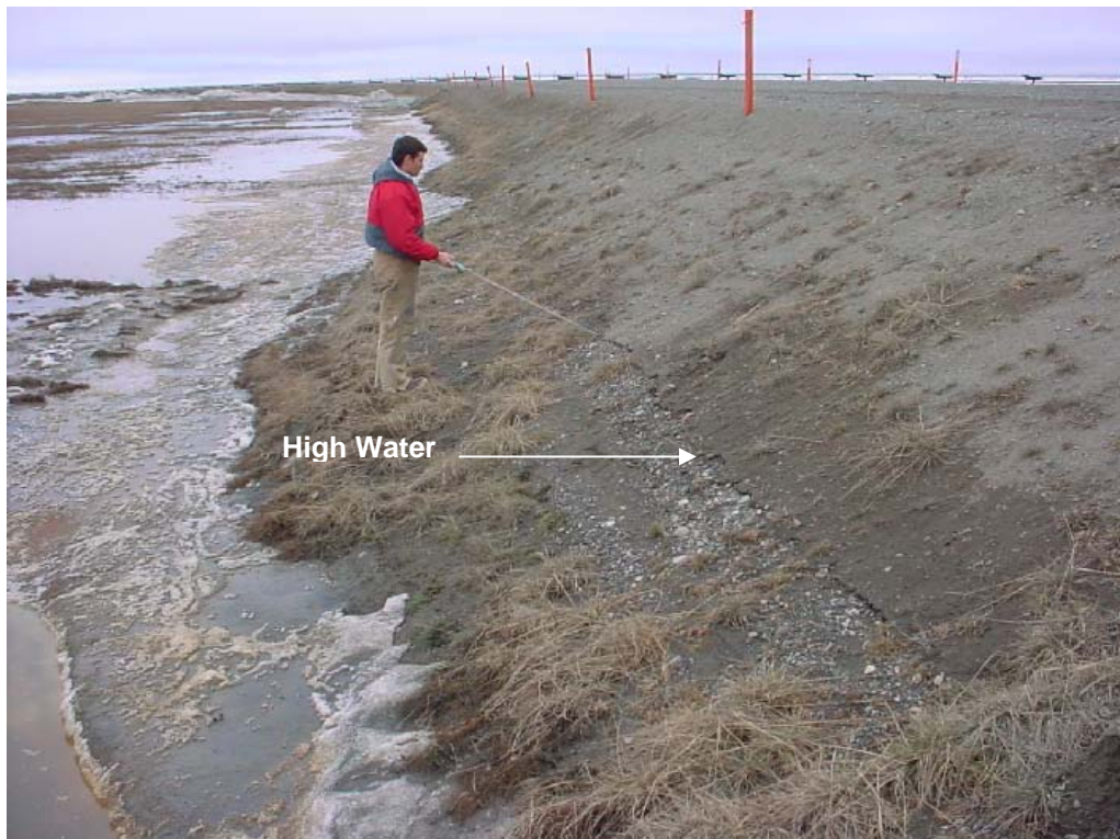
Photo 29 Looking west from culvert # 10 on south side of the CD2 road. (6/1/04)
