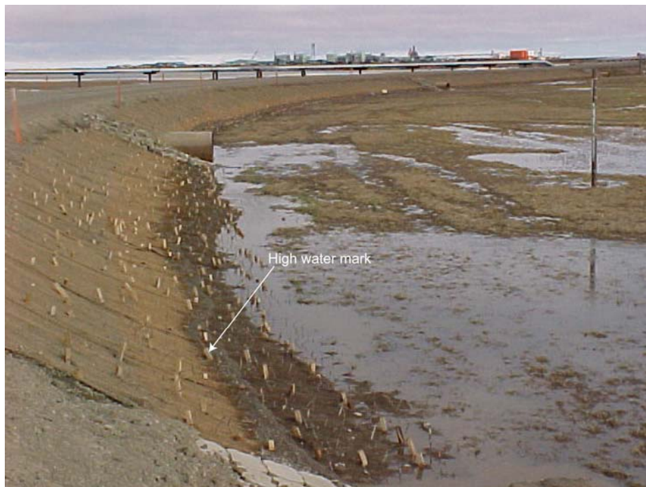
Photo 20 Facing east along the south side of the CD-2 access road from the 62-foot bridge. (5/31/02)
