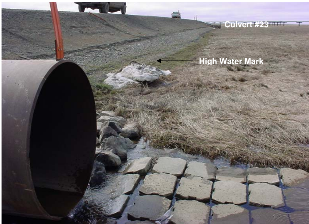
Photo 22 Looking west on the north side of the CD-2 access road from Culvert # 24. (6/13/03)
