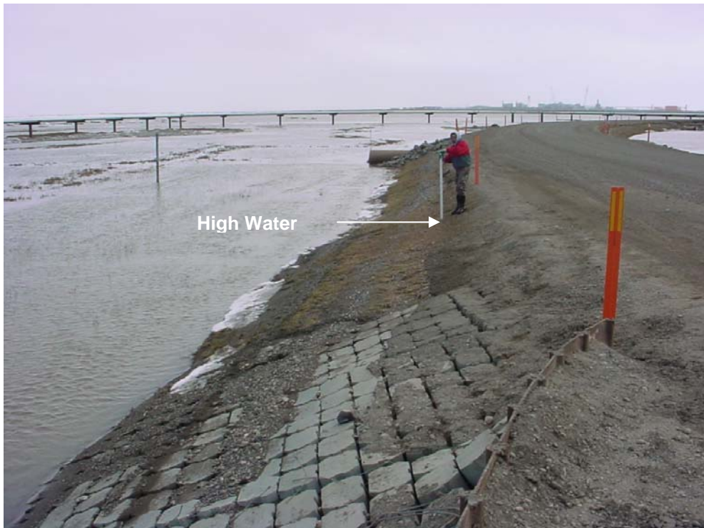
Photo 27 High water mark on north side of CD-2 road between the 62-foot bridge and Culvert #22 near Permanent Staff Gage #4. (6/1/04)
