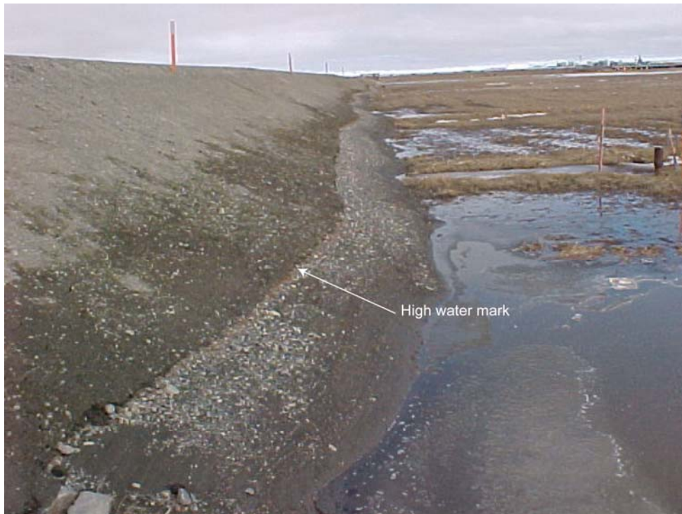
Photo 19 Facing east from culvert #20 along the south side of the CD-2 access road. (5/31/02)
