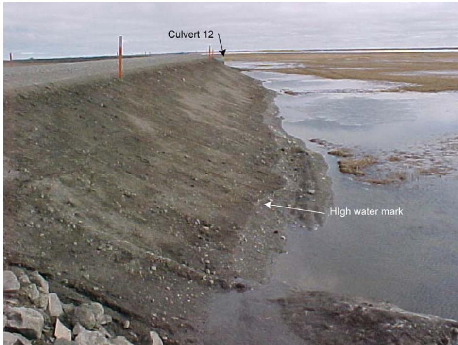
Photo 15 Facing east from culvert #11 along the south side of the CD-2 access road. (5/31/02)
