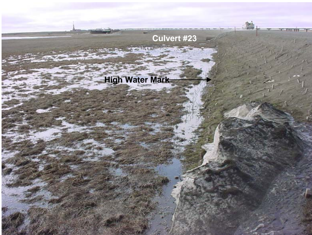
Photo 23 Looking west on the south side of the CD-2 access road from Culvert # 24. (6/13/03)
