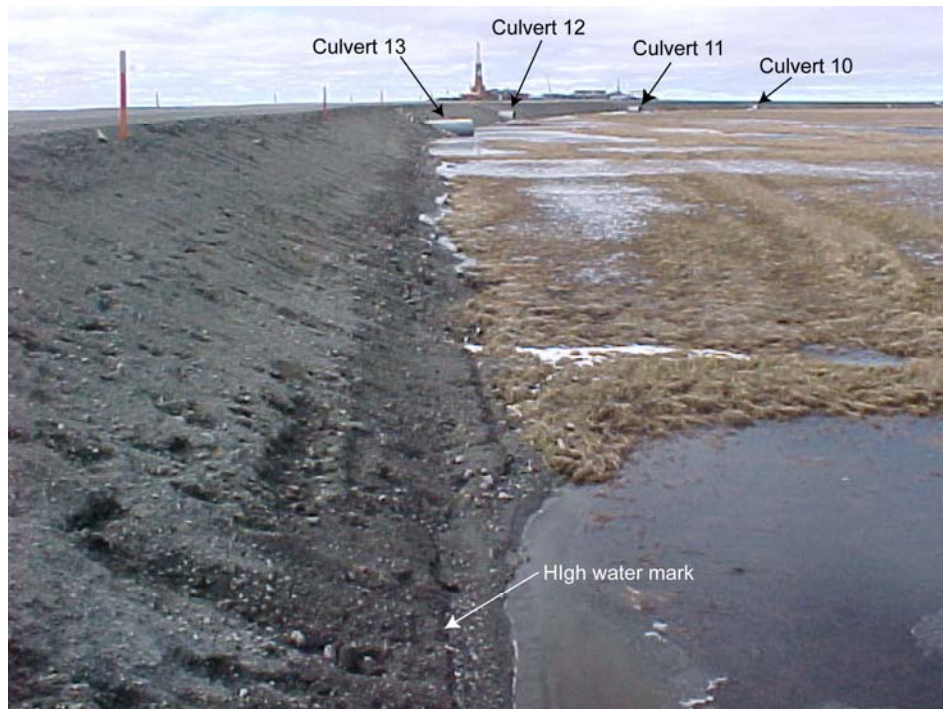
Photo 16 Facing west from culvert #14 along the north side of the CD-2 access road. (5/31/02)
