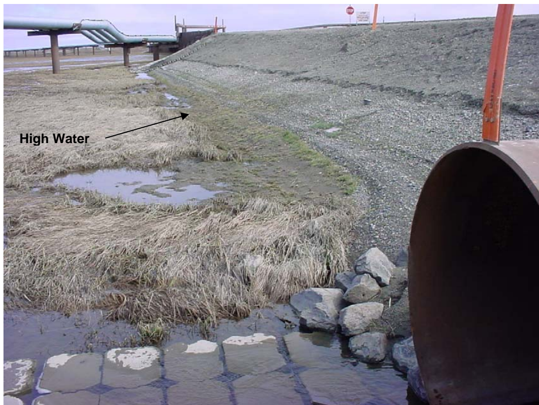
Photo 21 Looking east on the north side of the CD-2 access road from culvert #24. (6/13/03).
