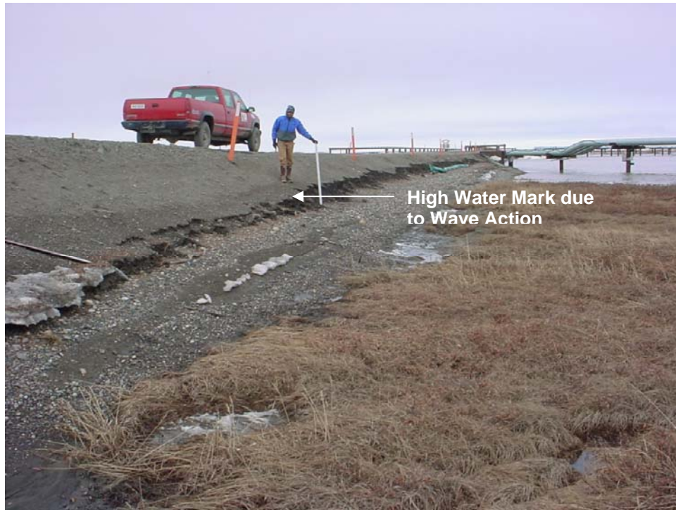
Photo 24 Sideslope erosion of surficial gravel due to wind-driven wave impact on north side of CD-2 road between the 452-foot bridge and Culvert #25. (6/1/04)
