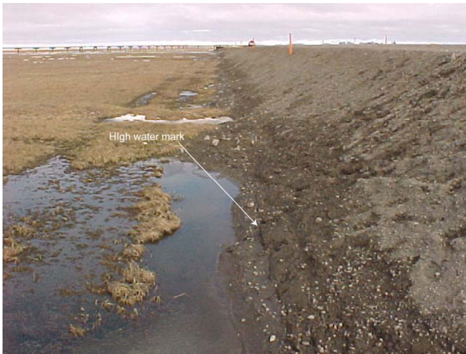
Photo 18 Facing east from culvert #20 along the north side of the CD-2 access road. (5/31/02)
