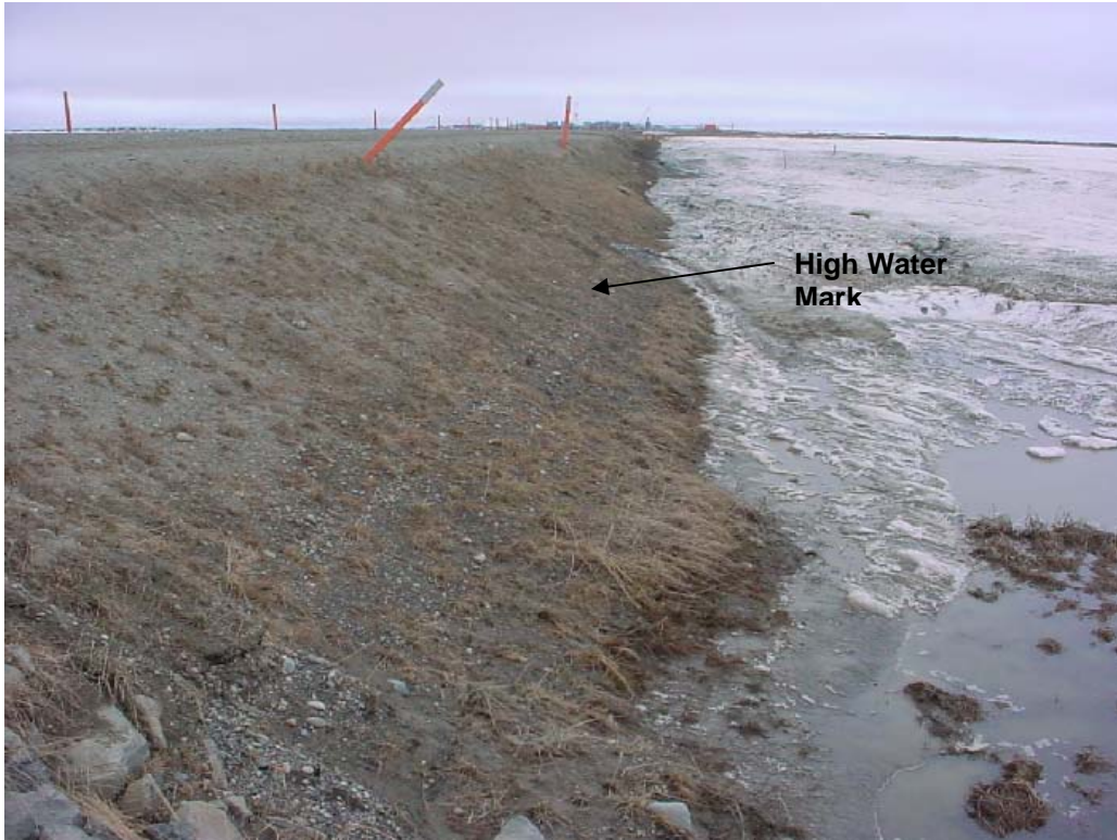
Photo 30 Looking west on south side of CD-2 road at culvert # 16 (6/1/04)
