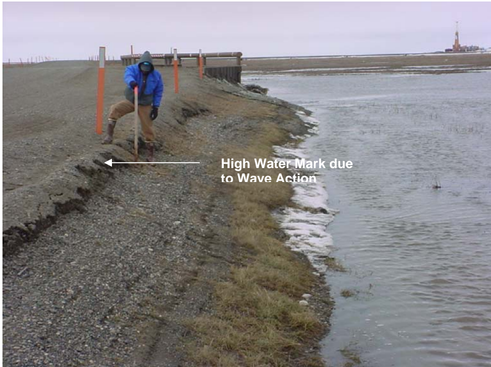
Photo 26 High water mark on north side of CD-2 road between the 62-foot bridge and Culvert #22. (6/1/04)
