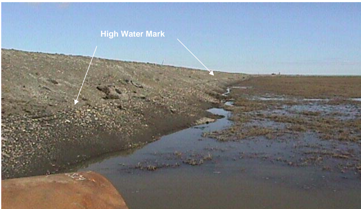
Photo 2 Looking east along the south side of the embankment on the CD-2 access road near culvert #24. (6/15/00)
