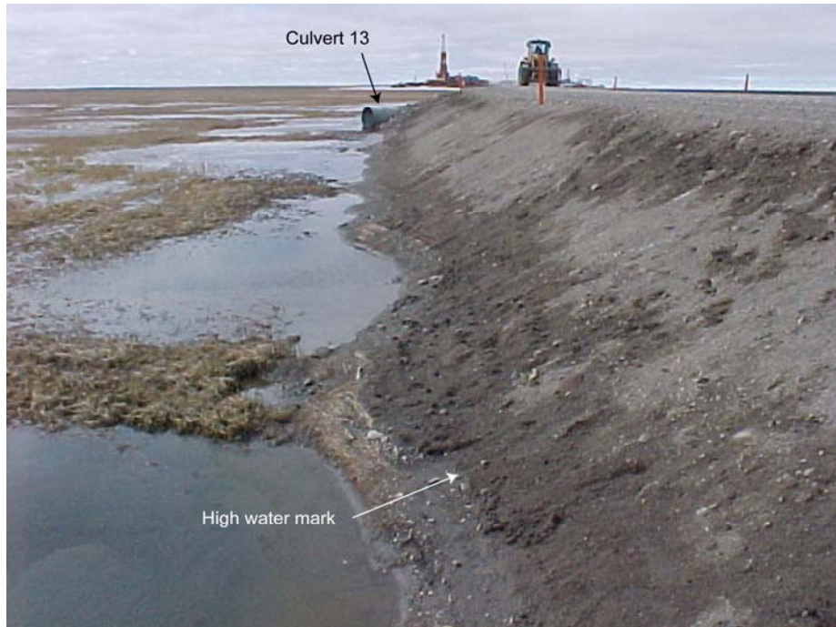
Photo 17 Facing west from culvert #14 along the south side of the CD-2 access road. (5/31/02)
