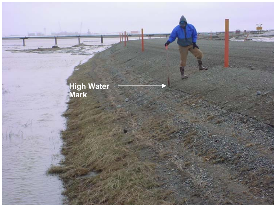
Photo 25 High water mark on north side of CD-2 road between the 62-foot and 452-foot bridges. (6/1/04)
