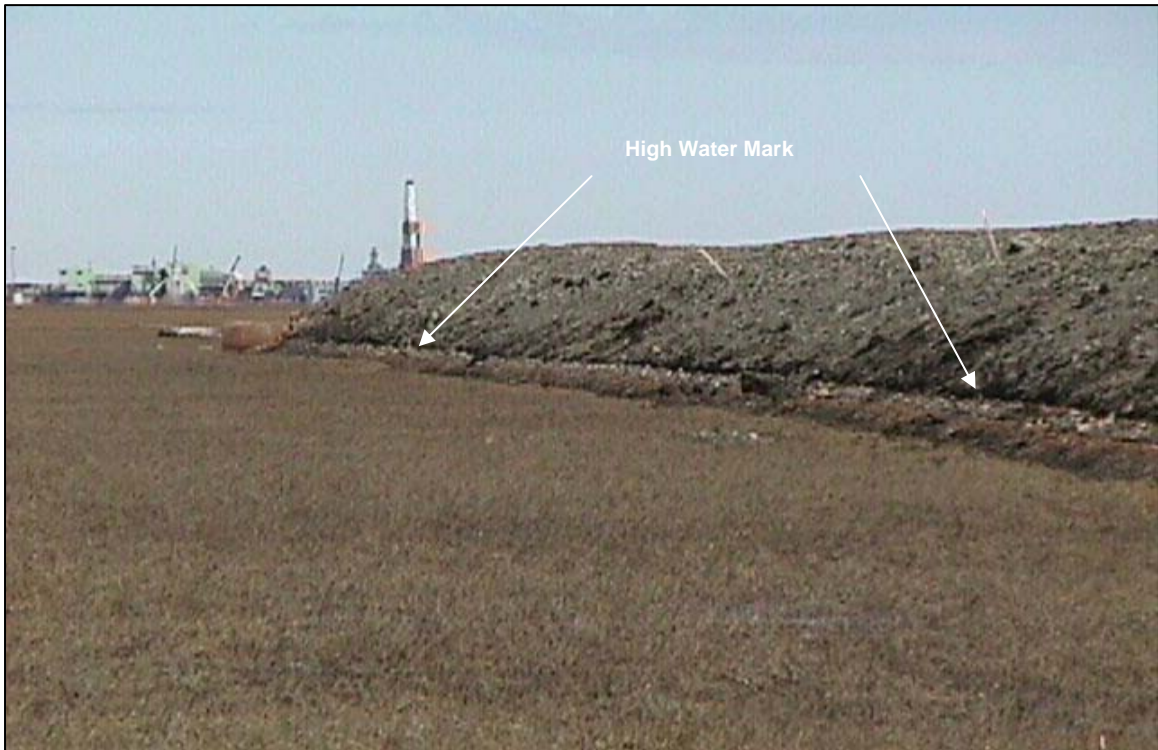
Photo 1 Looking east along the north side of the embankment on the road to CD-2 near culvert #24. (6/15/00)
