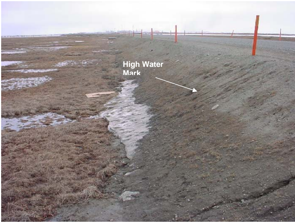
Photo 28 Looking east from culvert # 17 at the north side of the CD2 road. (6/1/04)
