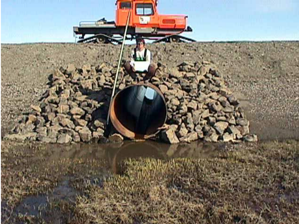
Photo 11 Looking north at the south end of culvert #4. (6/18/00)
