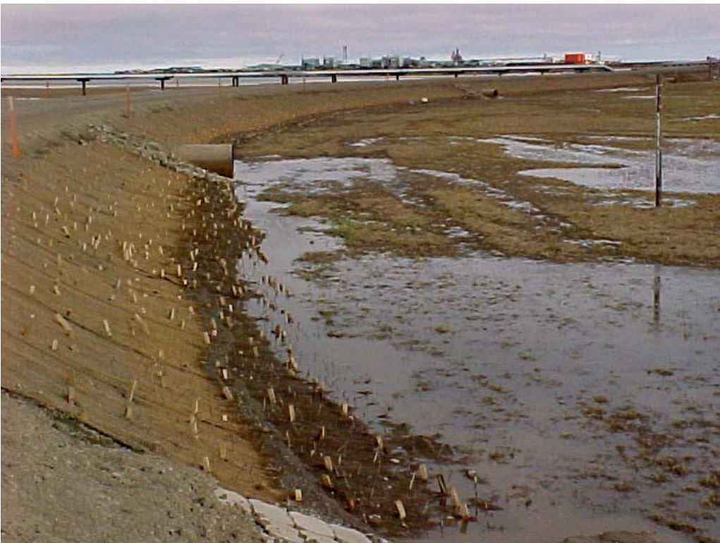
Photo 12 Facing east along the south side of the CD-2 access road from culvert #22. Looking at culverts #23 and #24. (5/31/02)
