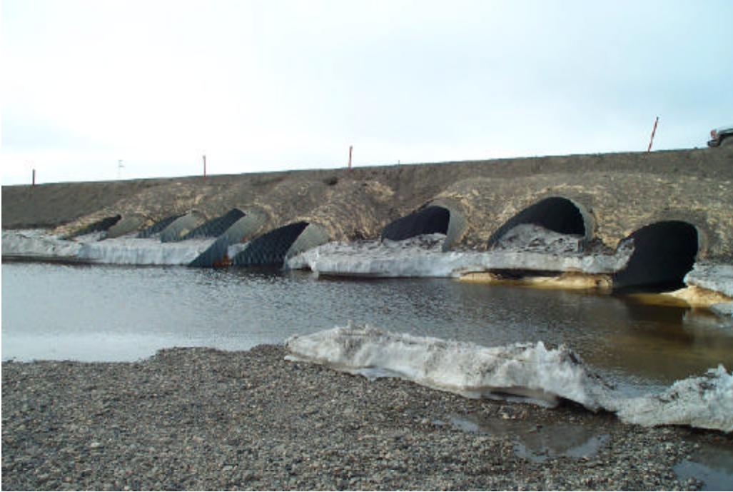
Photo 1 Culverts located in the East Creek in the Spine Road. (6/8/01)
