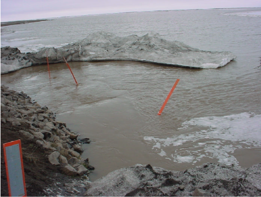
Photo 7 Flow conditions on the south (upstream) side of the CD-2 access road for culverts 4, 5, 6, and 7. (5/28/04)
