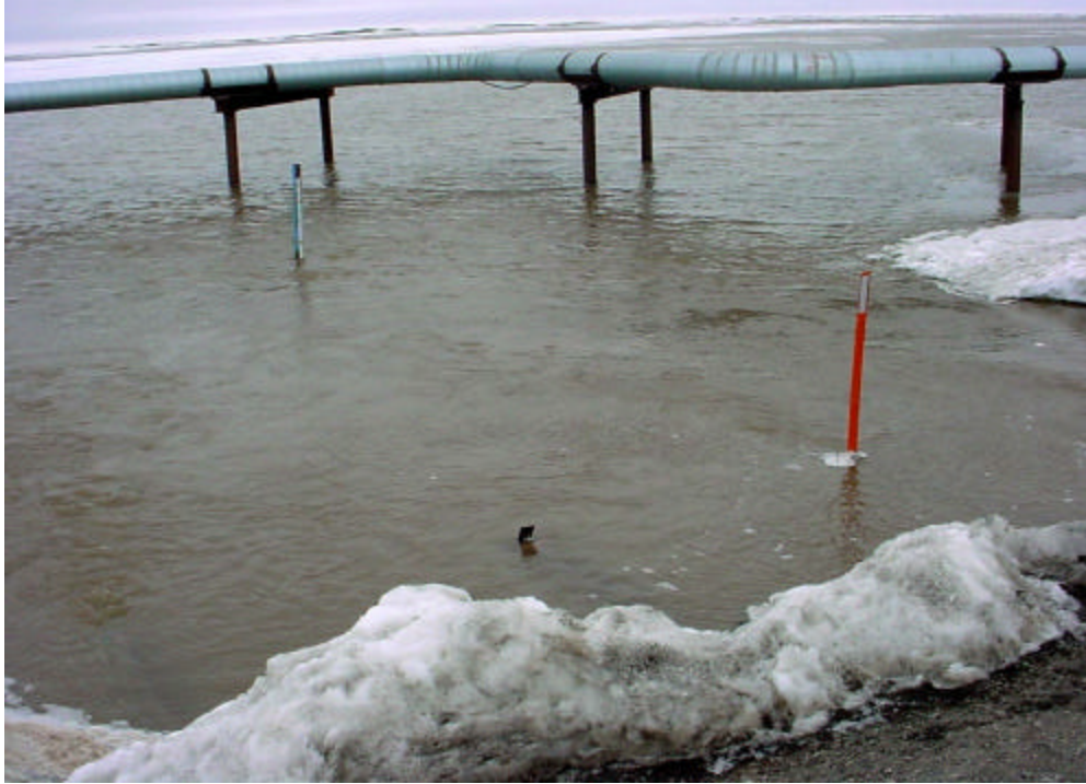
Photo 9 Looking northeast on north (downstream) side of road at culverts 4, 5, 6 and 7. Picture taken approximately 24 hours after peak stage was observed in the Alpine infield. (5/28/04)
