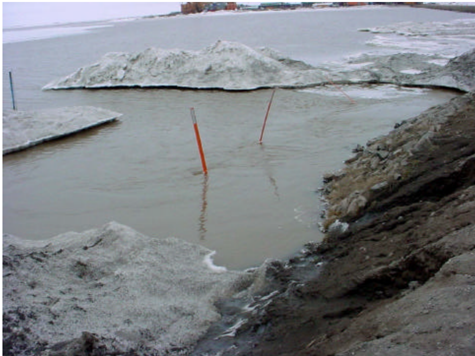
Photo 8 Looking west on south (upstream) side of road at culverts 4, 5, 6 and 7. Picture taken approximately 24 hours after peak stage was observed in the Alpine infield. (5/28/04)
