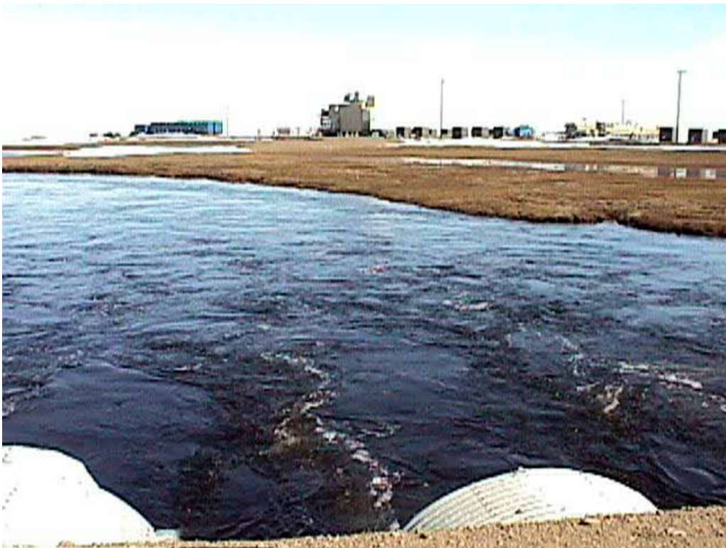
Photo 4 Downstream end of culverts located in the Prudhoe Bay Unit (WOA) near W pad. (6/16/00)
