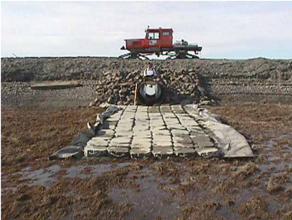
Photo 10 Looking south at the north end of culvert #2. (6/18/00)
