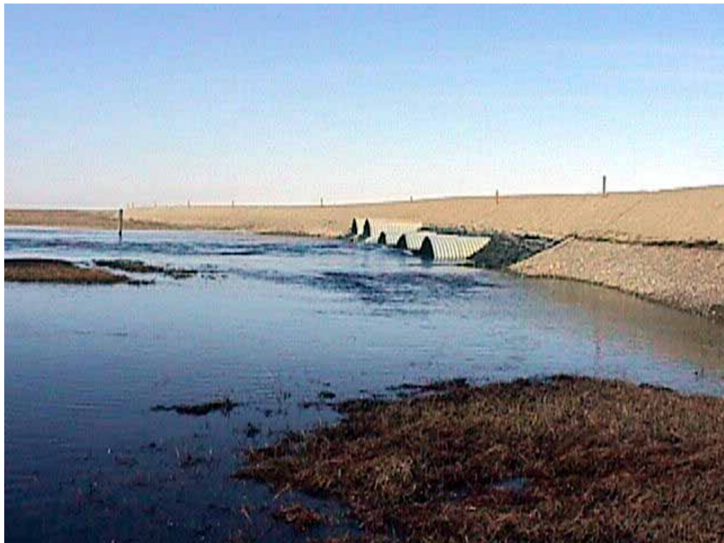
Photo 2 Culverts located in the Prudhoe Bay Unit (WOA) near W pad. (6/16/00)
