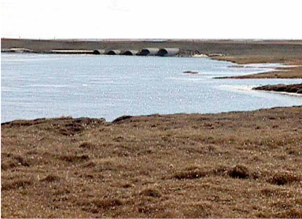
Photo 3 Culverts located in the Prudhoe Bay Unit (WOA) near W pad. (6/16/00)
