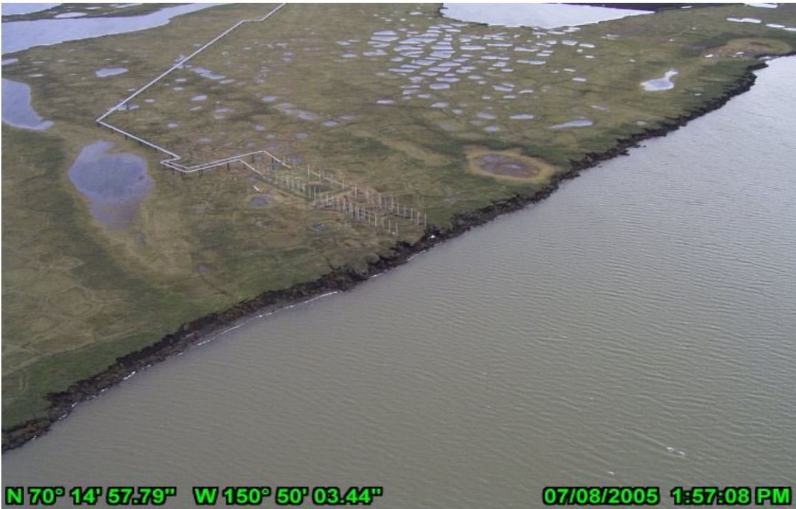
Photo 7 HDD River Crossing, east bank July 8, 2005. Aerial view of HDD crossing.
