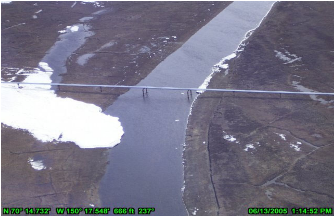
Photo 17 Miluveach River Crossing June 13, 2005. Aerial view of pipeline crossing.
