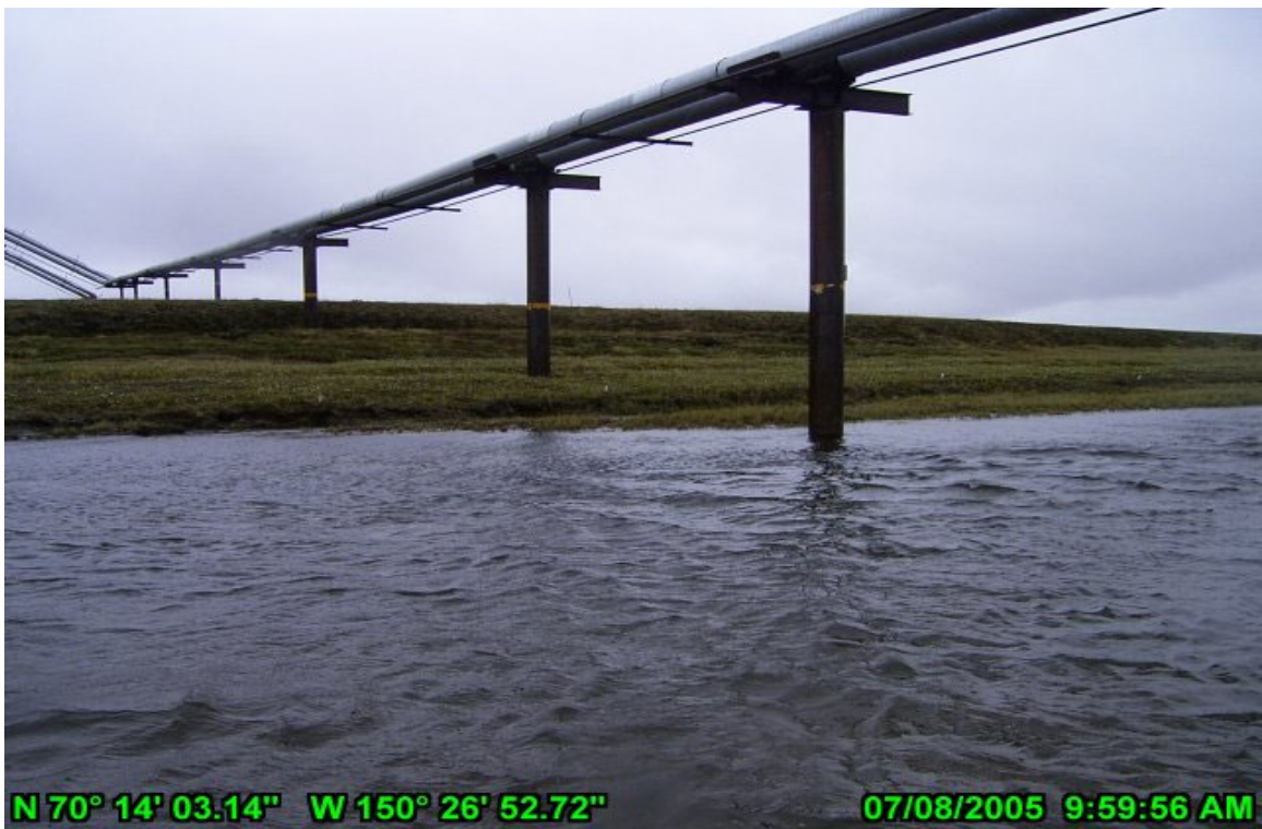
Photo 16 Kachemach River Crossing July 8, 2005. Pipeline VSM's.
