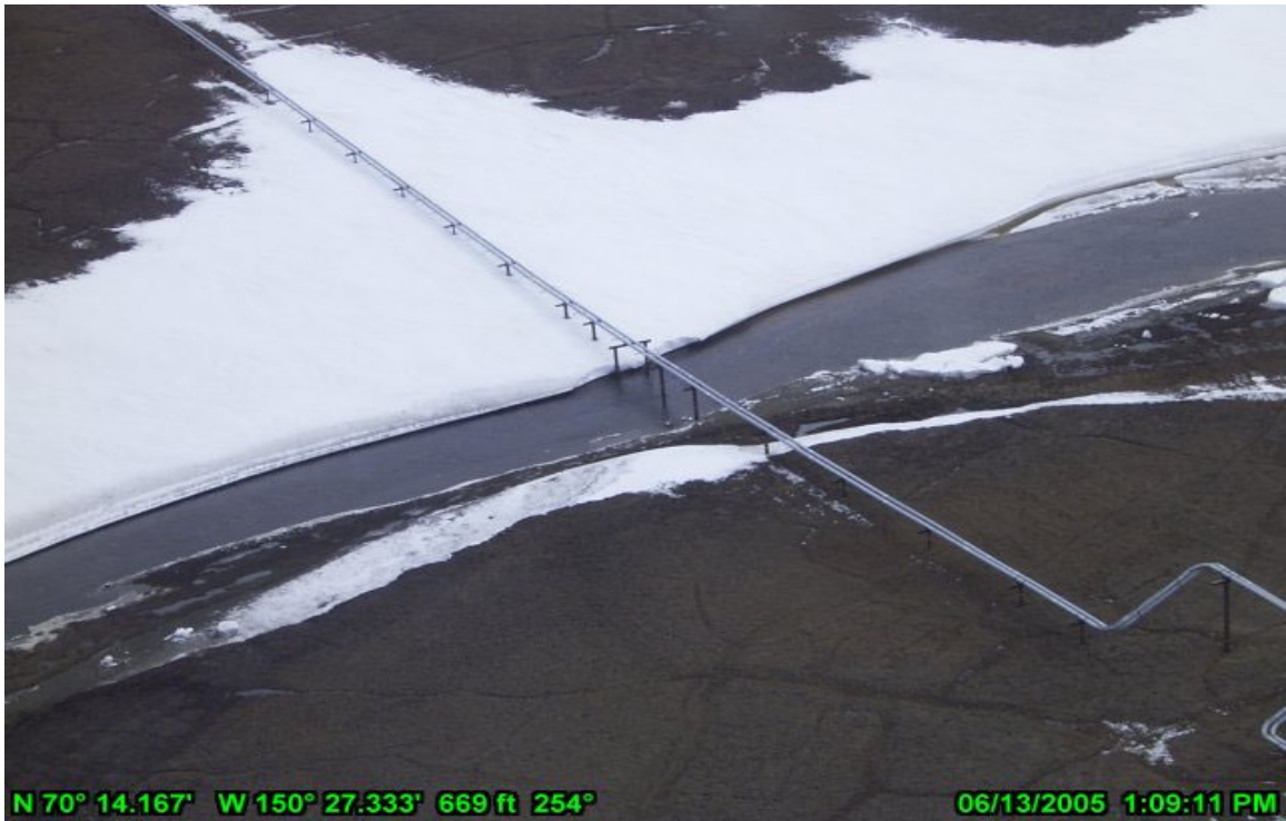
Photo 13 Kachemach River Crossing June 13, 2005. Aerial view of pipeline crossing.
