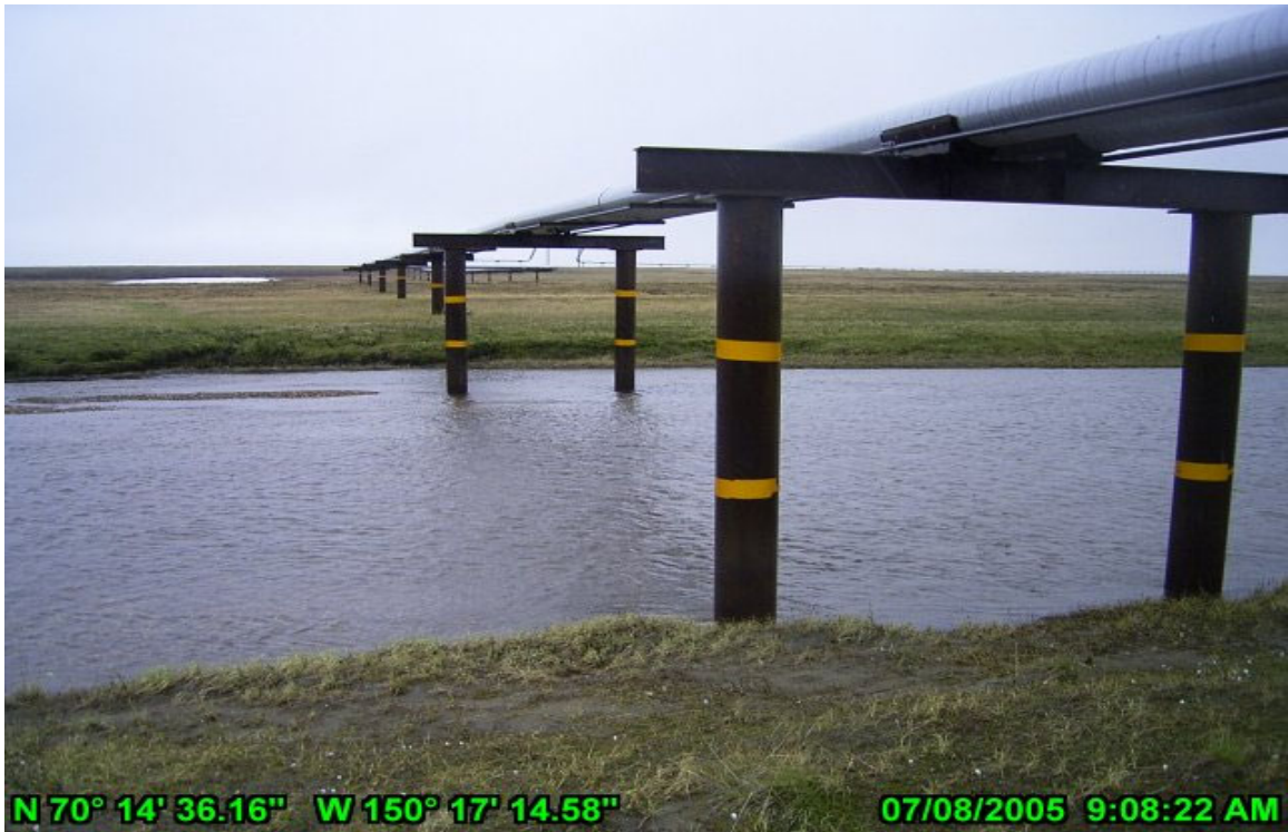
Photo 19 Miluveach River Crossing July 8, 2005. Pipeline VSM's.
