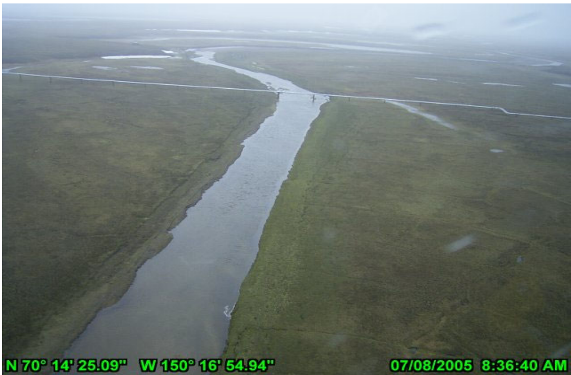
Photo 18 Miluveach River Crossing July 8, 2005. Aerial view of pipeline crossing.
