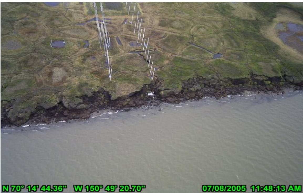
Photo 8 HDD River Crossing, east bank July 8, 2005. Aerial view of HDD crossing.
