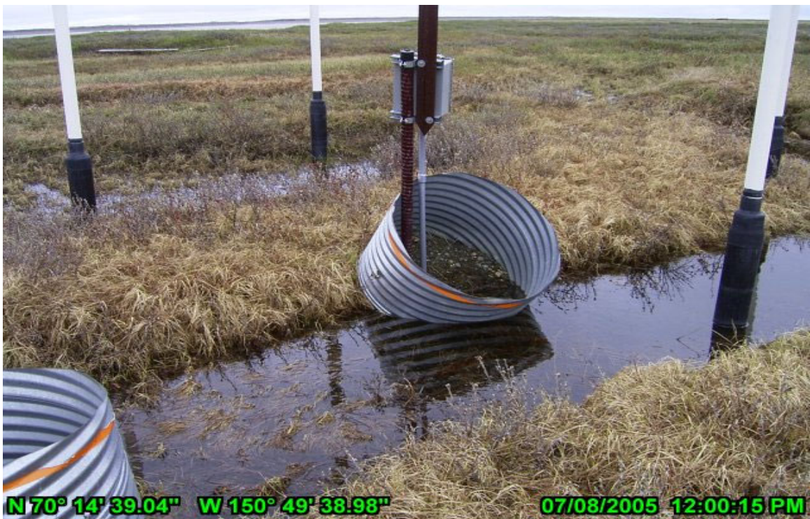
Photo 12 HDD River Crossing, east bank July 8, 2005. Thermistor casing.
