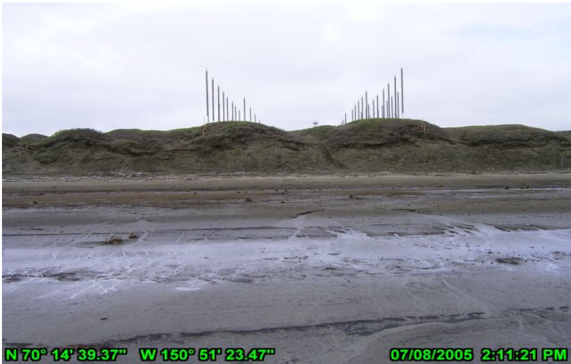
Photo 3 HDD River Crossing, West Bank July 8, 2005. Bluff high water mark.
