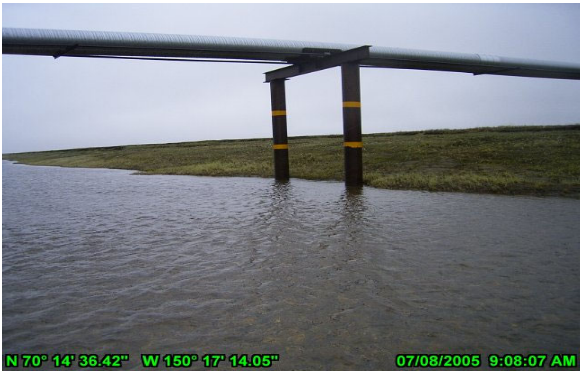
Photo 20 Miluveach River Crossing July 8, 2005. Pipeline VSM's.
