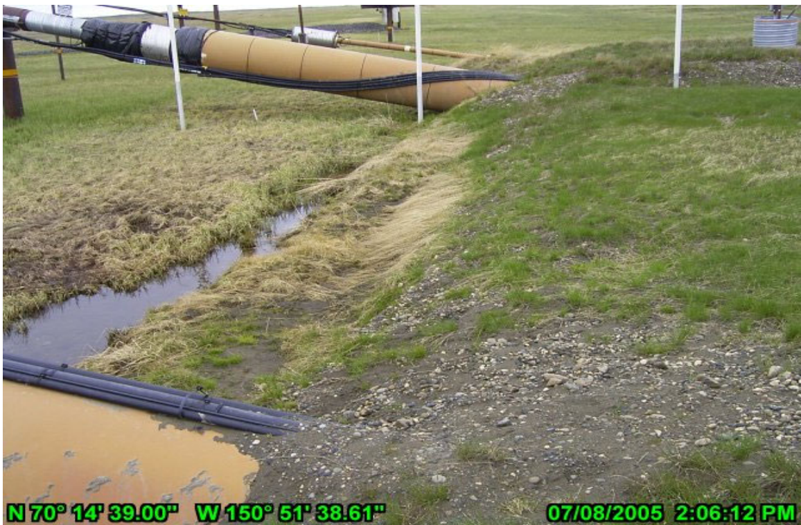
Photo 6 HDD River Crossing, West Bank July 8, 2005. HDD casing transition.
