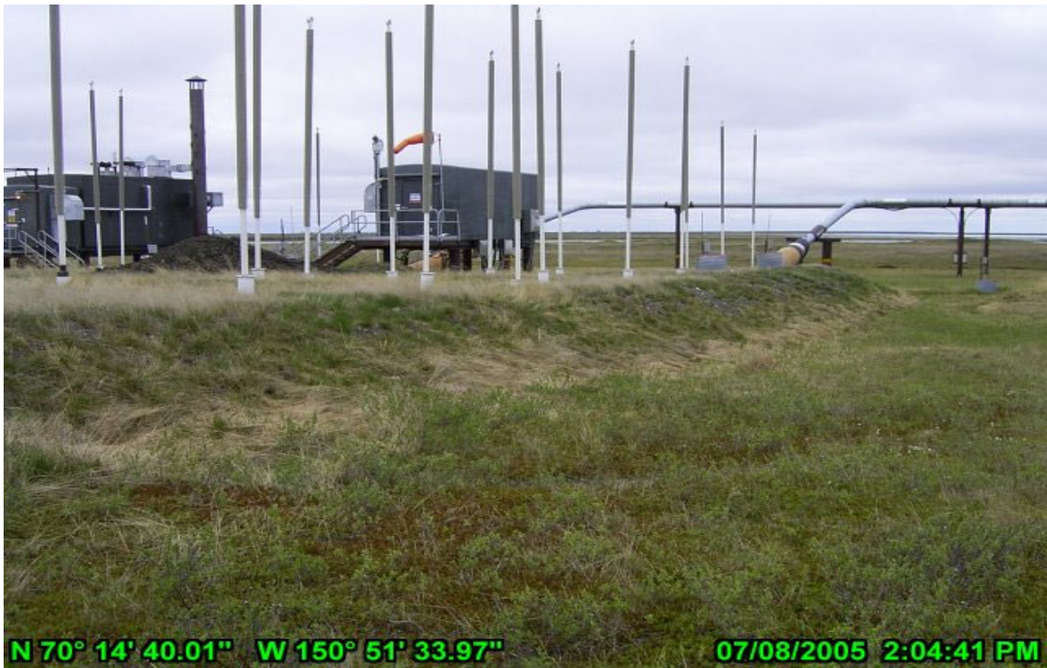
Photo 5 HDD River Crossing, West Bank July 8, 2005. Heat pipes.
