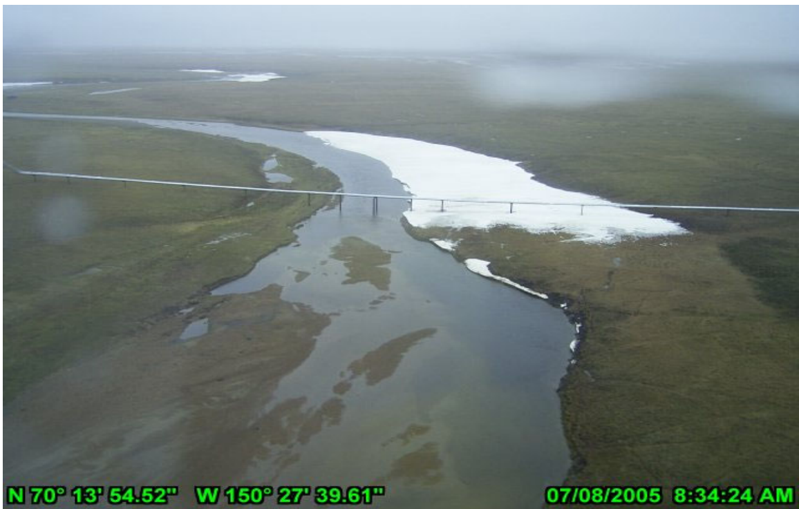
Photo 14 Kachemach River Crossing July 8, 2005. Aerial view of pipeline crossing.
