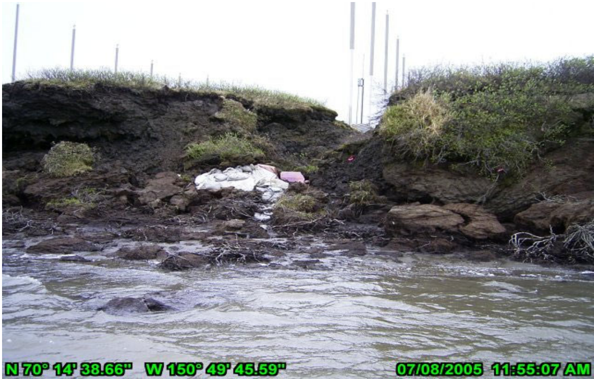
Photo 9 HDD River Crossing, east bank July 8, 2005. Erosion at polygon trough.
