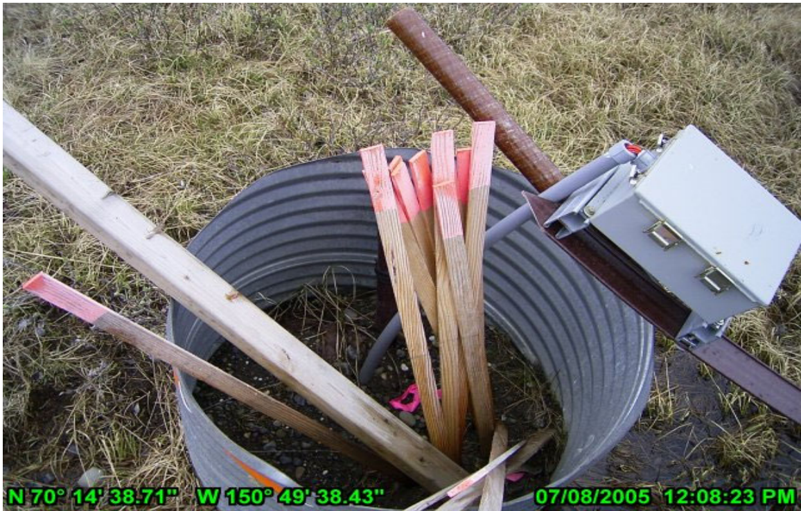
Photo 11 HDD River Crossing, east bank July 8, 2005. Thermistor casing.
