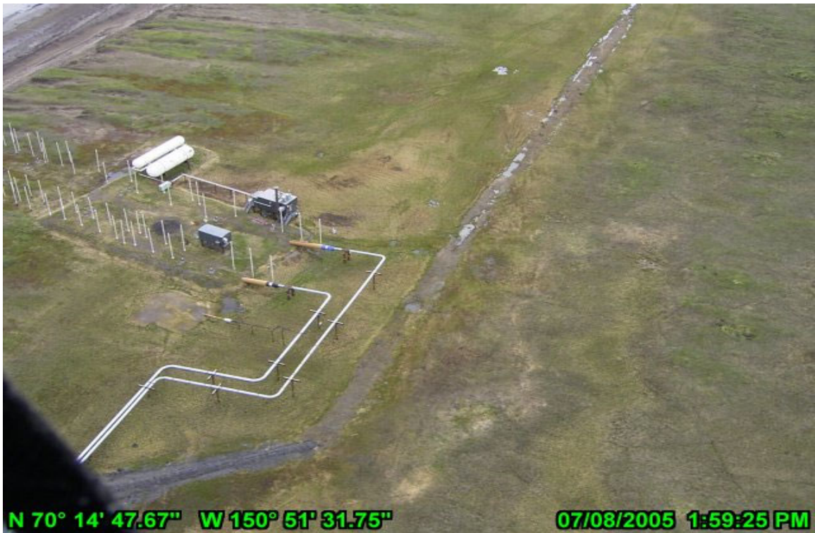
Photo 2 HDD River Crossing, West Bank July 8, 2005. Aerial view of HDD crossing.
