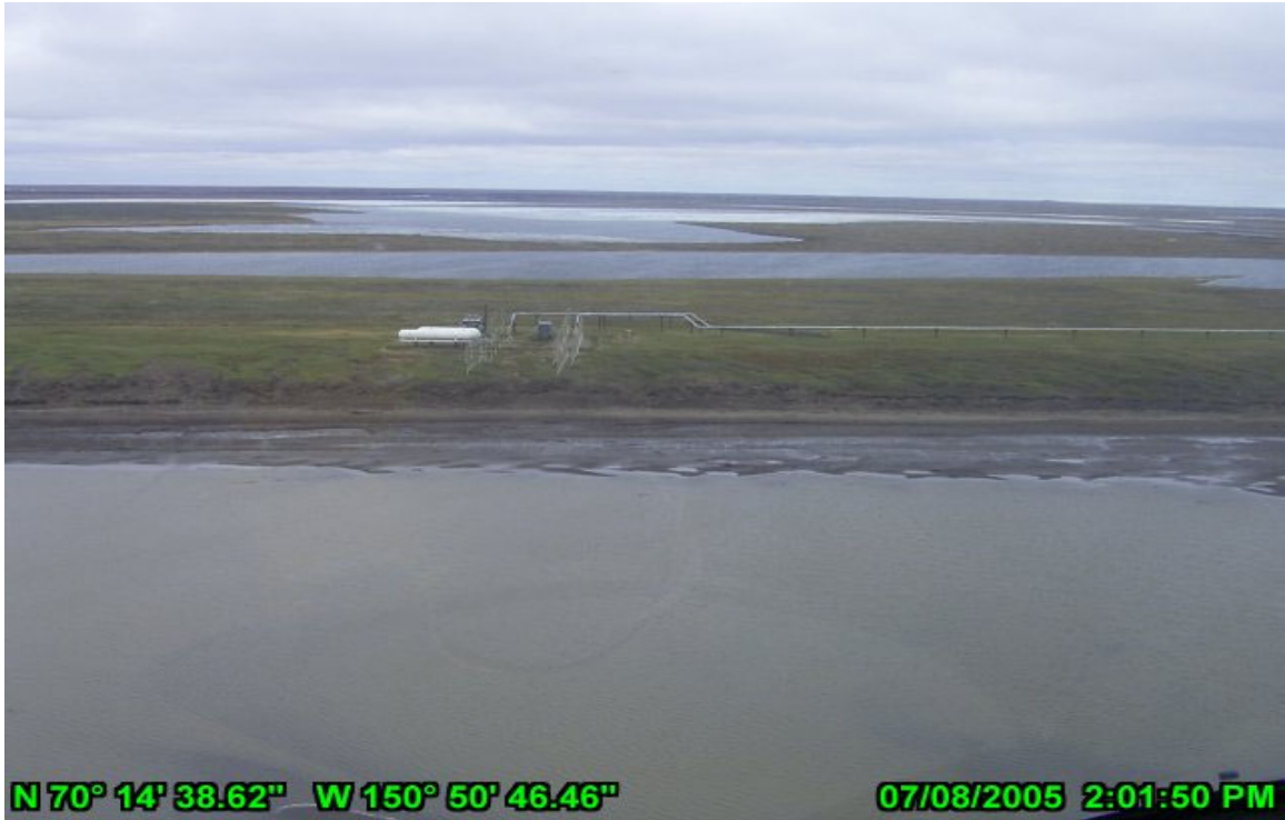
Photo 1 HDD River Crossing, West Bank July 8, 2005. Aerial view of HDD crossing.
