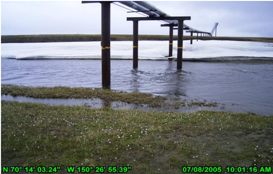
Photo 15 Kachemach River Crossing July 8, 2005. Pipeline VSM's.
