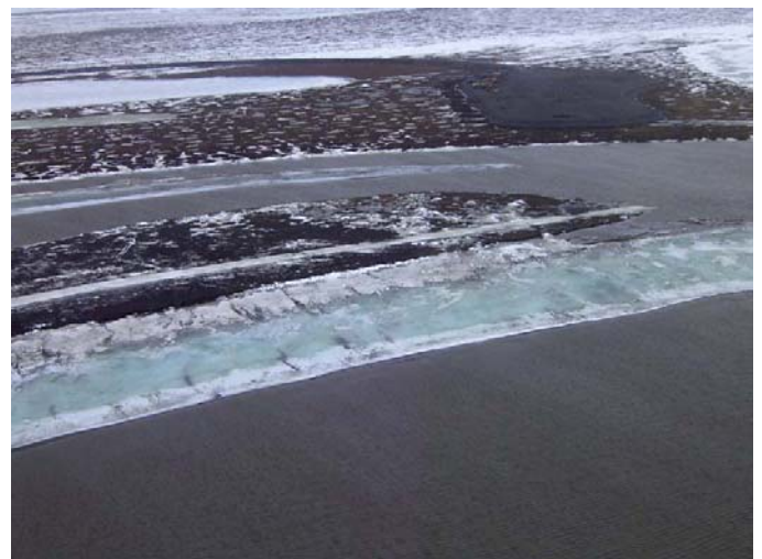
Photo 3-4 CD4 pad and access road, May 30, 2005
