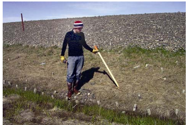
Photo 4-26 High water mark on CD2 road in the swale region, July 9, 2005
