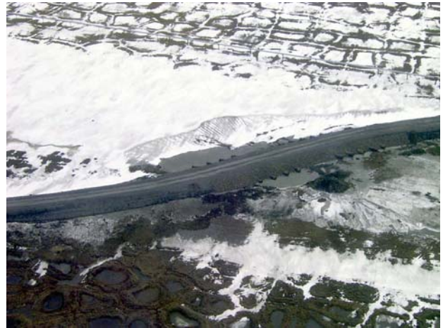
Photo 4-23 CD4 road northern Paleo culverts during peak stage, June 1, 2005
