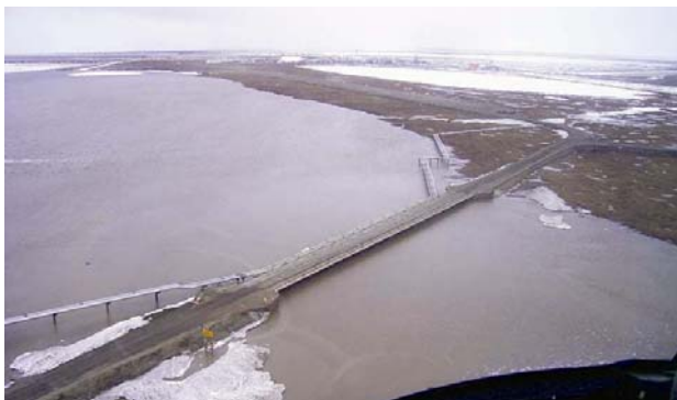
Photo 4-19 Conditions during direct discharge measurement at 452-foot swale bridge, June 2, 2005
