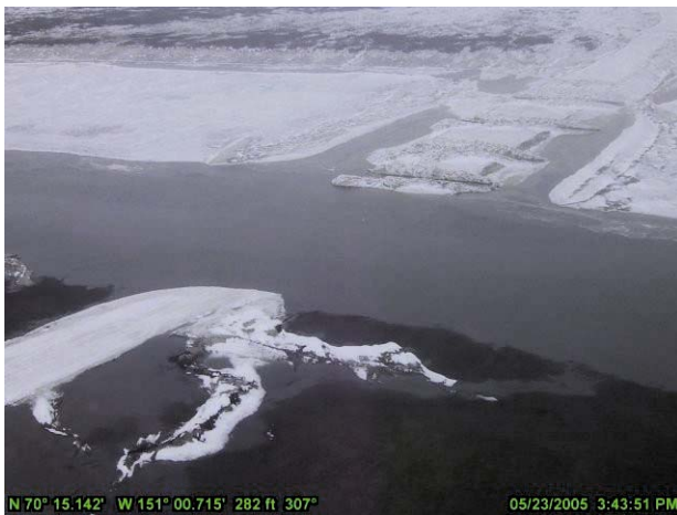
Photo 4-31 Colville Nigliq Channel Ice Bridge during breakup with the ice road in place, May 23, 2005
