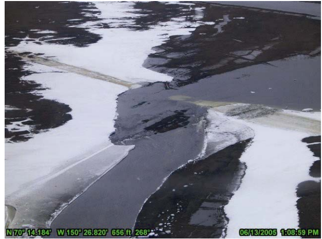
Photo 4-33 Kachemach River Ice Bridge during breakup with the ice road in place, June 13, 2005
