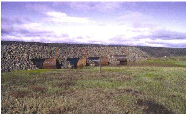
Photo 4-24 CD4 road alignment after recession of flood at the north Paleo culvert battery, July 10, 2005
