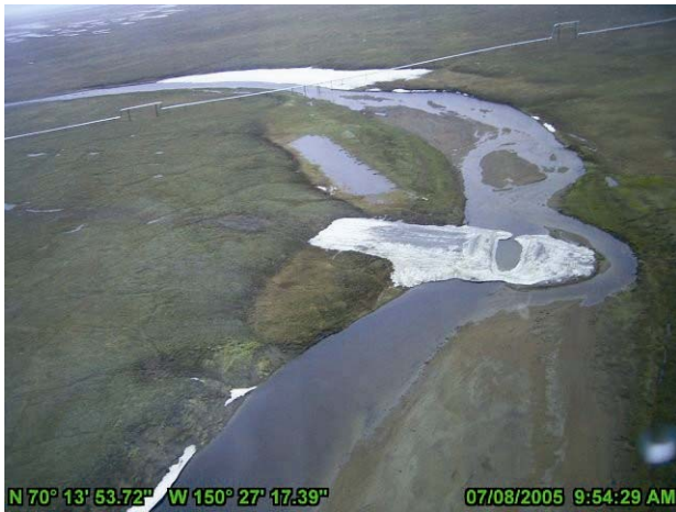
Photo 4-34 Kachemach River Ice Bridge after breakup with remnants of the ice road still in place, July 8, 2005
