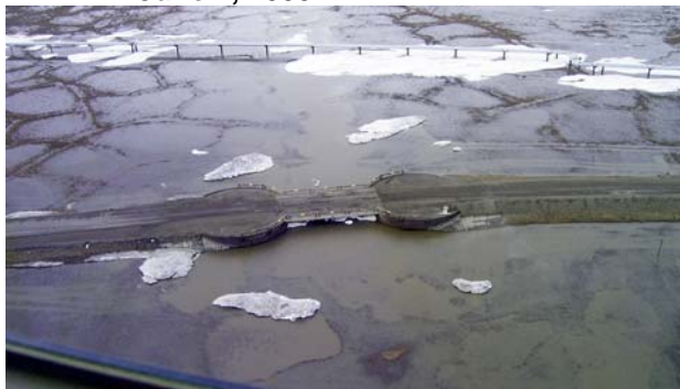
Photo 4-20 Conditions during peak stage at 62-foot swale bridge, June 2, 2005
