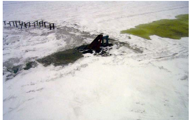
Photo 4-5 Sakoonang channel pipe bridge on CD3 pipeline, May 22, 2005
