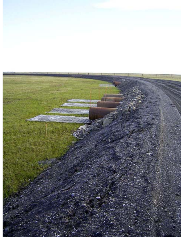
Photo 4-25 CD4 road alignment after recession of flood at the south Paleo culvert battery, July 10, 2005
