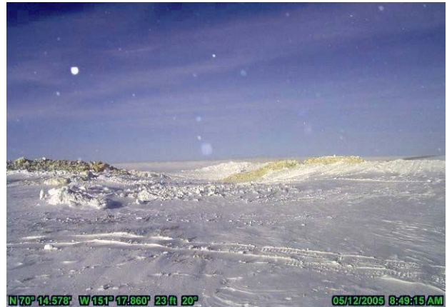
Photo 5-26 Ublutuoch River Ice Bridge prior to breakup with the ice road essentially removed from the drainage channel, May 12, 2005
