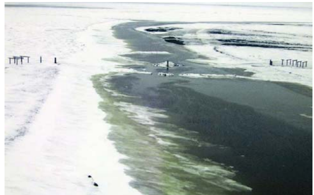
Photo 4-12 Ulamnigiaq channel at CD3 pipeline bridge, May 20, 2005
