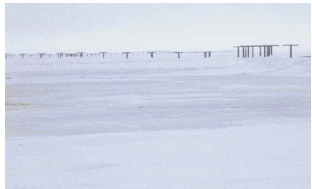
Photo 4-3 Tamayayak channel pipe bridge on CD3 pipeline, May 25, 2005
