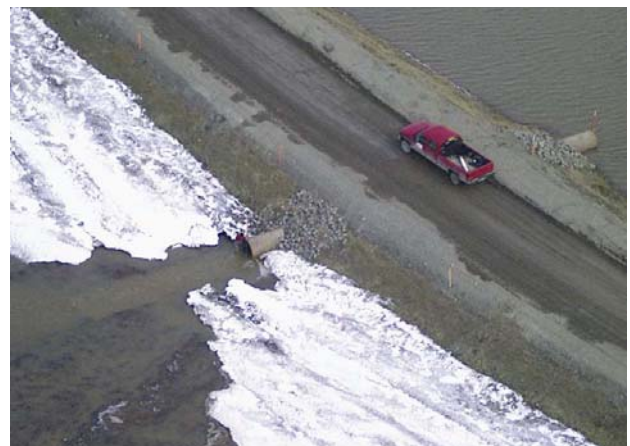
Photo 4-21 CD2 road culverts direct discharge measurement, June 2, 2005
