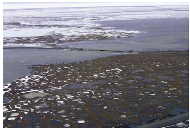
Photo 4-17 Peak stage at CD2 road and 452-foot swale bridge, May 31, 2005
