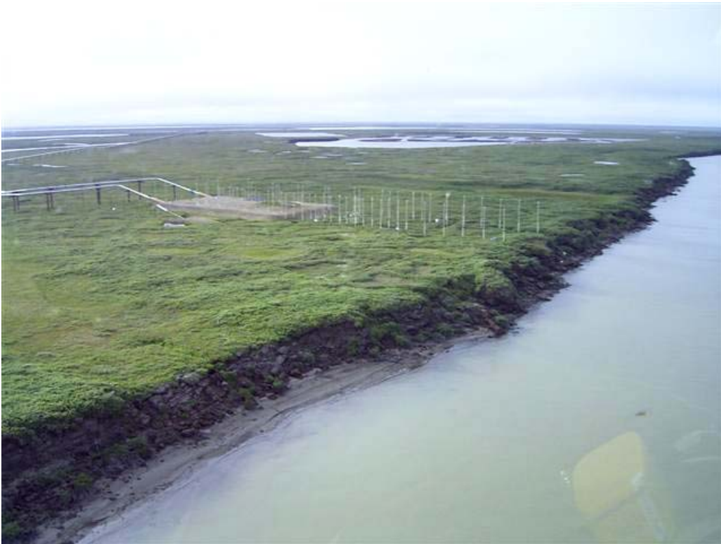
Photo A-7 HDD East, July 18, 2007. Bluff, thermosyphons, and pad at HDD East, looking southeast.
