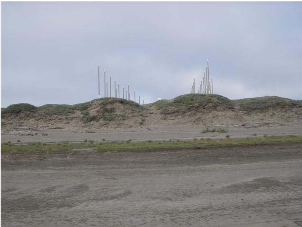
Photo A-4 HDD West, July 18, 2006. Bluff and thermosyphon at HDD West, looking west from Colville River.
