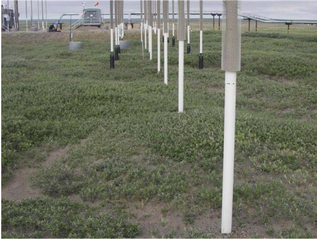
Photo A-5 HDD West, July 18, 2007. Thermosyphons, pads, and facilities at HDD West, looking west.
