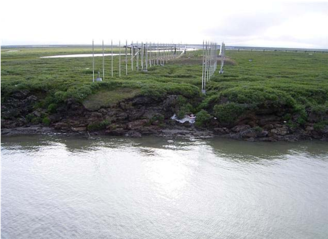
Photo A-8 HDD East, July 18, 2007. Bluff, thermosyphons, pad, and pipeline at HDD East, looking east.
