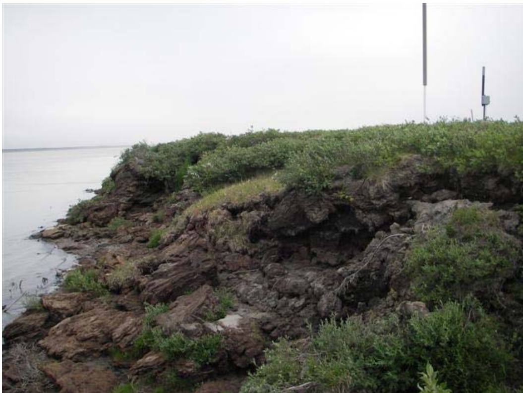
Photo A-10 HDD East, July 18, 2007. Bluff and northern thermosyphons at HDD East, looking north.
