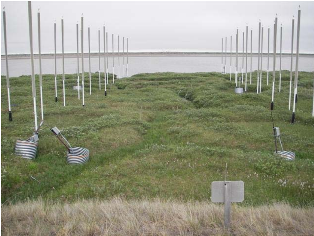
Photo A-9 HDD East, July 18, 2007. Thermosyphons and polygon trough at HDD East, looking west.
