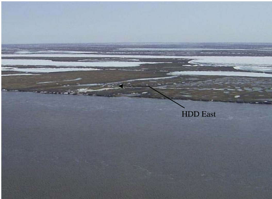
Photo A-6 HDD East, June 6, 2007. Bluff, thermosyphons, pad, and pipeline at HDD East 2 days after peak stage, looking east.
