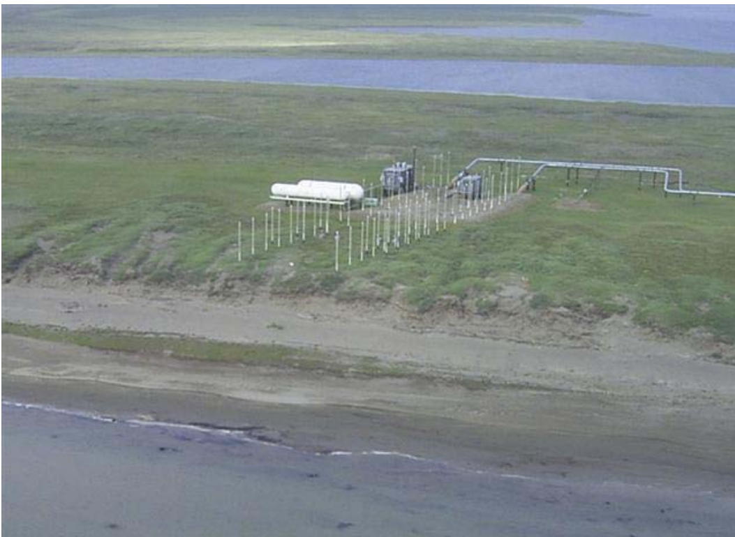
Photo A-2 HDD West, July 18, 2007. Bluff, thermosyphons, and pad at HDD West, looking west.
