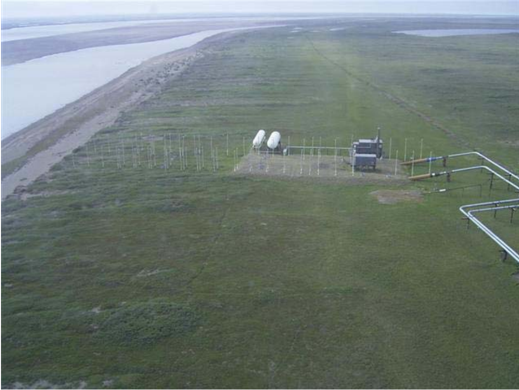
Photo A-3 HDD West, July 18, 2007. Bluff, thermosyphons, pad and pipeline at HDD West, looking south.
