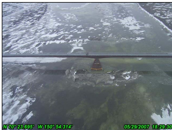
Photo 4-16 Early Floodwaters Reaching the Ulamnigaiq Pipeline Bridge Crossing, May 29, 2007
