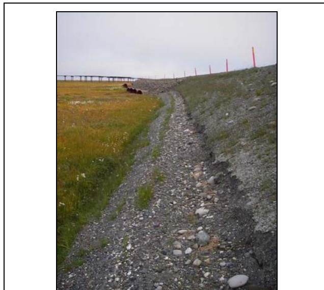
Photo 4-30 Fine Grained Sediment Settlement on Eastern Side of CD4 Road at STA 160+00 Looking South, August 28, 2007
