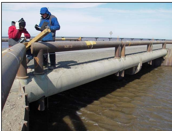
Photo 4-28 Discharge Measurement at 62-foot Swale Bridge, June, 5, 2007
