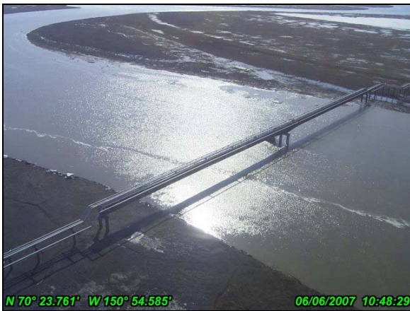
Photo 4-18 Tamayagiaq Pipeline Crossing After Peak Stage, June 6 2007
