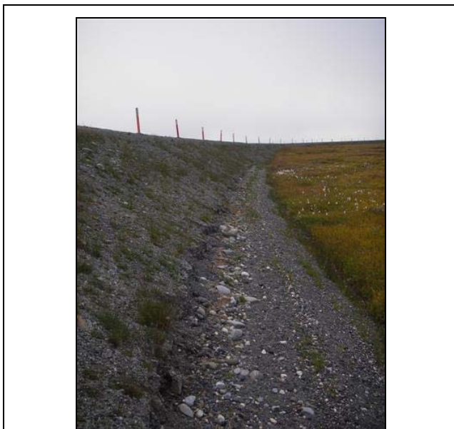
Photo 4-31 Fine Grained Sediment Settlement on Eastern Side of CD4 Road at STA 160+00 Looking North, August 28, 2007
