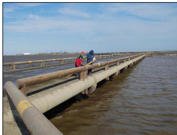
Photo 4-29 Discharge Measurement at 452-foot Swale Bridge, June, 5, 2007
