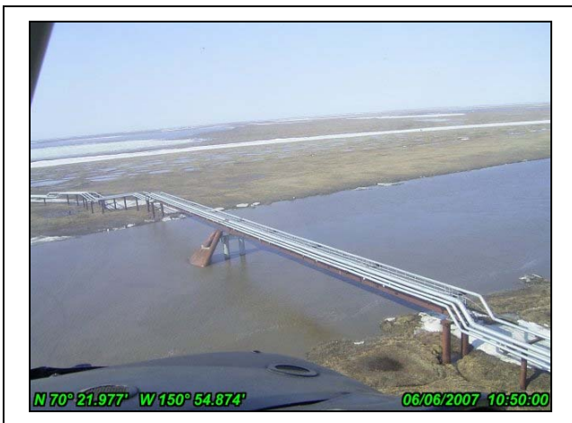
Photo 4-17 Sakoonang Pipeline Crossing After Peak Stage, June 6, 2007
