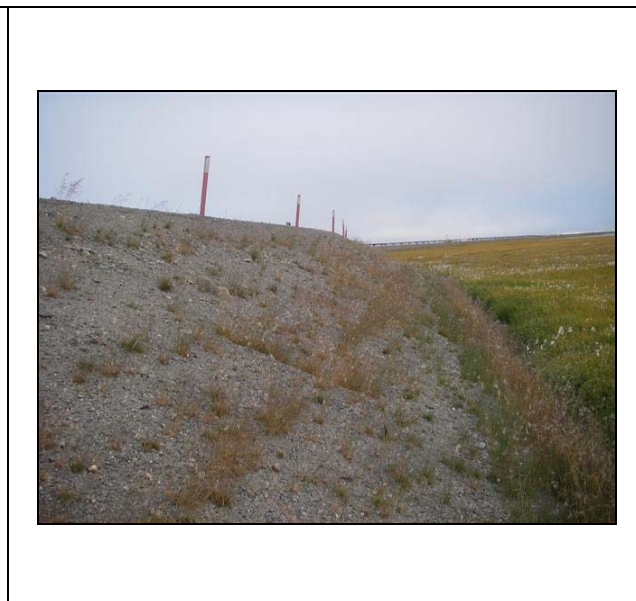
Photo 4-32 Western Side of CD4 Access Road after Breakup at STA 160+00 Looking South, August 28, 2007
