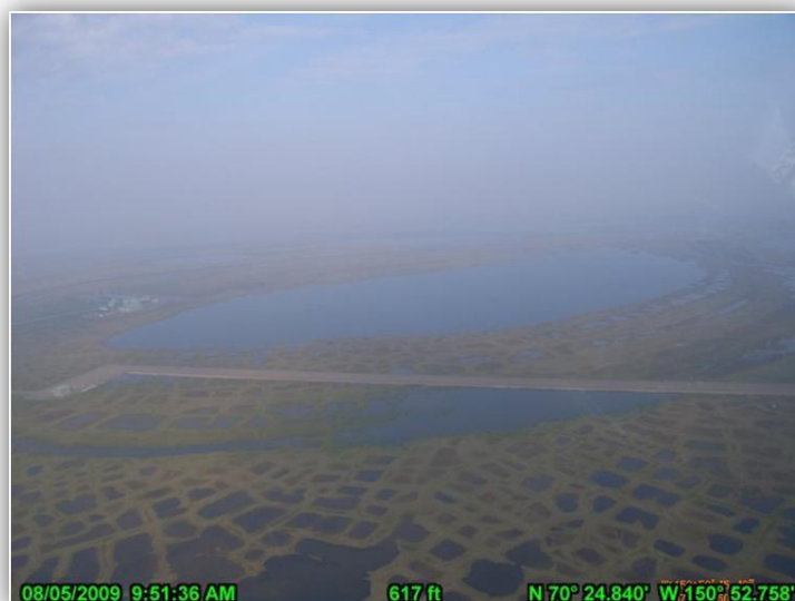
PHOTO 3.11: LAKE M9313 AND CD3 FACILITIES. AUGUST 5, 2009.
