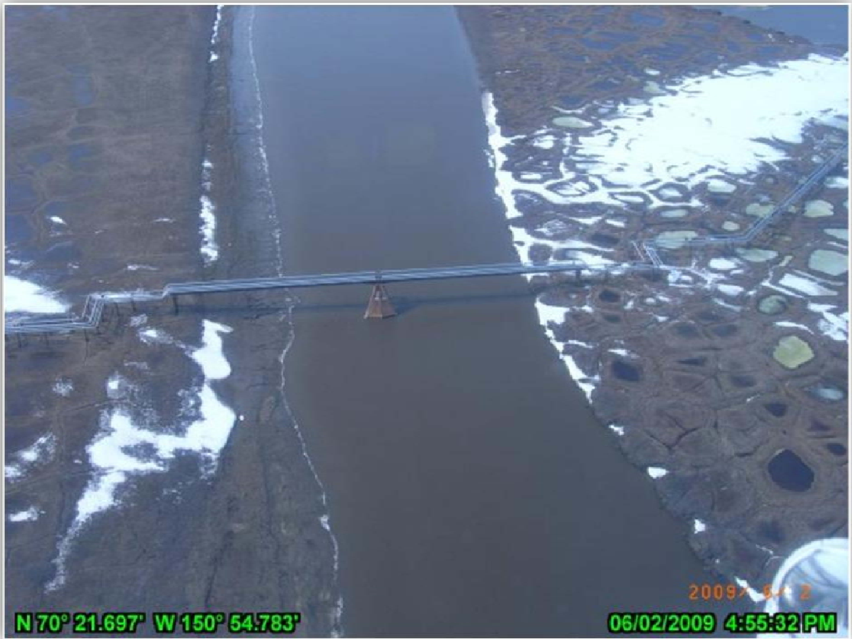
PHOTO 4.39: TAMAYAGIAQ PIPE BRIDGE. JUNE 2, 2009.
