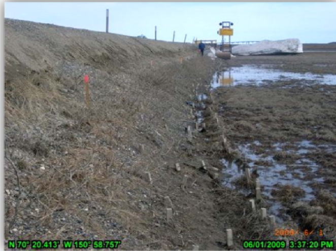
PHOTO 4.26: SOUTH SIDE OF CD2 ROAD BETWEEN THE SWALE BRIDGES. JUNE 1, 2009.
