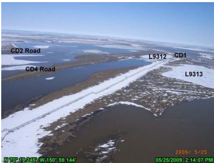
PHOTO 4.16: CD2 AND CD4 ACCESS ROADS. MAY 25, 2009.
