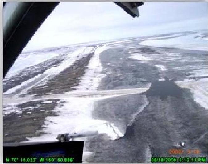
PHOTO 4.32: COLVILLE EAST CHANNEL ICE BRIDGE, LOOKING SOUTH. MAY 18, 2009.
