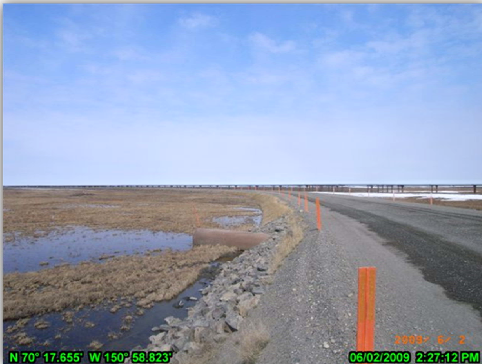
PHOTO 4.29: CD4 ACCESS ROAD NEAR CULVERT CD4-24. JUNE 2, 2009.
