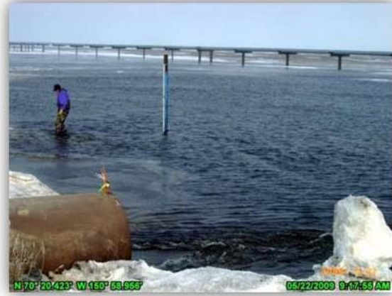
PHOTO 2.3: G4 AND CULVERT CD2-22. MAY 22, 2009
