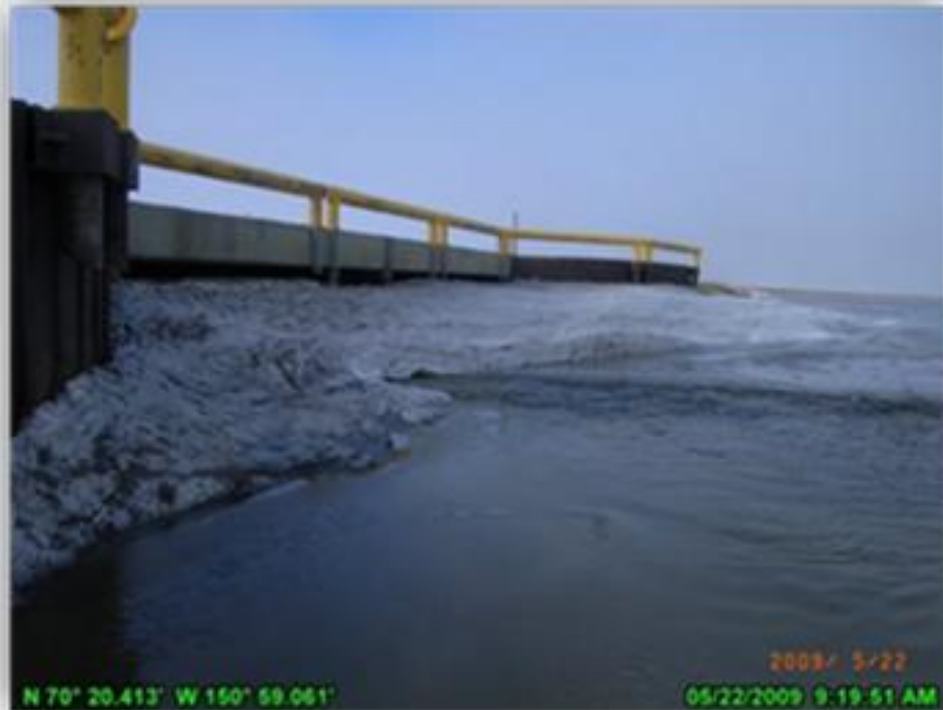
PHOTO 4.24: FLOW UNDER 62-FT SWALE BRIDGE, NORTH SIDE. MAY 22, 2009.
