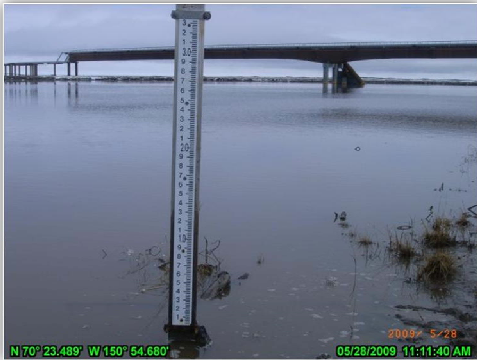
PHOTO 4.38: TAMAYAGIAQ PIPE BRIDGE AND GAGE TAM-B. MAY 28, 2009.
