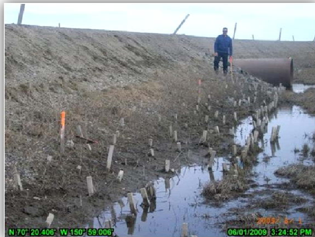
PHOTO 4.27: CD2 ROAD SOUTHEAST OF THE 62-FT SWALE BRIDGE. JUNE 1, 2009.
