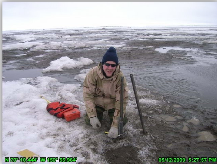
PHOTO 3.2: INSTALLATION OF PRESSURE TRANSDUCER, MON1D. MAY 12, 2009.
