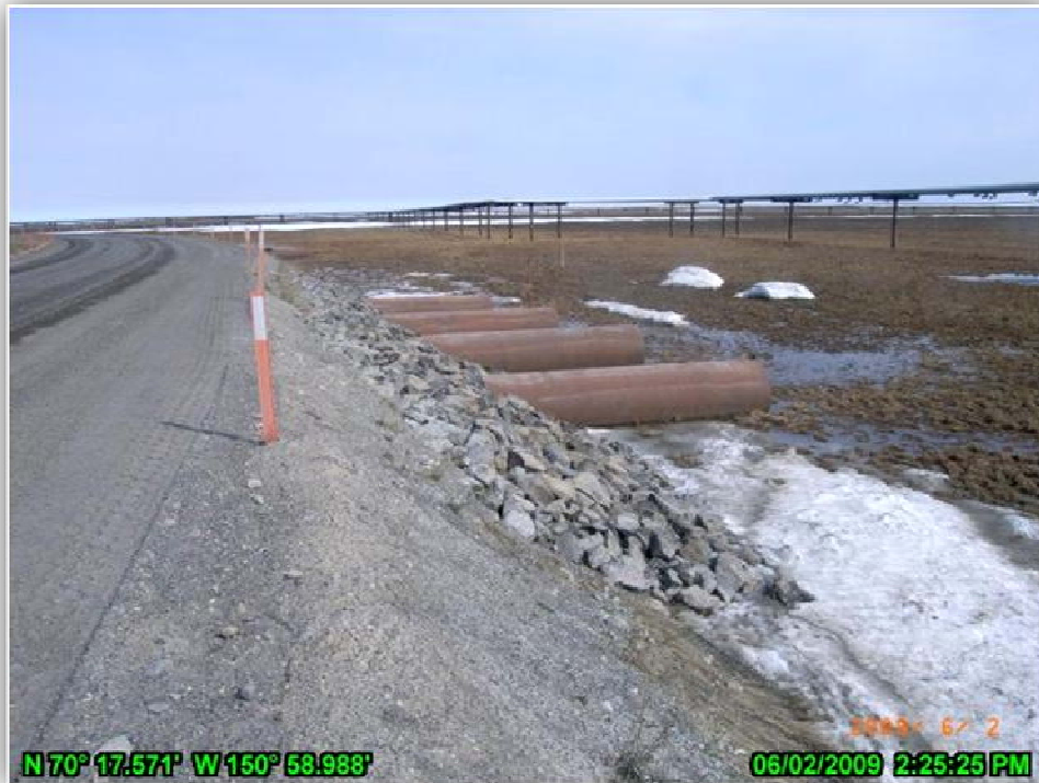
PHOTO 4.30: CD4 ACCESS ROAD CULVERT BATTERY CD4-29 THROUGH -32. JUNE 2, 2009.
