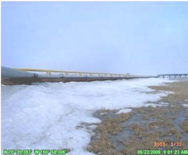
PHOTO 2.6: NORTH SIDE OF 452-FT SWALE BRIDGE; SNOW DAM. MAY 22, 2009.
