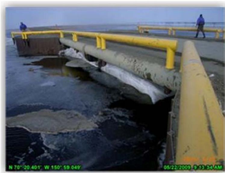
PHOTO 4.23: FLOW UNDER 62-FT SWALE BRIDGE, SOUTH SIDE. MAY 22, 2009.
