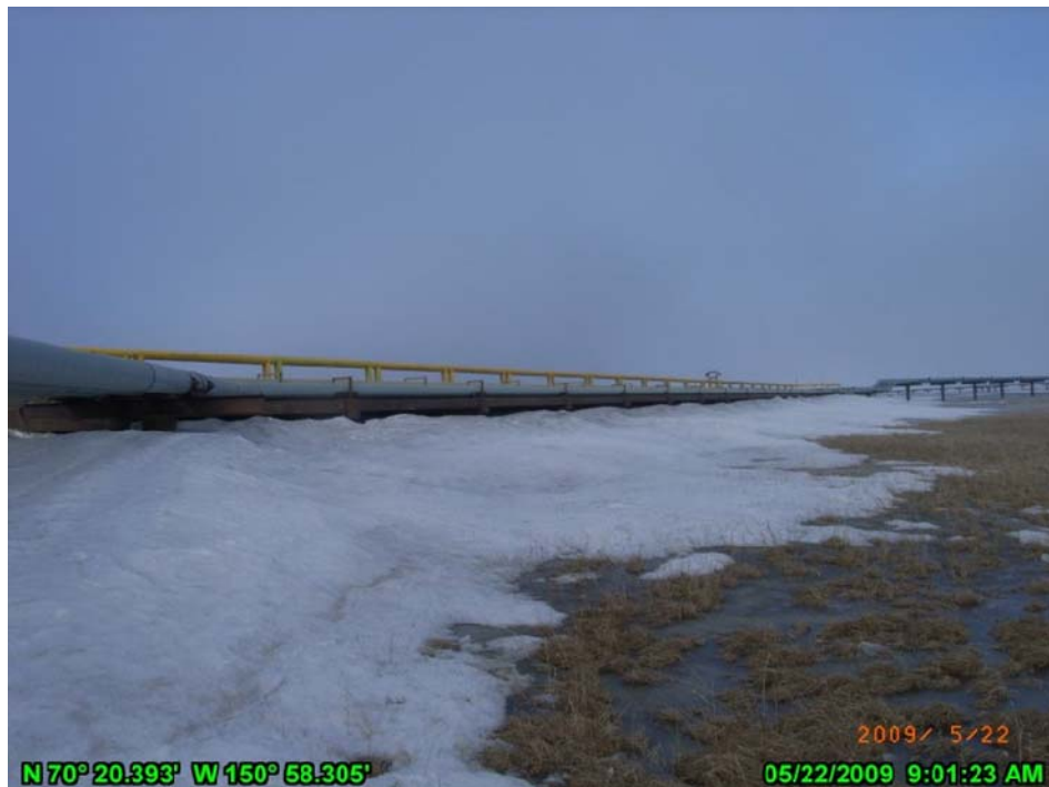
PHOTO 5.3: SNOW/ICE DAM ON UPSTREAM SIDE OF 452-FT SWALE BRIDGE. MAY 22, 2009.
