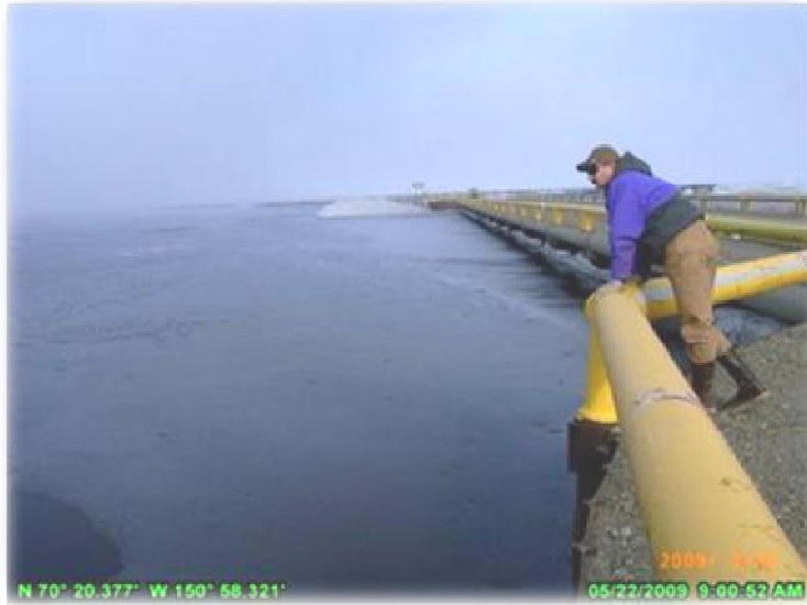
PHOTO 2.5: SOUTH SIDE 452-FT (LONG) SWALE BRIDGE; SNOW DAM PRESENT BLOCKING FLOW. MAY 22, 2009.
