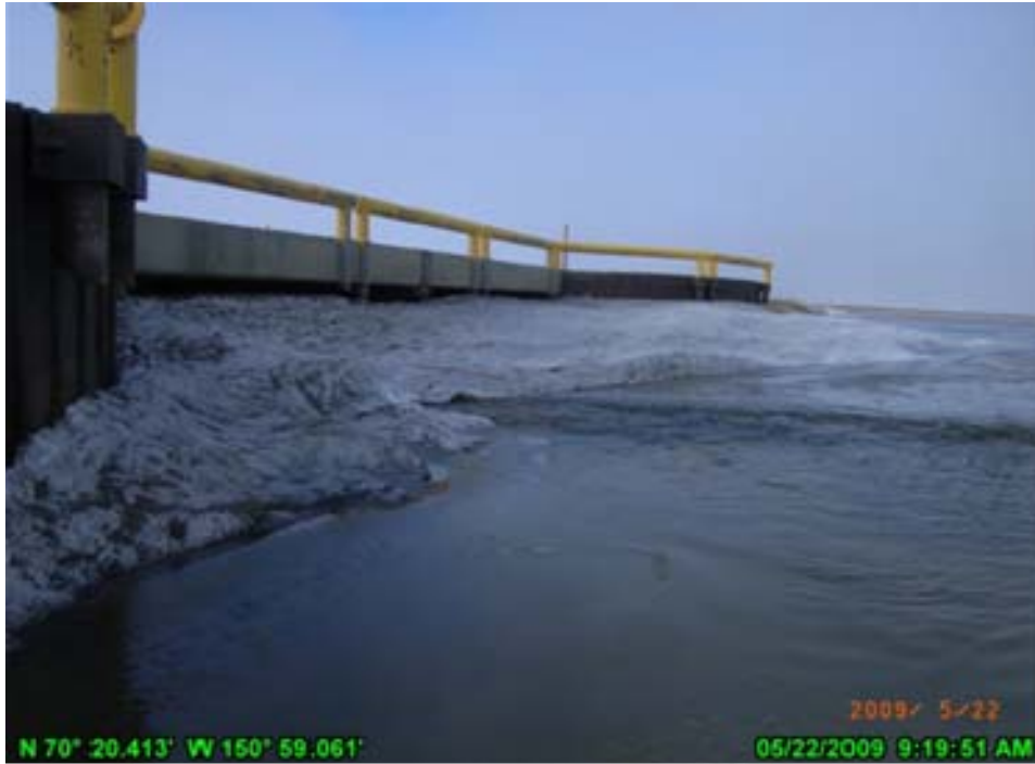
PHOTO 5.2: SNOW/ICE DAM ON UPSTREAM SIDE OF 62-FT SWALE BRIDGE. MAY 22, 2009.
