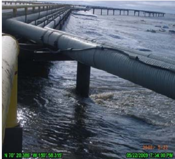
PHOTO 4.22: FAILURE OF ICE DAM UNDER THE 452-FT SWALE BRIDGE. MAY 22, 2009.
