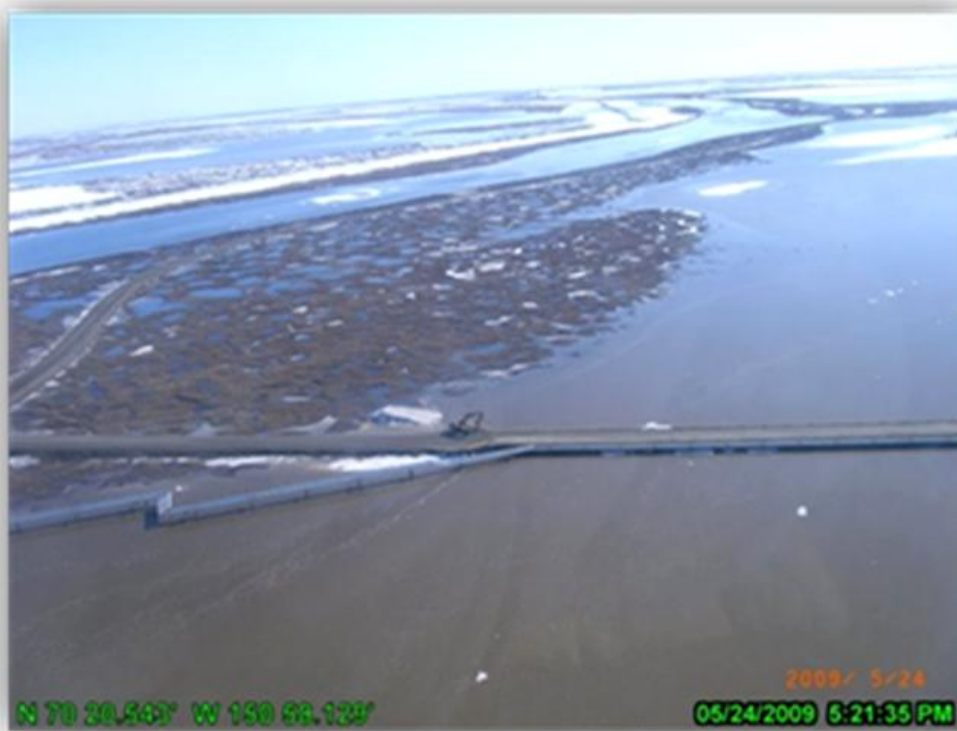
PHOTO 4.25: AERIAL VIEW, 452-FT SWALE BRIDGE. MAY 24, 2009.
