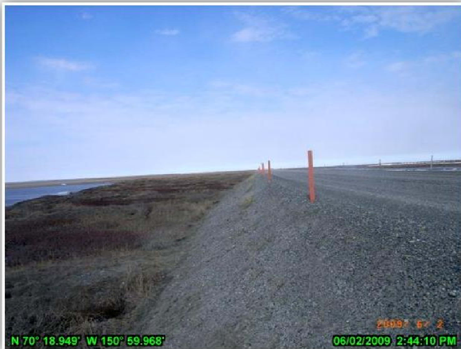
PHOTO 4.31: CD4 ACCESS ROAD. JUNE 2, 2009.
