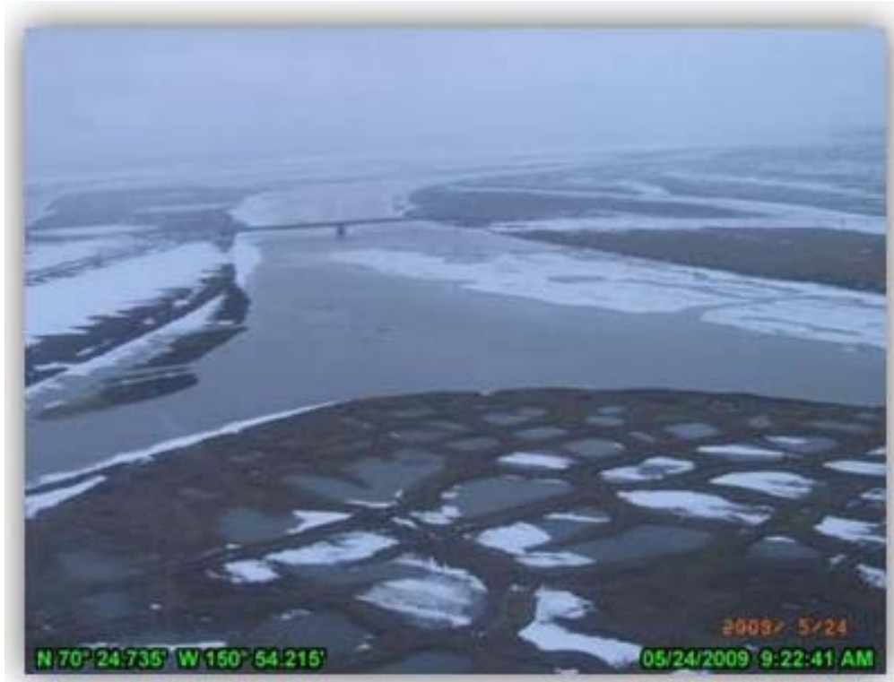
PHOTO 4.37: ULAMNIGIAQ PIPE BRIDGE. MAY 24, 2009.
