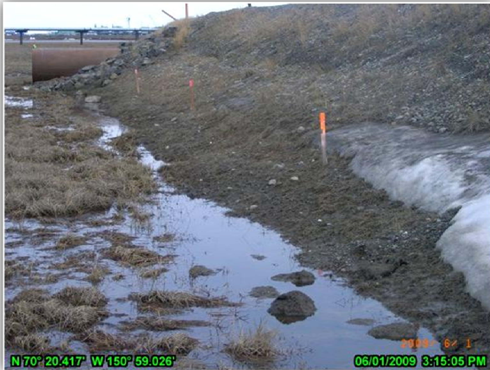
PHOTO 4.28: CD2 ROAD NEAR THE 62-FT SWALE BRIDGE. JUNE 1, 2009.
