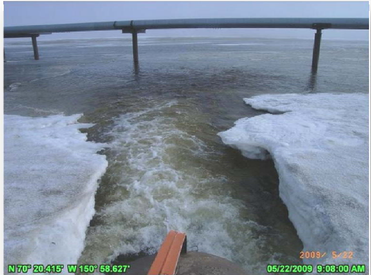
PHOTO 3.4: CULVERT CD2-24, CD2 ACCESS ROAD. MAY 22, 2009.
