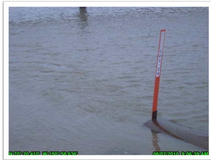
Photo 5.9: Near peak stage at culvert CD2-24; June 2, 2010.
