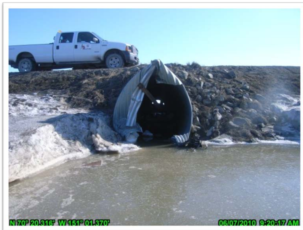
Photo 5.7: Damaged culvert CD2-9; June 7, 2010.
