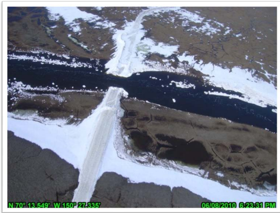
Photo 4.49: Kachemach River ice bridge breached and ice rafts observed in channel, looking east; June 8, 2010.
