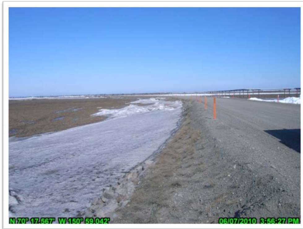
Photo 4.43: CD4 road prism looking east, vicinity of CD4; June 7, 2010.
