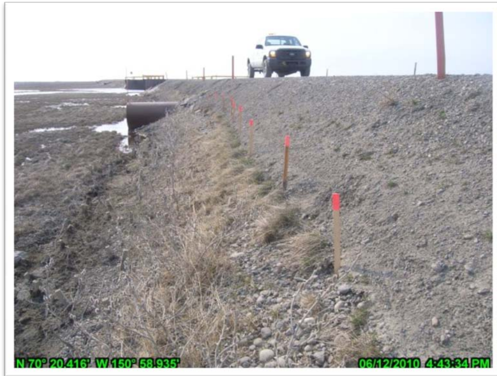
Photo 4.39: Orange lath used to indicate maximum elevation of erosion line along CD2 road; June 12, 2010.
