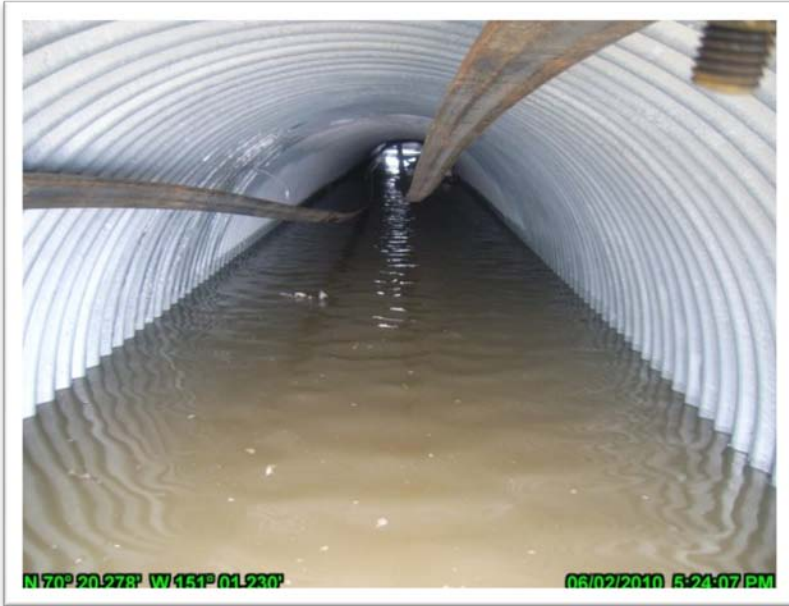
Photo 5.4: Interior CD2 road culvert CD2-10 showing smooth sleeve tie anchors inside CMP culvert; June 2, 2010.
