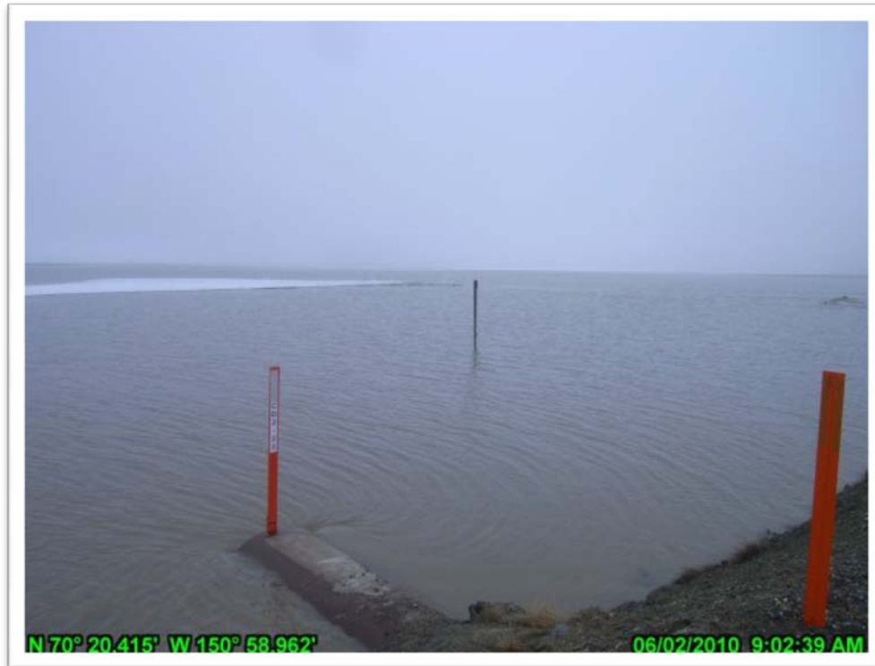
Photo 5.8: Near peak stage at culvert CD2-22; June 2, 2010.
