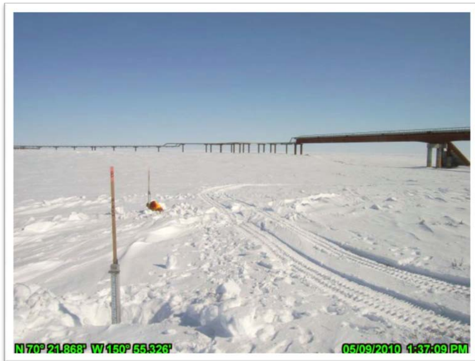
Photo 4.51: Installation of gages pre-breakup, Sagoonang Channel pipeline crossing; May 9, 2010.
