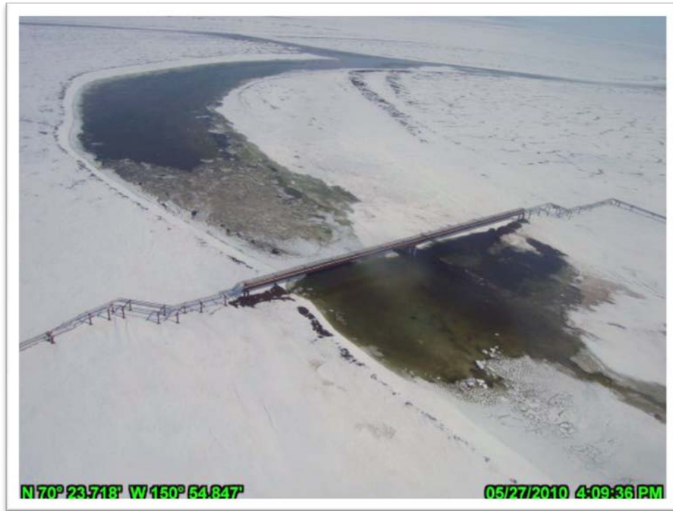
Photo 4.53: Initial floodwater passing under Tamayayak Channel pipeline bridge, looking northeast; May 27, 2010.
