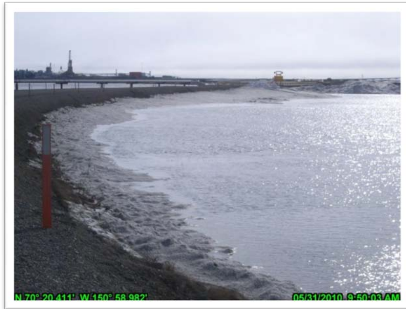
Photo 4.20: Floodwaters at CD2 road near swale bridges; May 31, 2010.
