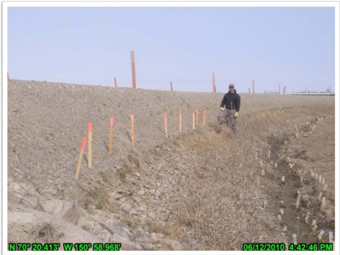
Photo 4.38: Fine-grained sands washed away due to floodwater erosion, CD2 road near long swale bridge; June 12, 2010.
