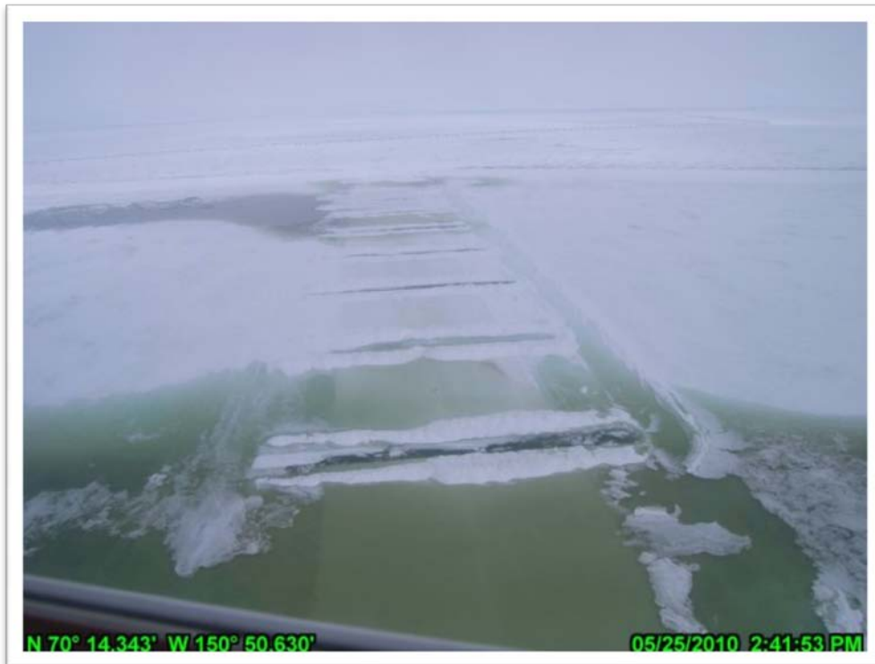
Photo 4.45: Water in slots of East Channel ice bridge, looking east; May 25, 2010.
