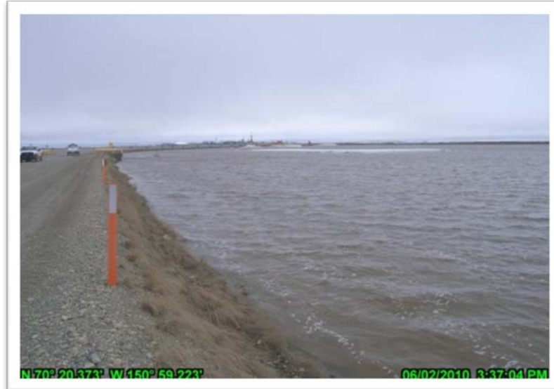
Photo 4.22: Floodwaters along CD2 road near peak stage; June 2, 2010.
