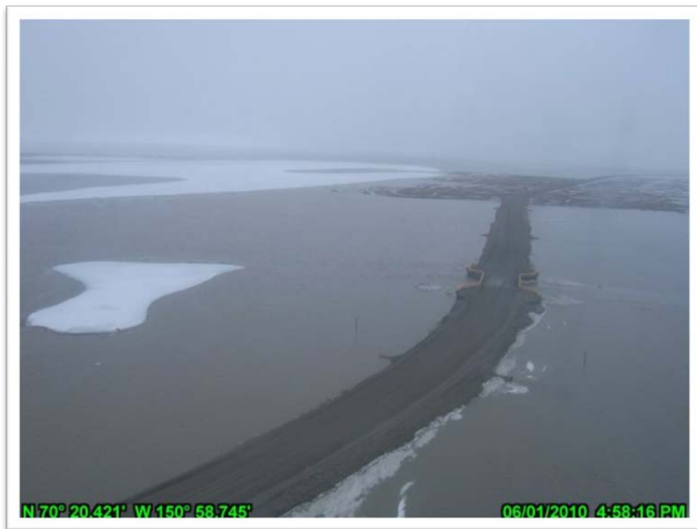
Photo 4.36: Aerial view of 62-ft swale bridge; June 1, 2010.
