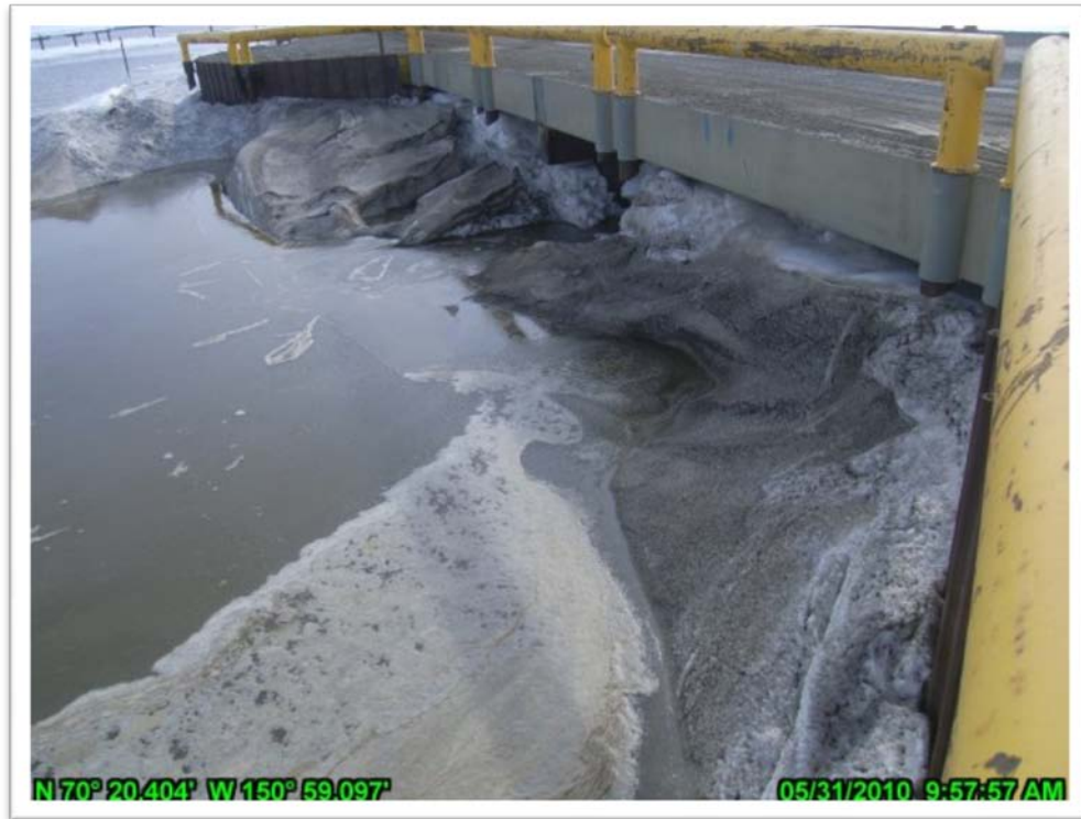
Photo 4.35: 62-ft swale bridge blocked by snow; May 31, 2010.
