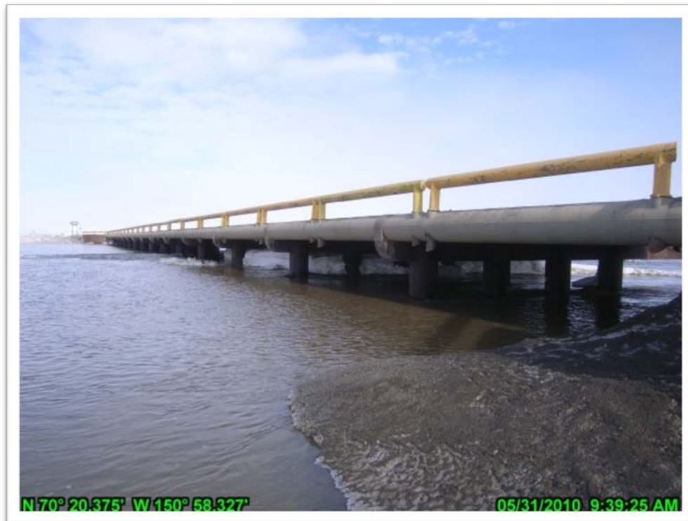
Photo 4.34: Snow blockage beneath 452-ft swale bridge; May 31, 2010.
