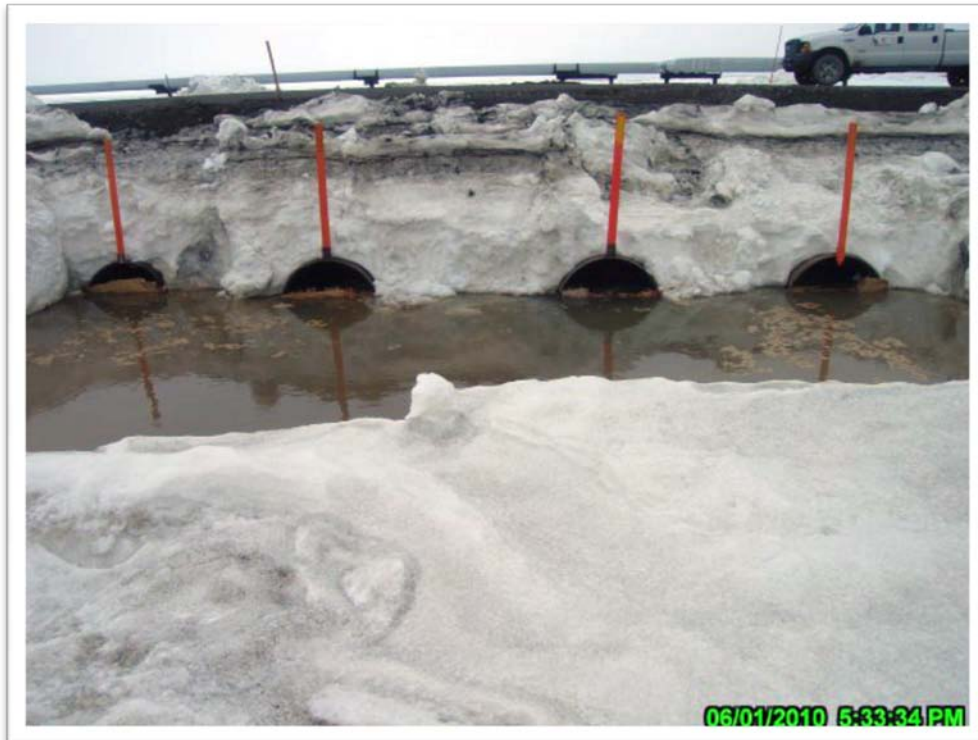
Photo 5.5: Plywood blockage of culverts CD2-7 through CD2-7 upstream along CD2 road; June 1, 2010.
