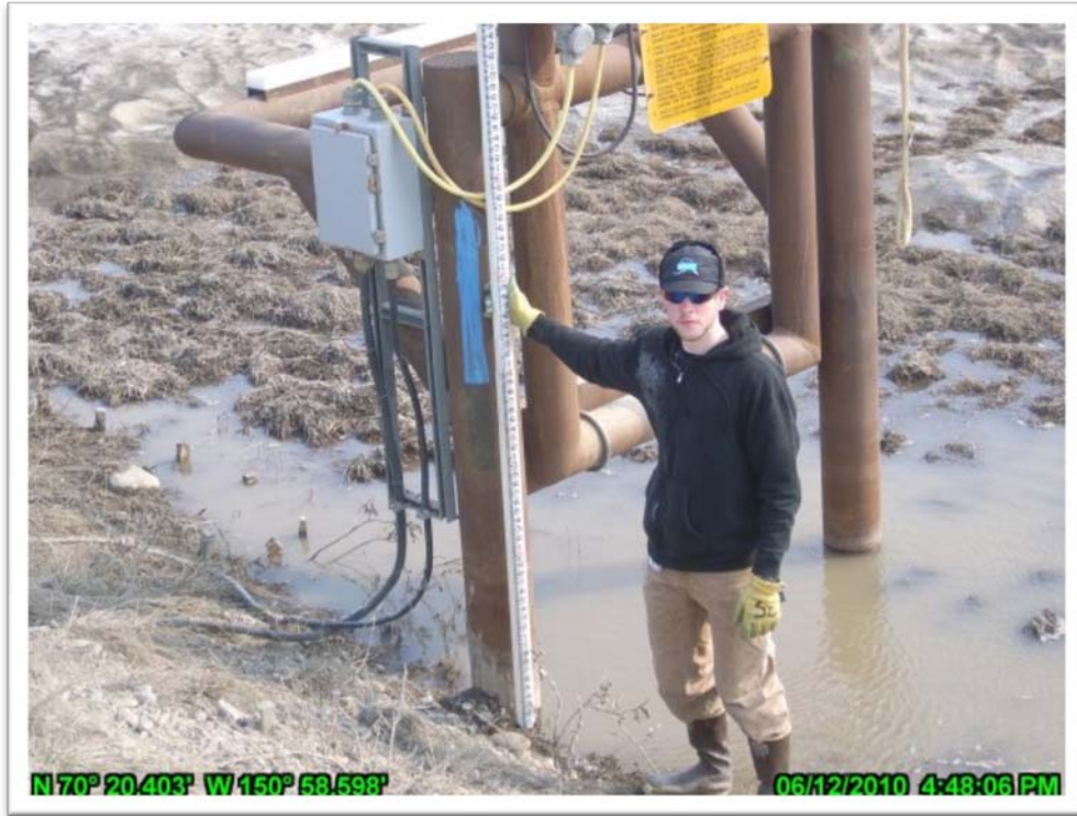
Photo 4.41: High water mark (bottom of blue chalk line) on runway signal light CD2 road at base of road prism; June 12, 2010.
