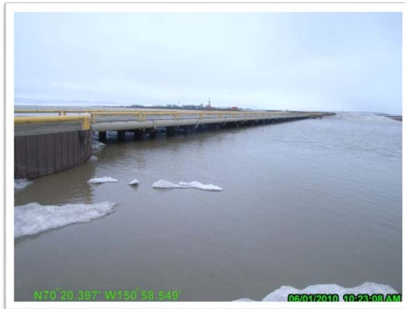
Photo 4.37: 452-ft swale bridge one day prior to peak stage; June 1, 2010.
