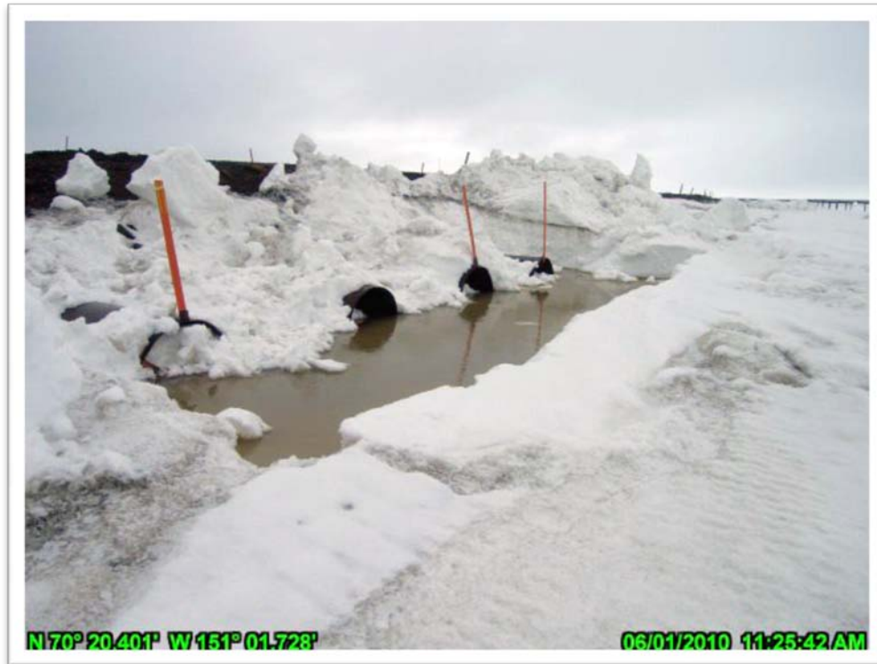
Photo 5.6: Snow blockage, downstream side CD2 road culverts CD2-4 through CD2-7; June 1, 2010.
