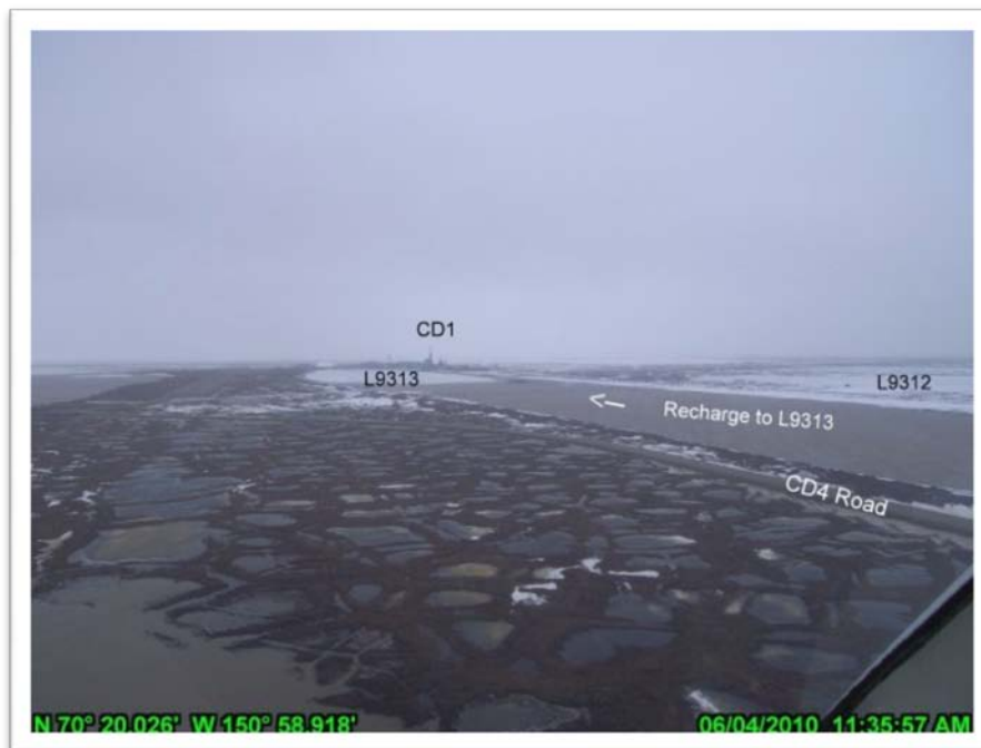
Photo 4.30: Floodwater recharge Lake L9313; June 4, 2010.
