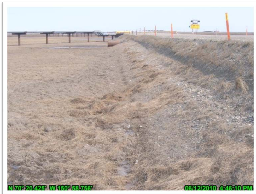
Photo 4.40: Erosion of the north side of the CD2 road prism in the vicinity of culvert CD2-24; June 12, 2010.
