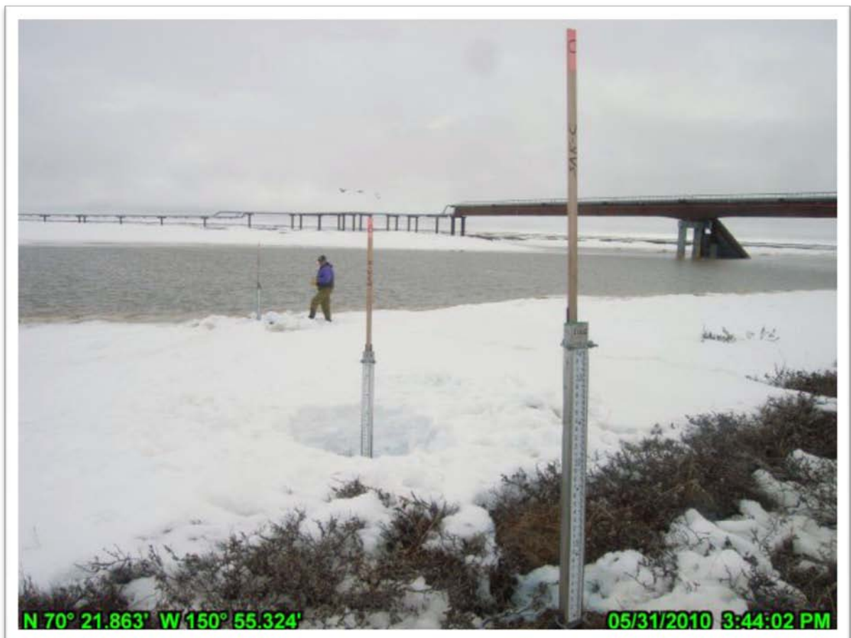
Photo 2.7: Monitoring gages at Sakoonang Channel crossing looking east; May 31, 2010.
