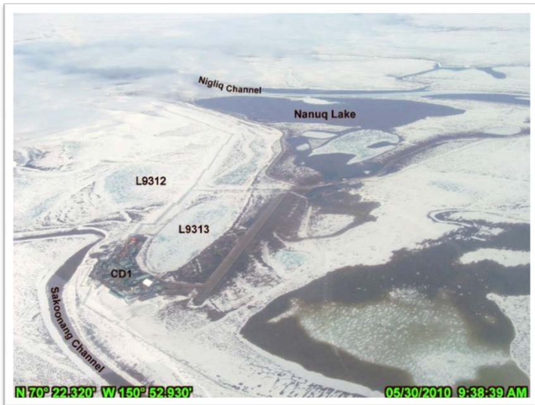
Photo 4.16: Nigliq Channel floodwaters reach Nanuq Lake; CD1 shown in foreground; May 30, 2010.
