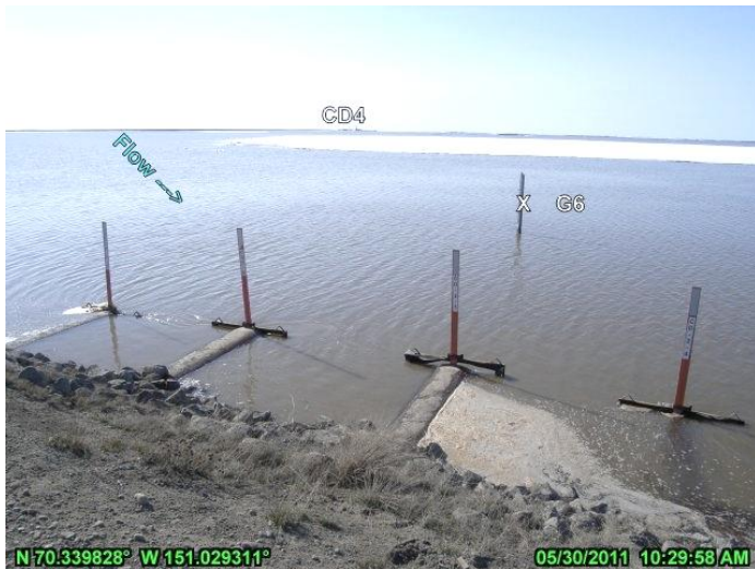
PHOTO 4.52: CD2 ROAD CULVERTS NEAR G6 PASSING FLOW AFTER PEAK STAGE, LOOKING UPSTREAM (SOUTH); MAY 30, 2011
