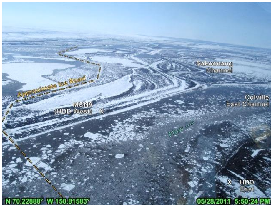
PHOTO 4.12: ICE FLOES IN THE VICINITY OF MON9 (HDD)—THE RESULT OF A MAJOR ICE JAM RELEASE UPSTREAM OF MON1, LOOKING DOWNSTREAM (NORTHWEST); MAY 28, 2011
