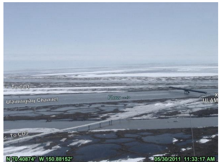
PHOTO 4.96: ULAMNIGIQ PIPELINE CROSSING JUST AFTER PEAK STAGE, LOOKING SOUTH; MAY 30, 2011
