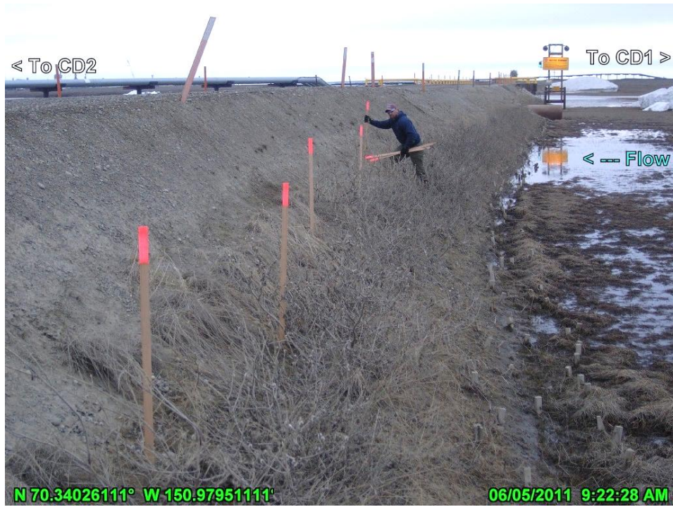
PHOTO 4.72: EROSION SURVEY CD2 ROAD POST-BREAKUP, BETWEEN SWALE BRIDGES, LOOKING EAST; JUNE 5, 2011
