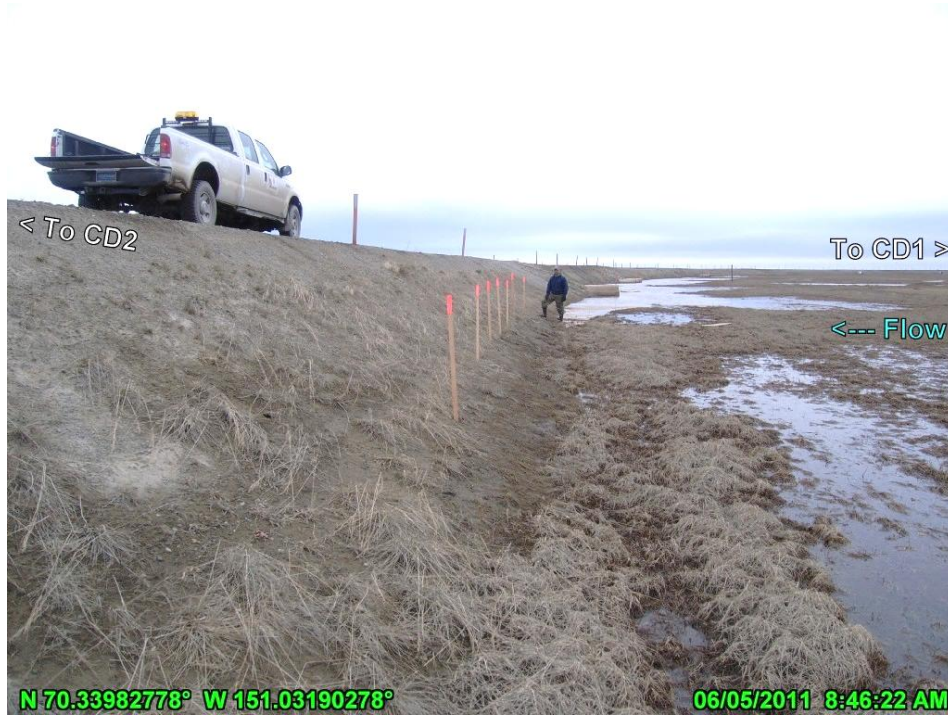
PHOTO 4.70: EROSION SURVEY OF CD2 ROAD PRISM POST-BREAKUP, LOOKING EAST; JUNE 5, 2011
