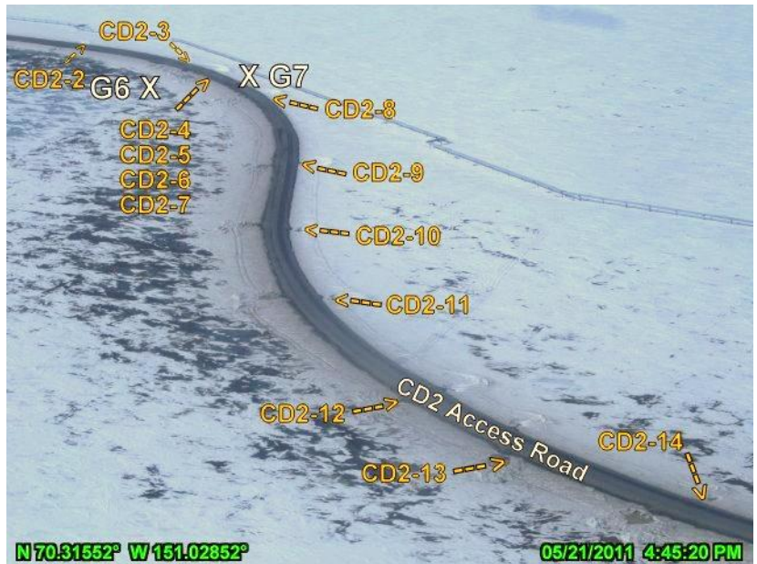
PHOTO 2.12: CD2 ROAD CULVERTS CLEARED OF SNOW AT INLETS AND OUTLETS PRIOR TO BREAKUP TO FACILITATE PASSAGE OF FLOOD FLOWS AND SEDIMENT, LOOKING NORTHWEST; MAY 21, 2011
