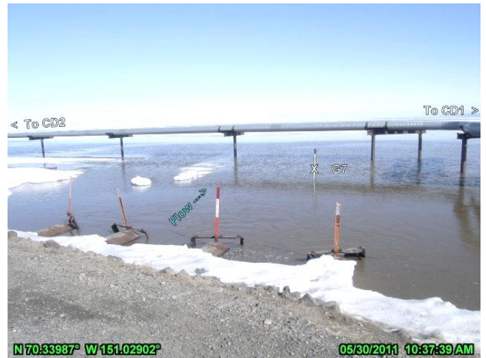
PHOTO 4.53: CD2 ROAD CULVERTS NEAR G7 PASSING FLOW AFTER PEAK STAGE, LOOKING DOWNSTREAM (NORTH); MAY 30, 2011
