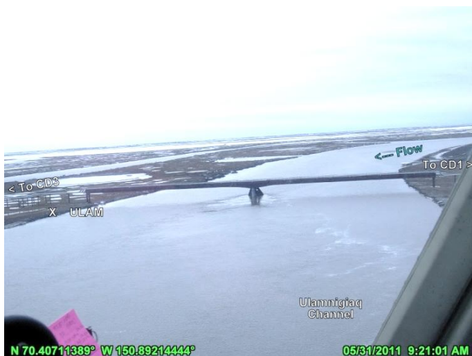
PHOTO 4.99: ULAMNIGLAQ PIPELINE CROSSING AS BREAKUP FLOWS RECEDE, LOOKING WEST; MAY 31, 2011
