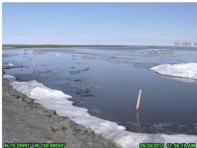
PHOTO 4.57: CD4 ROAD CULVERTS IN THE VICINITY OF G15 (LAKE M9525) AFTER PEAK STAGE, LOOKING NORTHEAST; MAY 30, 2011
