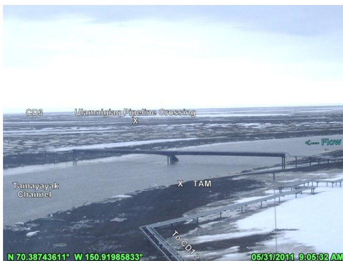
PHOTO 4.98: TAMAYYAK PIPELINE CROSSING AS BREAKUP FLOWS RECEDE, LOOKING NORTHEAST; MAY 31, 2011
