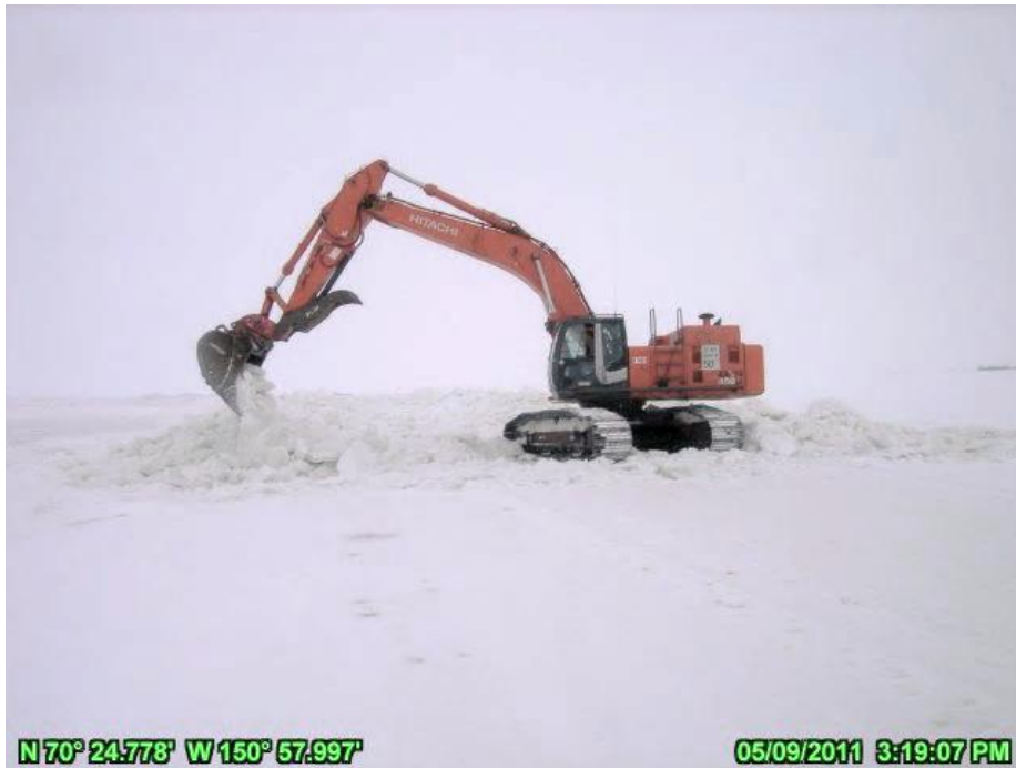
PHOTO 4.76: ICE ROAD CROSSINGS ARE DUG OUT PRIOR TO BREAKUP TO FACILITATE THE PASSAGE OF FLOOD FLOW; TAMAYAYAK ICE ROAD CROSSING; MAY 9, 2011
