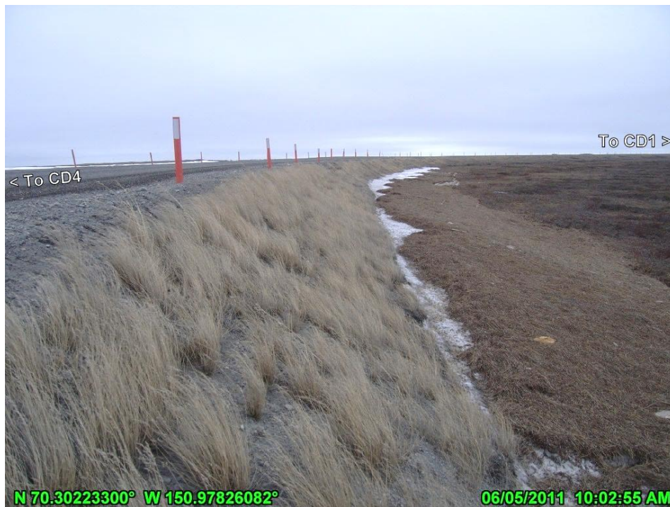
PHOTO 4.75: EROSION SURVEY CD4 ROAD, ORGANIC DEBRIS LEFT FROM RECEDED WATER AT TOE OF ROAD PRISM, LOOKING NORTH; JUNE 5, 2011
