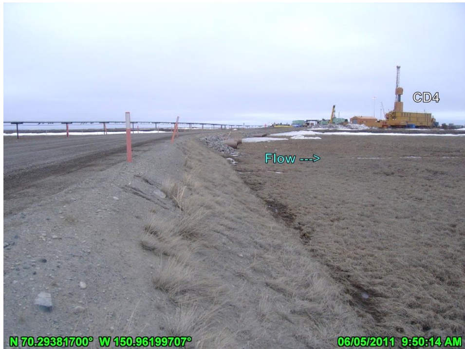
PHOTO 4.73: EROSION SURVEY CD4 ROAD PRISM POST-BREAKUP, LOOKING SOUTH; JUNE 5, 2011
