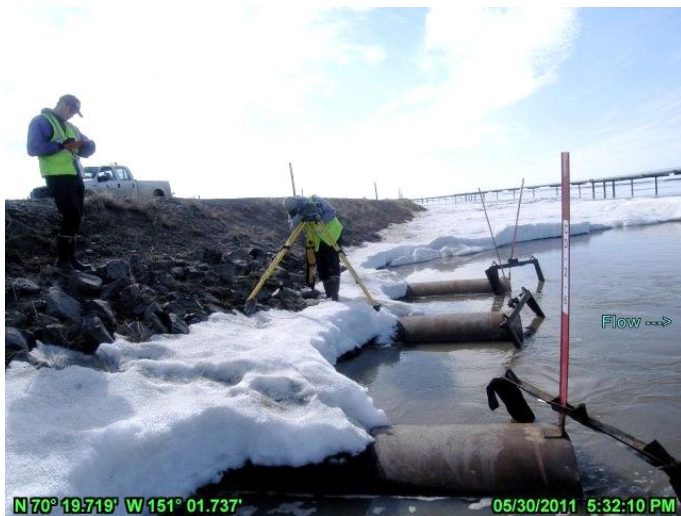
PHOTO 5.14: CULVERTS NEAR G3-G4, TAILWATER JUST AFTER PEAK STAGE; MAY 30, 2011
