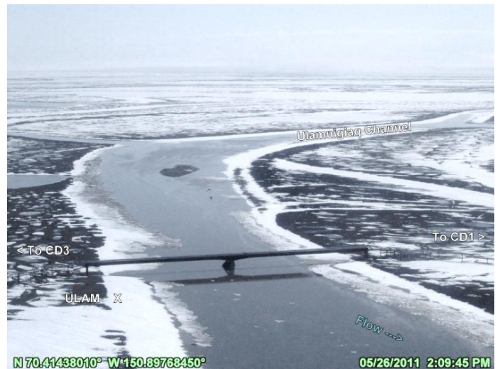
PHOTO 4.88: ULAMNIGIAQ PIPELINE CROSSING AS BREAKUP FLOWS PROGRESS, LOOKING UPSTREAM (SOUTHEAST); MAY 26, 2011
