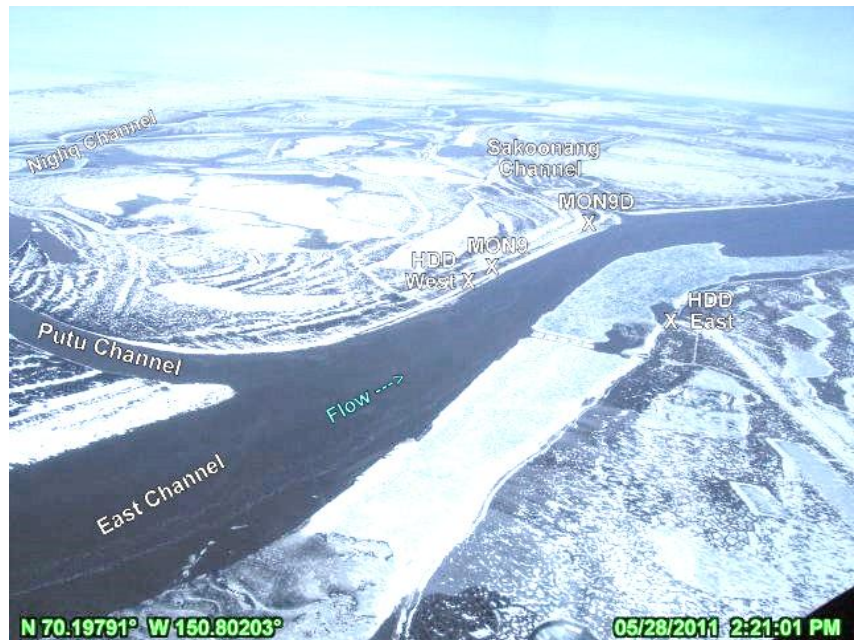
PHOTO 5.3: RIBBON ICE NEAR MON9, LOOKING DOWNSTREAM (NORTHWEST); MAY 28, 2011
