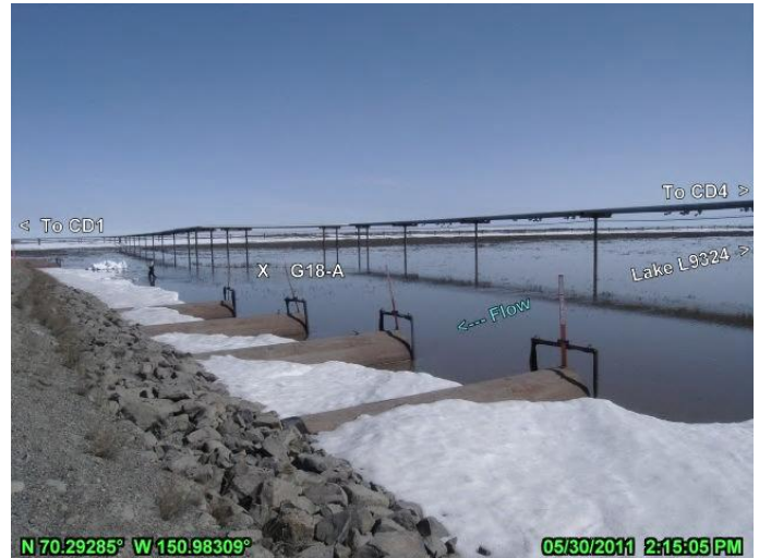
PHOTO 4.60: CD4 ROAD CULVERTS IN THE VICINITY OF G18 (LAKE L9324) AFTER PEAK STAGE, LOOKING WEST; MAY 30, 2011
