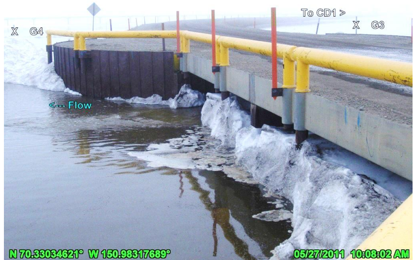
PHOTO 4.38: INITIAL FLOW THROUGH THE 62-FOOT SWALE BRIDGE, SNOW BLOCKAGE ON DOWNSTREAM (NORTH) SIDE, LOOKING EAST; MAY 27, 2011
