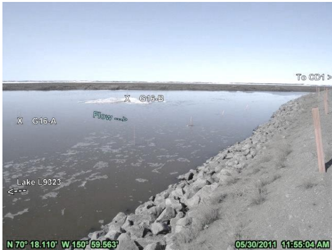
PHOTO 5.16: CULVERTS NEAR G15-G16, HEADWATER JUST AFTER PEAK STAGE; MAY 30, 2011
