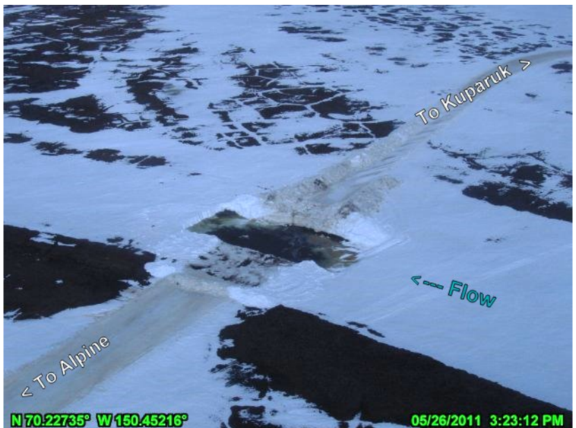
PHOTO 2.13: ICE ROAD CROSSING AT THE KACHEMACH RIVER SLOTTED PRIOR TO BREAKUP TO FACILITATE THE PASSAGE OF FLOOD FLOW, LOOKING NORTHEAST; MAY 26, 2011
