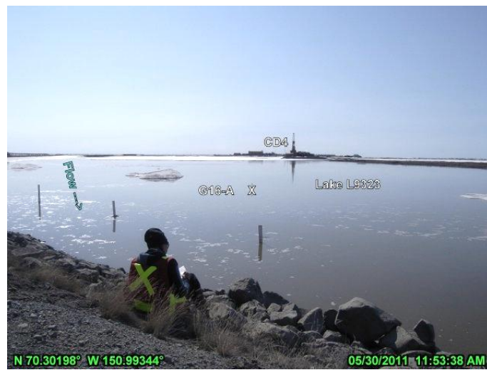
PHOTO 4.58: CD4 ROAD CULVERTS IN THE VICINITY OF G16 (LAKE L9323) AFTER PEAK STAGE, LOOKING SOUTHWEST; MAY 30, 2011
