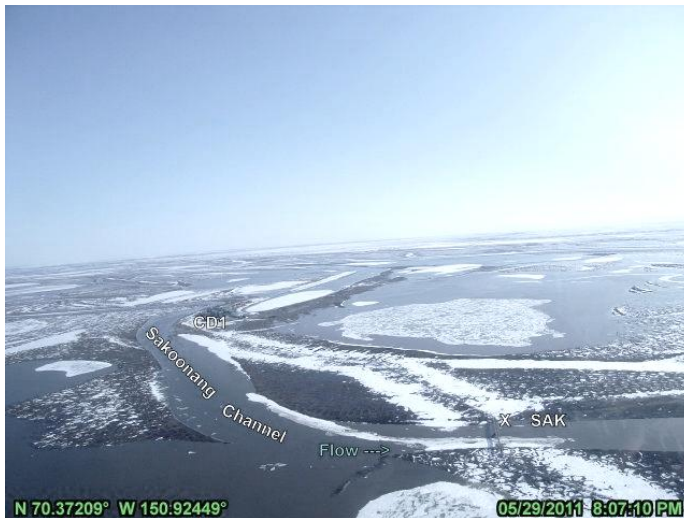
PHOTO 4.92: SAKOONGANG PIPELINE CROSSING JUST PRIOR TO PEAK STAGE, LOOKING UPSTREAM (SOUTHEAST); MAY 29, 2011
