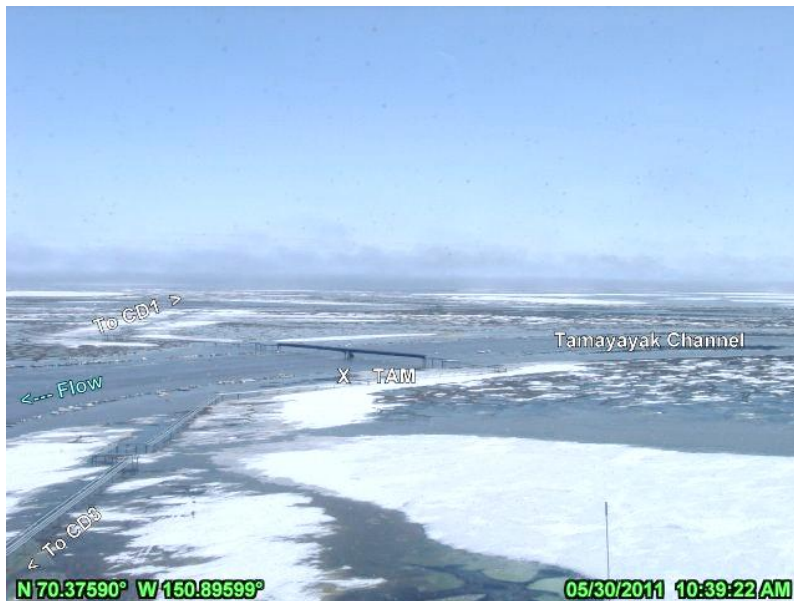
PHOTO 4.94: TAMAYAYAK PIPELINE CROSSING JUST AFTER PEAK STAGE, LOOKING WEST; MAY 30, 2011
