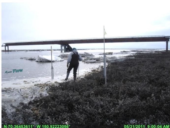
PHOTO 4.97: SAKOONGANG PIPELINE CROSSING AS BREAKUP FLOWS RECEDE, LOOKING NORTHEAST; MAY 31, 2011
