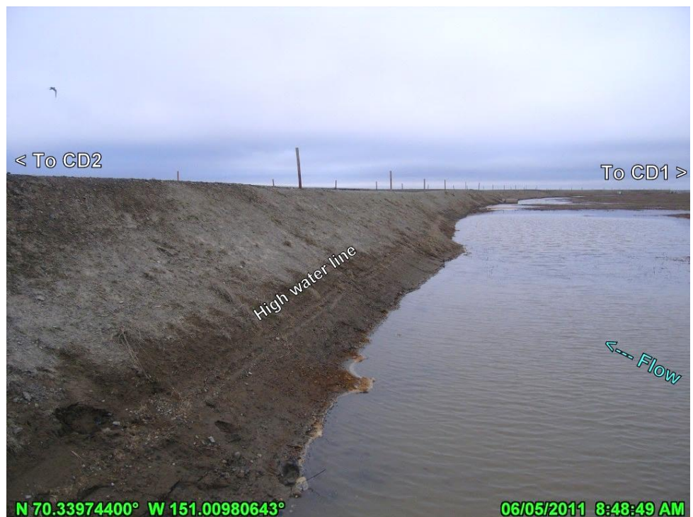
PHOTO 4.69: FINE-GRAINED MATERIAL REMOVED FROM ROAD PRISM, SOUTH SIDE OF CD2 ROAD, LOOKING EAST; JUNE 5, 2011
