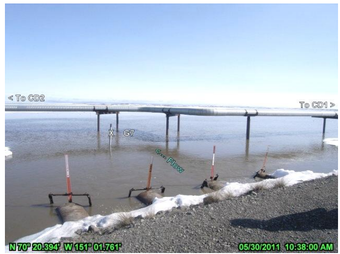
PHOTO 5.15: CULVERTS NEAR G6-G7, TAILWATER JUST AFTER PEAK STAGE; MAY 30, 2011
