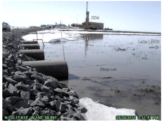
PHOTO 5.17: CULVERTS NEAR G17-G18, TAILWATER JUST AFTER PEAK STAGE; MAY 30, 2011
