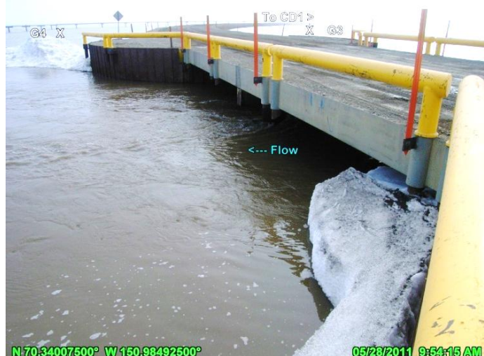
PHOTO 4.40: FLOW PASSING MOSTLY UNIMPEDED BY SNOW THROUGH THE 62-FOOT SWALE BRIDGE, DOWNSTREAM (NORTH) LOOKING WEST; MAY 28, 2011
