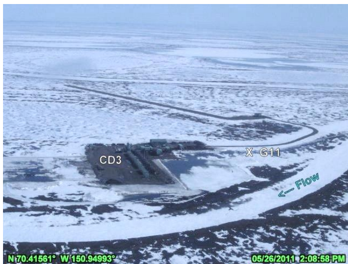
PHOTO 4.34: LOCAL MELT NEAR CD3 FACILITIES, LOOKING EAST; MAY 26, 2011
