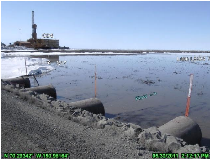
PHOTO 4.59: CD4 ROAD CULVERTS IN THE VICINITY OF G17 (LAKE L9323) AFTER PEAK STAGE, LOOKING EAST; MAY 30, 2011
