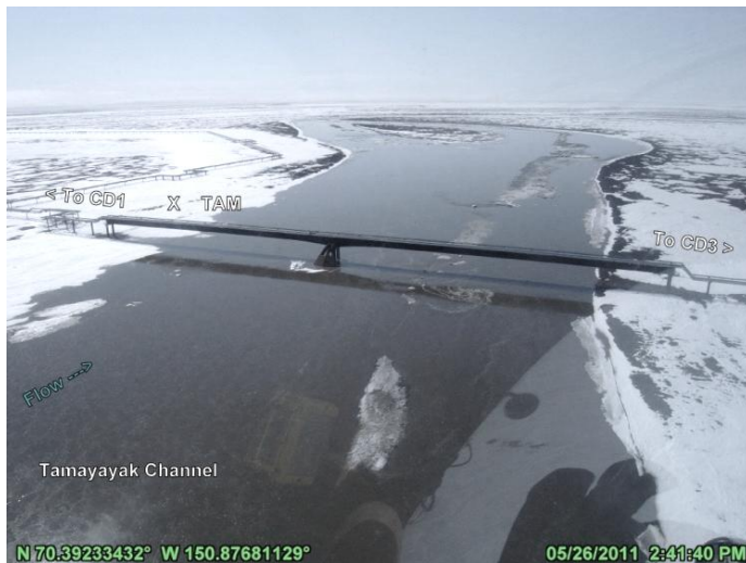
PHOTO 4.87: TAMAYAYAK PIPELINE CROSSING AS BREAKUP FLOWS PROGRESS, LOOKING DOWNSTREAM (WEST); MAY 26, 2011
