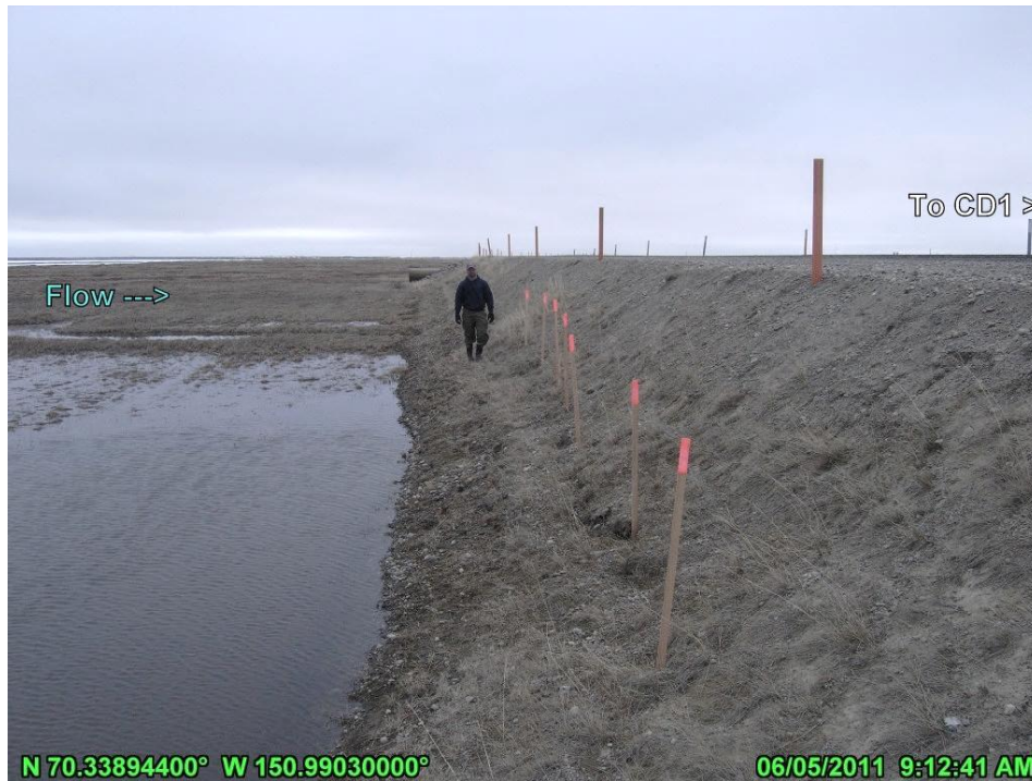
PHOTO 4.71: EROSION SURVEY CD2 ROAD PRISM POST-BREAKUP, LOOKING WEST; JUNE 5, 2011
