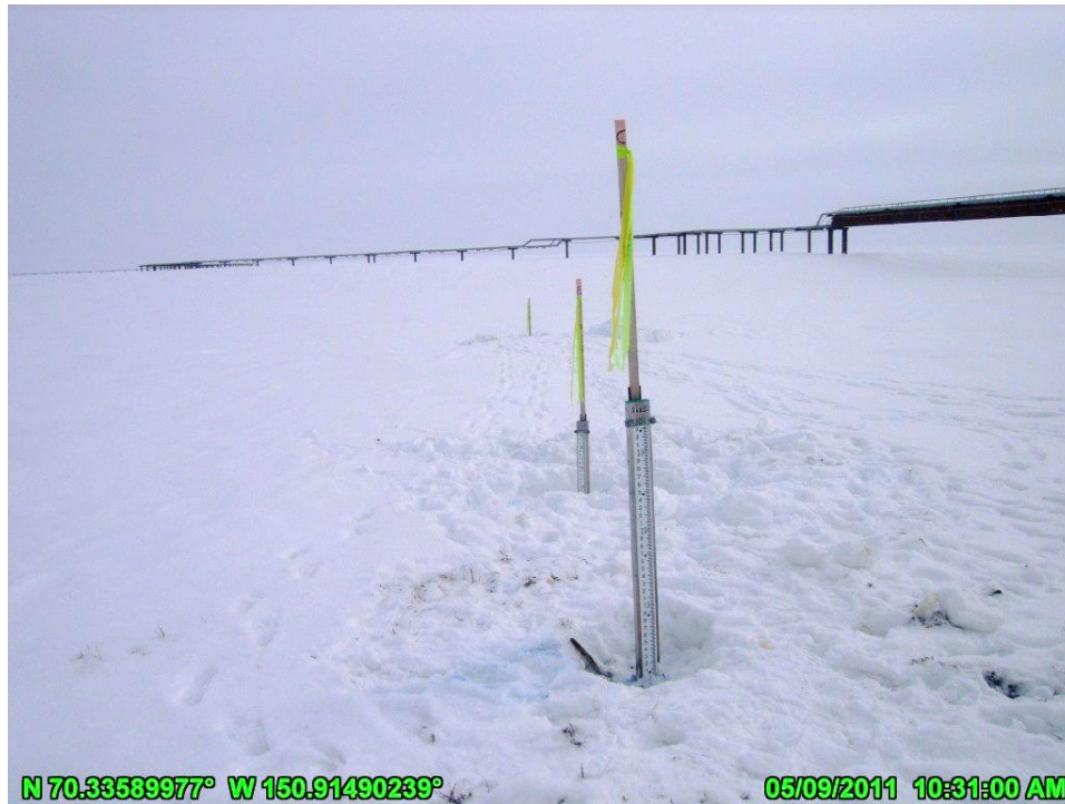
PHOTO 3.3: TEMPORARY INDIRECT-READ GAGES AT THE SAKOONANG PIPELINE CROSSING; GAGE A IS NEAREST TO THE CHANNEL CENTERLINE, LOOKING NORTHEAST; MAY 9, 2011
