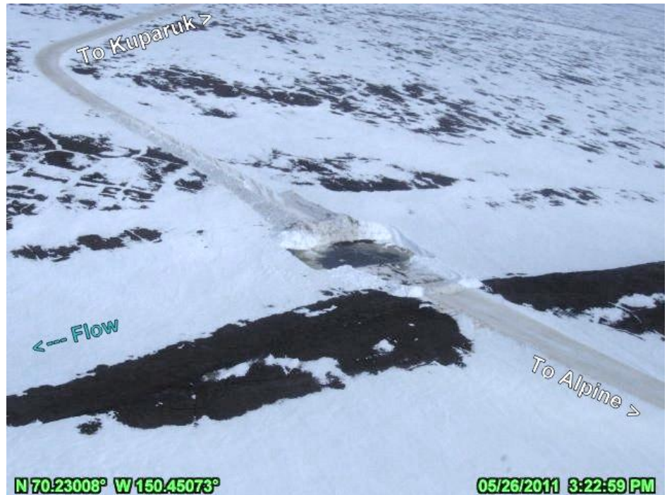
PHOTO 4.82: KACHEMACH RIVER ICE BRIDGE SLOTTED PRE-BREAKUP, LOOKING SOUTHEAST; MAY 26, 2011
