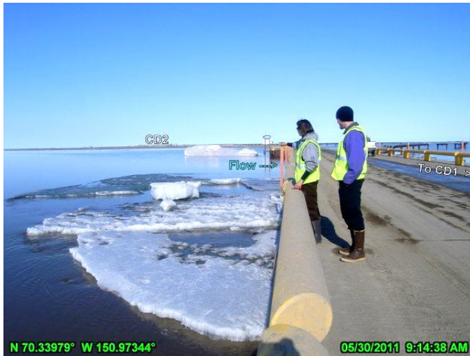
PHOTO 4.49: UPSTREAM (SOUTH) SIDE OF LONG SWALE BRIDGE AFTER PEAK STAGE, LOOKING WEST; MAY 30, 2011
