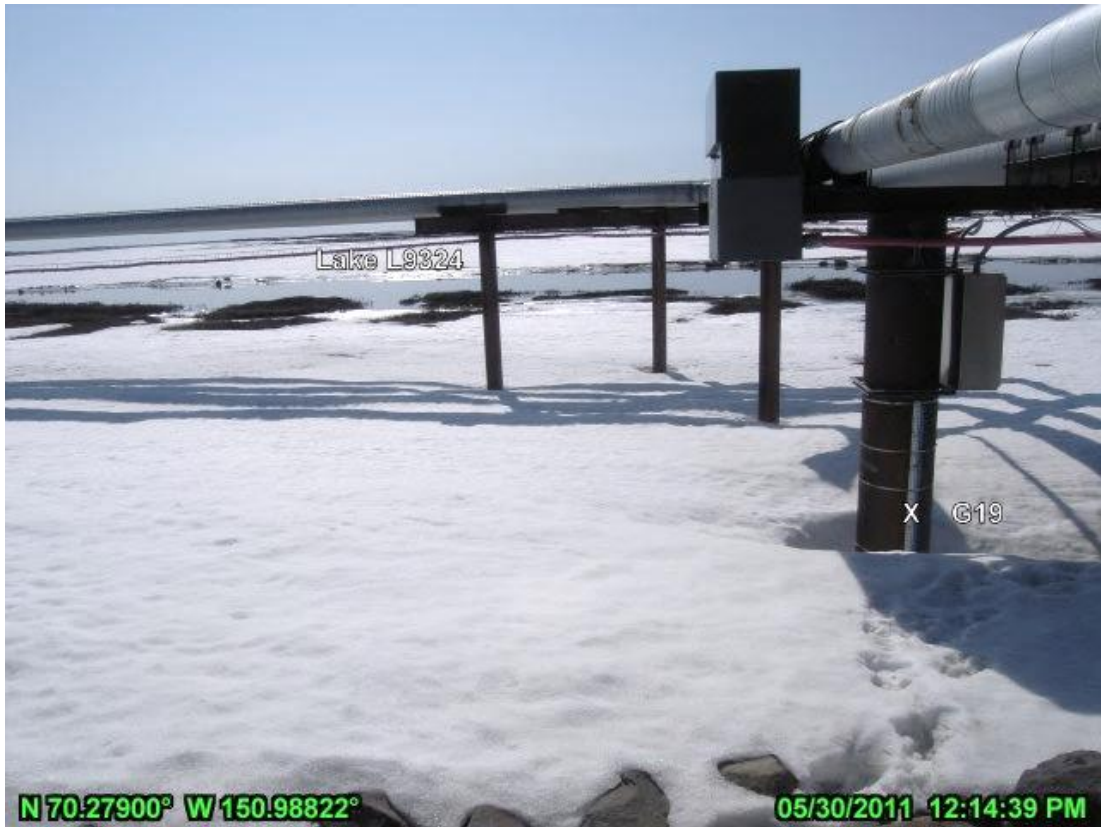
PHOTO 4.62: NO EVIDENCE OF BREAKUP FLOOD FLOW IN THE VICINITY OF G19 ON THE SOUTH SIDE OF CD4 PAD, LOOKING SOUTH; MAY 30, 2011
