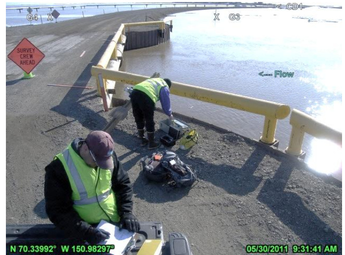
PHOTO 4.50: UPSTREAM (SOUTH) SIDE OF SHORT SWALE BRIDGE AFTER PEAK STAGE, LOOKING EAST; MAY 30, 2011
