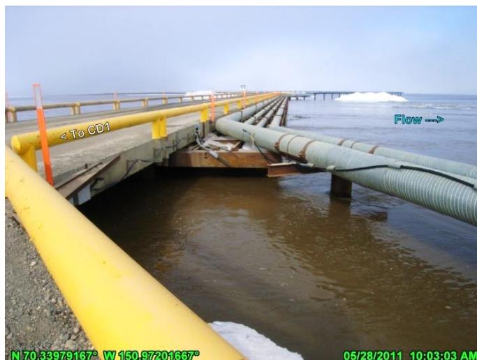
PHOTO 4.41: FLOW PASSING UNIMPEDED BY SNOW THROUGH THE 452-FOOT SWALE BRIDGE, DOWNSTREAM (NORTH) LOOKING EAST; MAY 28, 2011
