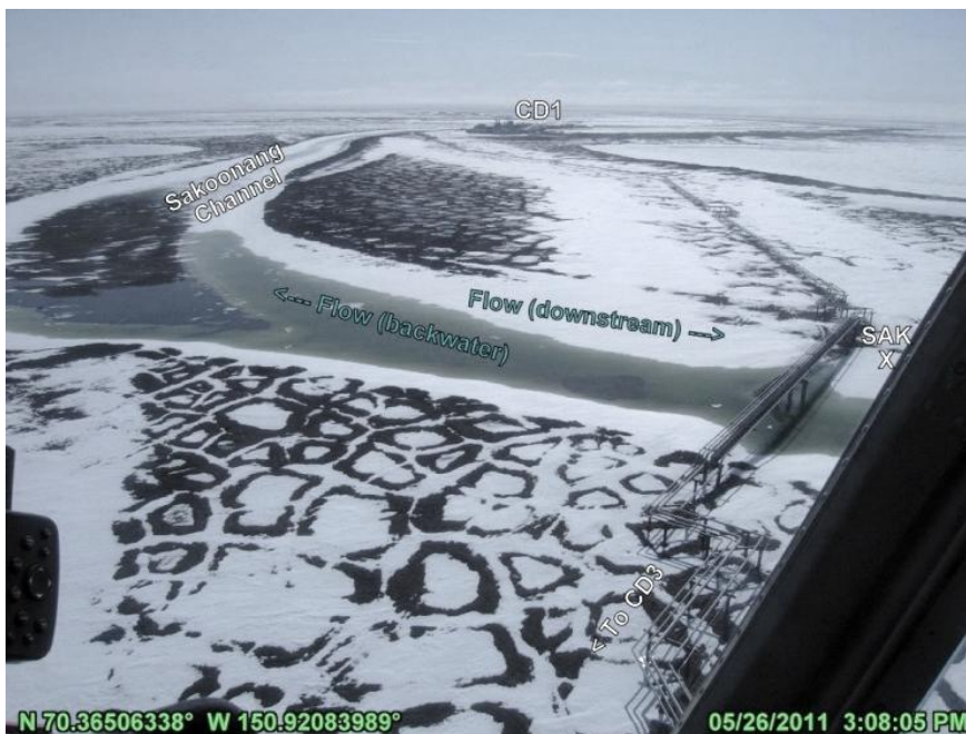
PHOTO 4.86: FLOW FROM THE TAMAYAYAK BACKING UPSTREAM IN THE SAKOONGANG PAST THE PIPELINE CROSSING, LOOKING UPSTREAM (SOUTH); MAY 26, 2011
