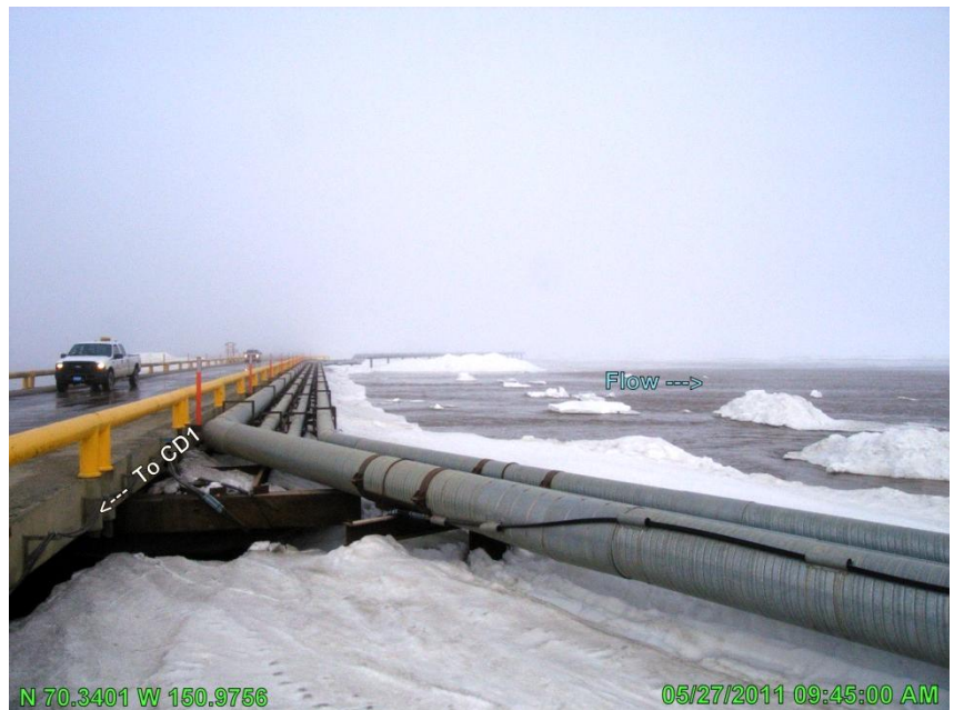
PHOTO 4.39: FLOW THROUGH THE 452-FOOT SWALE BRIDGE, SOME SNOW BLOCKAGE ON DOWNSTREAM (NORTH) SIDE, LOOKING WEST; MAY 27, 2011
