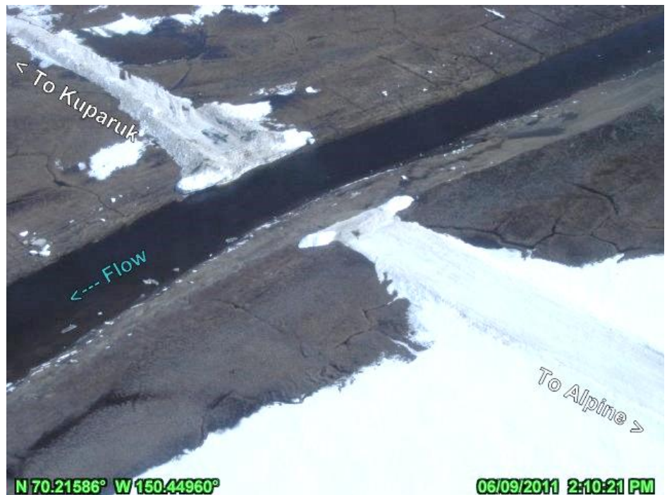
PHOTO 4.83: KACHEMACH RIVER ICE BRIDGE AS BREAKUP FLOWS RECEDE, LOOKING SOUTHEAST; JUNE 9, 2011
