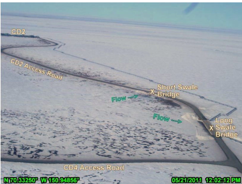
PHOTO 2.11: CD2 ROAD DRAINAGE STRUCTURES PRIOR TO BREAKUP, LOOKING WEST; MAY 21, 2011
