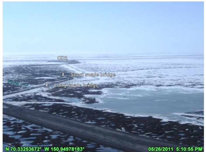
PHOTO 4.33: LOCAL MELT NEAR CD2 ROAD ACCESS STRUCTURES, LOOKING WEST; MAY 26, 2011
