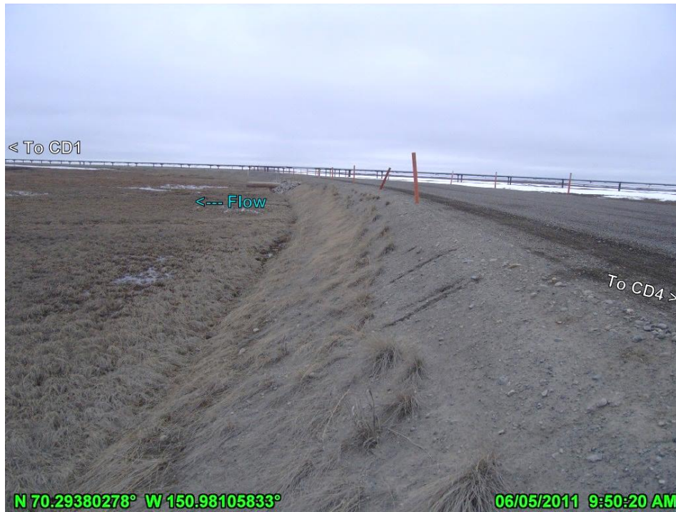
PHOTO 4.74: EROSION SURVEY CD4 ROAD PRISM POST-BREAKUP VICINITY OF CD4 PAD, LOOKING NORTH, JUNE 5, 2011
