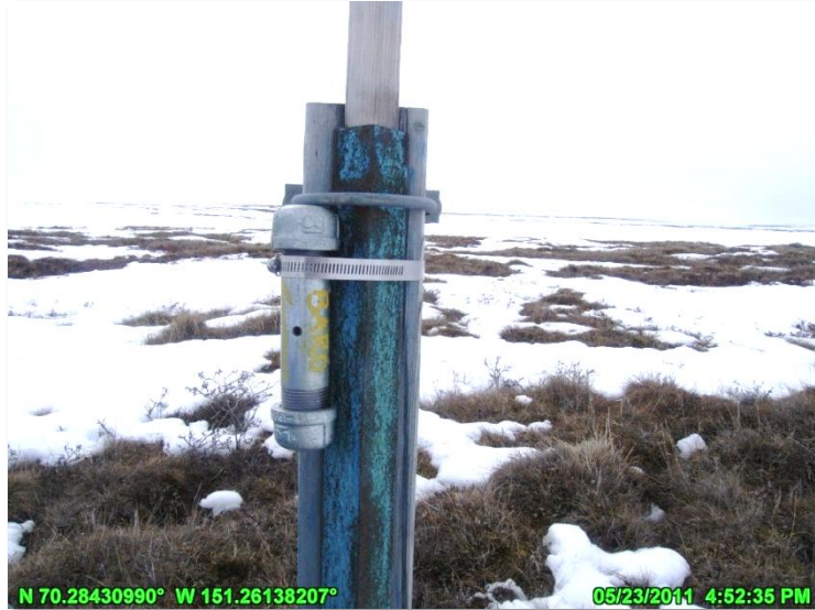
Photo 3.4: Barometric PT installed on UB6.8 Gage D, pre-breakup; May 23, 2011
