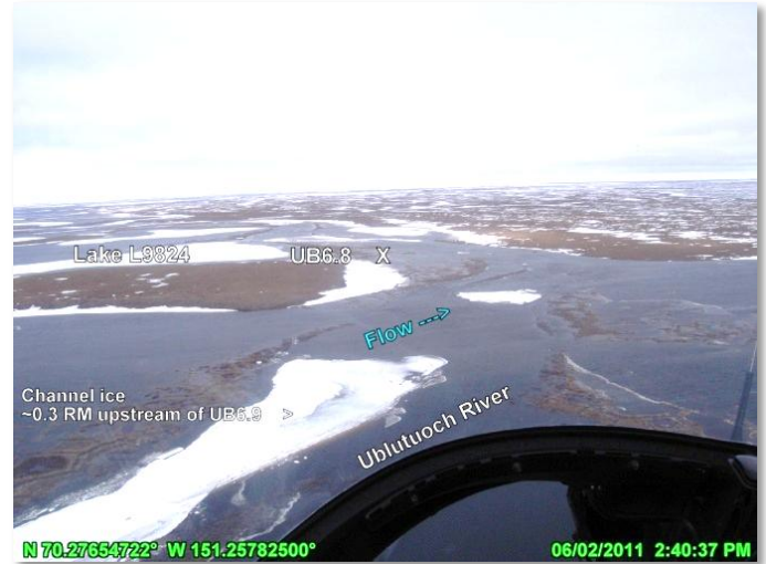
Photo 4.54: Peak stage in the Ublutuoch River at the proposed bridge crossing (UB6.8), upstream of UB6.9 looking downstream (northeast); June 2, 2011
