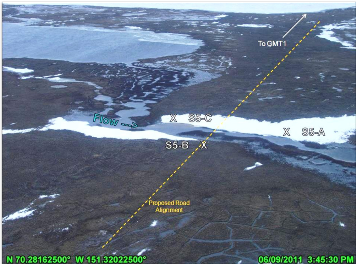
Photo 2.6: GMT 1 road crossing at S5, looking west; June 9, 2011
