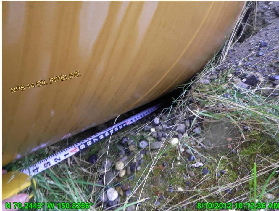
Photo A.11 Sloughing of the HDD East gravel pad, August 10, 2012
