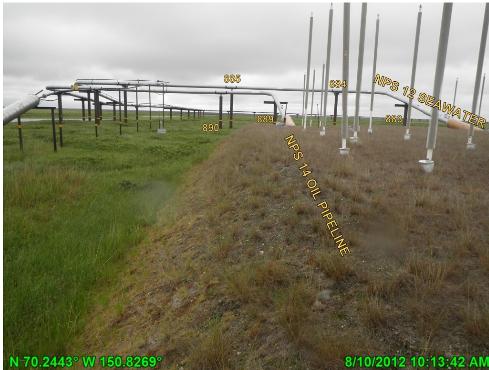
Photo A.12 North side of HDD East gravel pad, looking east, August 10, 2012
