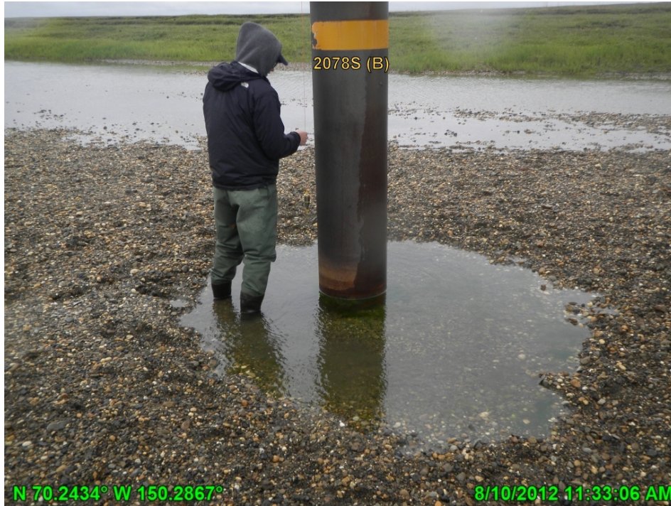
Photo A.25 Miluveach River VSM 2048S (B) scour, looking south, August 10, 2012
