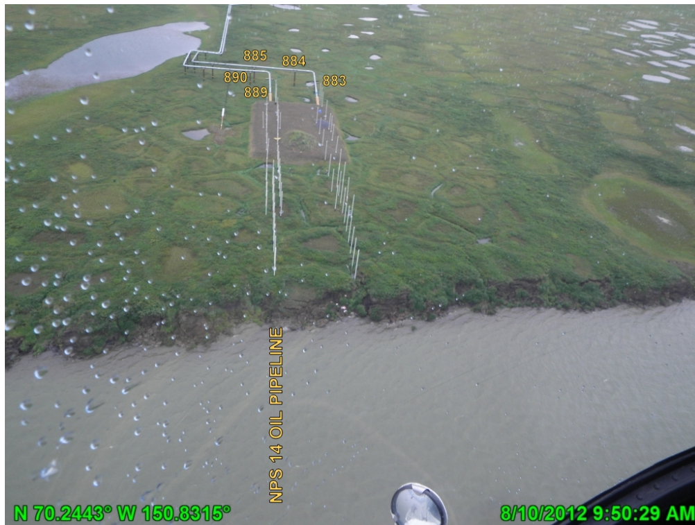
Photo A.10 HDD East bank, looking east, August 10, 2012
