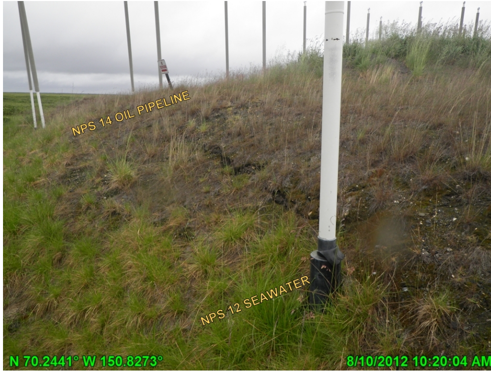
Photo A.15 Sloughing of the HDD East gravel pad west slope, August 10, 2012
