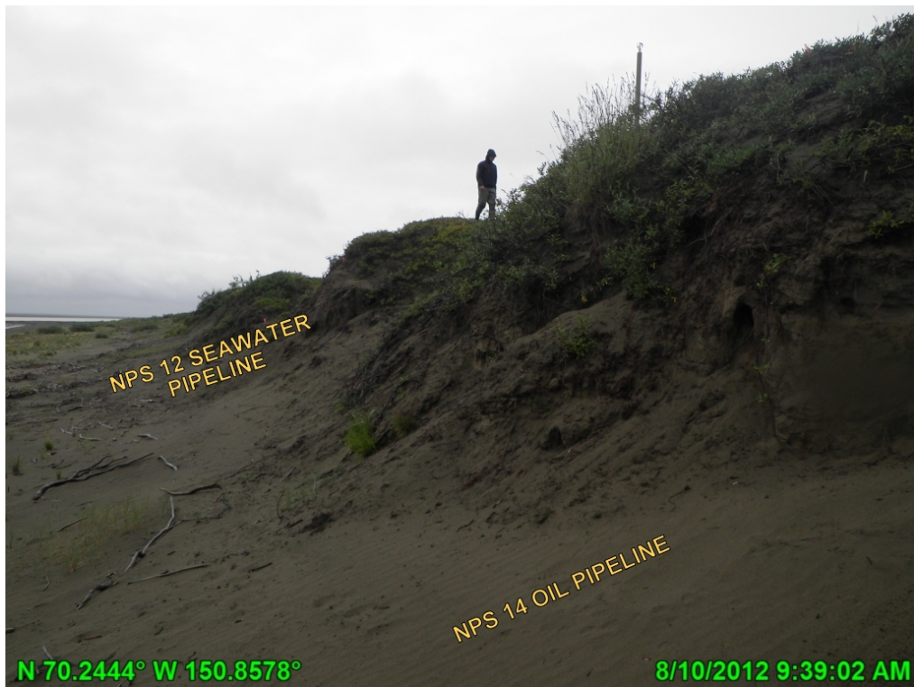
Photo A.6 HDD West bank, looking south, August 10, 2012
