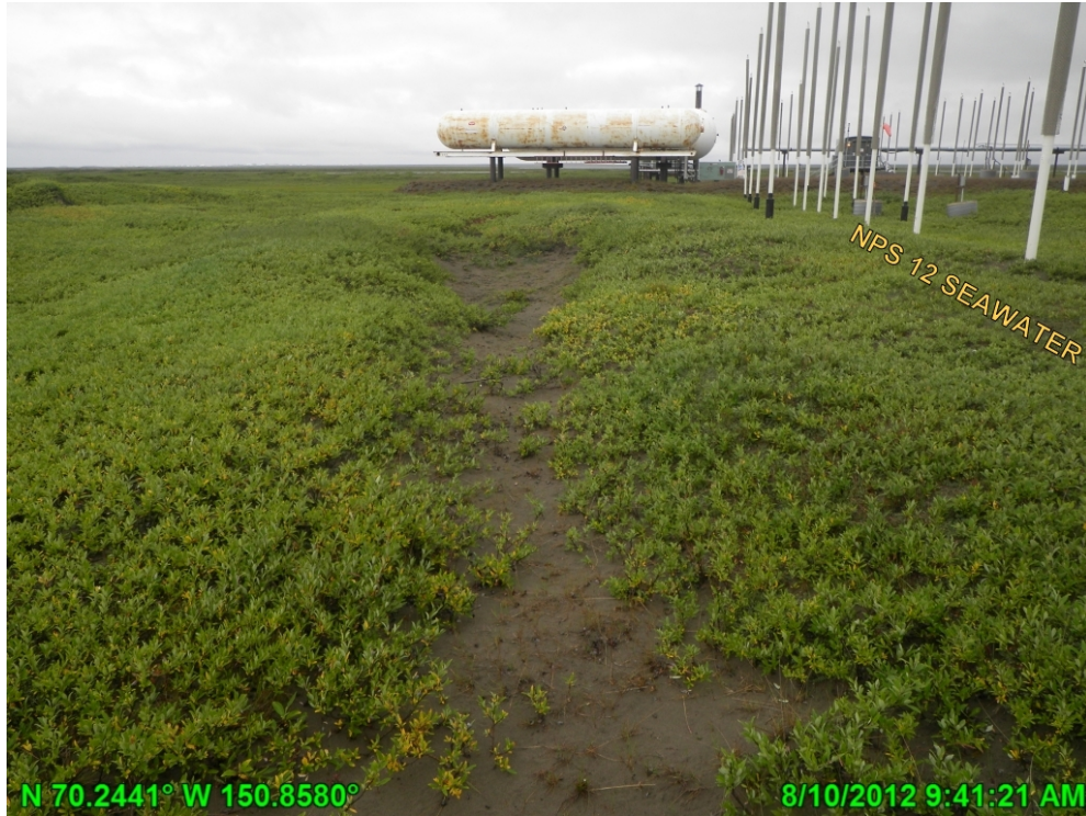
Photo A.7 HDD West depression off NPS 12 Seawater pipeline centerline, August 10, 2012
