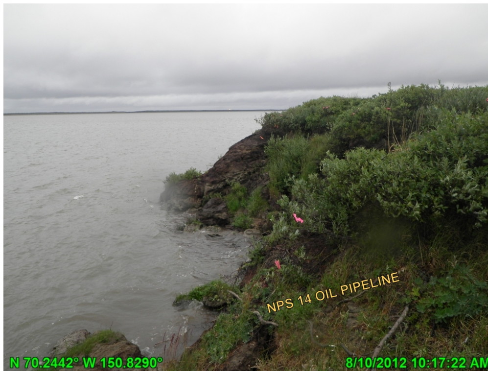
Photo A.14 HDD East bank looking north, August 10, 2012
