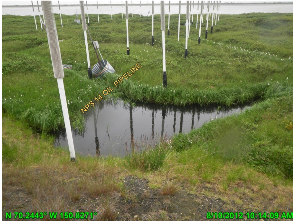
Photo A.13 Polygonal trough over NPS 14 Oil pipeline, August 10, 2012
