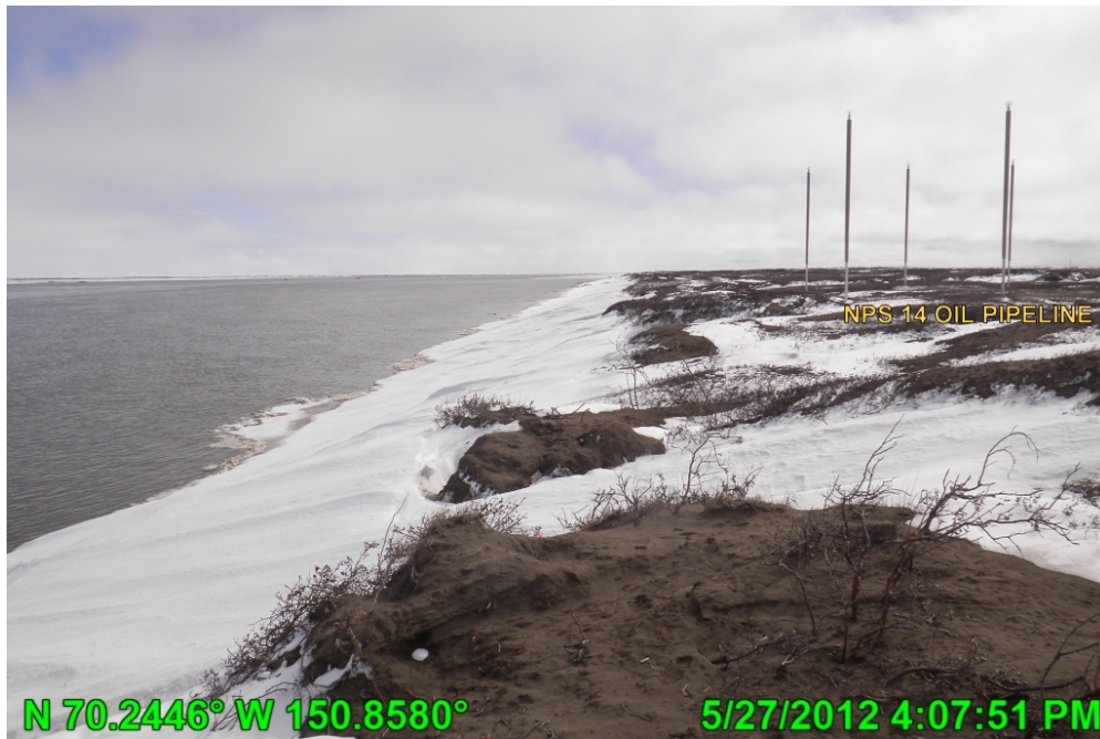
Photo A.1 HDD West bank during spring breakup, looking south, May 27, 2012
