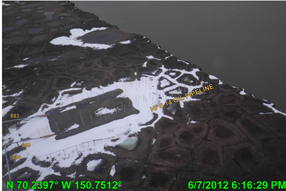
Photo A.9 HDD East during breakup, looking southwest, June 7, 2012
