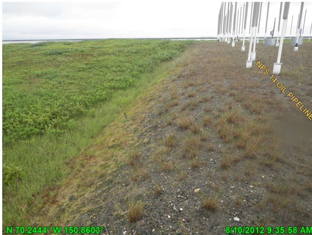
Photo A.4 HDD West north side of gravel pad, looking east, August 10, 2012
