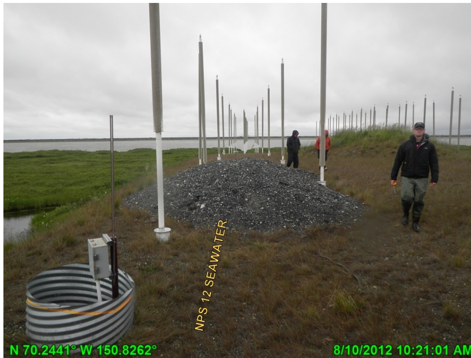
Photo A.16 HDD East, looking west through thermo-siphons, August 10, 2012
