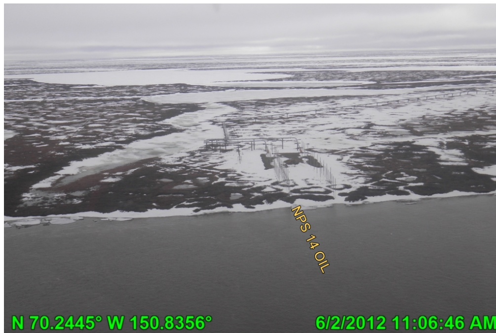
Photo A.8 HDD East bank during breakup, looking east, June 2, 2012
