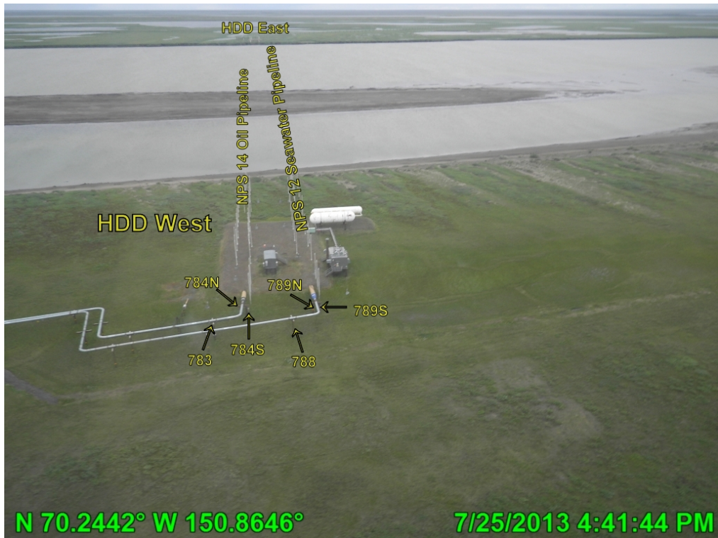
Photo A.7 HDD West post breakup, looking east; July 25, 2013
