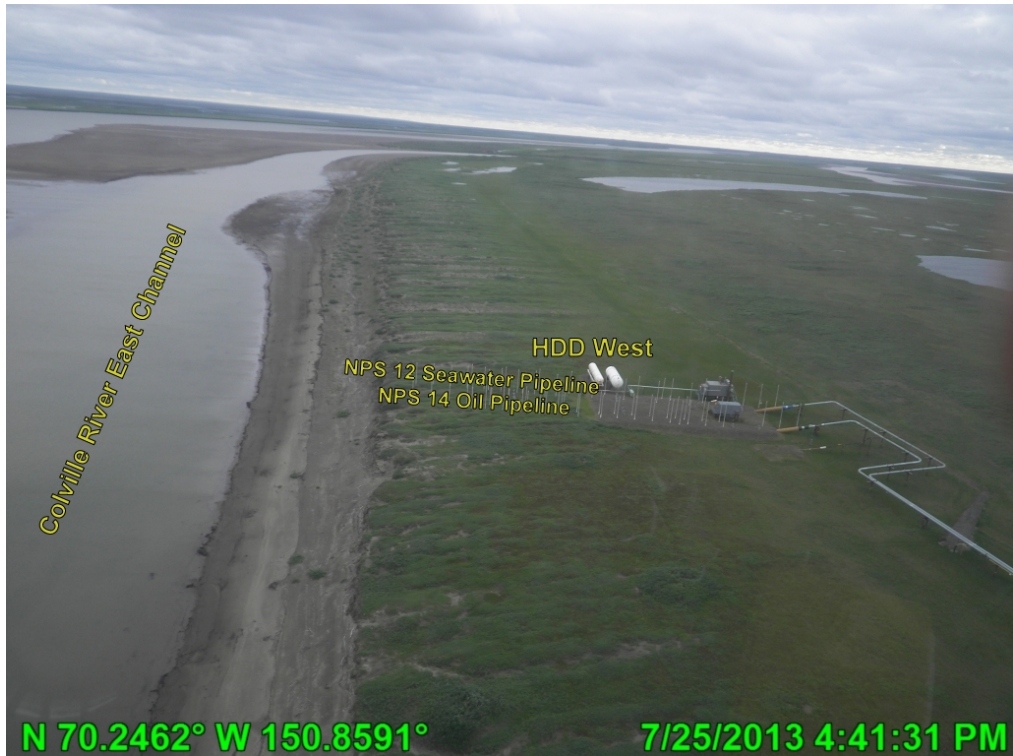
Photo A.6 HDD West post breakup, looking south; July 25, 2013
