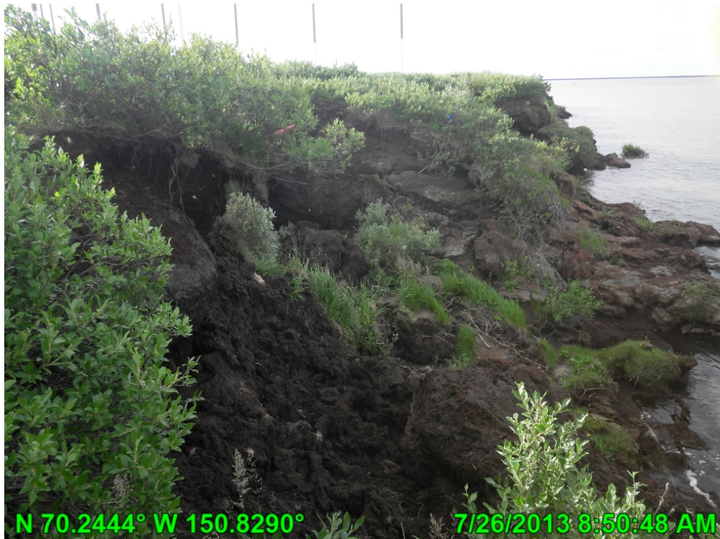
Photo A.19 HDD East bank, looking south; July 26, 2013
