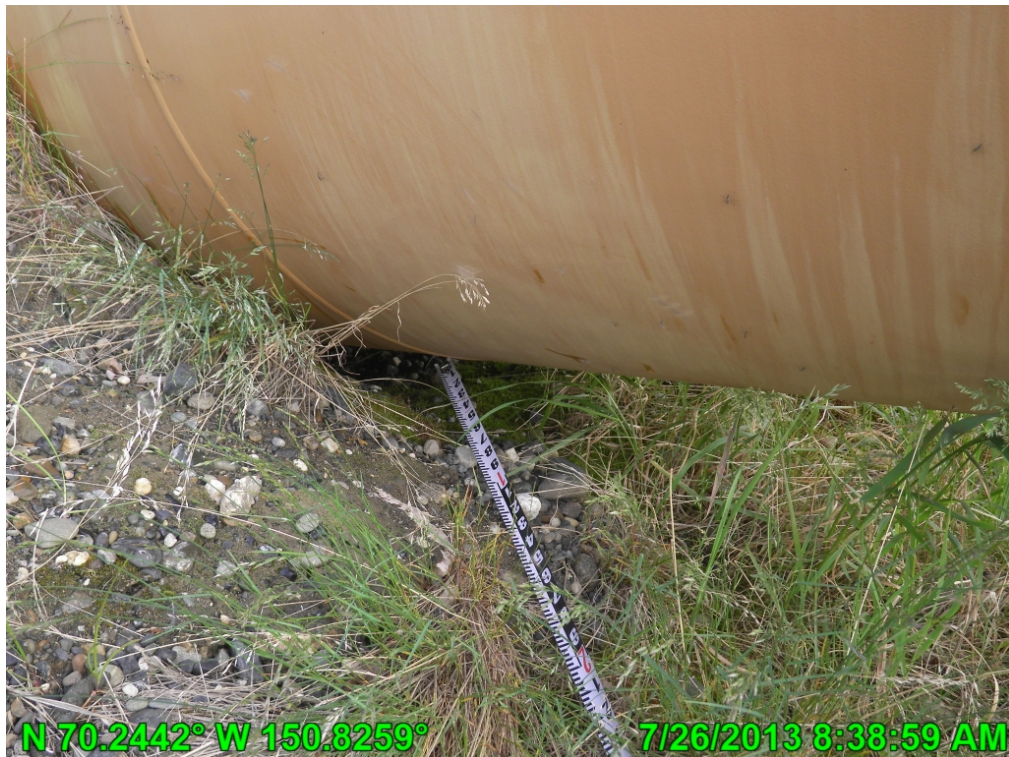
Photo A.24 HDD East sloughing of gravel pad; July 26, 2013
