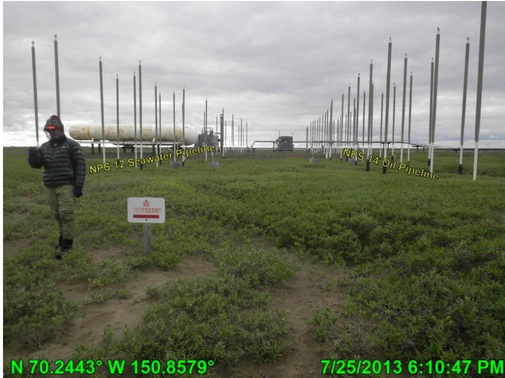
Photo A.13 HDD West, looking west through thermo-siphons; July 25, 2013
