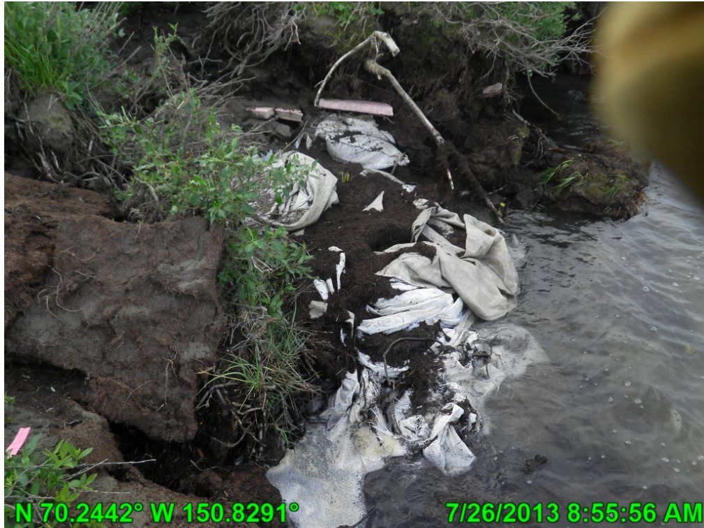
Photo A.23 HDD East exposed sandbags on bank; July 26, 2013
