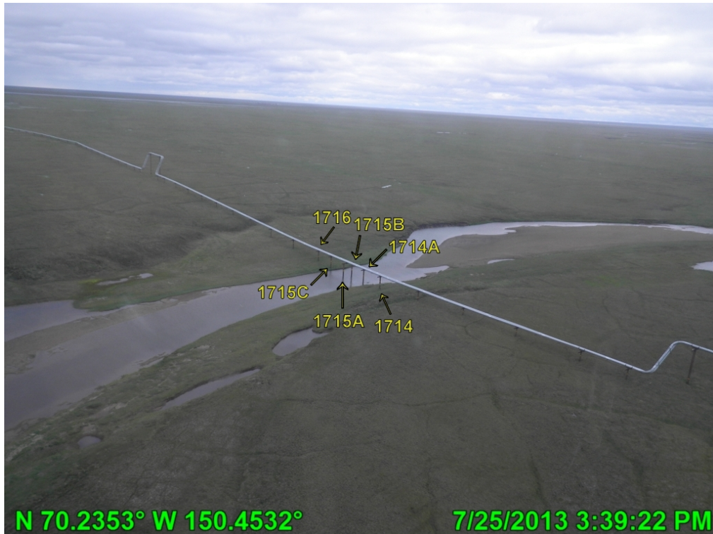
Photo A.28 Kachemach River post breakup, looking southwest; July 25, 2013
