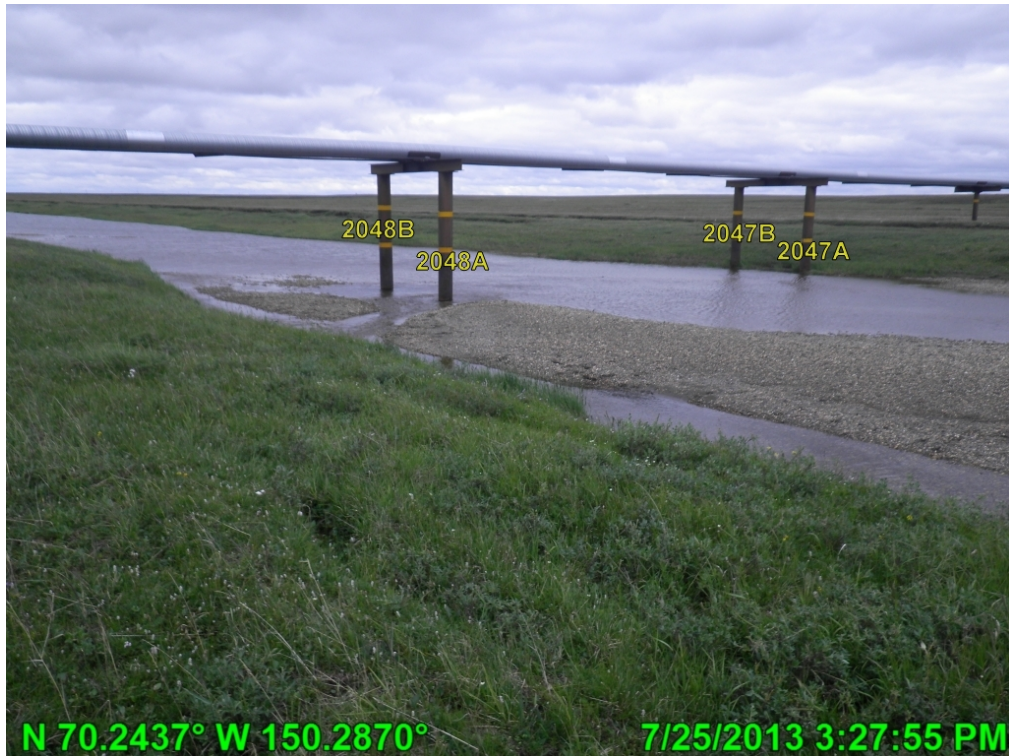
Photo A.38 Miluveach River post breakup, looking south; July 25, 2013
