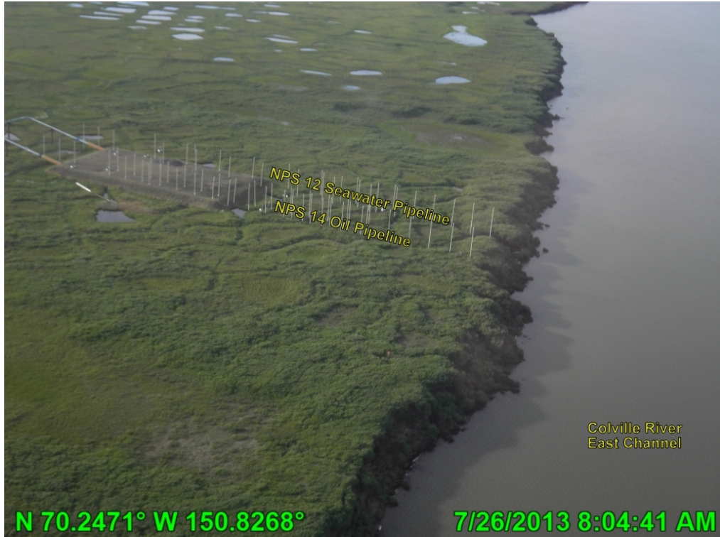
Photo A.17 HDD East post breakup, looking south; July 26, 2013
