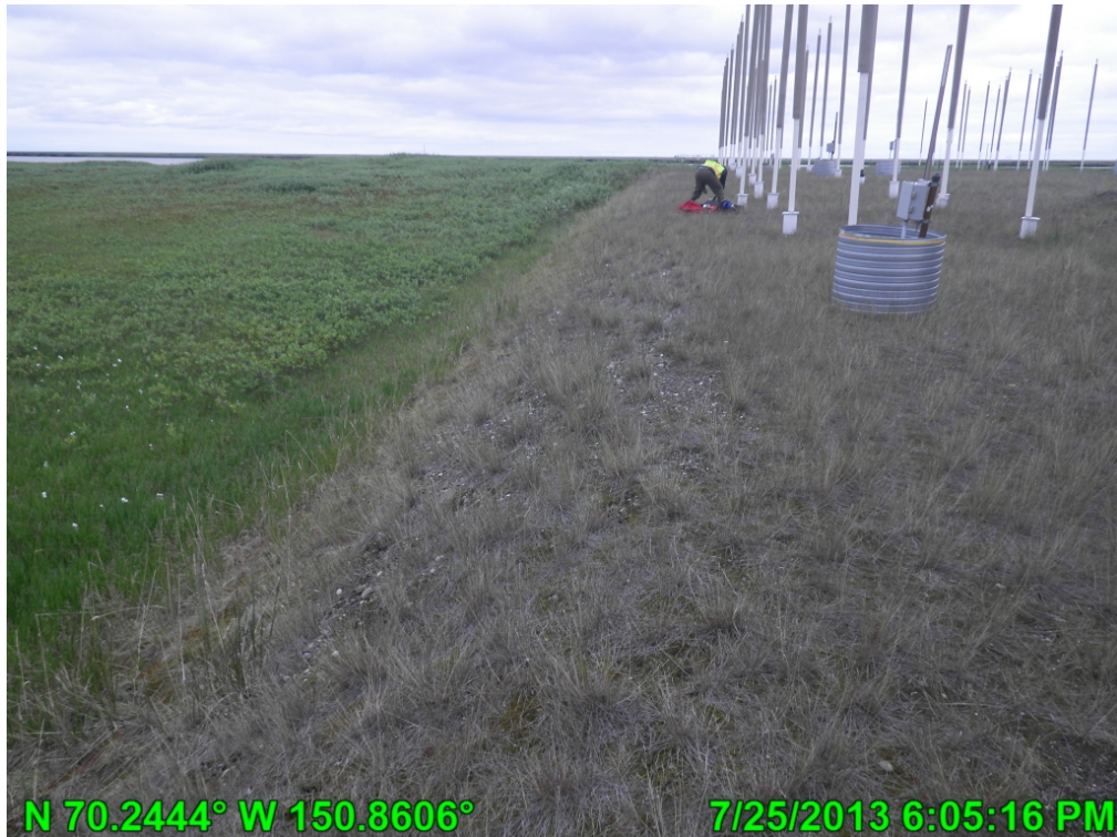
Photo A.10 HDD West north side gravel pad, looking east; July 25, 2013
