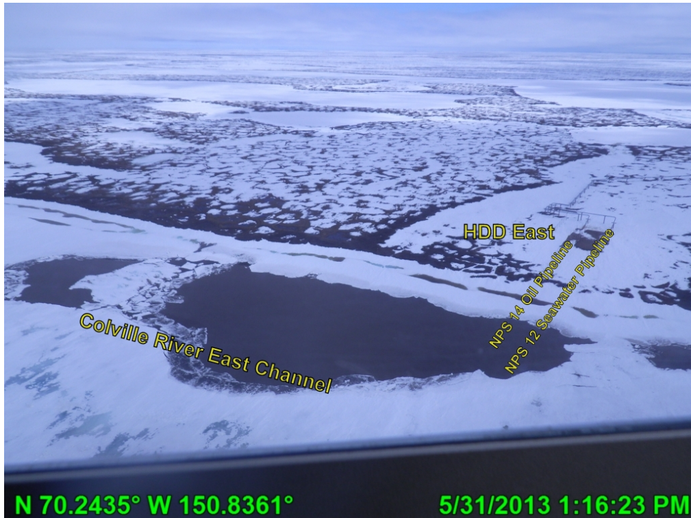
Photo A.14 HDD East pre breakup, looking northeast; May 31, 2013
