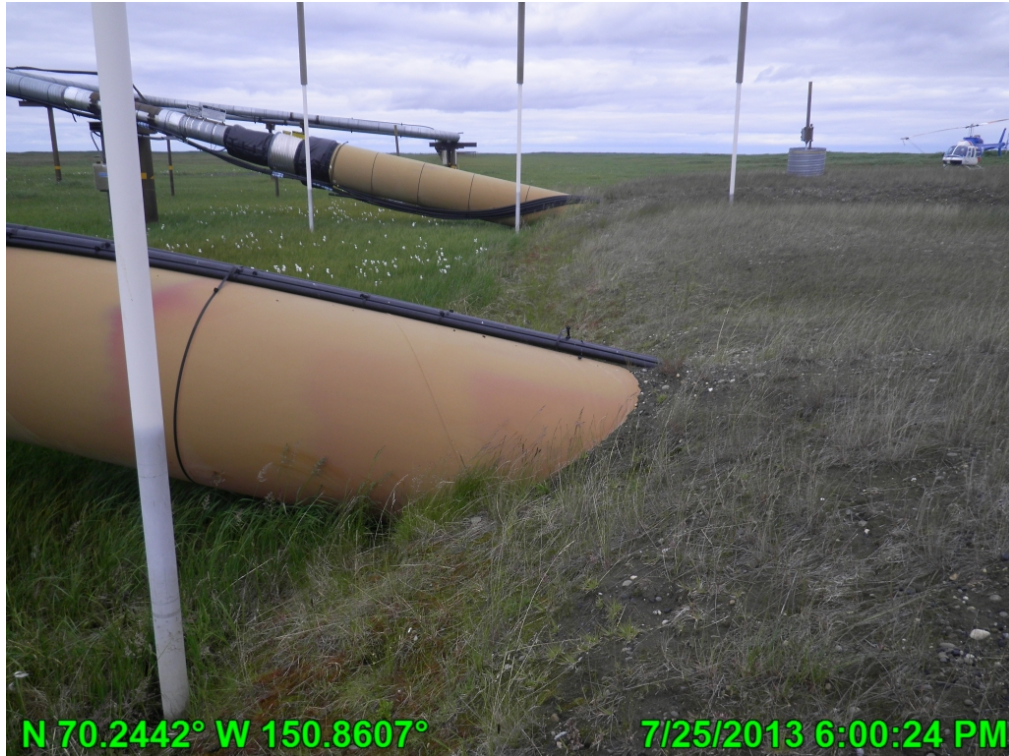
Photo A.11 HDD West pipeline entrance, looking northwest; July 25, 2013
