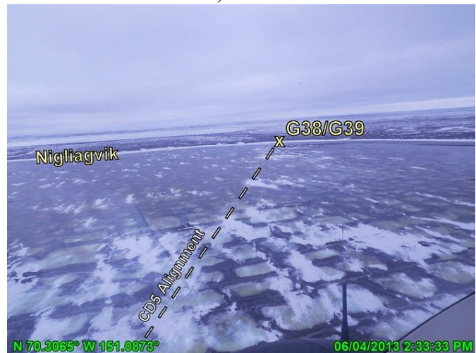
Photo 3.60: Extensive flooding along the proposed CD5 road alignment between the proposed Lake L9341 and Nigliagvik crossings, looking west; June 4, 2013
