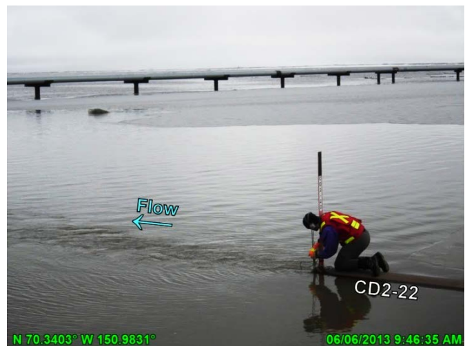
Photo 2.6: Measuring velocity at a culvert along the CD2 access road using a wading rod and Price AA velocity meter; June 6, 2013
