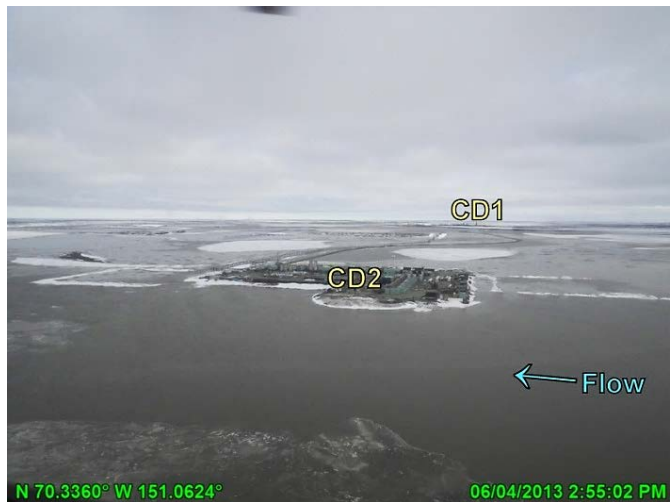
Photo 3.27: Floodwaters around CD2 road and pad near peak flood conditions, looking east; June 4, 2013
