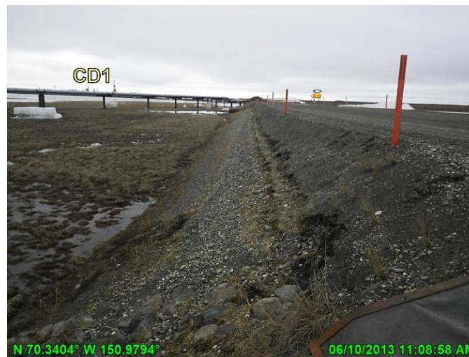
Photo 3.39: Winnowing of fine grained material on the south side of the CD2 road; June 10, 2013
