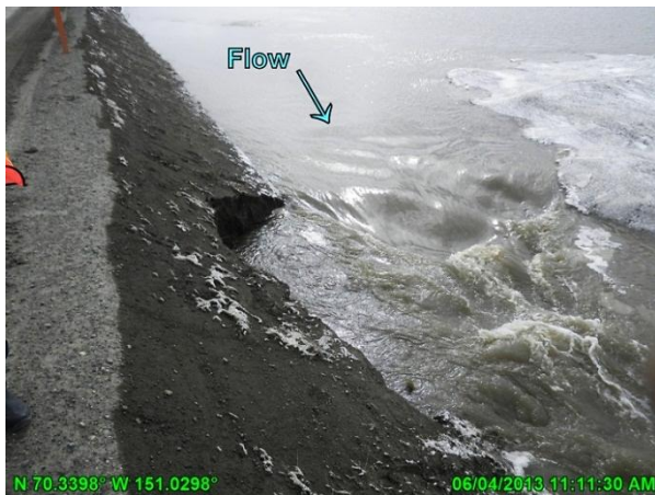
Photo 3.37: Localized erosion at the CD2 culvert battery, looking east; June 4, 2013
