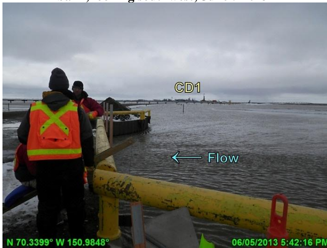
Photo 3.35: Conditions upstream of the short swale bridge while preparing for the direct discharge measurements, looking east; June 5, 2013
