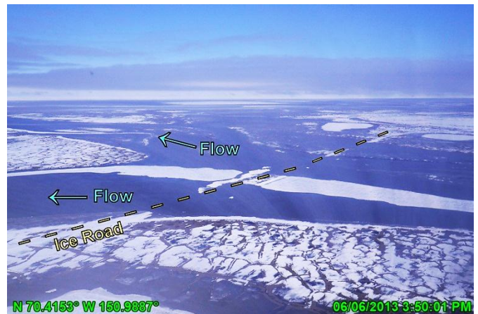
Photo 3.47: Tamayayak Channel ice bridge crossing, looking east; June 6, 2013
