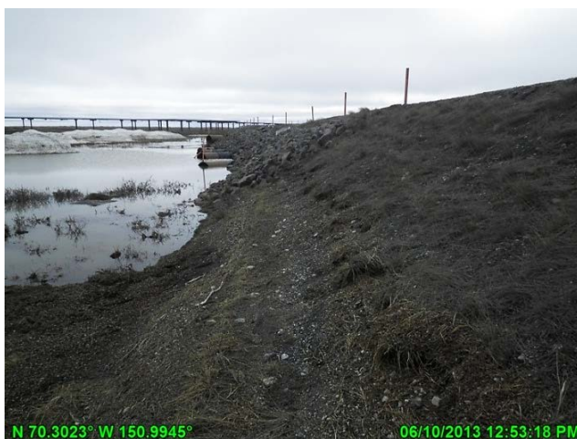
Photo 3.40: Representative conditions for CD4 culvert batteries, looking southeast; June 10, 2013
