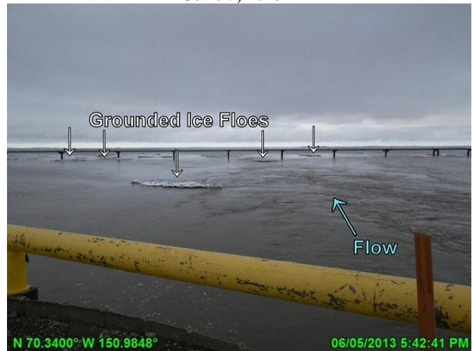
Photo 3.36: Grounded ice downstream of short swale bridge, looking north; June 5, 2013
