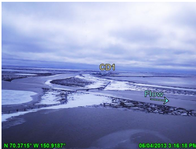
Photo 3.51: Overbank flooding at the Sakoonang Channel pipeline crossing, looking south; June 4, 2013
