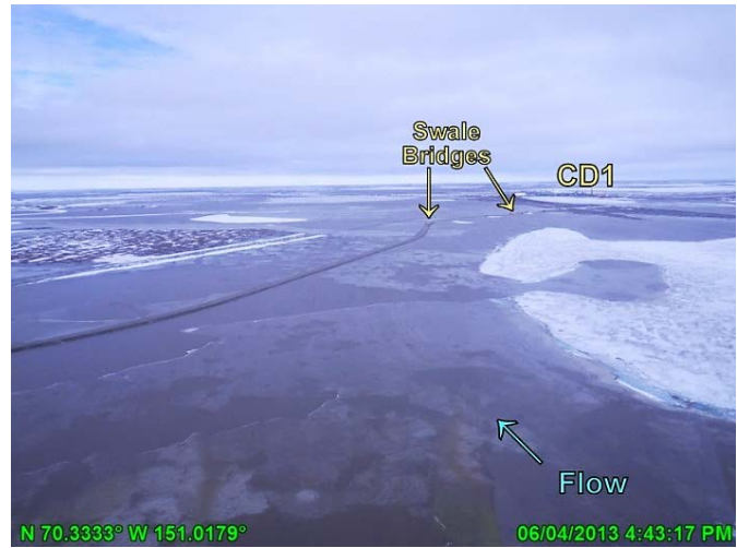
Photo 3.28: CD2 road during peak flood conditions, looking east; June 4, 2013
