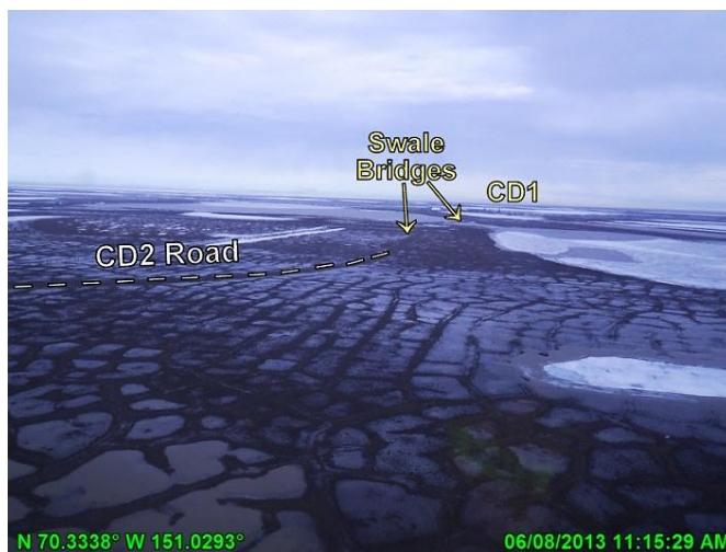
Photo 3.31: Recession of floodwater along the CD2 road, looking east; June 8, 2013
