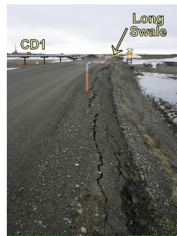
Photo 3.41: Tension cracks after flood water receded from the road prism near culvert CD2-23; June 10, 2013
