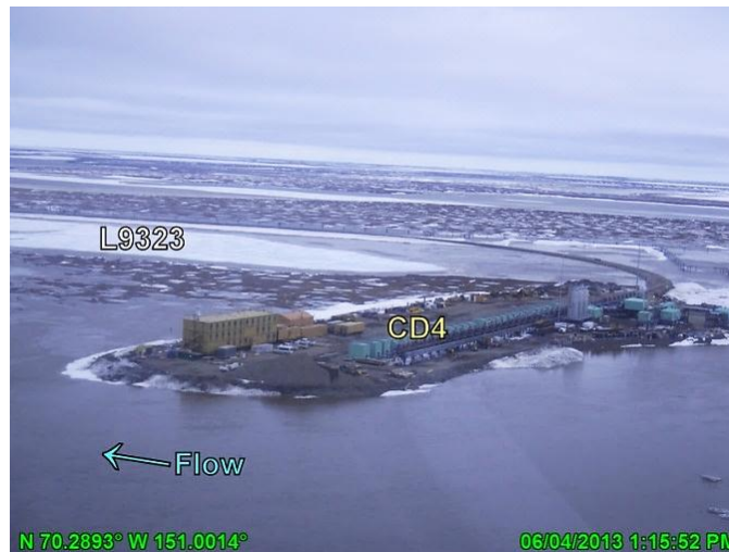
Photo 3.29: CD4 road and pad with accumulating backwater from the Nigliq Channel ice jam, looking east; June 4, 2013
