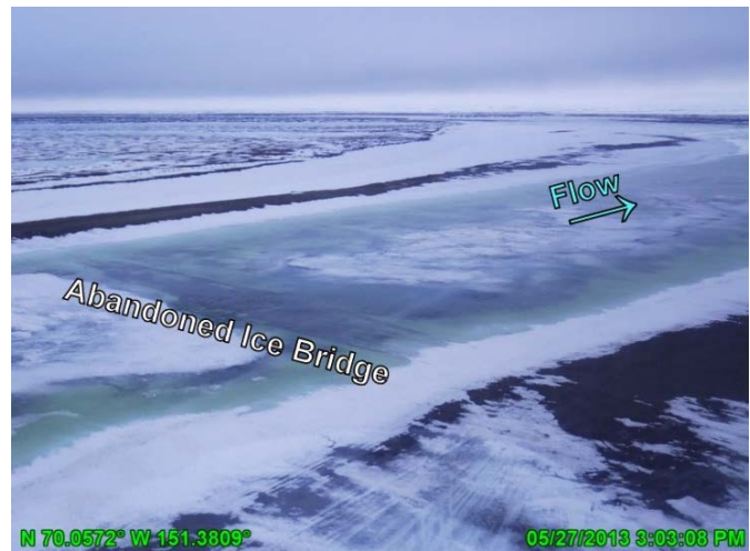
Photo 3.2: Melt water emerging from below the ice cover and flowing over remnants of an ice bridge near Ocean Point; May 27, 2013
