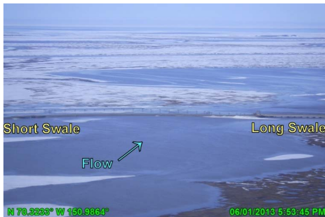
Photo 3.7: Floodwater passing through the CD2 swale bridges and adjacent culverts, looking southwest; June 1, 2013
