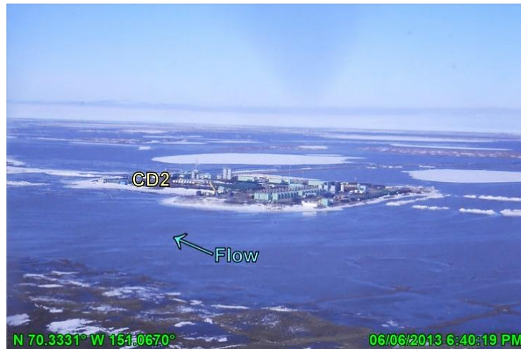
Photo 3.30: Nigliq Channel floodwaters remained high around the CD2 pad, looking northeast; June 6, 2013
