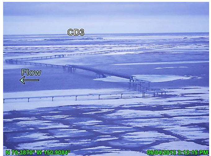
Photo 3.52: Overbank flooding at the Tamayayak Channel pipeline crossing, looking north; June 4, 2013
