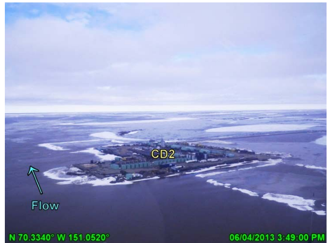
Photo 3.12: CD2 facility during peak; June 4, 2013
