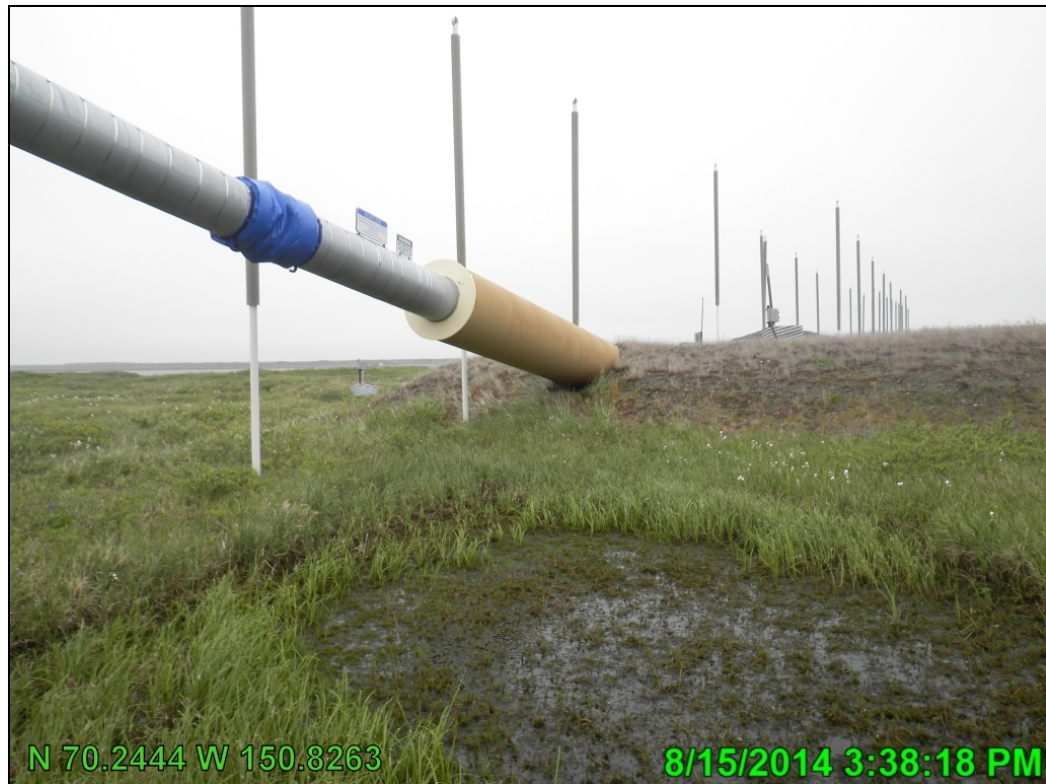
Photo A.25 HDD East pipeline entrance, looking southwest
