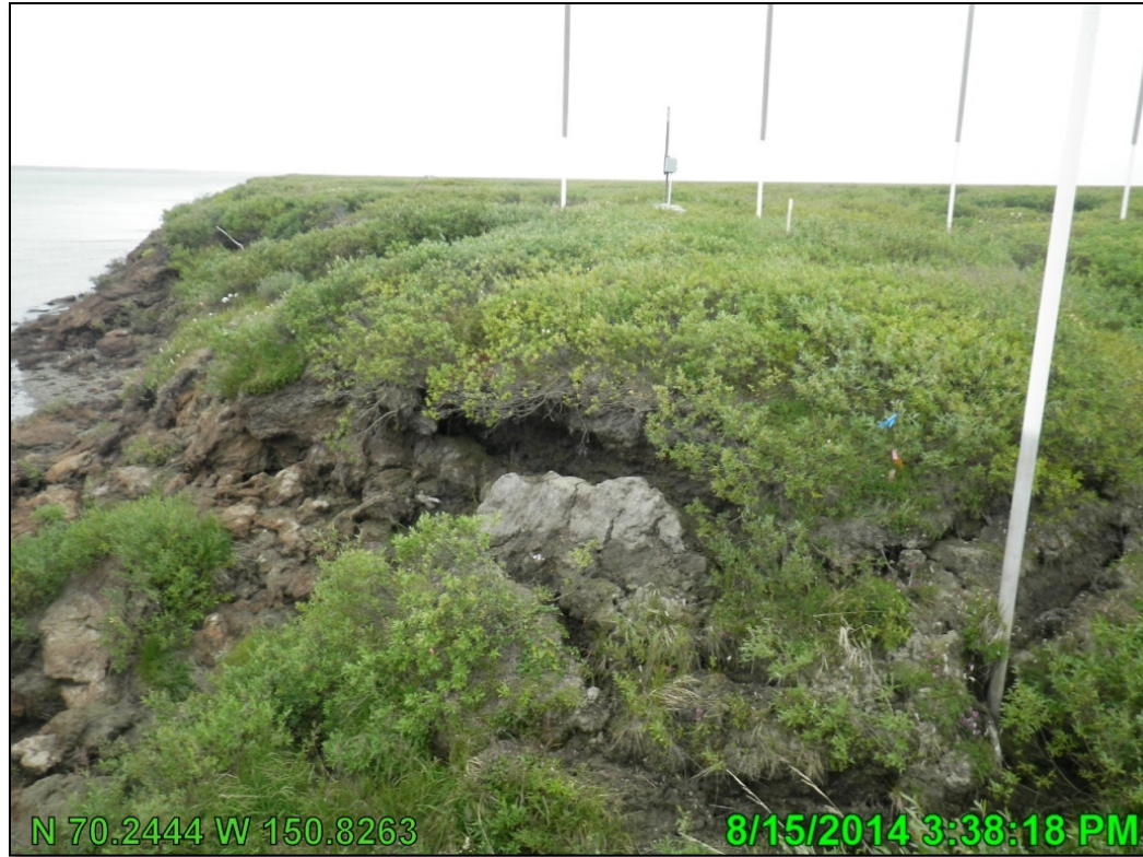
Photo A.18 HDD East bank, looking north; August 15, 2014
