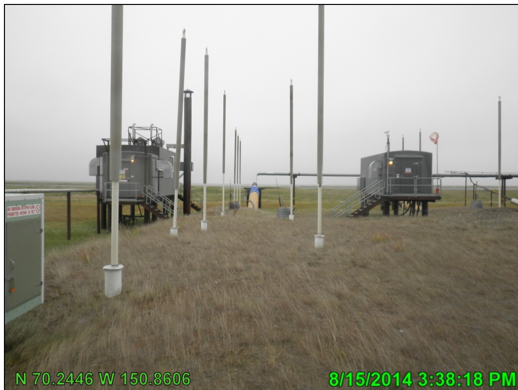
Photo A.12 HDD West south side of gravel pad, looking west; August 15, 2014
