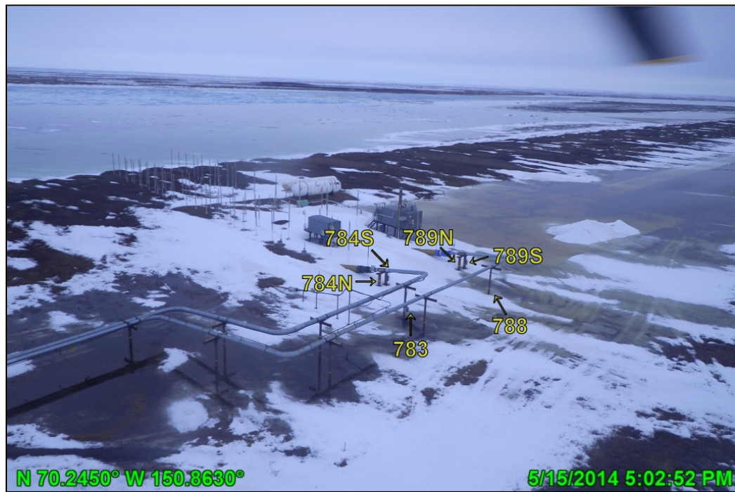
Photo A.2 HDD West during breakup, looking southeast; May 15, 2014
