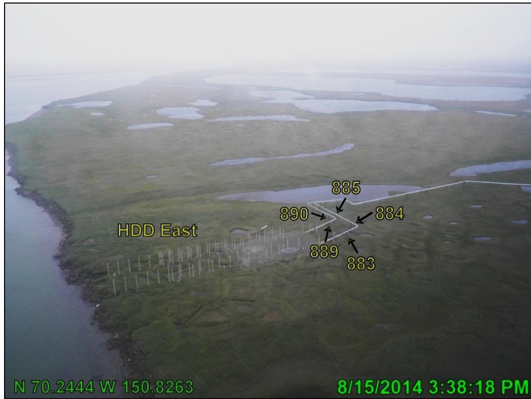
Photo A.17 HDD East post breakup, looking northeast; August 15, 2014
