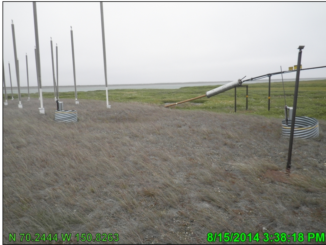
Photo A.22 HDD East depression over the NPS Oil Pipeline, looking northwest; August 15, 2014
