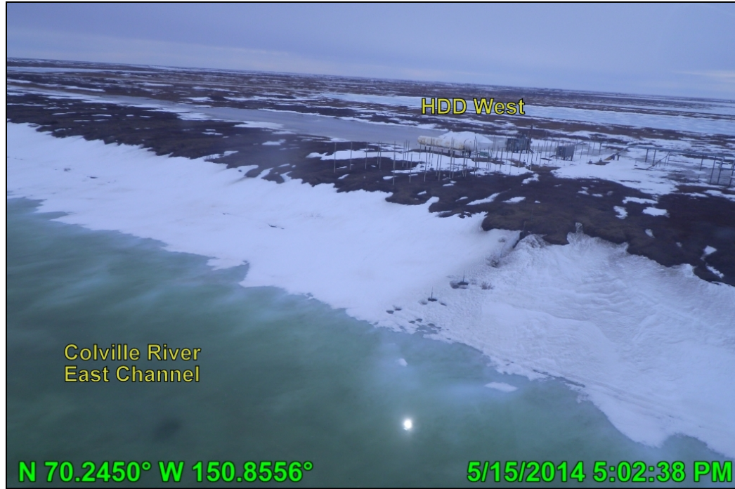
Photo A.3 HDD West during breakup, looking southwest; May 15, 2014
