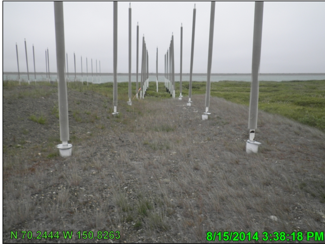
Photo A.26 HDD East looking west through thermo-siphons; August 15, 2014
