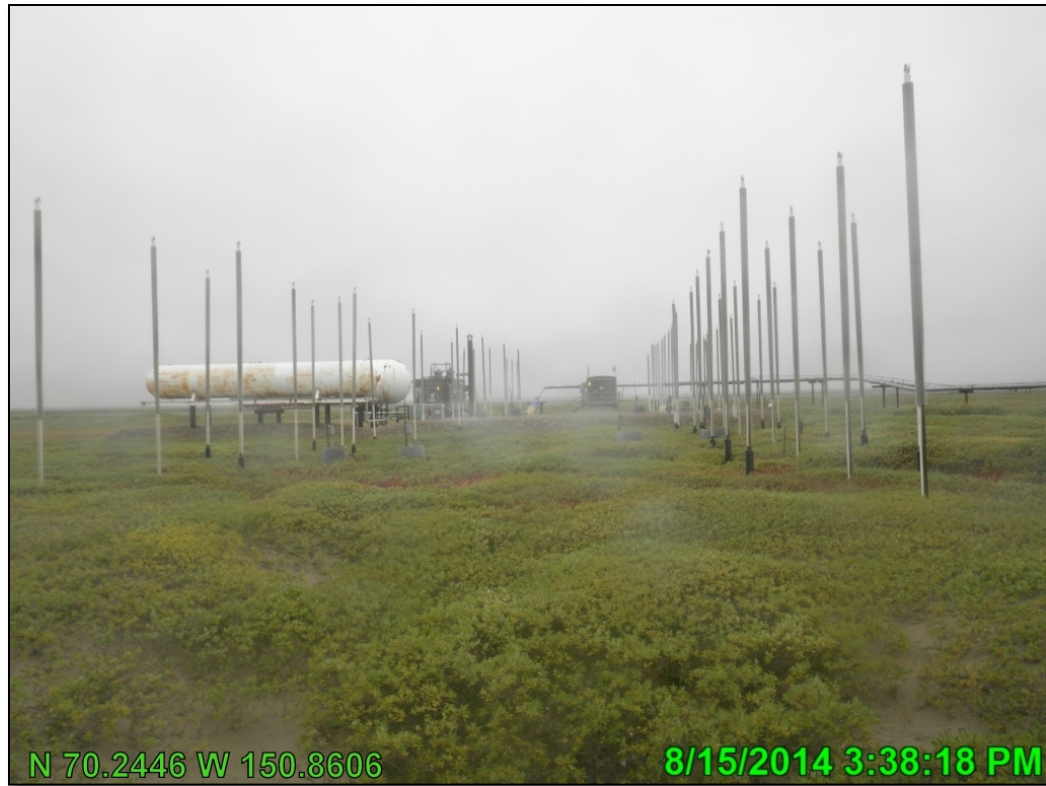
Photo A.13 HDD West looking west through thermo-siphons; August 15, 2014
