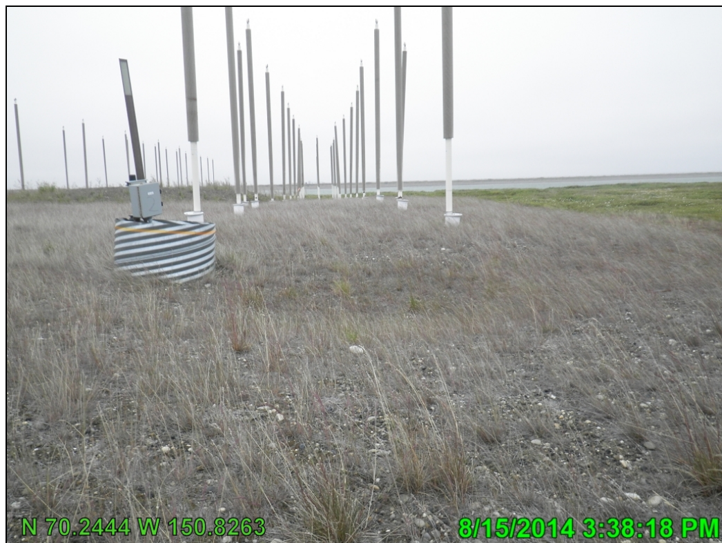
Photo A.23 HDD East depression over the NPS Oil Pipeline, looking west; August 15, 2014
