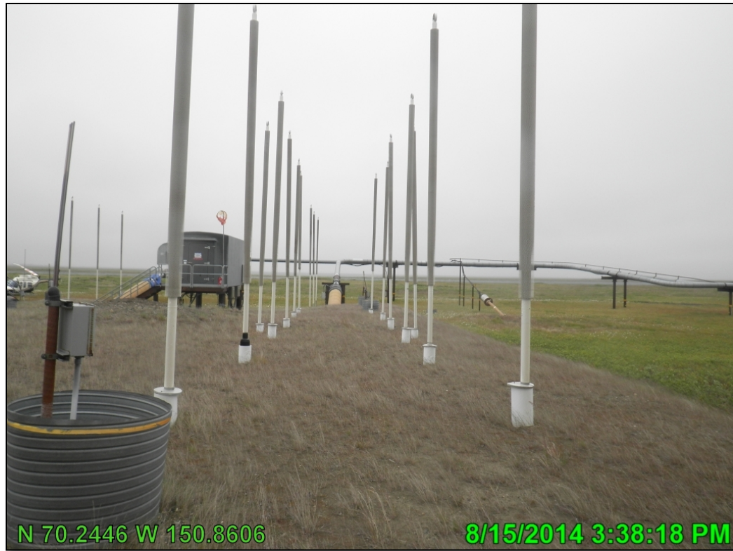
Photo A.11 HDD West north side of gravel pad, looking west; August 15, 2014
