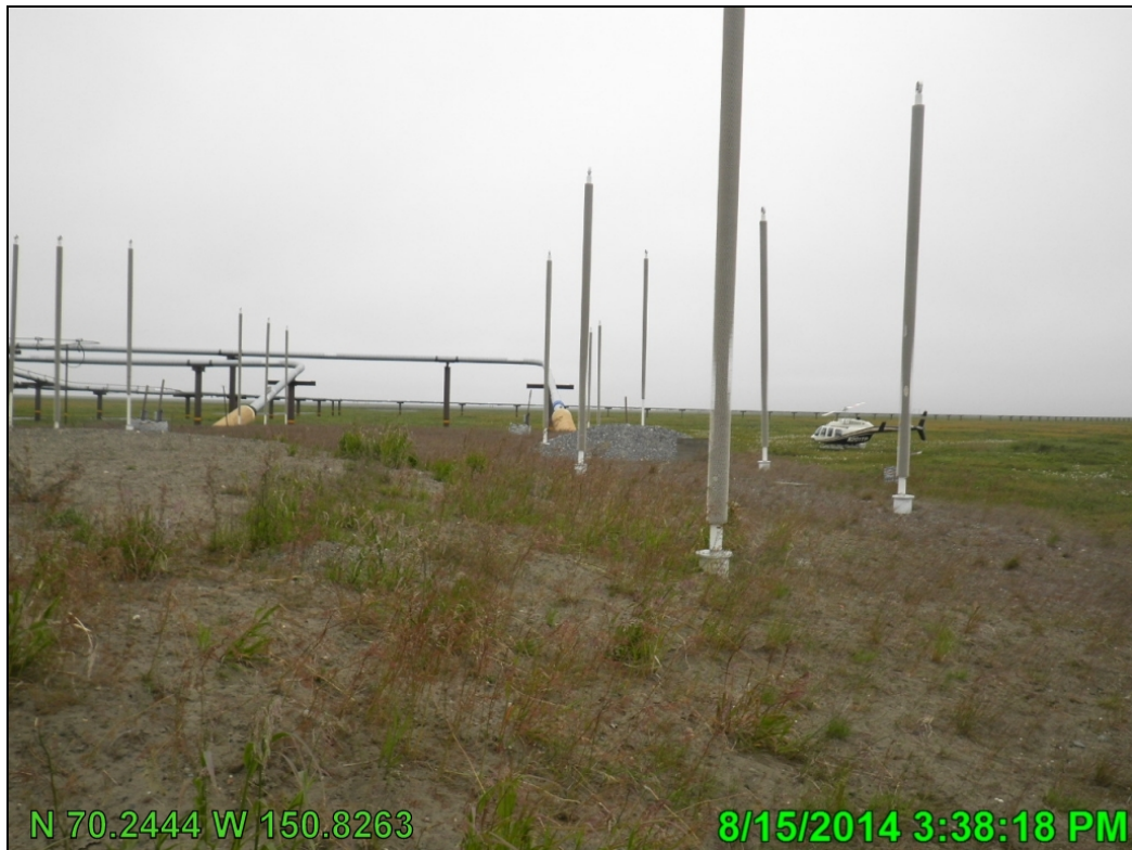
Photo A.21 HDD East south side of gravel pad, looking east; August 15, 2014
