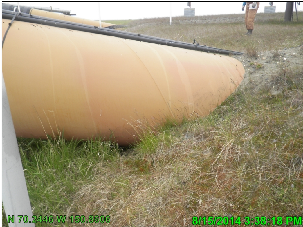
Photo A.10 HDD West pipeline entrance, looking south; August 15, 2014
