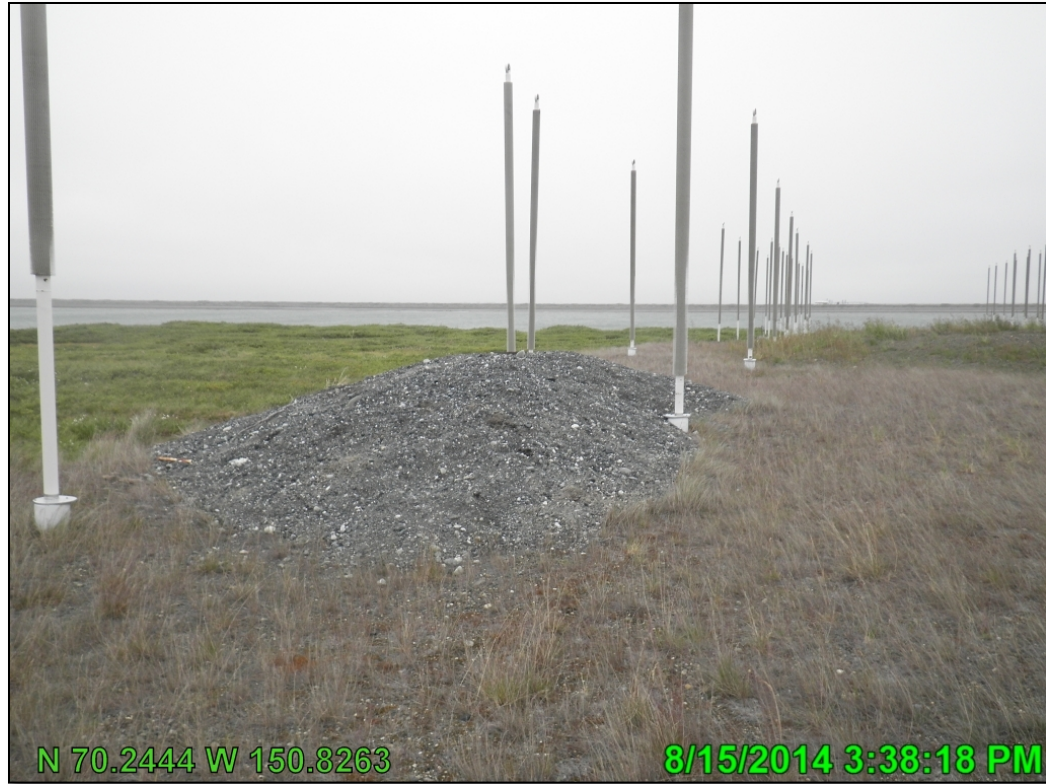
Photo A.24 HDD East fill over Seawater Pipeline, looking southwest; August 15, 2014
