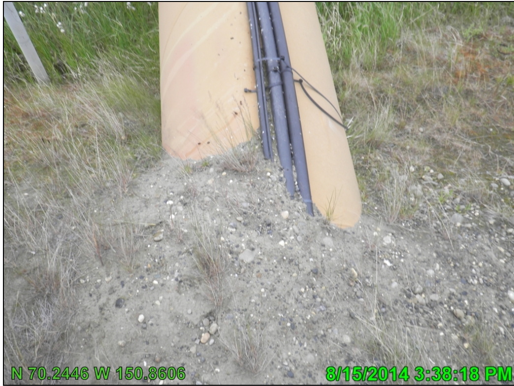
Photo A.9 HDD West pipeline entrance, looking east; August 15, 2014
