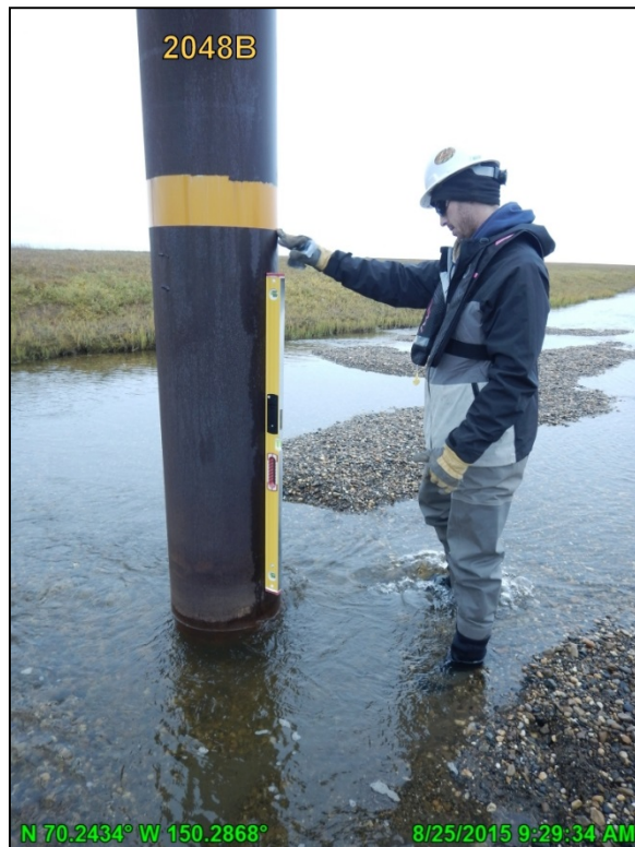
Photo A.50: Miluveach River VSM measurement with level, looking southeast; August 25, 2015
