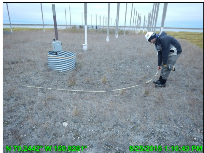
Photo A.27: HDD East depression over the NPS oil pipeline, looking west; August 25, 2015
