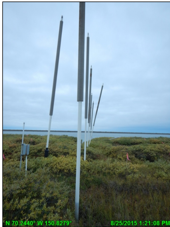
Photo A.32: HDD East looking west through thermosyphons; August 25, 2015
