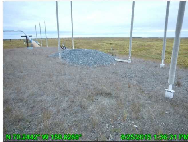
Photo A.28: HDD East fill over seawater pipeline, looking southeast; August 25, 2015
