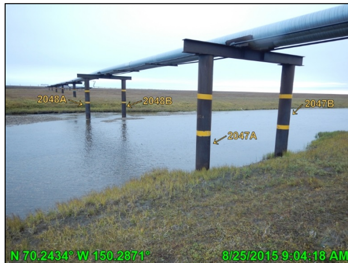
Photo A.48: Miluveach River VSMs, looking southeast; August 25, 2015
