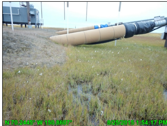
Photo A.9: HDD West pipeline entrance, looking south; August 25, 2015
