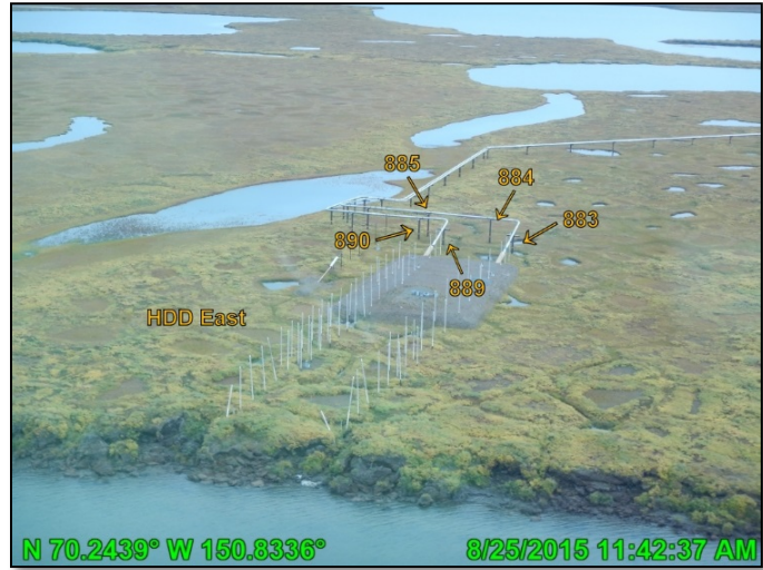
Photo A.22: HDD East post breakup, looking northeast; August 25, 2015
