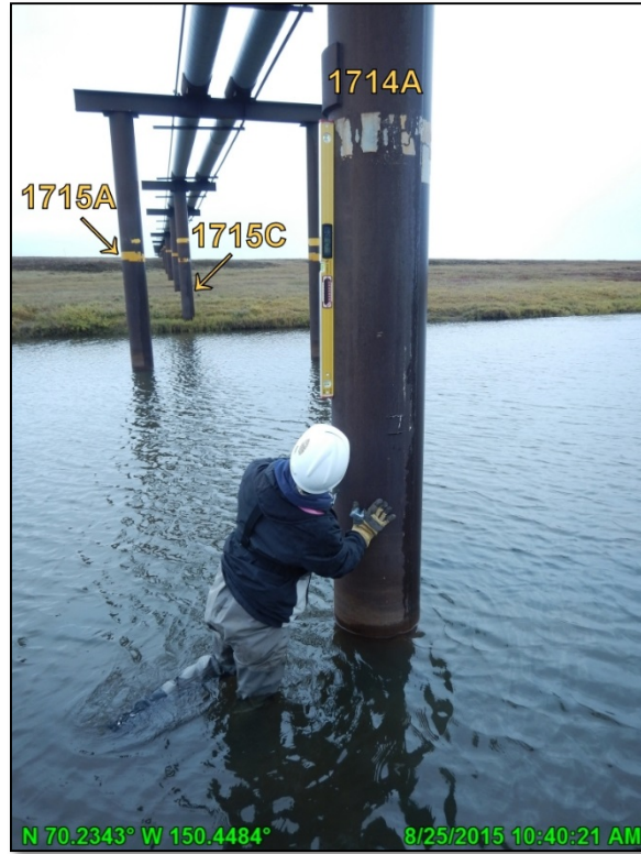
Photo A.41: Kachemach River VSM measurement with level, looking east; August 25, 2015
