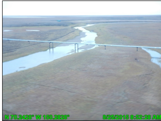
Photo A.46: Miluveach River post breakup, looking northwest; August 25, 2015
