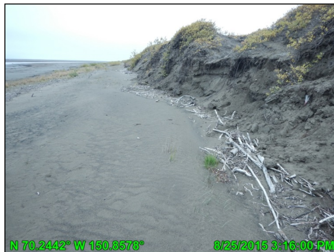
Photo A.12: HDD West bank post breakup, looking south (upstream); August 25, 2015
