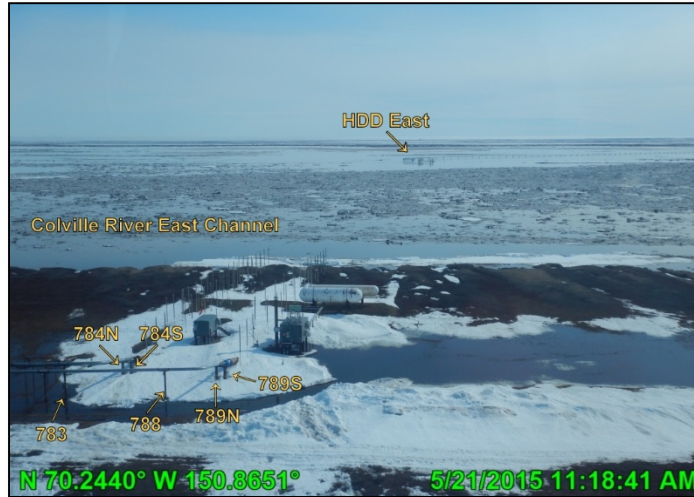
Photo A.7: HDD West during breakup, looking east; May 21, 2015
