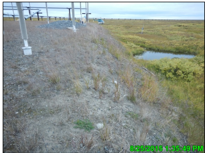
Photo A.26: HDD East south side of gravel pad, looking east; August 25, 2015
