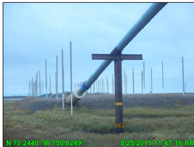
Photo A.29: HDD East pipeline entrance, looking northwest; August 25, 2015
