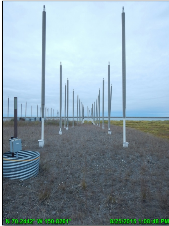
Photo A.31: HDD East looking west through thermosyphons; August 25, 2015
