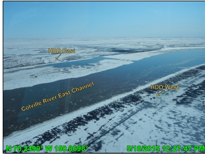
Photo A.4: HDD West during breakup, looking southeast; May 18, 2015
