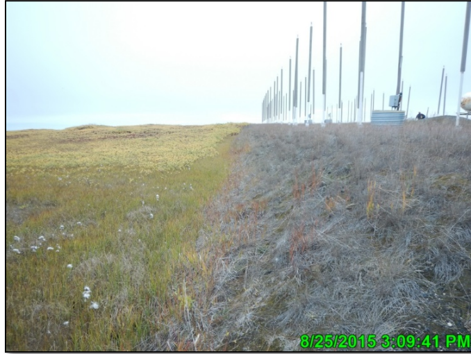
Photo A.13: HDD West north side of gravel pad, looking east; August 25, 2015
