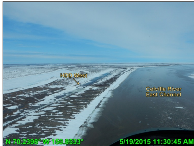
Photo A.6: HDD West during breakup, looking north; May 19, 2015
