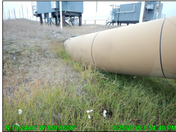
Photo A.10: HDD West pipeline entrance, looking southeast; August 25, 2015
