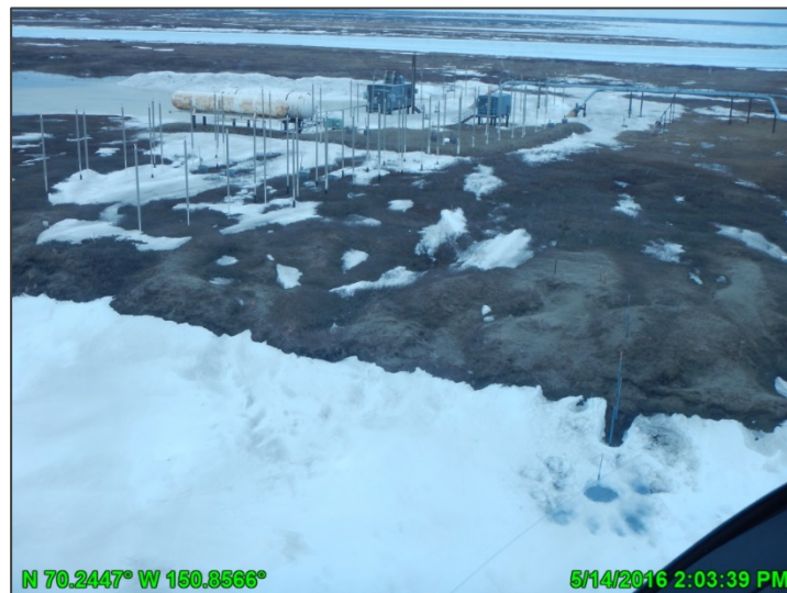
Photo A-3: HDD West pre-breakup, looking southwest; May 14, 2016
