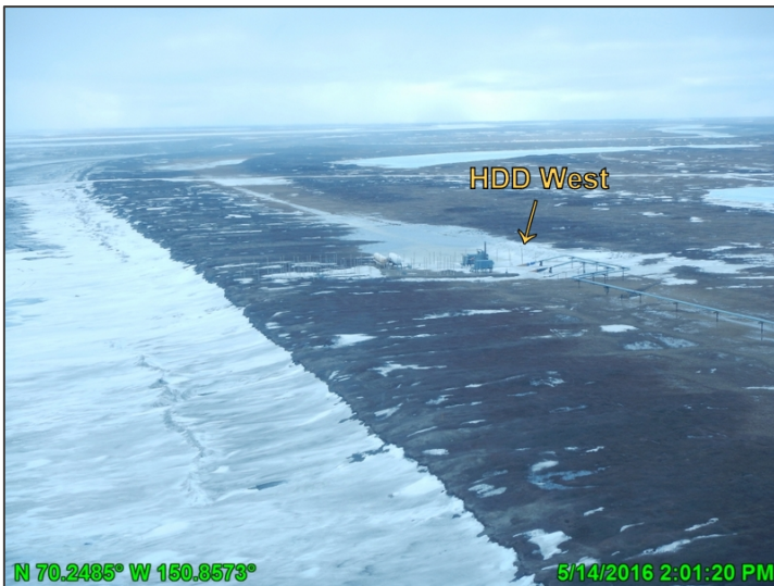
Photo A-1: HDD West pre-breakup, looking southwest; May 14, 2016
