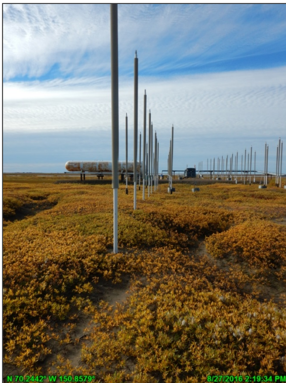
Photo A-13: HDD West south side thermosyphons, looking west; August 27, 2016
