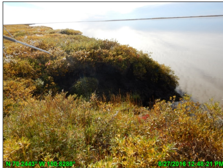
Photo A-21: HDD East bank post breakup, looking south; August 27, 2016
