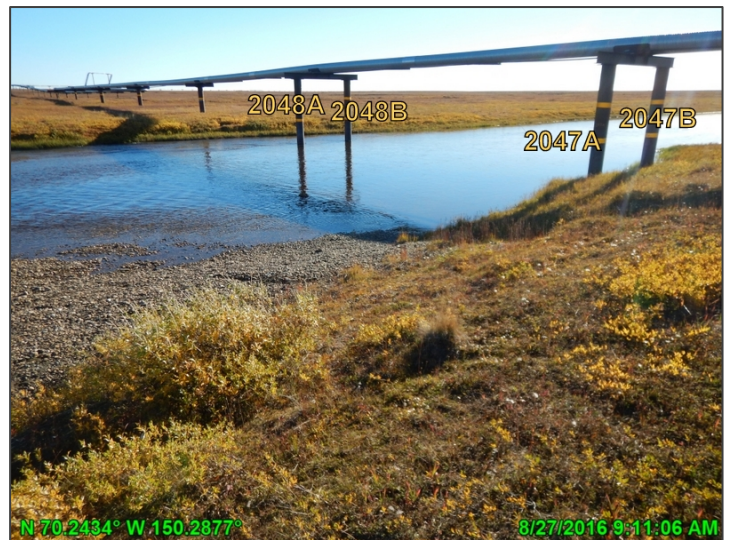
Photo A-51: Miluveach River post breakup, looking southeast; August 27, 2016
