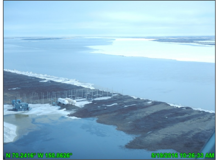
Photo A-5: HDD West during breakup, looking northeast; May 19, 2016
