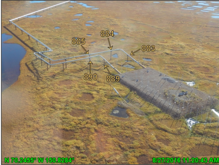
Photo A-19: HDD East post breakup, looking southeast; August 27, 2016
