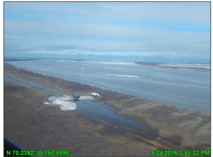
Photo A-7: HDD West during breakup, looking northeast; May 24, 2016
