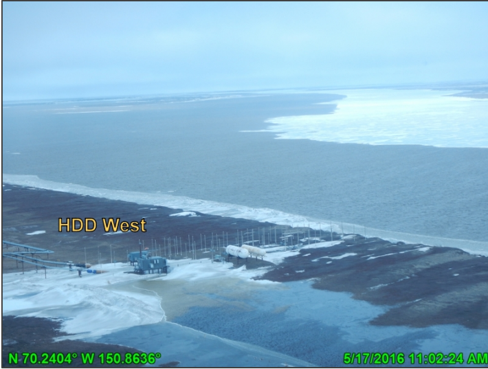
Photo A-4: HDD West during breakup, looking northeast; May 17, 2016
