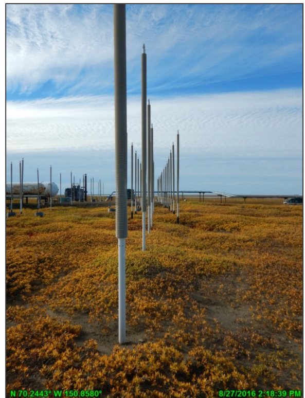
Photo A-14: HDD West north side thermosyphons, looking west; August 27, 2016
