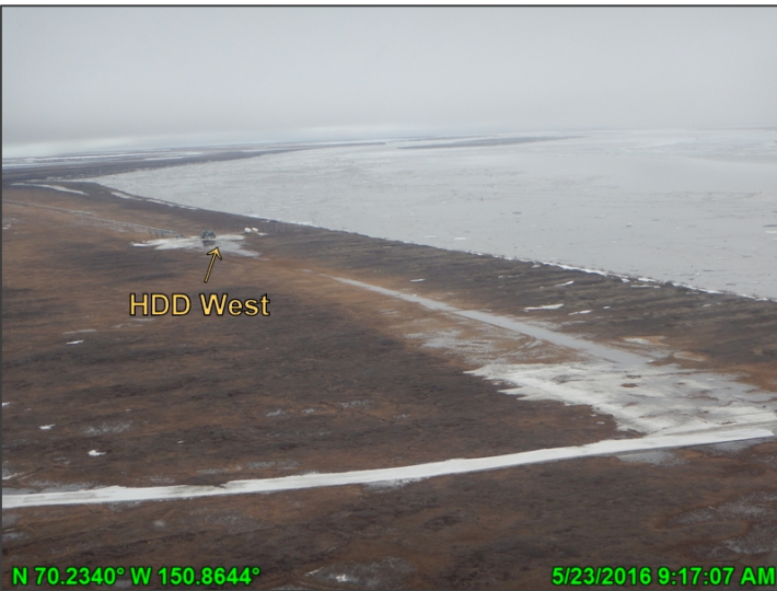
Photo A-6: HDD West during breakup, looking northeast; May 23, 2016
