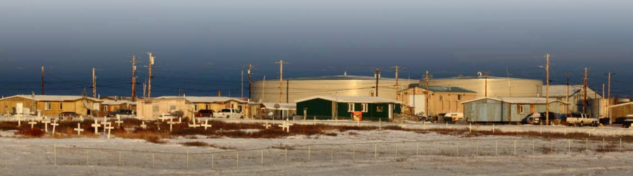
99789 Nuiqsut, Alaska, November 2013, houses on Nigliq Street with water and power plant in background, village cemetery in foreground
