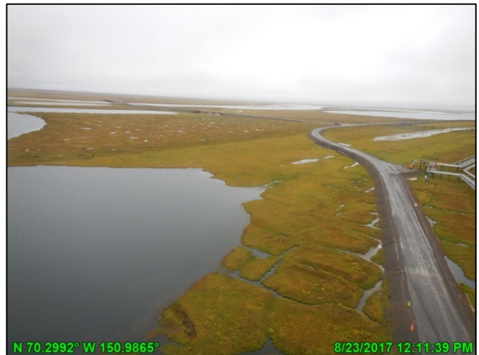
Photo 3.4: Lake L9323, looking northeast toward culvert battery CD4-20A to CD4-23D; August 23, 2017
