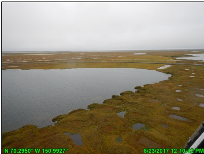
Photo 3.3: Lake L9323, looking southeast toward culvert battery CD4-29 to CD4-33; August 23, 2017
