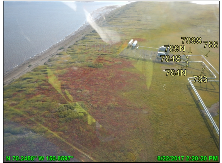
Photo A-6: HDD West, looking southeast; August 22, 2017
