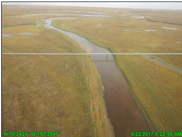
Photo A-29: Miluveach River, looking northwest (downstream); August 22, 2017
