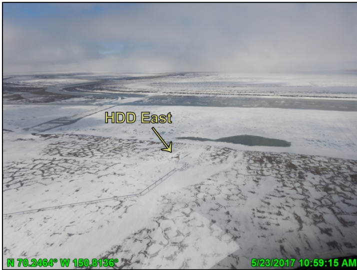
Photo A-11: HDD East during spring breakup, looking southwest; May 23, 2017
