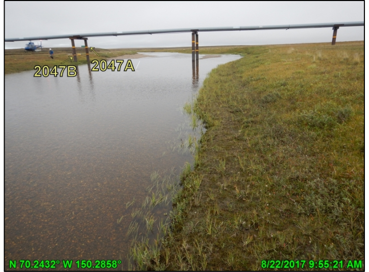
Photo A-34: Miluveach River east bank, looking northwest (downstream); August 22, 2017
