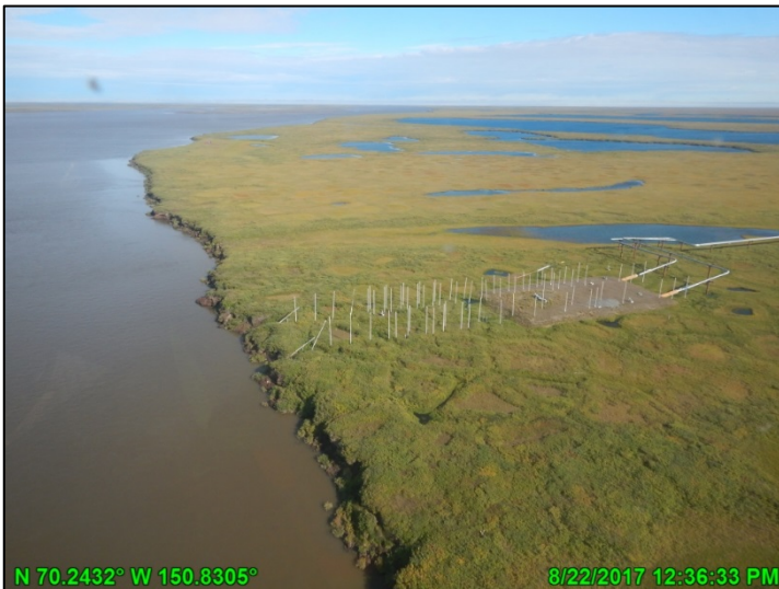
Photo A-15: HDD East, looking north (downstream); August 22, 2017
