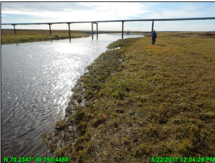
Photo A-27: Kachemach River east bank, looking north (downstream); August 22, 2017
