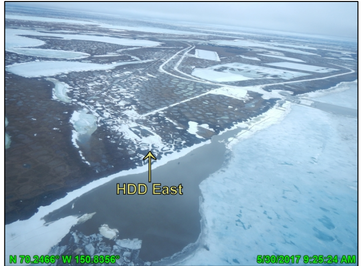
Photo A-14: HDD East during spring breakup, looking southeast; May 30, 2017
