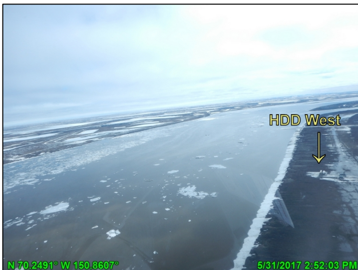
Photo A-1: HDD West during spring breakup, looking south (upstream); May 31, 2017
