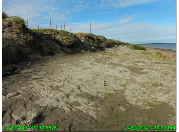
Photo A-10: HDD West bank, looking north (downstream); August 22, 2017
