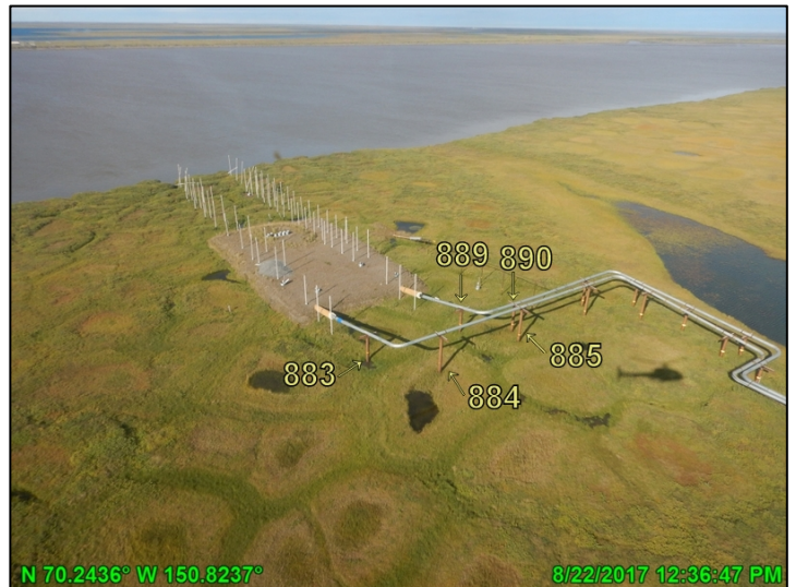
Photo A-16: HDD East, looking west; August 22, 2017
