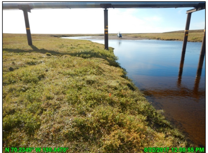
Photo A-28: Kachemach River west bank, looking north (downstream); August 22, 2017
