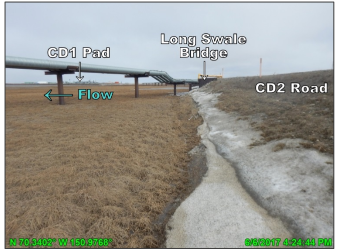
Photo D.6: North side of CD2 road west of the Long Swale Bridge, looking east; June 6, 2017
