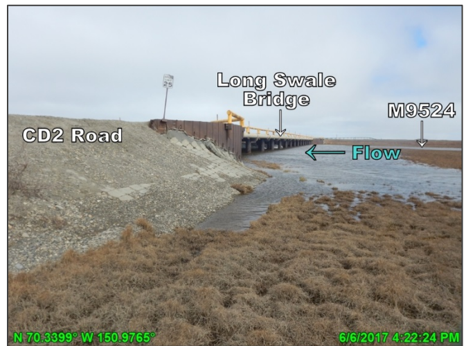
Photo D.8: South side of CD2 road west of the Long Swale Bridge, looking east; June 6, 2017
