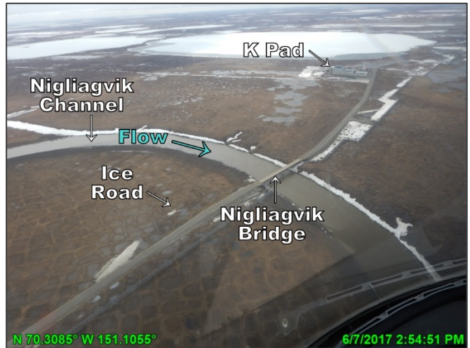
Photo D.24: Nigliagvik Bridge post-breakup, looking southwest; June 7, 2017
