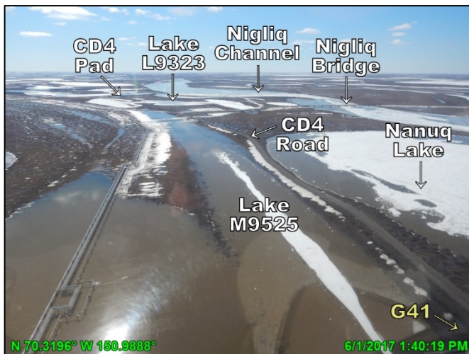
Photo 4.14: North end of CD4 road one day after peak stage, looking south; June 1, 2017
