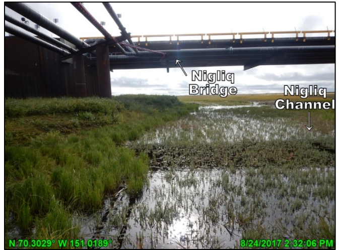
Photo 6.2: East bank of the Nigliq Channel north of the Nigliq Bridge, looking south; August 24, 2017
