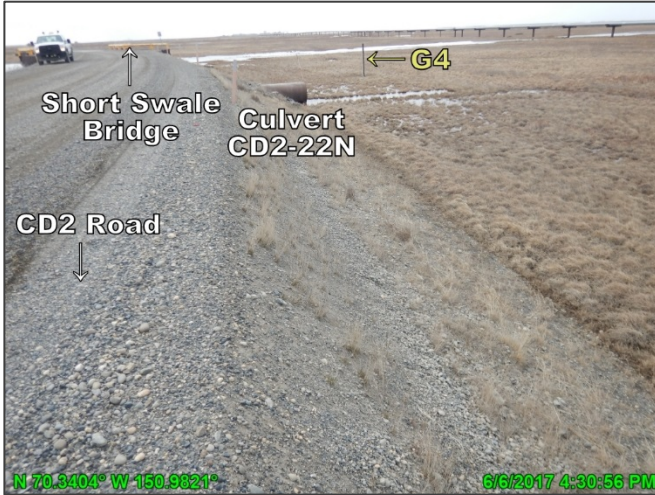
Photo D.1: North side of CD2 road east of Short Swale Bridge, looking west; June 6, 2017
