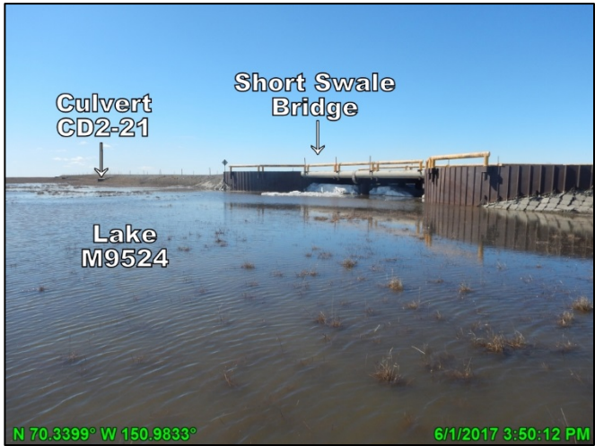
Photo 4.10: Conditions at the CD2 road Short Swale Bridge the day after peak stage, looking northwest (downstream); June 1, 2017
