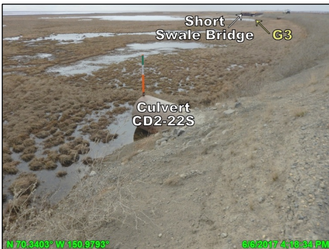
Photo 5.3: South side of CD2 road, looking west; June 6, 2017
