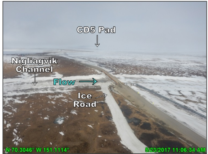
Photo D.22: Nigliagvik Bridge pre-breakup, looking northeast; May 23, 2017
