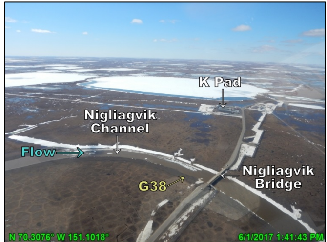
Photo 4.23: Nigliagvik Bridge conditions the day of discharge measurement, looking east; June 1, 2017
