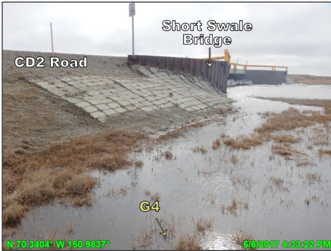
Photo D.5: North side of CD2 road east of the Short Swale Bridge, looking southwest; June 6, 2017
