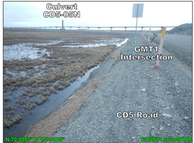
Photo D.14: East side of CD5 road south of CD5 pad near the GMT1 Road, looking south; June 7, 2017
