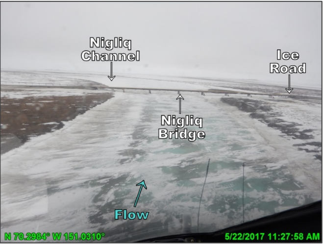
Photo D.28: Nigliq Bridge pre-breakup, looking north (downstream); May 22, 2017
