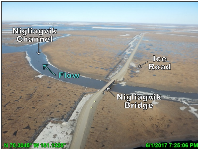
Photo D.23: Nigliagvik Bridge during breakup, looking east; June 1, 2017
