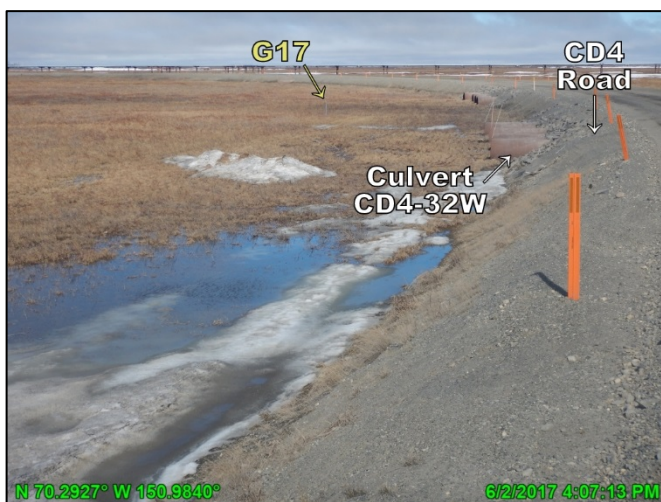
Photo 4.16: CD4 road at gage G17 and associated culverts the day of measured discharge, looking east; June 2, 2017
