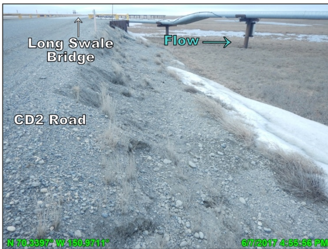
Photo D.7: North side of CD2 road east of Long Swale Bridge, looking west; June 7, 2017
