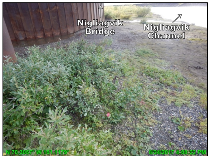
Photo 6.4: East bank of Nigliagvik Channel at the Nigliagvik Bridge abutment, looking south; August 24, 2017
