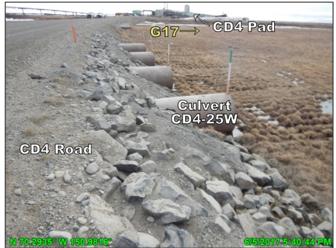
Photo D.10: North side of CD4 road east of CD4 pad, looking west; June 5, 2017
