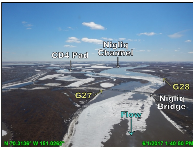
Photo 4.19: Nigliq Bridge the day of peak discharge and the day after peak stage, looking south (upstream); June 1, 2017
