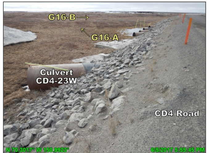
Photo D.12: West side of CD4 road south of CD5 road, looking north; June 5, 2017
