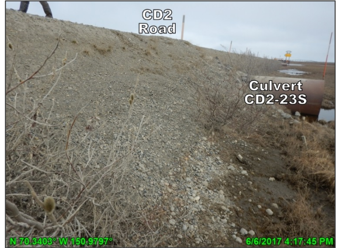
Photo D.2: South side of CD2 road east of Short Swale Bridge, looking east; June 6, 2017
