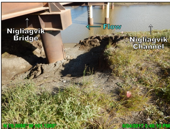
Photo 6.3: Bank subsidence at the west bank of the Nigliagvik Bridge, looking east; August 24, 2017
