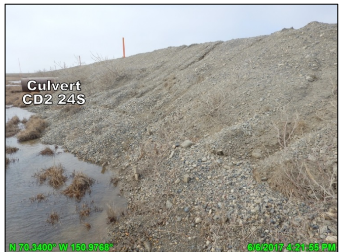
Photo 5.4: South side of CD2 road near the Long Swale Bridge looking west; June 6, 2017
