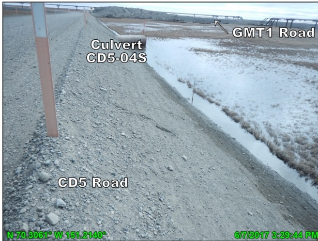
Photo D.13: West side of CD5 road south of CD5 pad, looking south; June 7, 2017
