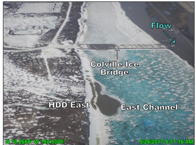
Photo D.16: Colville River East Channel at HDD during breakup, looking southeast (upstream); May 26, 2017
