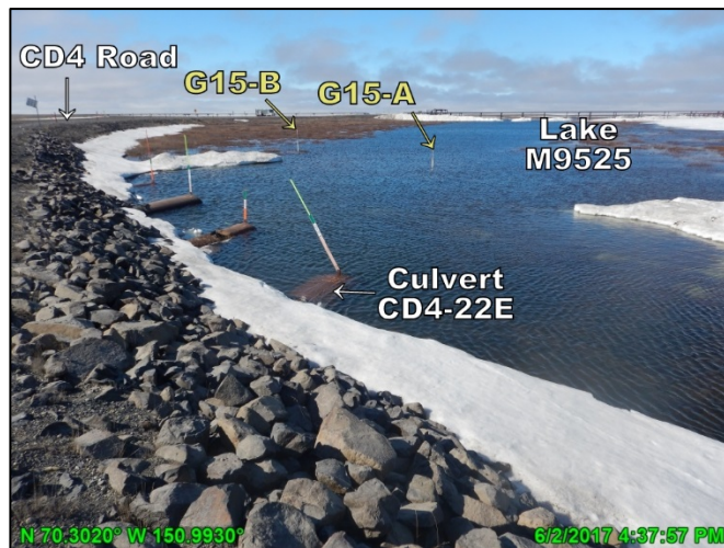
Photo 4.15: Equalization at CD4 road culverts at gage G15/G16 two days after peak stage, looking northeast; June 2, 2017
