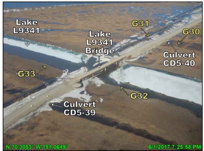
Photo 4.25: Low flow through a culvert associated with gages G30/31, looking west; June 1, 2017
