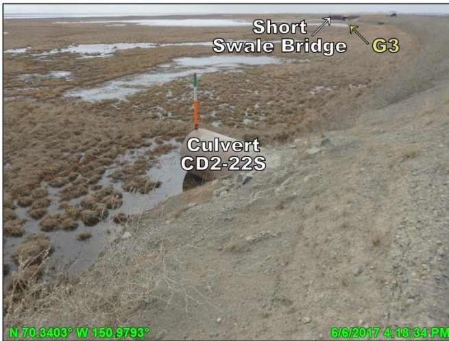
Photo D.3: South side of CD2 road, looking south; June 6, 2017
