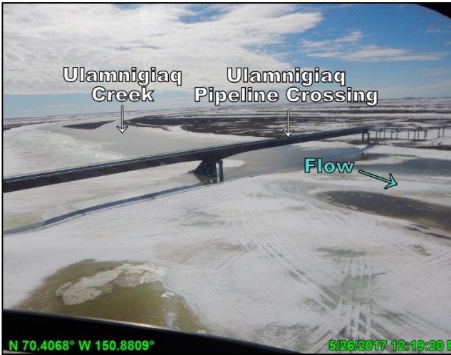
Photo 3.4: Floodwater at the Ulamniglaq Pipeline Crossing, looking southeast (upstream); May 26, 2017
