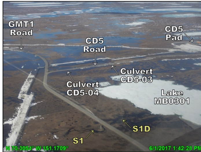
Photo 4.26: Hydraulic connections through CD5 culverts CD5-03 and CD5-04 and culverts at S1/S1D gages, looking northwest; June 1, 2017
