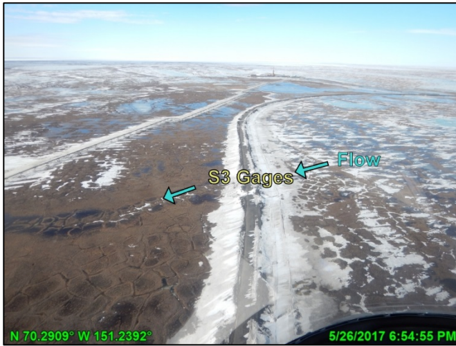
Photo A.1: GMT1 access road, looking northeast; May 26, 2017
