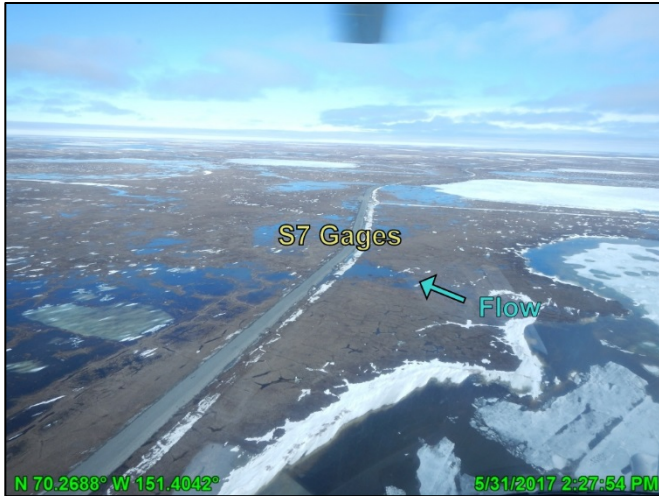
Photo A.36: GMT1 access road, looking east; May 31, 2017
