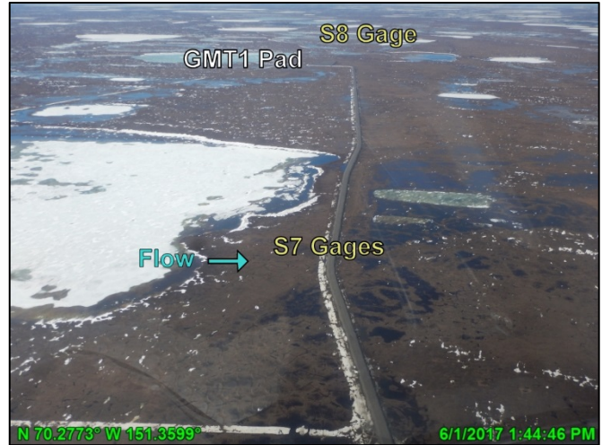
Photo A.37: GMT1 access road, looking west; June 1, 2017
