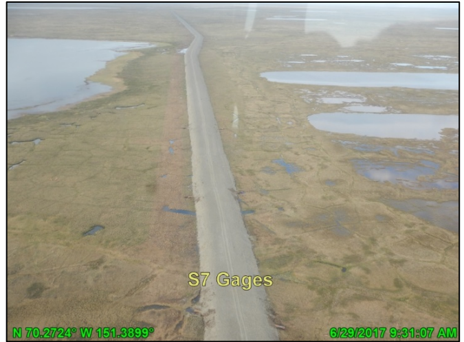
Photo A. 43: GMT1 access road near S7 monitoring location, looking west; June 29, 2017
