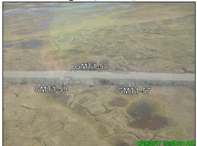
Photo A.10: GMT1 culverts 57, 58, and 59, looking southeast; June 29, 2017
