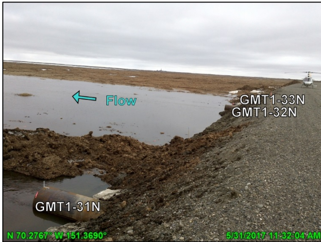
Photo A.24: Culverts GMT1-31 through 33, looking northeast; May 31, 2017
