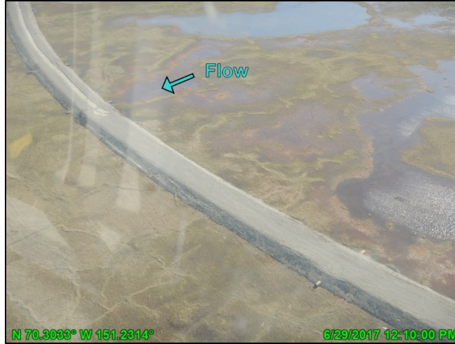
Photo A.11: GMT1 access road, looking east; June 29, 2017
