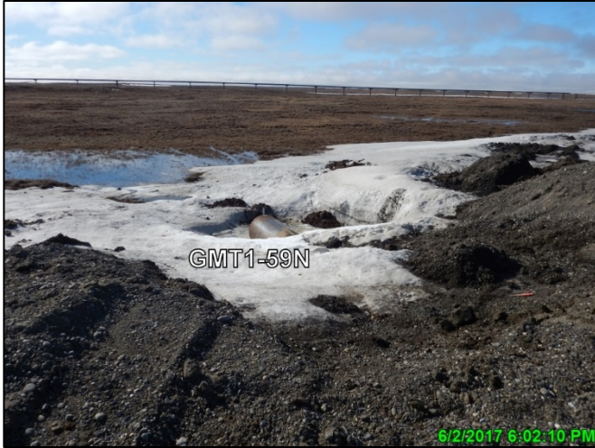
Photo A.5: GMT1-59N culvert, looking north; June 2, 2017
