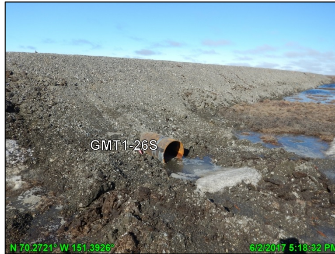
Photo 3.8: Culvert GMT1-26, looking northeast; June 2, 2017
