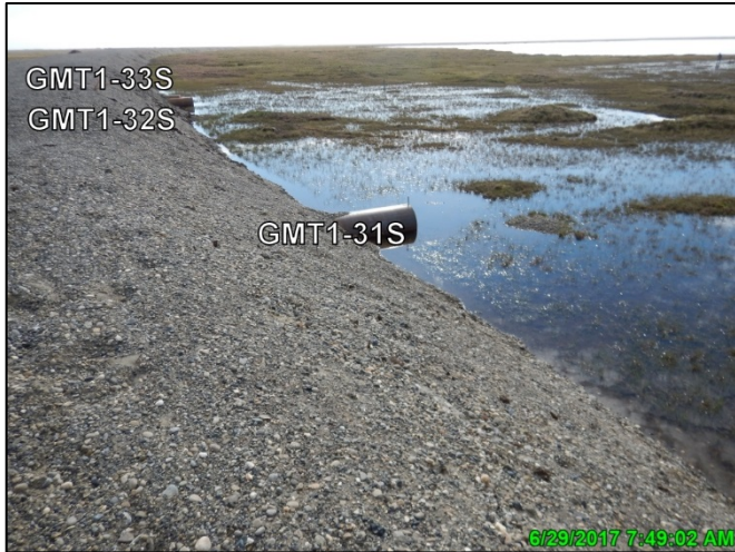
Photo A.32: Post-breakup conditions at culverts GMT1-31 through 33, looking east; June 29, 2017
