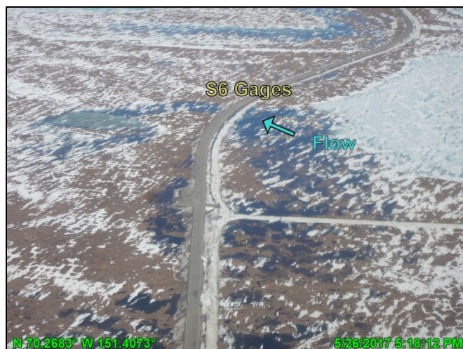
Photo 3.2: Drifted snow and ice road along upstream (south) side of the GMT1 access road, looking east; May 26, 2017
