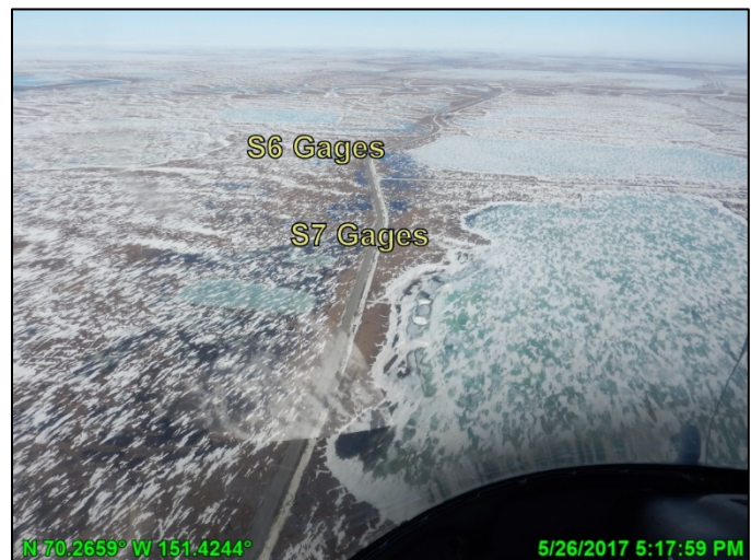
Photo 3.1: Local melt accumulating along GMT1 access road, looking east; May 26, 2017
