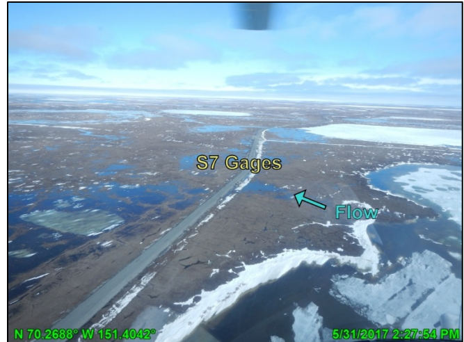
Photo 3.7: GMT1 access road, looking east; May 31, 2017
