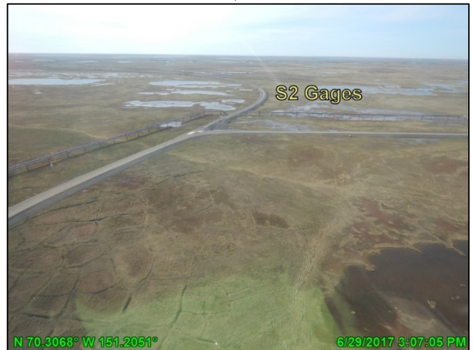
Photo A.8: GMT1 access road at intersection with CD5 road near S2 monitoring location, looking west; June 29, 2017
