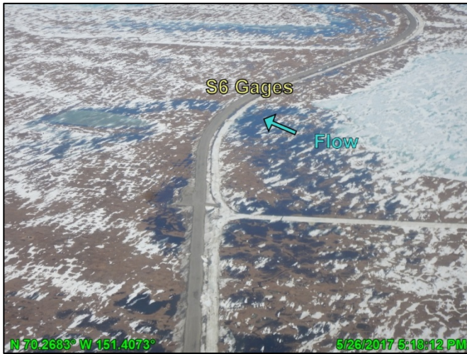
Photo A.22: GMT1 access road conditions, looking northeast; May 26, 2017
