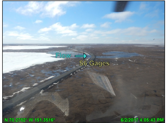
Photo A.27: GMT1 access road, looking west; June 2, 2017
