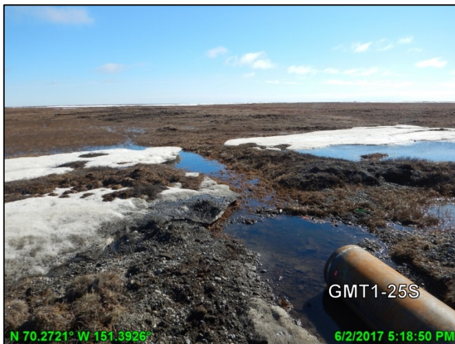
Photo A.40: Culvert GMT1-25, looking south; June 2, 2017
