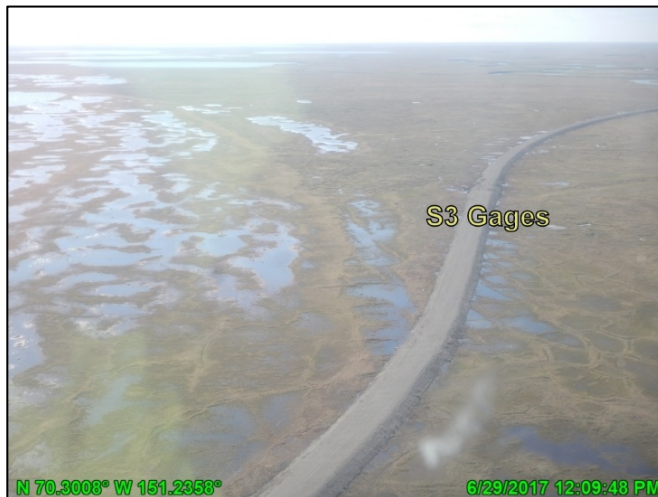
Photo A.9: GMT1 access road near S3 monitoring location, looking southwest; June 29, 2017
