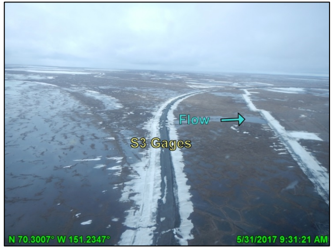
Photo A.2: GMT1 access road, looking southwest; May 31, 2017
