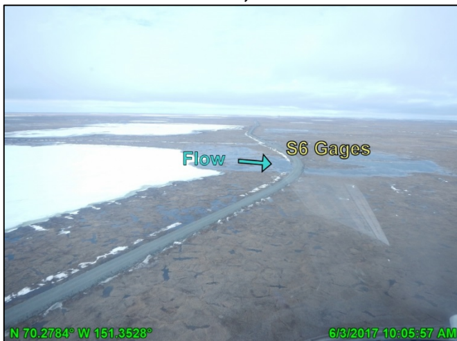
Photo A.30: GMT1 access road, looking west; June 3, 2017
