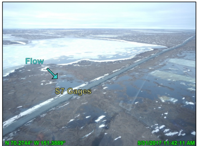
Photo A.35: Breakup monitoring, looking southwest; May 31, 2017
