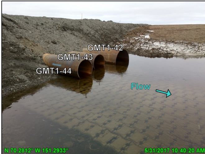
Photo A.16: Culverts GMT1-42 through 44, looking west; May 31, 2017
