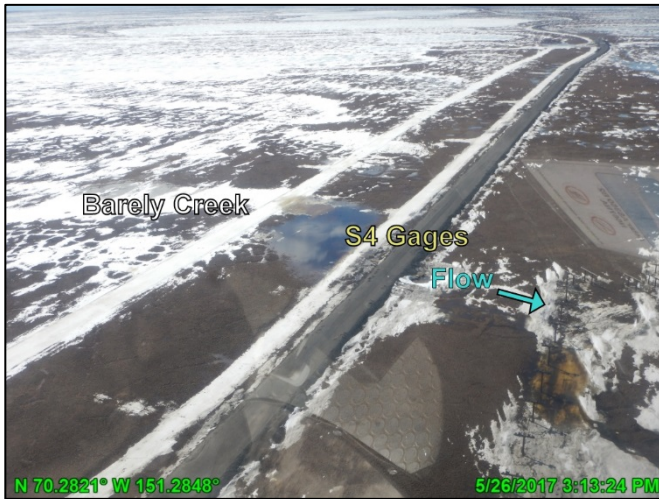
Photo A.12: Conditions along GMT1 access road, looking southwest; May 26, 2017
