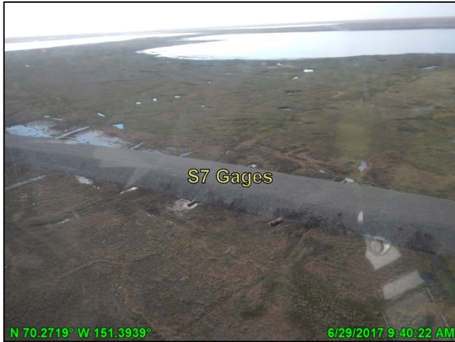
Photo A.42: Post-breakup conditions at S7 gages, looking southeast; June 29, 2017
