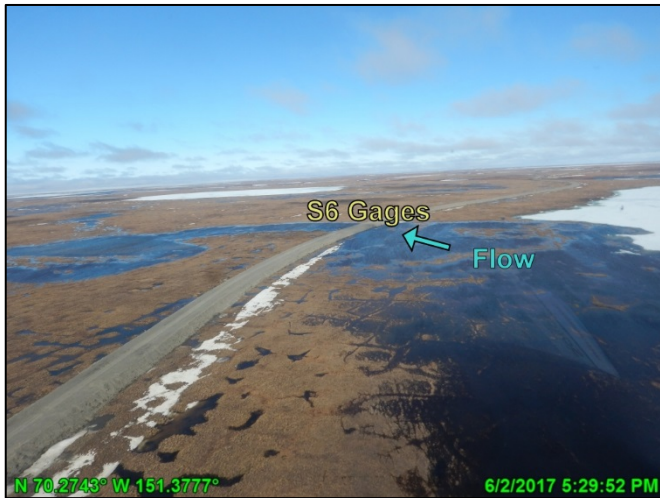
Photo A.28: GMT1 access road, looking east; June 2, 2017
