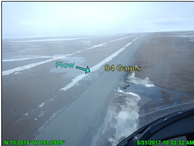
Photo A.14: Culverts GMT1-42 through 44, looking east; May 31, 2017
