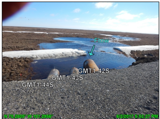
Photo A.19: Culverts GMT1-42 through 44, looking southwest; June 2, 2017
