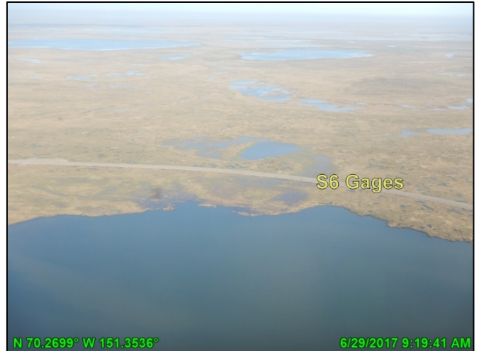
Photo A.33: GMT1 access road near S6 monitoring location, looking northwest; June 29, 2017
