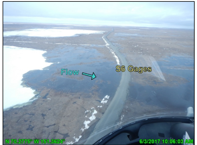
Photo A.29: GMT1 access road, looking west; June 3, 2017
