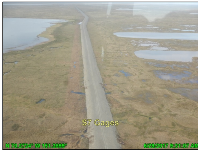
Photo D.36: S7 gages and culverts, looking west; June 29, 2017
