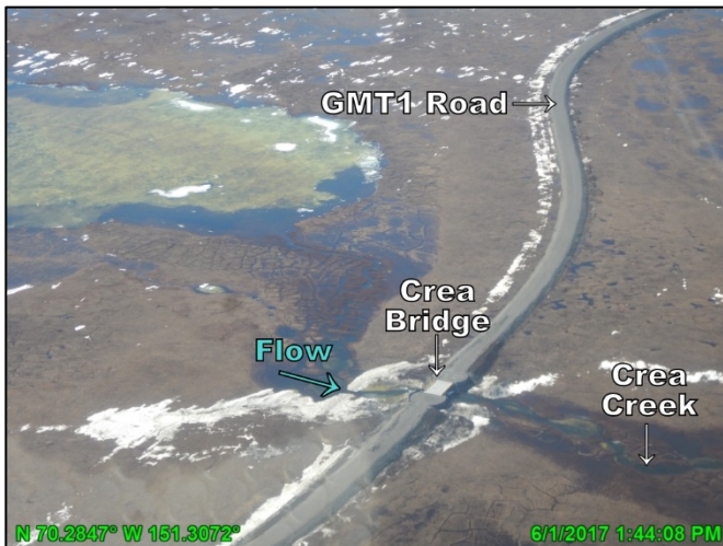
Photo 4.11: Ice and snow influence at the Crea Bridge the day of spring peak discharge, looking southwest; June 1, 2017
