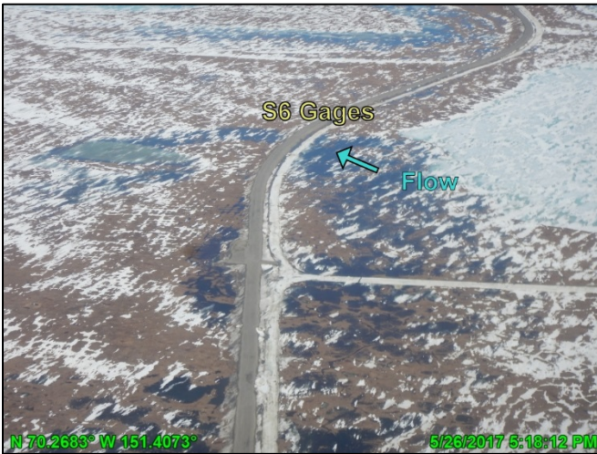
Photo D.21: S6 gages and culverts, looking east; May 26, 2017
