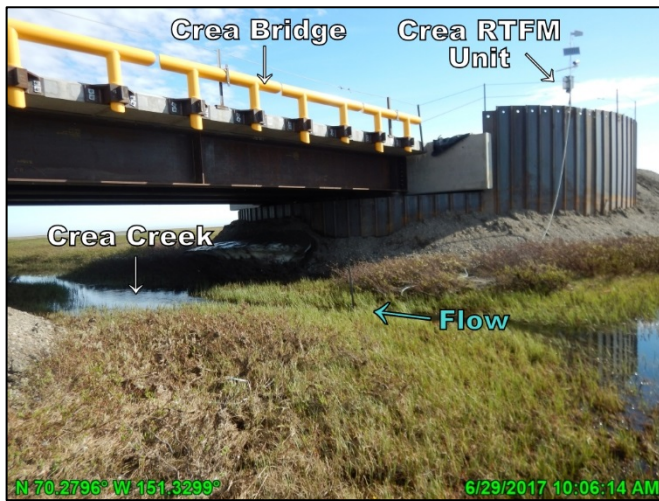
Photo 7.1: Crea Bridge right (east) abutment, looking northeast (downstream); June 29, 2017
