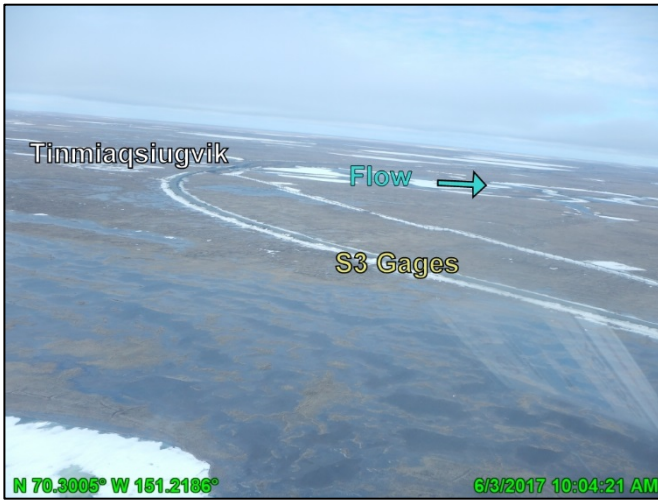
Photo D.17: S3 gages and culverts, looking west; June 3, 2017
