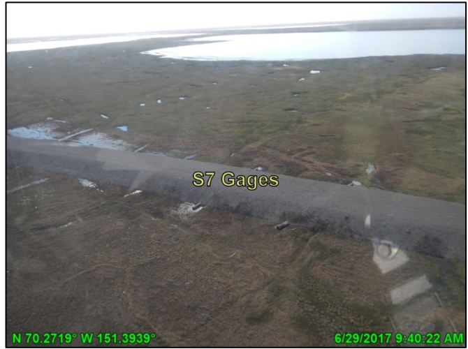
Photo D.35: S7 gages and culverts, looking southeast; June 29, 2017
