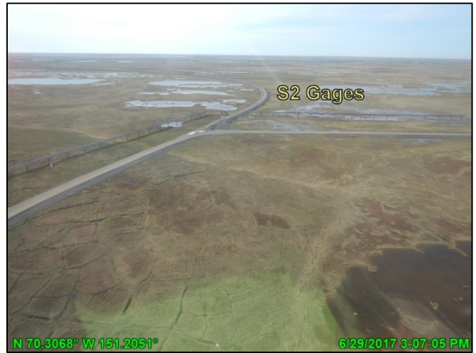
Photo D.18: S2 gages and culverts, looking west; June 29, 2017
