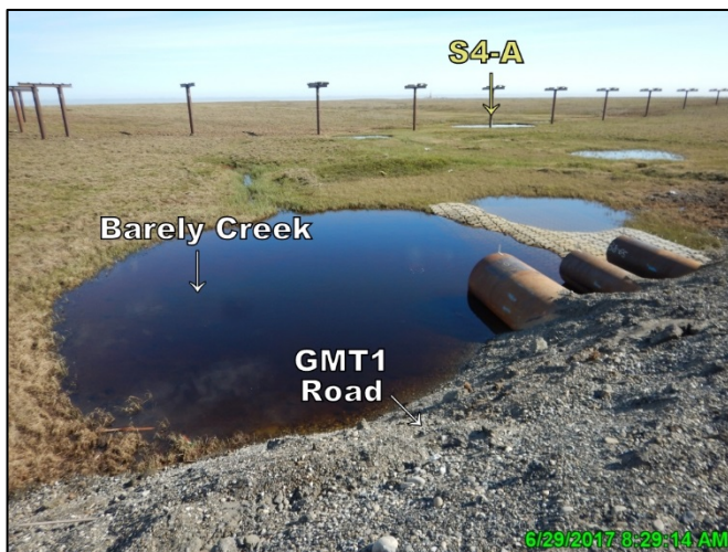
Photo 7.3: Barely Creek culvert battery outlet, looking northeast (downstream); June 29, 2017
