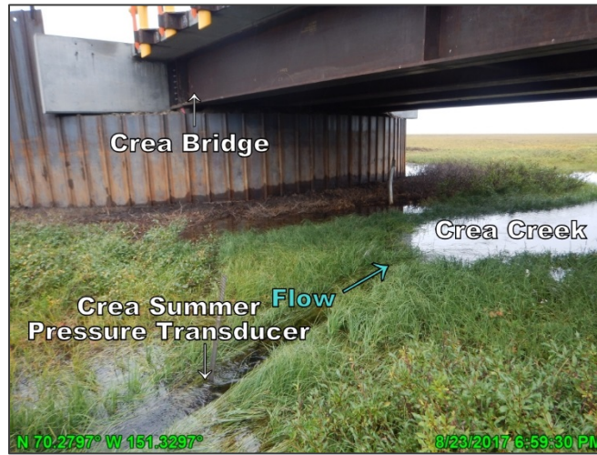
Photo D.9: Crea Bridge left (west) abutment, looking northwest (downstream); August 23, 2017
