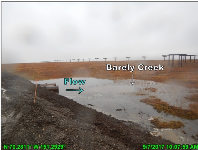
Photo D.3: Barely Creek culvert battery outlet, looking northwest; September 7, 2017
