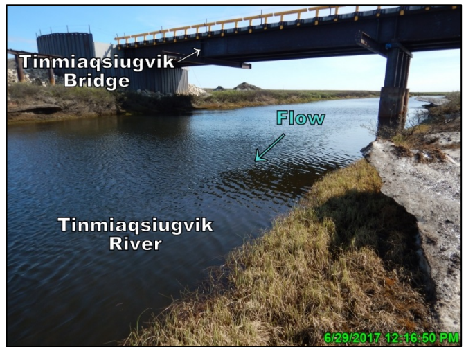
Photo 7.2: Tinmiaqsiugvik Bridge right (east) abutment and east bank, looking southeast (upstream); June 29, 2017
