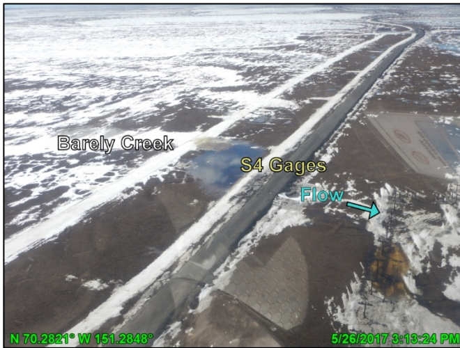
Photo 4.15: Conditions at the Barely Creek culvert battery the day of spring peak stage at gage S4-C, looking west; May 26, 2017
