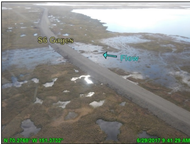
Photo D.27: S6 gages and culverts, looking east; June 29, 2017
