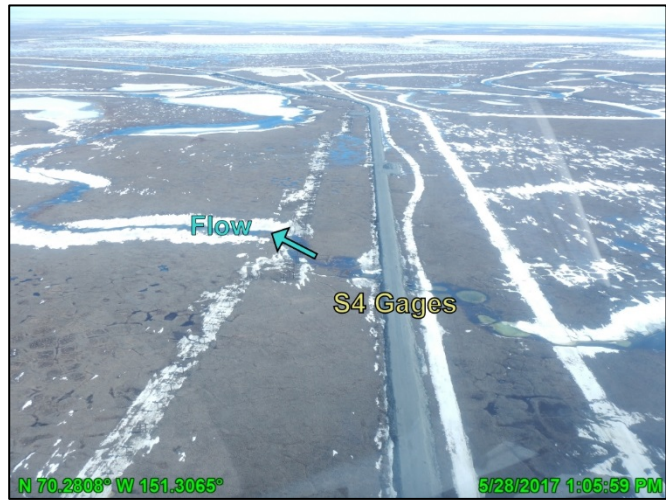
Photo 4.16: Flow through the Barely Creek culvert battery, looking east; May 28, 2017
