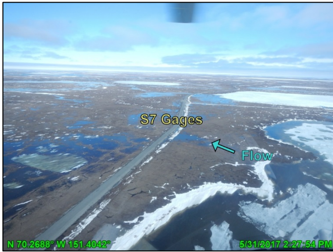
Photo D.30: S7 gages and culverts, looking east; May 31, 2017
