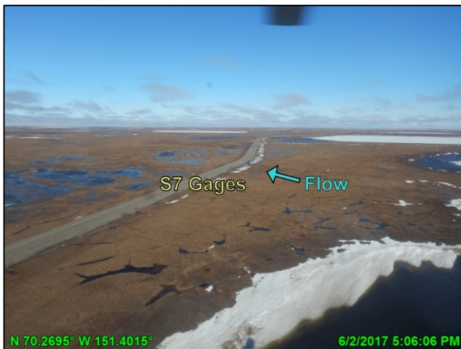
Photo D.32: S7 gage and culverts, looking east; June 2, 2017
