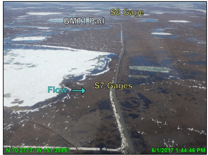
Photo D.31: S7 gages and culverts, looking west; June 1, 2017
