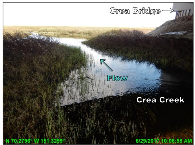
Photo D.8: Flow under Crea Bridge, looking north (downstream); June 29, 2017
