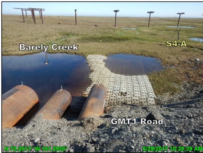
Photo 4.22: Summer flow through one Barely Creek culvert, looking north; June 29, 2017
