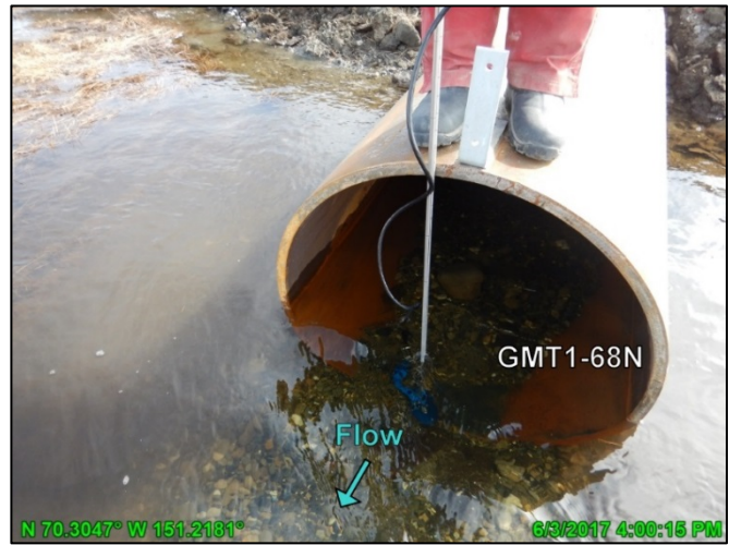
Photo 4.25: Culvert GMT1-68 the day of spring discharge measurement, looking south; June 3, 2017
