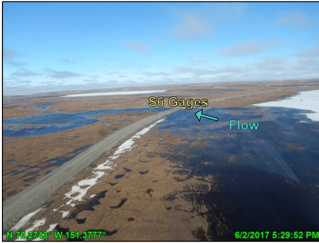
Photo D.25: S6 gages and culverts, looking east; June 2, 2017
