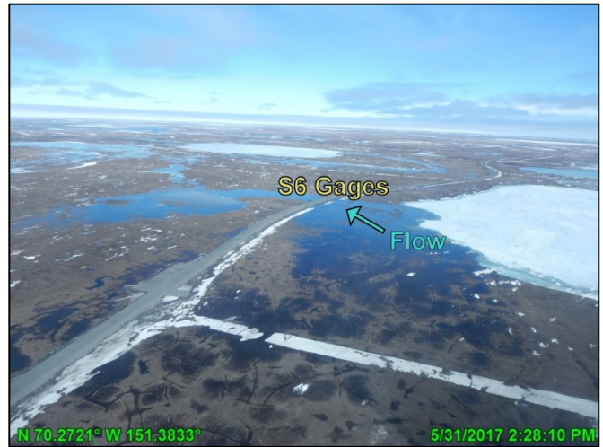
Photo D.22: S6 gages and culverts, looking northeast; May 31, 2017
