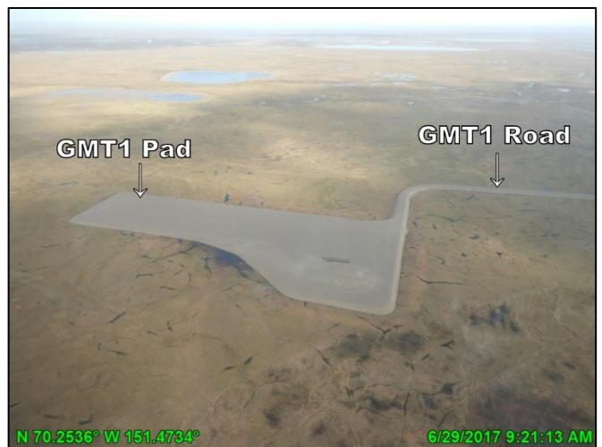
Photo 7.4: GMT1 pad, looking northwest; June 29, 2017
