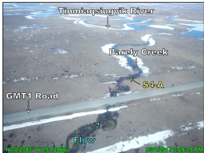
Photo 4.18: Conditions at the Barely Creek culvert battery the day of spring peak discharge, looking northeast (downstream); May 31, 2017
