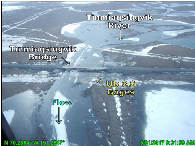
Photo 4.1: Conditions at the Tinmiaqsiugvik Bridge the day of spring peak stage and discharge, looking southeast; May 31, 2017
