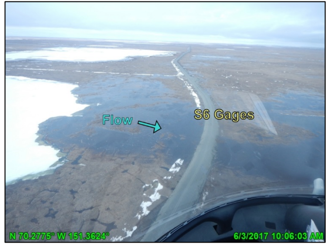
Photo D.26: S6 gages and culverts, looking west; June 3, 2017
