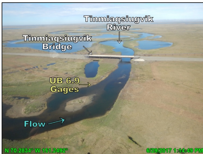
Photo 4.4: Open channel conditions at the Tinmiaqsiugvik Bridge, looking northwest (downstream); June 29, 2017
