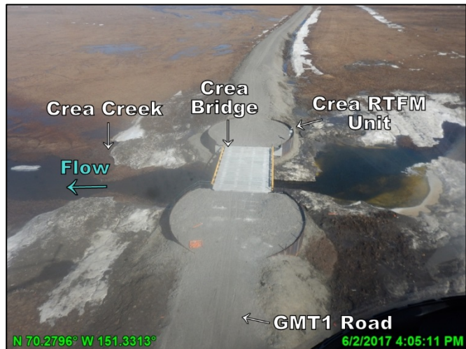
Photo 4.12: Conditions at the Crea Bridge the day of spring discharge measurement, looking east; June 2, 2017
