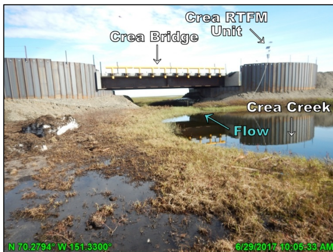
Photo 4.13: Open channel conditions at the Crea Bridge, looking northeast (downstream); June 29, 2017
