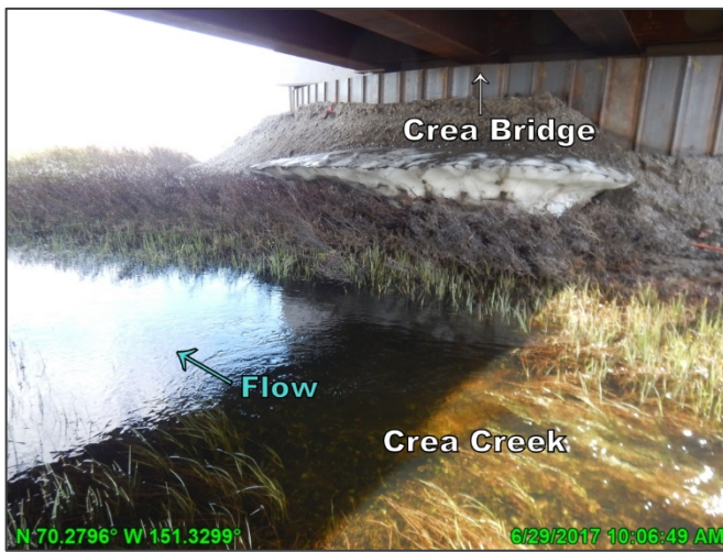
Photo D.7: Crea Bridge right (east) abutment, looking northeast (downstream); June 29, 2017
