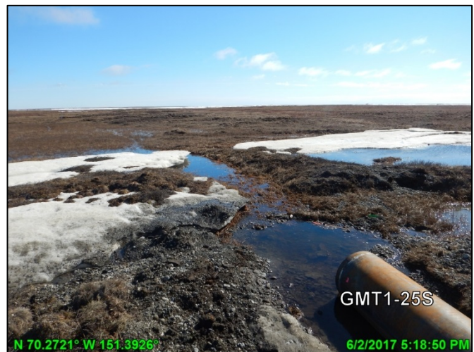
Photo D.33: S7 culvert GMT1-25, looking south; June 2, 2017
