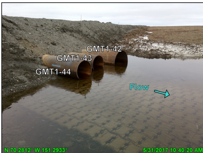
Photo 4.17: Conditions at the Barely Creek culvert battery outlet the day of spring peak discharge, looking west; May 31, 2017
