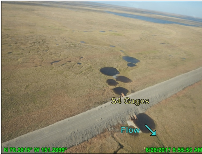
Photo D.1: Barely Creek culvert battery, looking southwest (upstream); June 28, 2017
