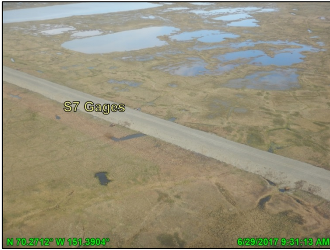
Photo D.34: S7 gages and culverts, looking northwest; June 29, 2017
