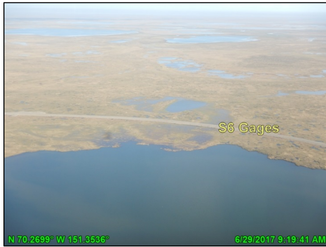
Photo D.29: S6 gages and culverts, looking northwest; June 29, 2017
