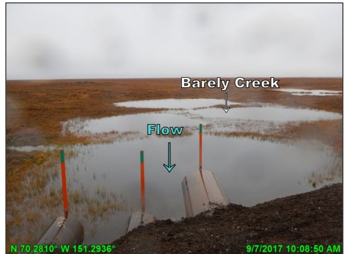
Photo D.4: Barely Creek culvert battery inlet, looking south (upstream); September 7, 2017
