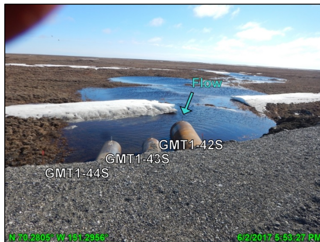
Photo 4.21: Barely Creek culvert battery the day of spring measured discharge, looking southwest (upstream); June 2, 2017
