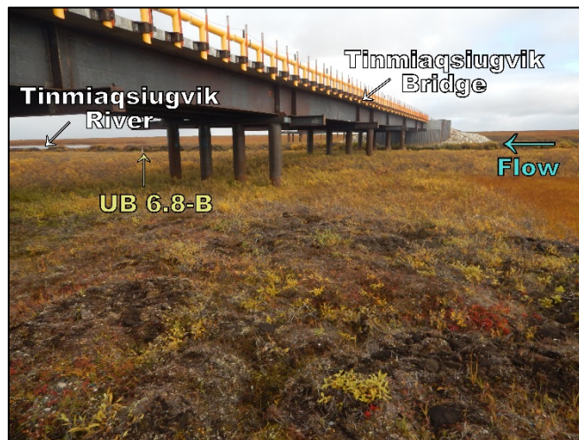
Photo 4.8: Flow confined within the main channel at the Tinmiaqsiugvik Bridge the day of summer discharge measurement, looking northeast; September 9, 2017
