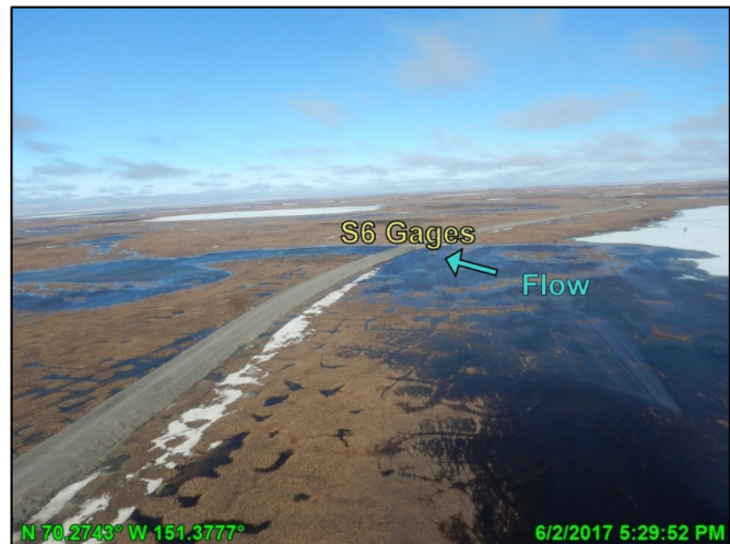
Photo 4.33: S6 gages and culverts the day of spring measured discharge, looking northeast; June 2, 2017
