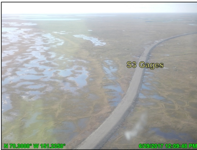
Photo D.19: S3 gages and culverts, looking west; June 29, 2017
