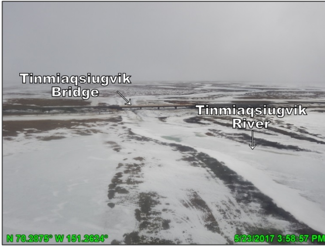
Photo D.40: Tinmiaqsiugvik River pre-breakup, looking southeast (upstream); May 23, 2017
