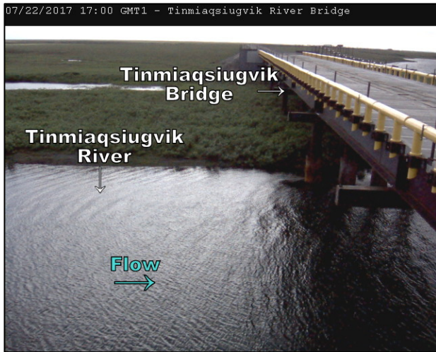
Photo 4.6: Peak summer discharge (upstream flow direction) at the Tinmiaqsiugvik Bridge, looking southwest; July 22, 2017
