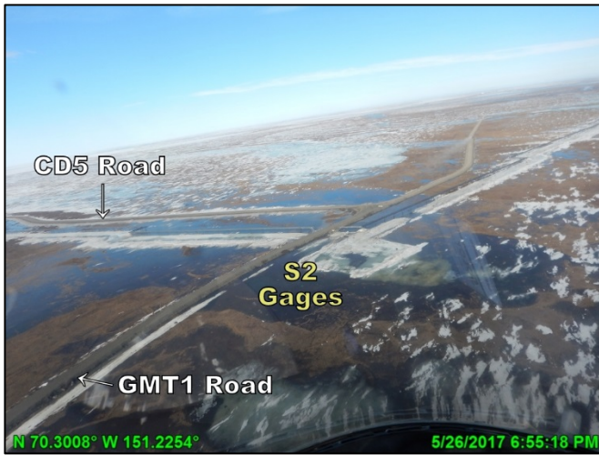
Photo 4.24: S2 gages and culverts the day prior to spring peak stage and the day after spring peak discharge, looking northeast; May 26, 2017
