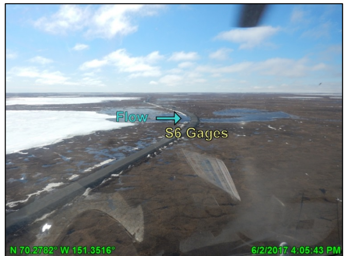
Photo D.24: S6 gages and culverts, looking west; June 2, 2017
