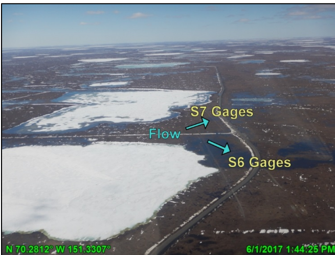
Photo D.23: S6 and S7 gages and culverts, looking west; June 1, 2017
