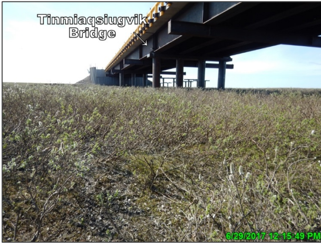
Photo D.14: Tinmiaqsiugvik Bridge left (west) abutment, looking northwest; June 29, 2017
