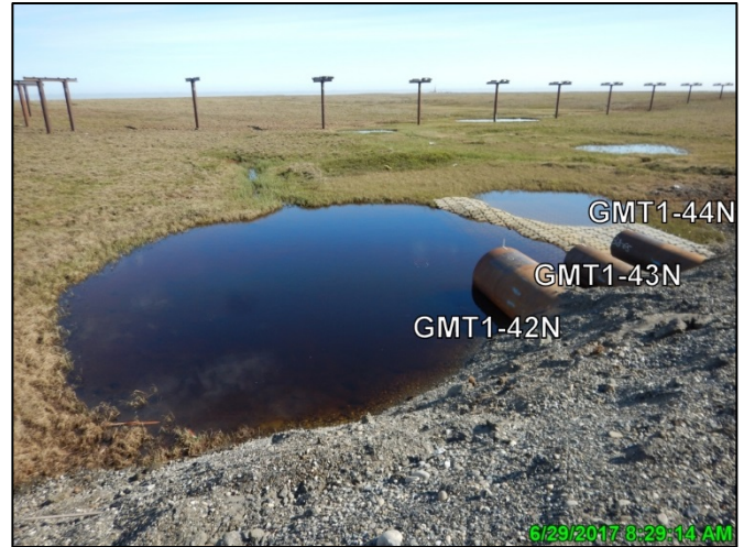
Photo D.2: Barely Creek culvert battery outlet, looking northeast (downstream); June 29, 2017
