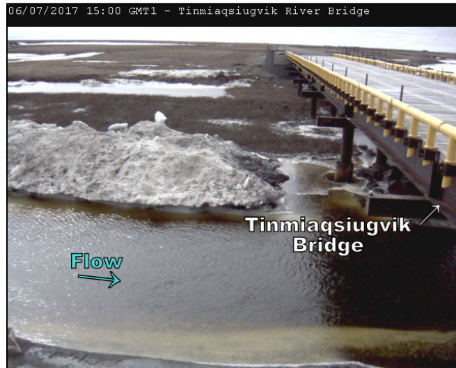
Photo 3.10: Stage receding at the Tinmiaqsiugvik Bridge, looking southwest; June 7, 2017
