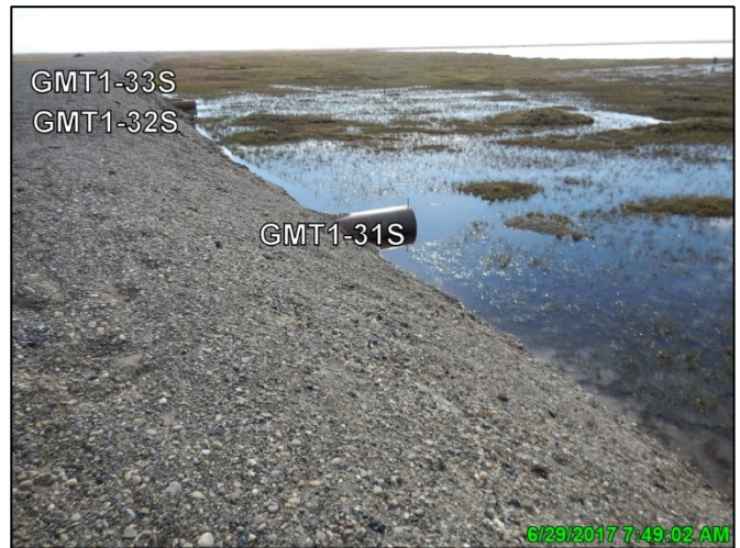
Photo D.28: S6 culverts GMT1-31 through 33, looking east; June 29, 2017
