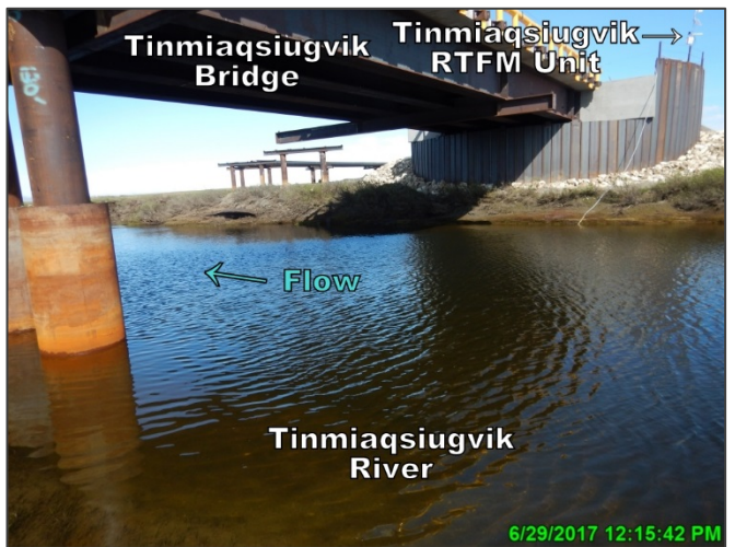
Photo D.13: Tinmiaqsiugvik Bridge right (east) abutment, looking northeast; June 29, 2017
