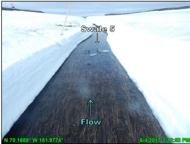
Photo 4.41: Conditions at Swale 5 the day of measured discharge and highest recorded stage, looking north (downstream); June 4, 2017
