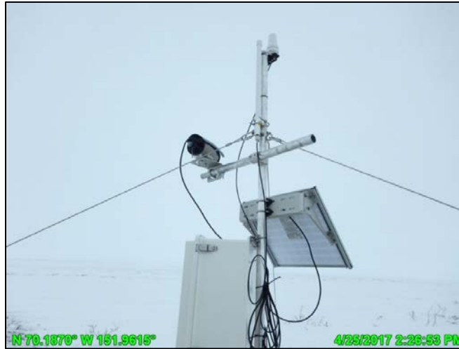
Photo 2.3: Remote camera setup at J 13.8; April 25, 2017
