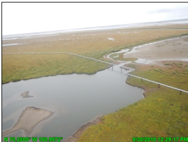
Photo 9: Hydraulic connection between Lake L9324 and South Paleo Lake, looking northeast; August 30, 2018
