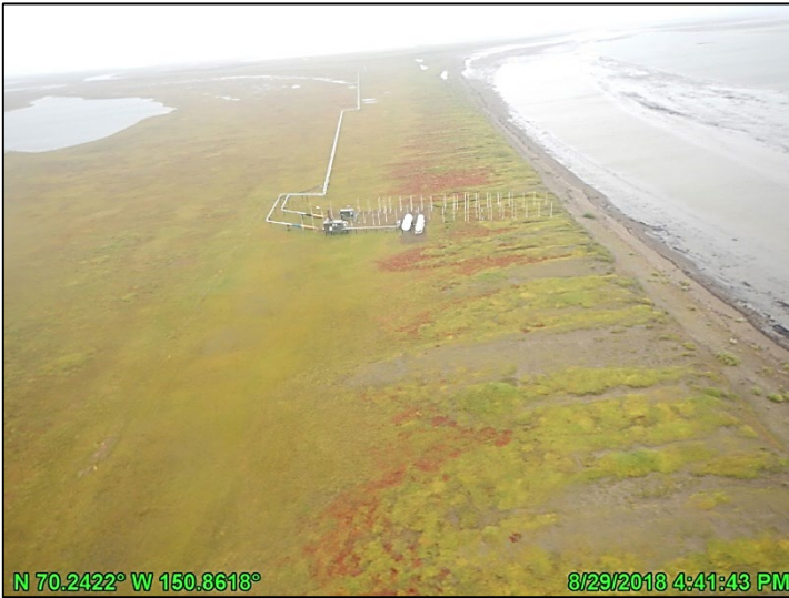
Photo A.5: HDD West after spring breakup, looking north; August 29, 2018
