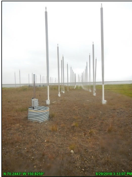
Photo A.17: HDD East gravel pad and north side thermosyphons, looking west; August 29, 2018
