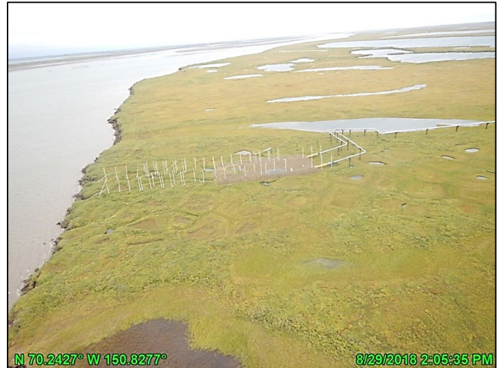
Photo A.14: HDD East after spring breakup, looking north; August 29, 2018
