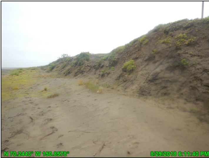
Photo A.9: HDD West bank, looking south (downstream); August 29, 2018
