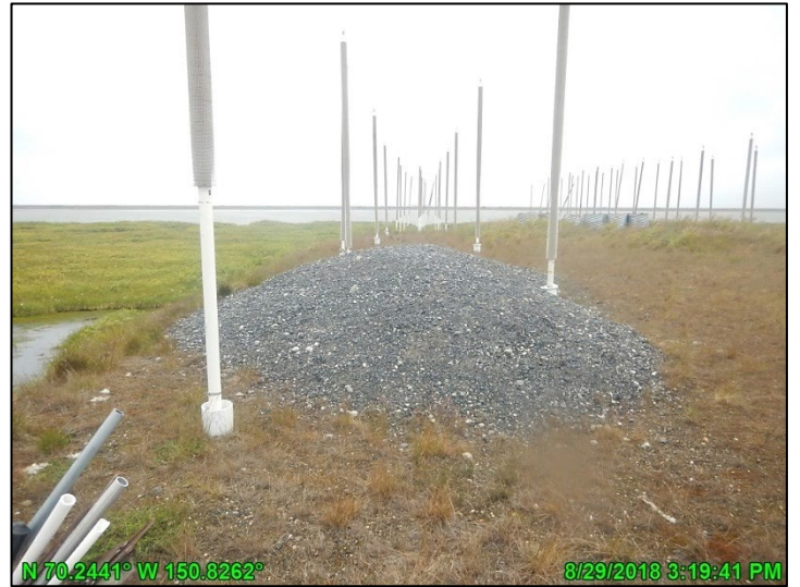
Photo A.18: HDD East gravel pad and south side thermosyphons, looking west; August 29, 2018
