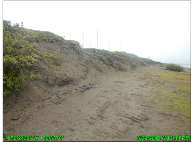
Photo A.10: HDD West bank, looking north (downstream); August 29, 2018
