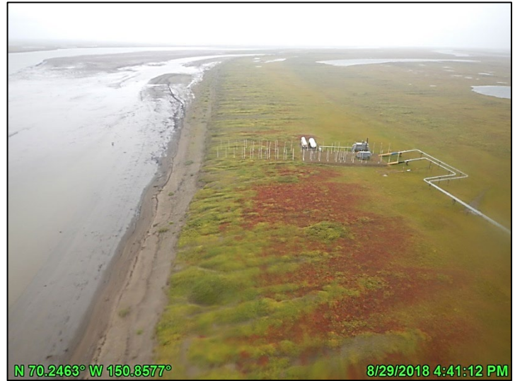
Photo A.6: HDD West after spring breakup, looking south; August 29, 2018
