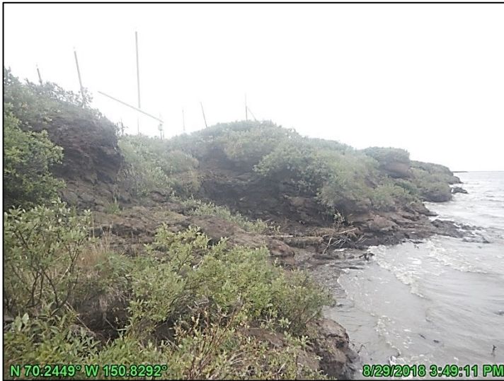
Photo A.19: HDD East bank, looking south (upstream); August 29, 2018
