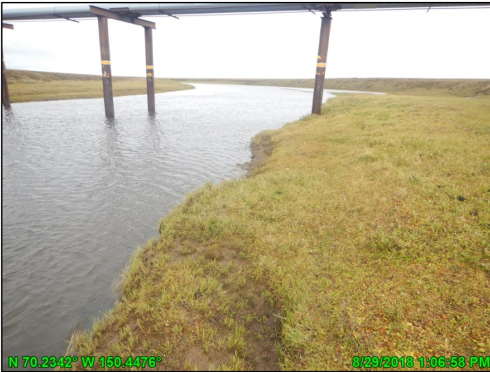
Photo A.27: Kachemach River east bank, looking north (downstream); August 29, 2018
