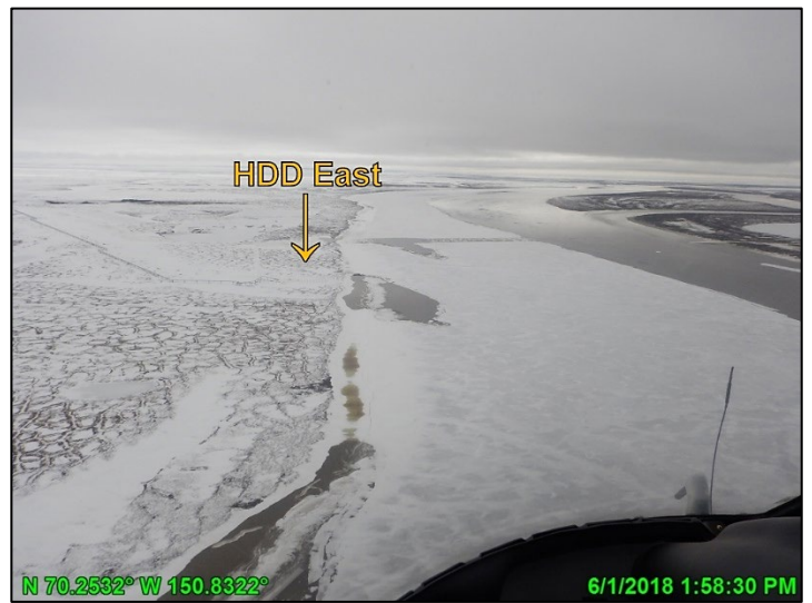
Photo A.12: HDD East pre-breakup, looking south; June 1, 2018
