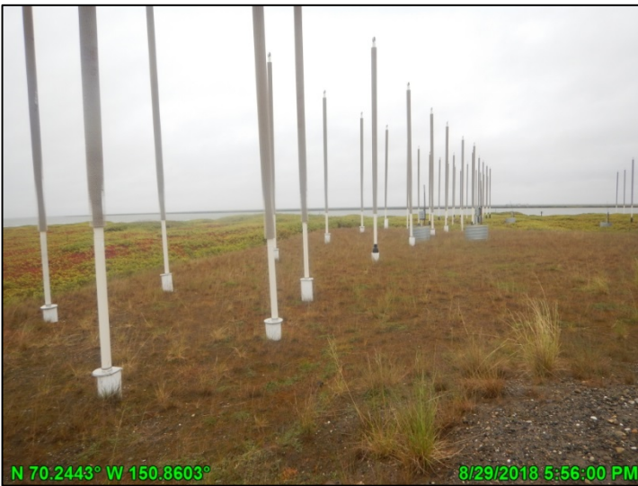
Photo A.7: HDD West gravel pad and north side thermosyphons, looking east; August 29, 2018
