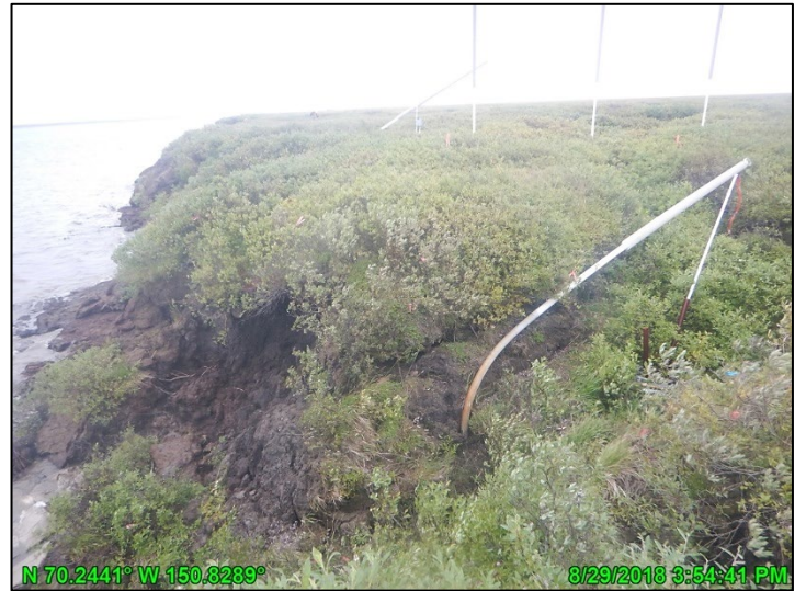
Photo A.20: HDD East bank, looking north (downstream); August 29, 2018
