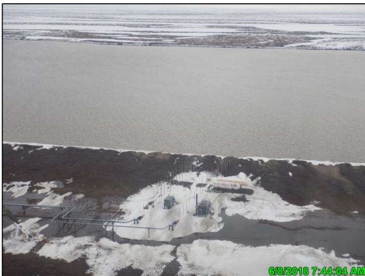
Photo A.3: HDD West during spring breakup, looking northeast; June 8, 2018
