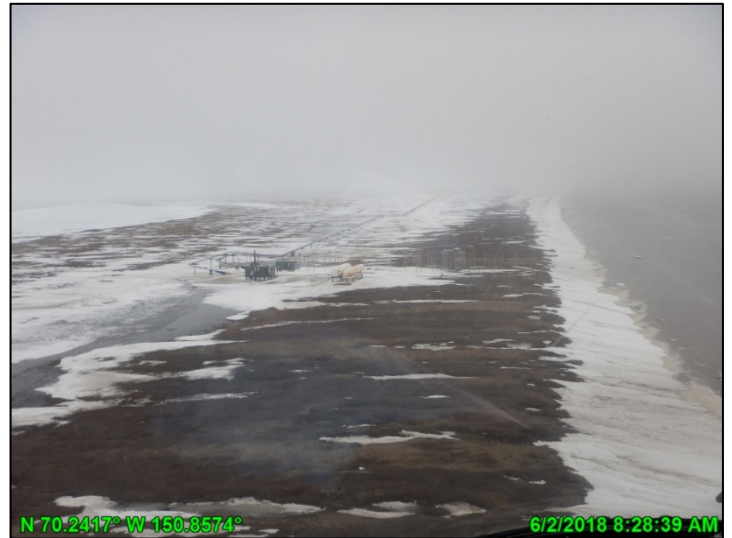
Photo A.2: HDD West during spring breakup, looking north; June 2, 2018
