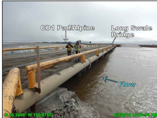
Photo 4.22: Long Swale Bridge the day of the discharge measurement, looking east; June 3, 2018
