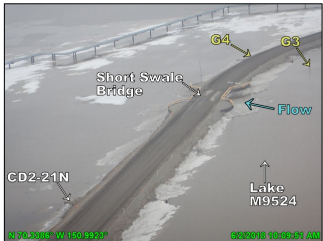
Photo 4.21: CD2 road Short Swale Bridge the day of peak stage, looking northeast (downstream); June 2, 2018
