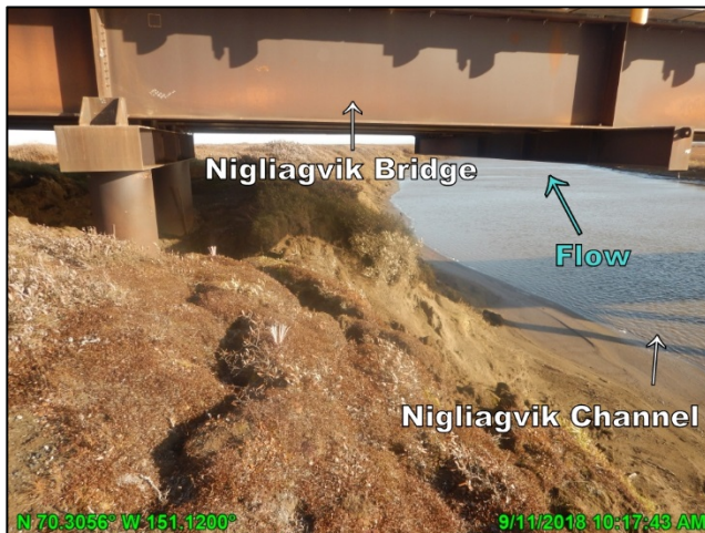
Photo 6.3: West bank of the Nigliagvik Channel at the Nigliagvik Bridge, looking north; September 11, 2018
