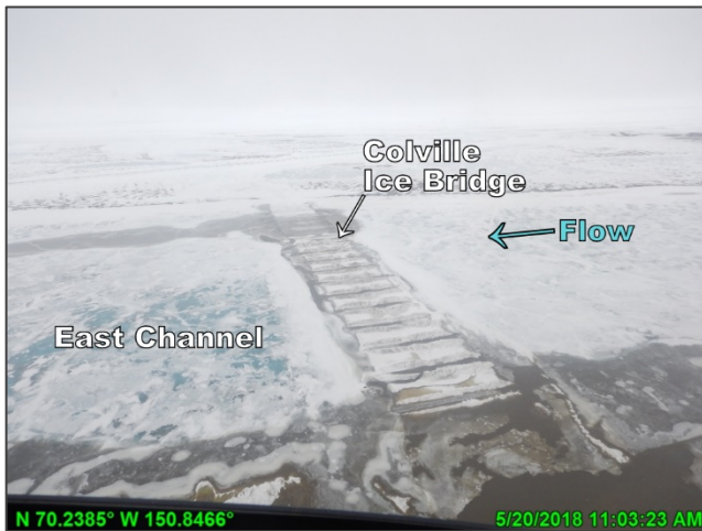
Photo D.6: Colville River East Channel at HDD pre-breakup, looking east; May 20, 2018
