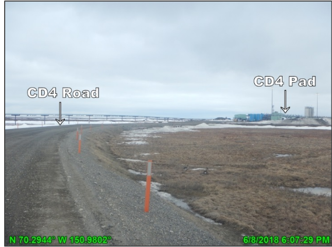
Photo D.2: CD4 road near the CD4 Pad, looking west; June 8, 2018
