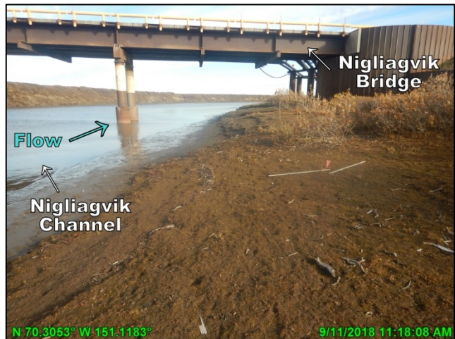
Photo 6.4: East bank of the Nigliagvik Channel at the Nigliagvik Bridge abutment, looking north; September 11, 2018
