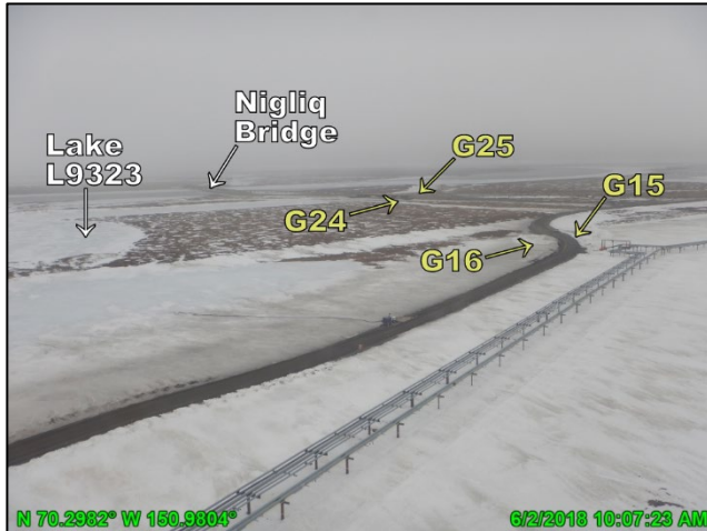
Photo 4.26: North end of CD4 road the day of peak stage at G16, looking north; June 2, 2018
