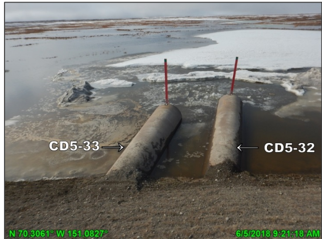
Photo D.4: Culverts along the CD5 road, looking south; June 5, 2018
