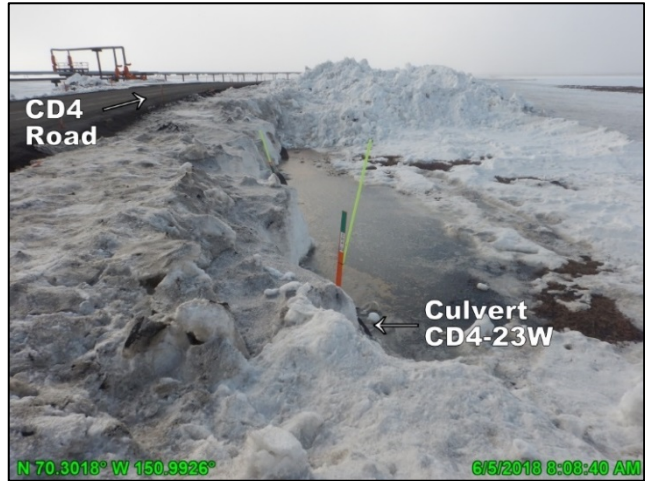
Photo 5.2: West side of CD4 road near CD5 intersection, looking southeast; June 5, 2018
