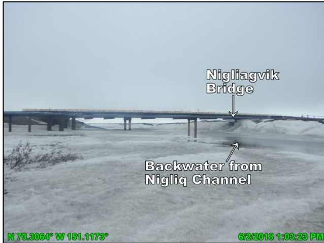
Photo 4.35: Nigliagvik Channel the day prior to peak stage, looking south (upstream); June 2, 2018
