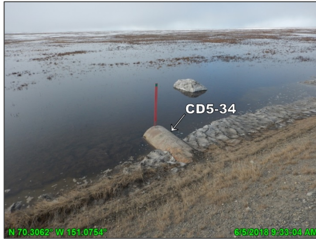
Photo D.5: Culverts along the CD5 road, looking south; June 5, 2018
