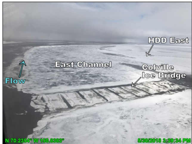
Photo D.7: Colville River East Channel at HDD during breakup, looking north; May 30, 2018
