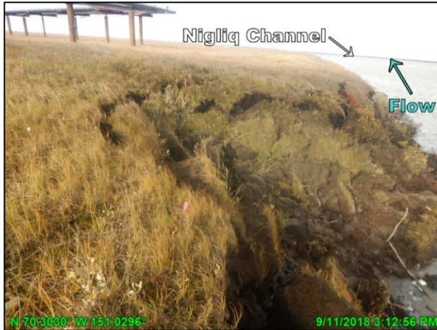
Photo 6.1: West bank of the Nigliq Channel under the Nigliq Bridge, looking north; September 11, 2018
