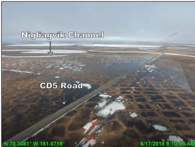
Photo D.3: CD5 road between Lake L9341 and the Nigliagvik Channel, looking southwest; June 17, 2018
