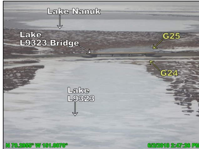
Photo 4.30: CD5 road at gage G24/G25 two days prior to peak stage at G25, looking north; June 2, 2018
