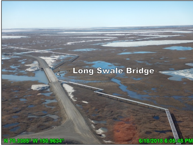
Photo D.1: CD2 road at the Long Swale Bridge post breakup, looking west; June 18, 2018
