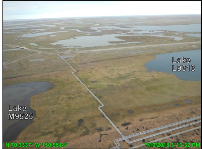
Photo 4.17: Hydraulic connection between Lake M9525 and Lake L9313 looking northwest; July 10, 2018
