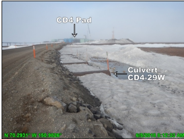
Photo 5.1: North side of CD4 road near CD4 pad, looking west; June 5, 2018
