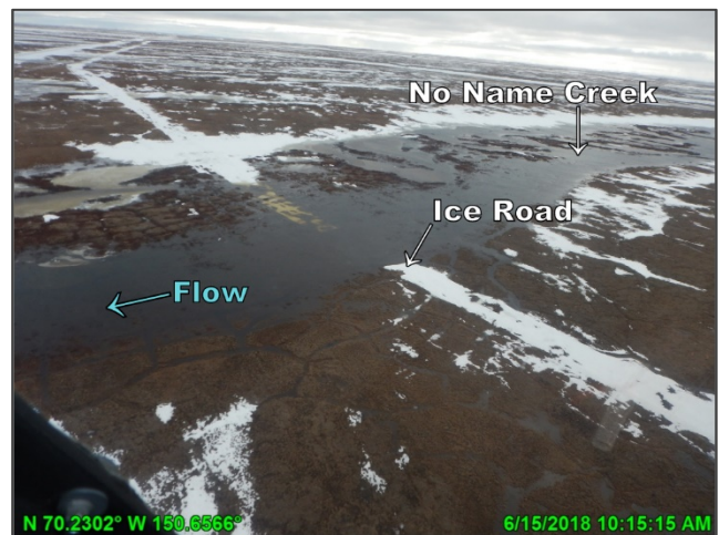
Photo D.19: No Name Creek post-breakup, looking northwest; June 15, 2018
