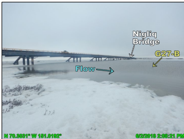
Photo 4.31: Nigliq Bridge, the day before peak stage, looking west; June 2, 2018
