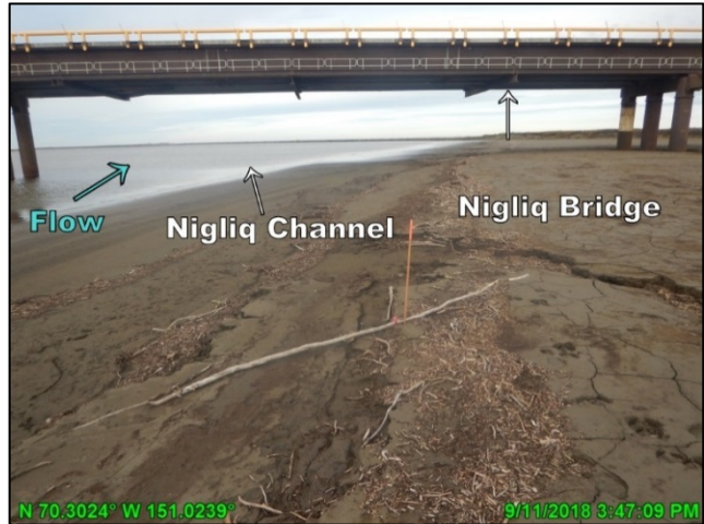
Photo 6.2: East bank of the Nigliq Channel near the Nigliq Bridge, looking north; September 11, 2018
