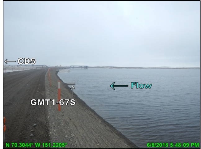
Photo F.2: Culvert GMT1-67 on south side of GMT1 access road, looking east; June 8, 2018
