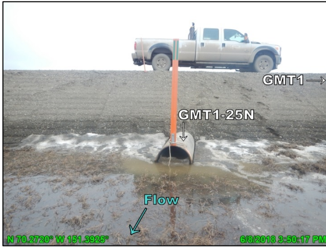
Photo F.14: Culvert GMT1-25 on north side of GMT1 access road blocked, looking south; June 8, 2018
