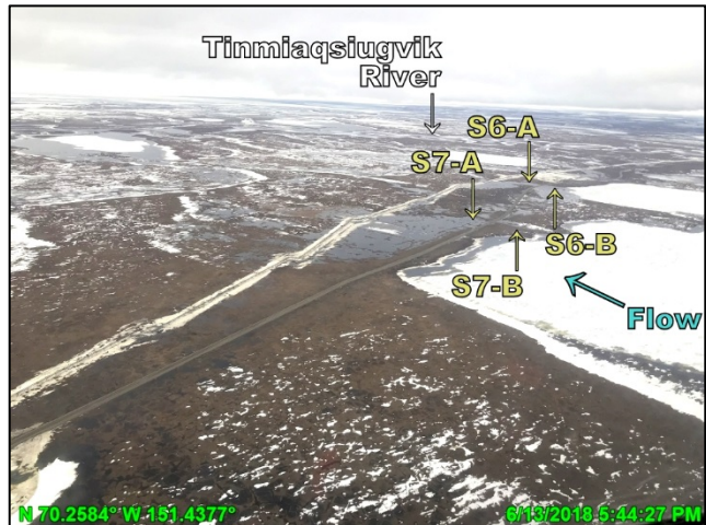
Photo 6: Water equalizing across the GMT1 access road, looking northeast; June 13, 2018
