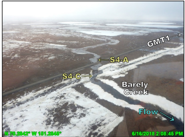
Photo F.11: Drainage at the S4 monitoring location (Barely Creek), looking southwest; June 16, 2018
