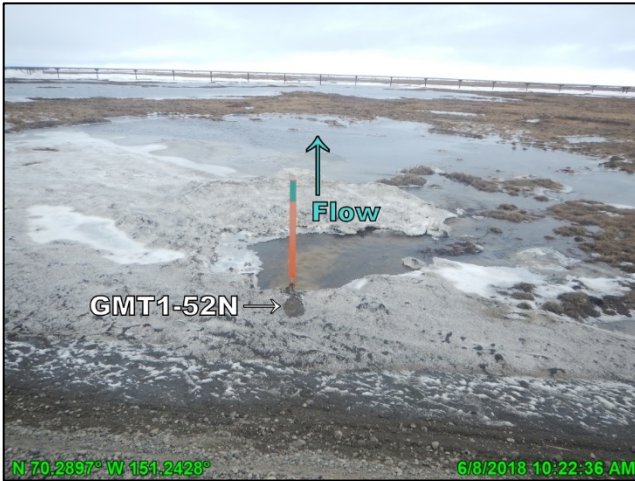
Photo F.4: Culvert GMT1-52 on north side of GMT1 access road, looking west; June 8, 2018
