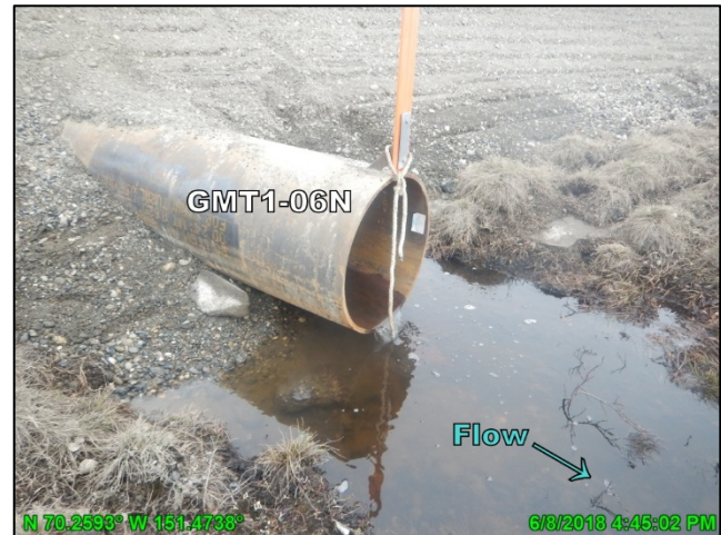
Photo 8: Culvert GMT1-06 perched on the north (DS) side of the GMT1 access road; June 8, 2018
