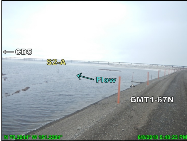
Photo F.1: Culvert GMT1-67 on north side of GMT1 access road, looking east; June 8, 2018
