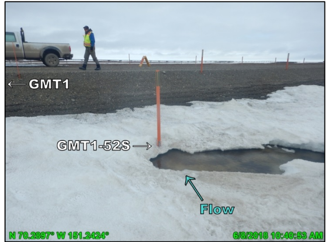
Photo F.5: Culvert GMT1-52 on south side of GMT1 access road, looking west; June 8, 2018
