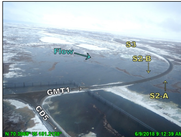
Photo F.3: GMT1 access road at CD5 intersection, looking southwest; June 9, 2018
