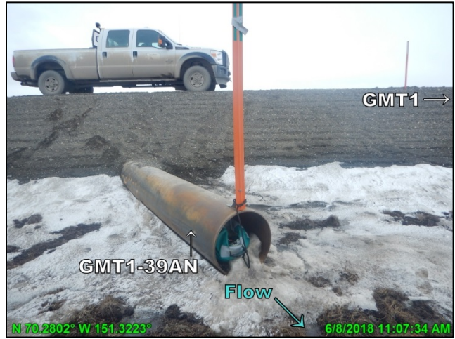
Photo F.9: Culvert GMT1-39A on north side of GMT1 access road with culvert bladder still inside, looking south; June 8, 2018
