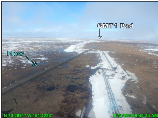
Photo 5: Ponded water on upstream side of GMT1 access road, looking west; June 11, 2018
