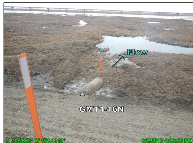
Photo 2: Culvert GMT1-16 on north side of GMT1 access road dry because a culvert bladder blocked flow, looking north; June 8, 2018
