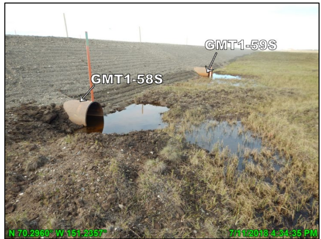
Photo D.20: S3 culverts GMT1-58 through 59, looking north; July 11, 2018
