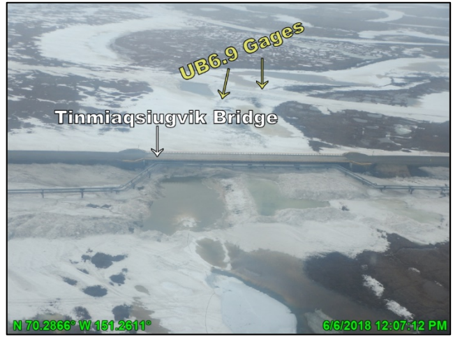
Photo 3.2: Tinmiaqsiugvik Bridge, looking south (upstream); June 6, 2018.
