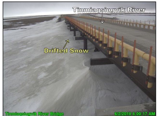
Photo 6.2: Drifted snow remaining under the Tinmiaqsiugvik Bridge, looking west; June 2, 2018
