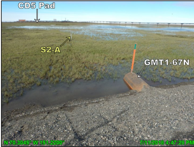
Photo D.17: S2 gages and culverts, looking north; July 11, 2018
