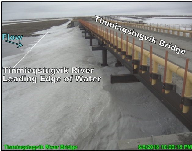
Photo 4.1: Tinmiaqsiugvik Bridge, looking west June 8, 2018
