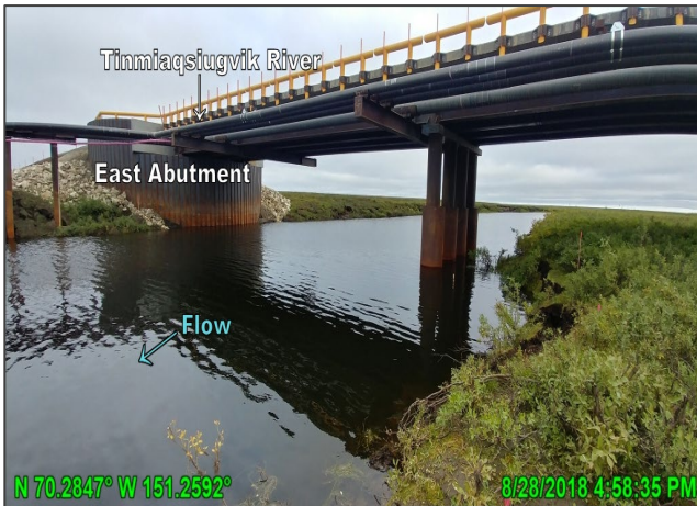
Photo D.12: Tinmiaqsiugvik Bridge, looking southeast (upstream); August 28, 2018
