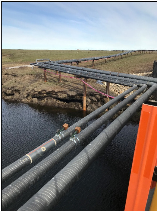
Photo 7.1: Erosion along east bank of Tinmiaqsiugvik River, looking northeast; July 2018
