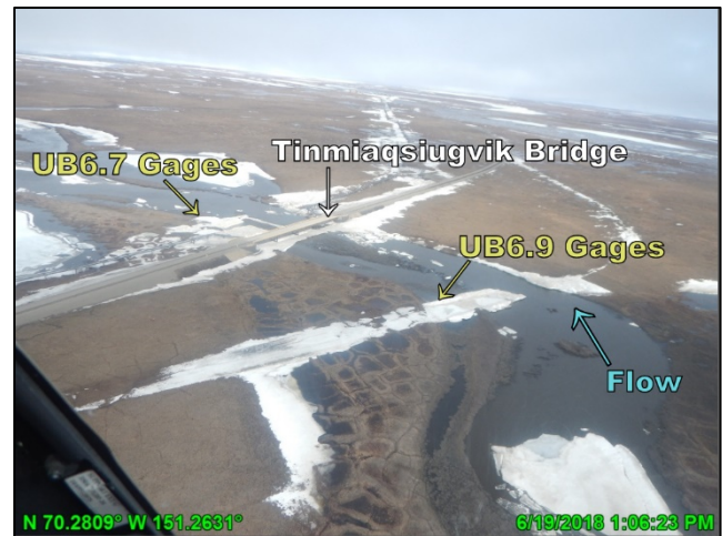
Photo 4.4: Tinmiaqsiugvik Bridge, looking northeast; June 19, 2018
