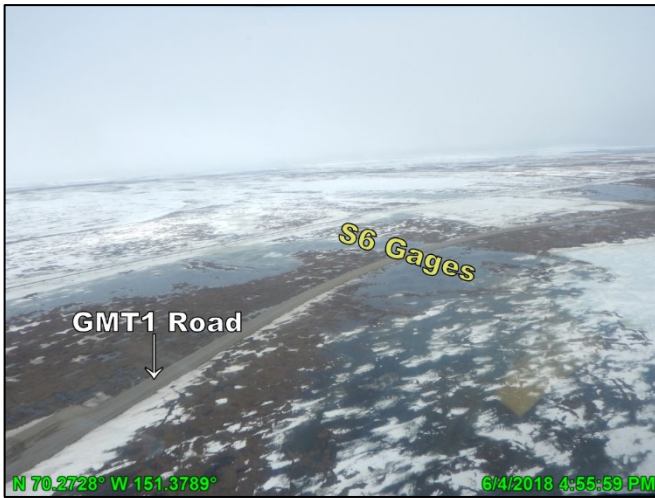
Photo 4.25: S6, looking south; June 4, 2018
