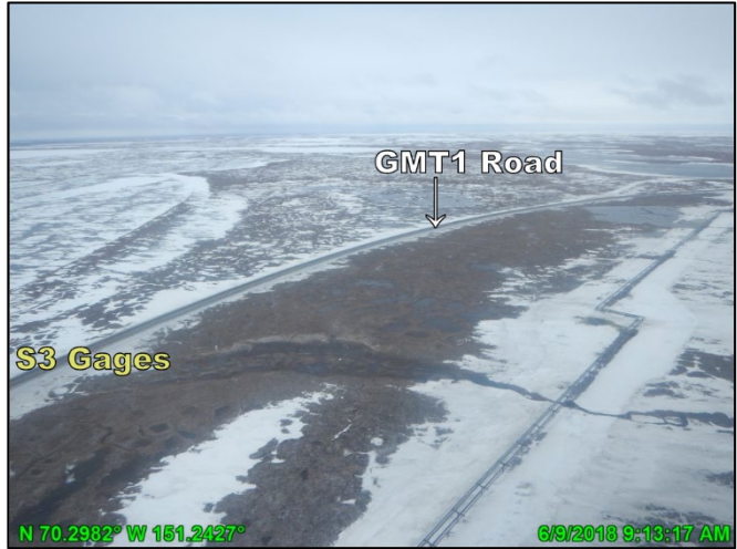
Photo 4.24: S3, looking south; June 9, 2018
