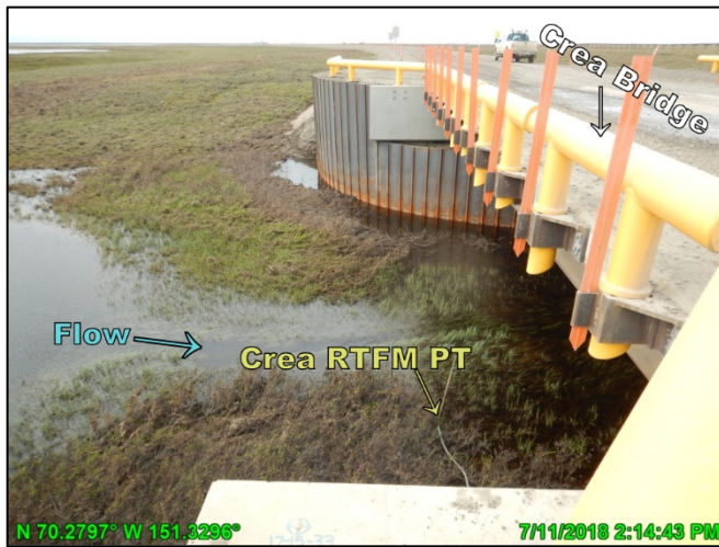
Photo 4.11: Crea Bridge, looking west; July 11, 2018
