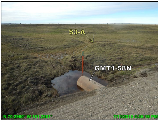
Photo D.19: S3 gages and culverts, looking north; July 11, 2018
