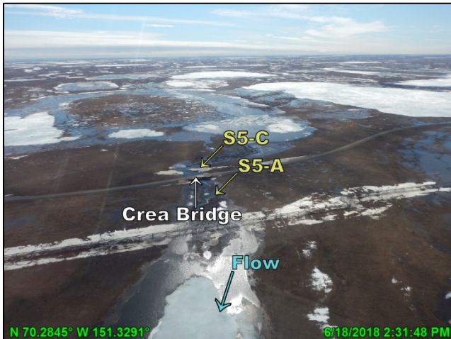
Photo 4.9: Crea Bridge, looking south; June 18, 2018
