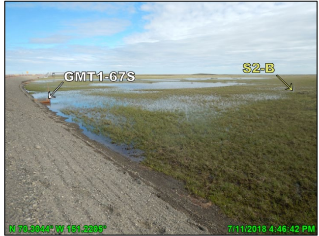
Photo D.18: S2 gages and culverts, looking east; July 11, 2018
