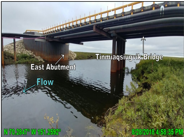
Photo 4.5: Tinmiaqsiugvik Bridge, looking southeast; August 28, 2018
