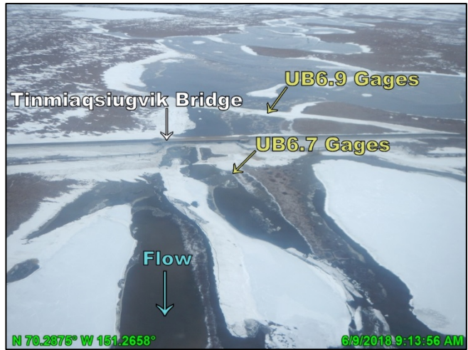
Photo 4.2: Backwater upstream of the Tinmiaqsiugvik Bridge, looking south; June 9, 2018
