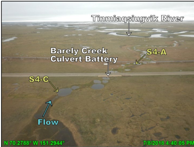
Photo D.1: Barely Creek culvert battery, looking north (downstream); July 8, 2018
