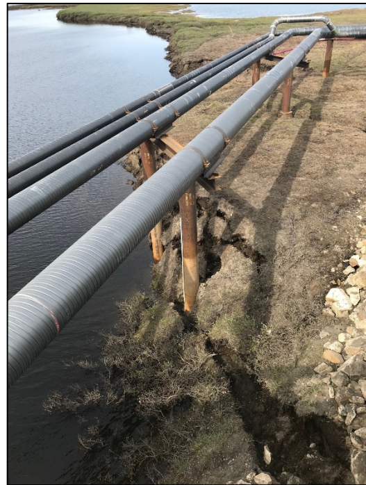
Photo 7.2: Pipeline VSM in channel, east bank Tinmiaqsiugvik Bridge, looking north (downstream); July 2018
