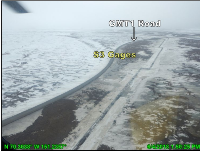
Photo 4.23: S3, looking south; June 4, 2018
