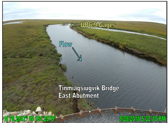
Photo 4.6: Tinmiaqsiugvik Bridge, looking south; August 28, 2018
