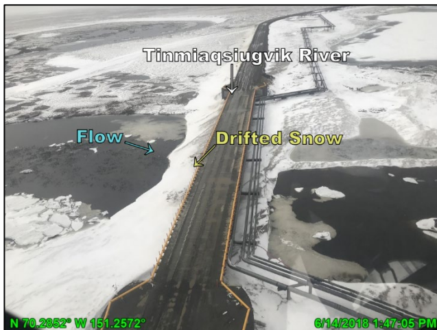
Photo 6.1: Drifted snow remaining intact and flow concentrated along the east abutment at the Tinmiaqsiugvik Bridge, looking west; June 14, 2018
