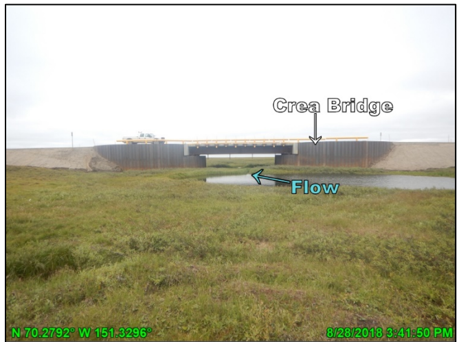
Photo 4.12: Crea Bridge, looking north (downstream); August 28, 2018
