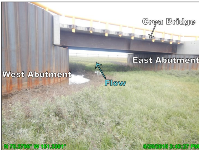
Photo D.7: Crea Bridge, looking northeast (downstream); August 28, 2018
