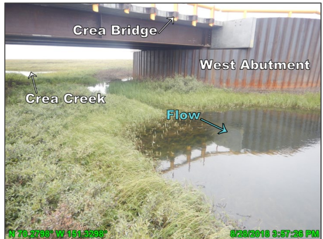
Photo D.8: Flow under Crea Bridge, looking south (upstream); August 28, 2018
