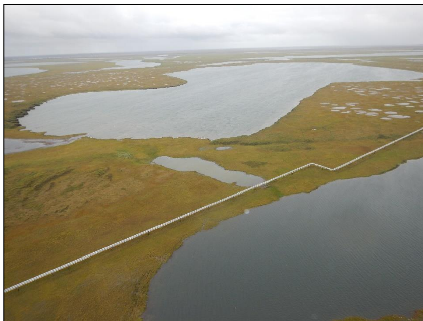
Photo 7: Lake L9327, looking southwest past the Alpine Sales pipeline; August 14, 2019
