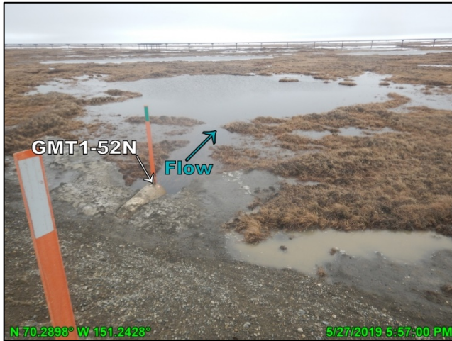
Photo F.4: Culvert GMT1-52, looking north; May 27, 2019
