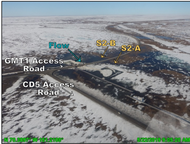
Photo F.1: Local meltwater around S2, looking southwest; May 22, 2019
