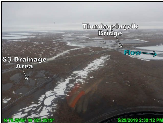
Photo F.6: S3 drainage area, looking south; May 29, 2019
