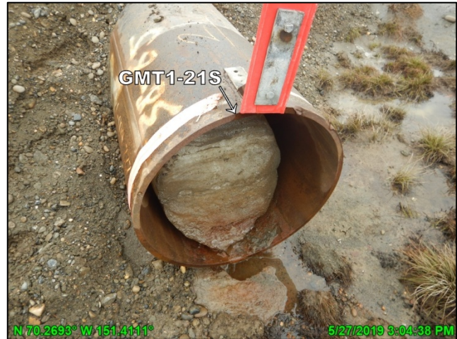
Photo 3.5: Culvert GMT1-21 with ice blockage, looking north; May 27, 2019
