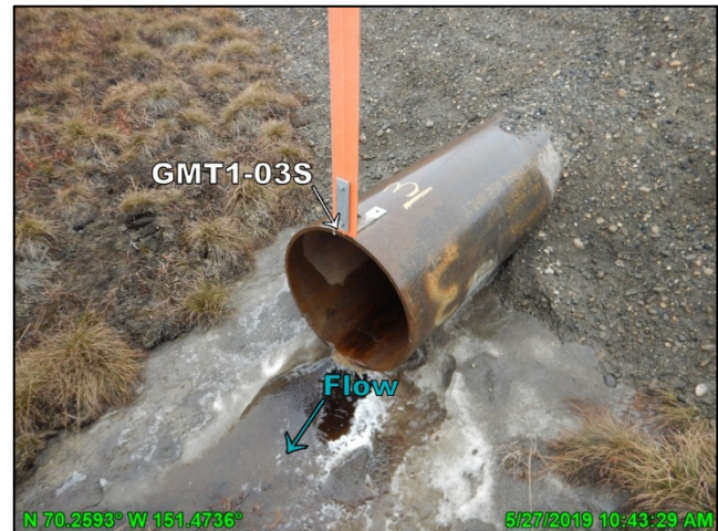
Photo 3.9: Perched culvert GMT1-03 with minimal flow, looking north; May 27, 2019
