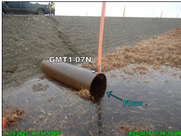
Photo 3.8: Water flowing freely through culvert GMT1-07, looking north; May 27, 2019
