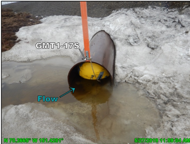
Photo 3.4: Culvert GMT1-17 with culvert bladder blockage, looking north; May 27, 2019
