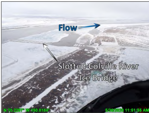
Photo D.27: Meltwater progression through the slotted Colville River Ice Bridge, looking north (downstream); May 26, 2020
