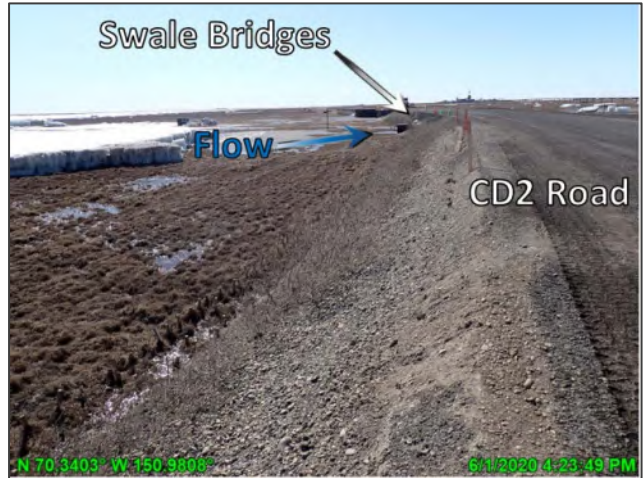
Photo D.2: CD2 road between long swale and short swale bridges, looking northeast; June 1, 2020
