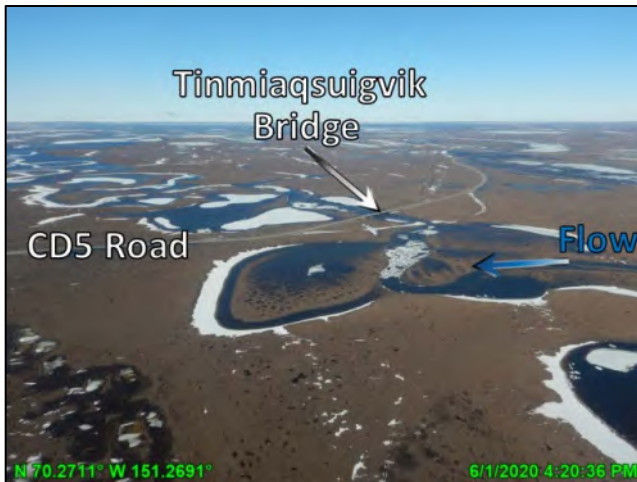
Photo 4-69: Ice jam upstream of Tinmiaqsuigvik Bridge in place after peak stage, looking north (downstream); June 1, 2020
