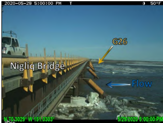
Photo 4-47: Peak stage at the Nigliq Bridge, looking east; May 29 2020
