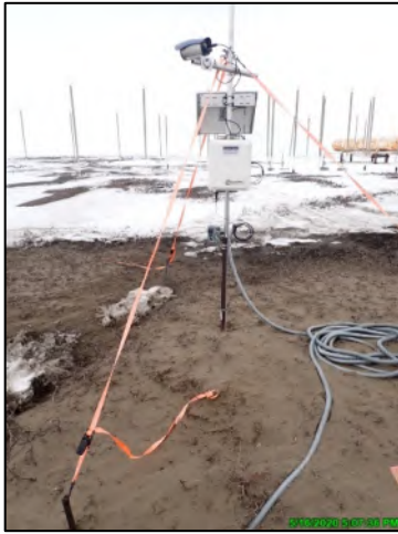
Photo 2-11: Remote camera setup at HDD West bank; May 16, 2020
