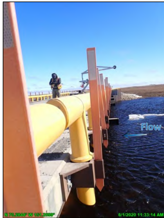
Photo 4-70: Tinmiaqsuigvik Bridge during discharge measurement looking east; June 1, 2020
