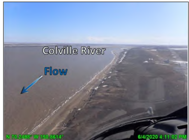
Photo D.28: Open channel at Colville River Ice Bridge, looking south (upstream); June 4, 2020
