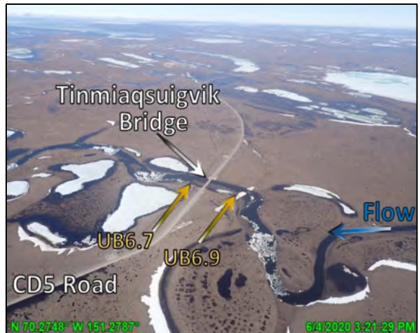
Photo 4-68 Ice jam still in place upstream from the bridge crossing, looking northeast (downstream); June 4, 2020
