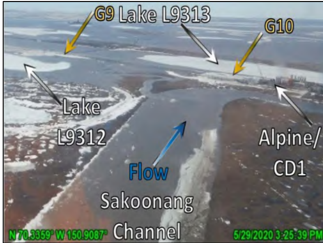
Photo 4-23: Overland recharge of both Lakes L9312 and L9313 near peak stage, looking east; May 29 2020
