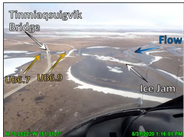
Photo 4-66: Ice jam upstream of the Tinmiaqsiugvik Bridge, looking southeast (upstream); May 31, 2020
