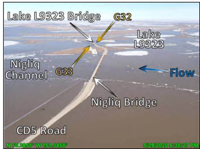
Photo 4-42: Lake L9323 bridge near peak stage, looking east; May 29, 2020
