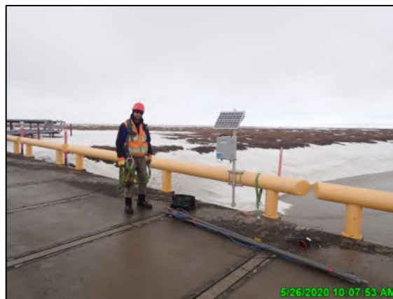
Photo 2-10: Installation of real-time pier scour equipment on the Nigliagvik Bridge; May 26, 2020
