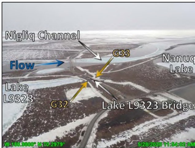
Photo 4-41: Lake L9323 bridge and vicinity prior to peak stage, looking west; May 28, 2020
