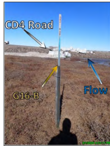
Photo D.16: CD4 road with stranded ice in vicinity of north CD4 culvert battery post-breakup, looking north; June 1, 2020
