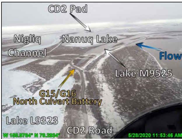
Photo 4-35: Floodwater in Lake M9525 reaching CD4 road north culvert battery, looking north; May 28, 2020
