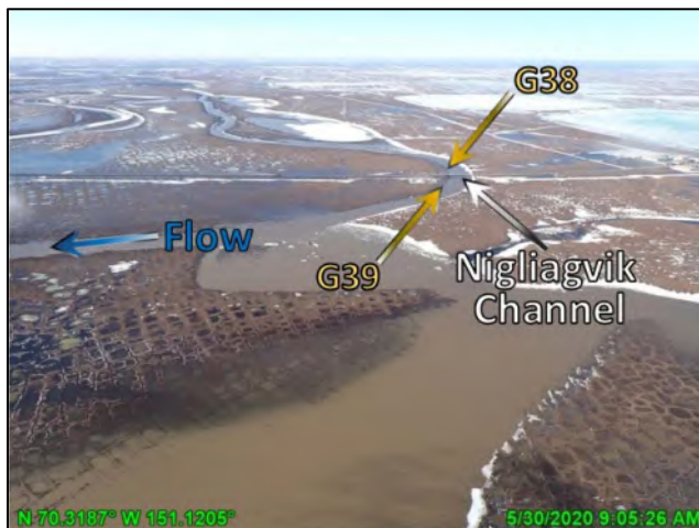
Photo 4-61: Conditions at the Nigliagvik Bridge one day after peak stage, looking southwest (upstream); May 30, 2020
