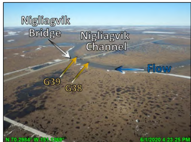
Photo 4-62: Stage below bankfull in the Nigliagvik Channel, looking northeast (downstream); June 1, 2020
