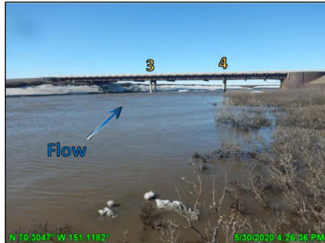
Photo 6-2: Pier numbers on the Nigliagvik Bridge, looking north; May 30, 2020
