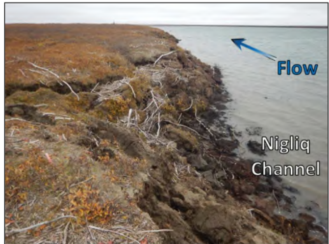
Photo D.24: East bank of Nigliq channel north of CD5 road during fall setup, looking north; September 7, 2020
