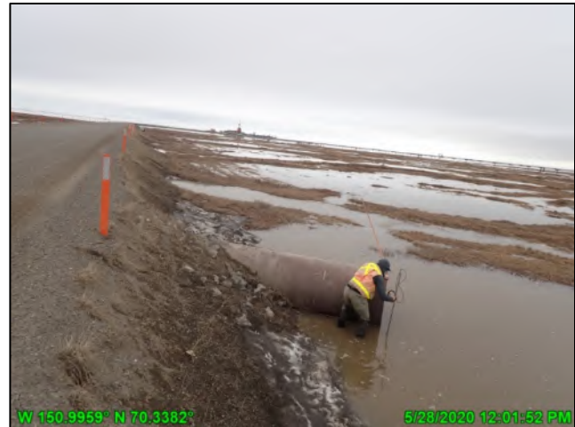
Photo 2-9: Measuring discharge at a culvert along the CD2 road; May 28, 2020
