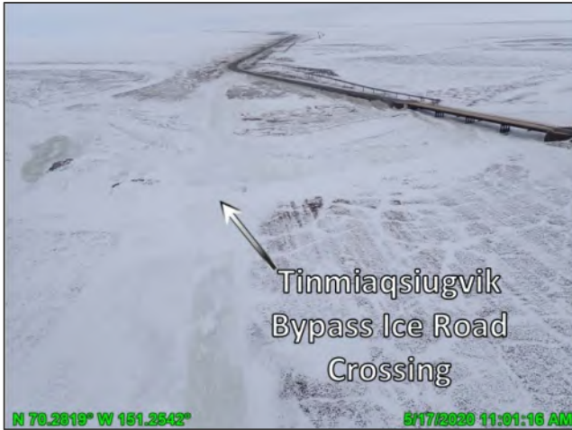
Photo D.55: Pre-breakup conditions at the slotted Tinmiaqsiugvik Bypass ice road crossing, looking northwest; May 17, 2020
