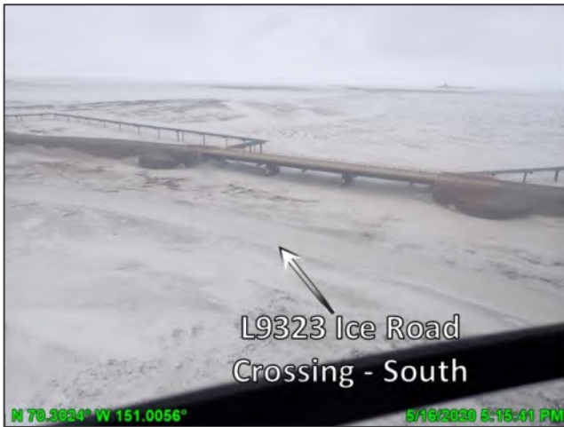
Photo D.31: Pre-breakup near the L9323 ice road crossing-south, looking northwest, May 16, 2020
