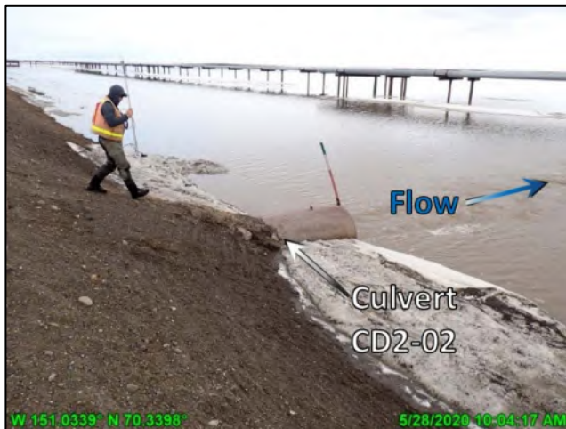
Photo 4-30: Crew measuring discharge through culvert CD2-02, looking northwest; May 28, 2020
