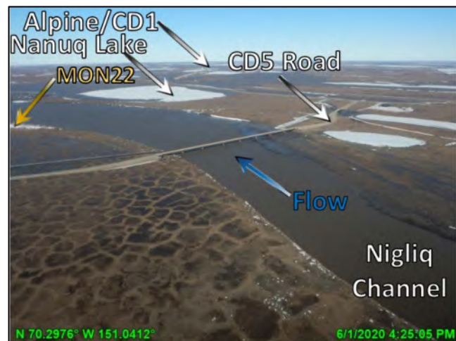
Photo 4-20: Receding stage in Nigliq Channel, looking north (downstream); June 1, 2020
