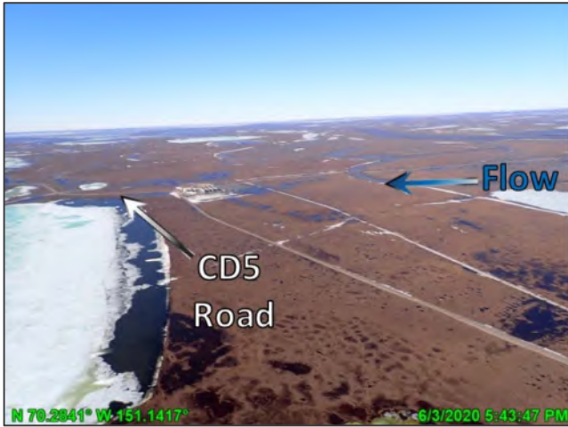
Photo D.17: CD5 road in the vicinity of K-Pad as breakup subsides, looking south; June 3, 2020
