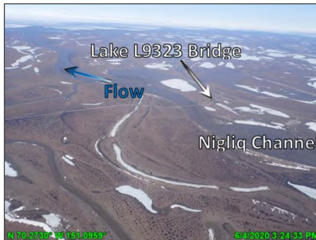
Photo D.33: Post-breakup conditions at Nigliq and Lake L9323 ice road crossings; June 4, 2020
