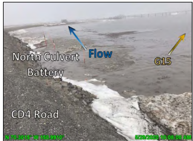
Photo 4-36: Turbulent flow through north culvert battery at G15/G16 near peak stage, looking north (downstream); May 29, 2020
