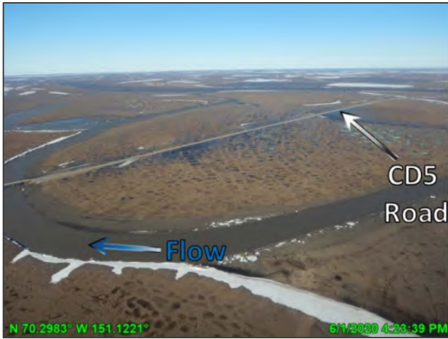
Photo D.21: CD5 road near Nigliagvik Bridge post-breakup, looking north; June 1, 2020
