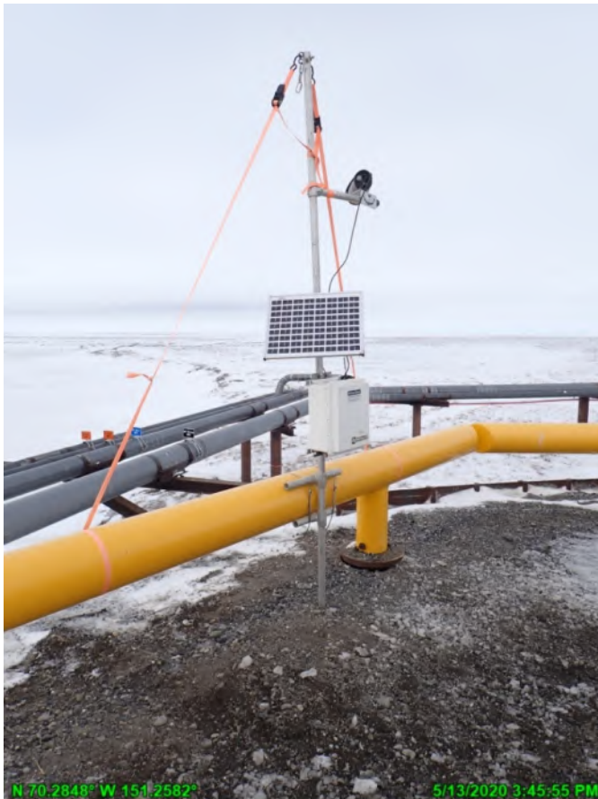
Photo 2-14: Installation of telemetry and solar/battery RTFM equipment at the Tinmiaqsiugvik Bridge; May 13, 2020
