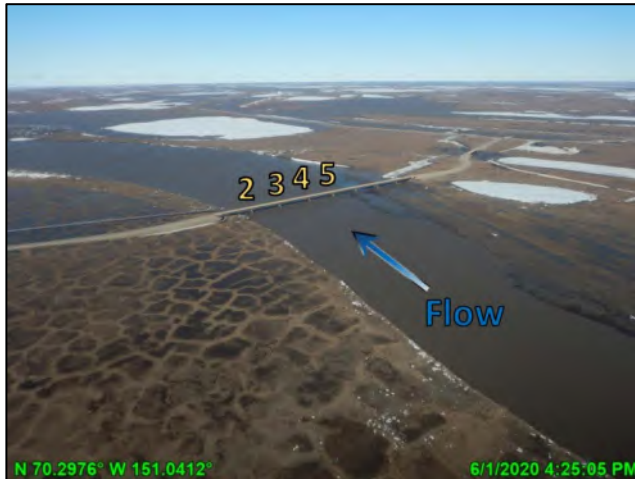
Photo 6-1: Pier numbers on the Nigliq Bridge, looking northeast; June 1, 2020
