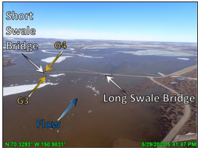
Photo 4-29: Floodwater passing through the swale bridges near peak stage; looking north (downstream) May 29, 2020
