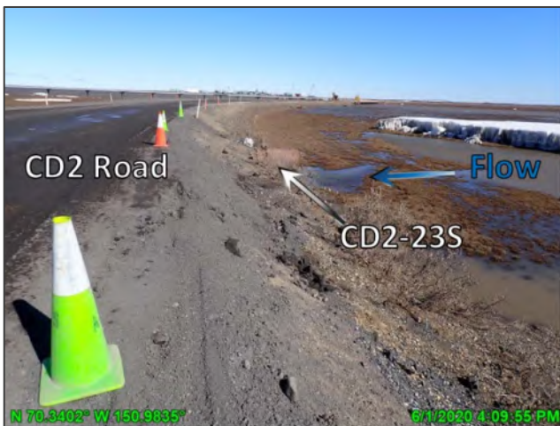
Photo D.3: CD2 road between long swale and short swale bridges, looking southeast; June 1, 2020
