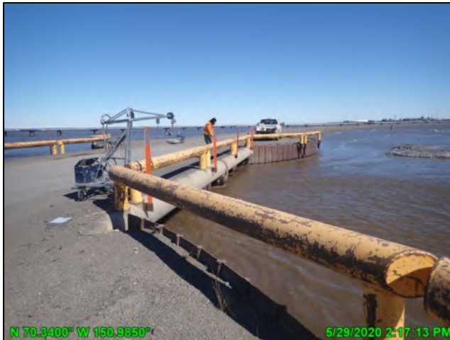
Photo 2-8: Measuring discharge at the CD2 Road Short Swale Bridge; May 29, 2020
