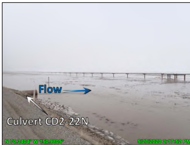
Photo 4-26: Floodwater along the CD2 road, looking northwest; May 27, 2020
