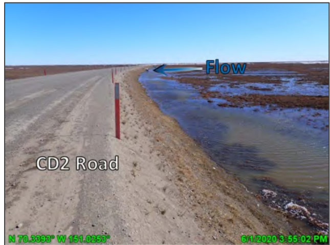
Photo D.8: Road in vicinity of culvert CD2-8S post-breakup, looking southwest; June 1, 2020
