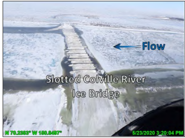
Photo D.26: Initial flow through the slotted Colville River Ice Bridge, looking east; May 23, 2020
