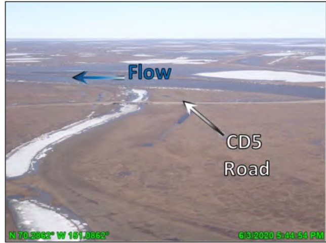
Photo D.18: CD5 road Lake L9341 Bridge as breakup subsides, looking North; June 3, 2020
