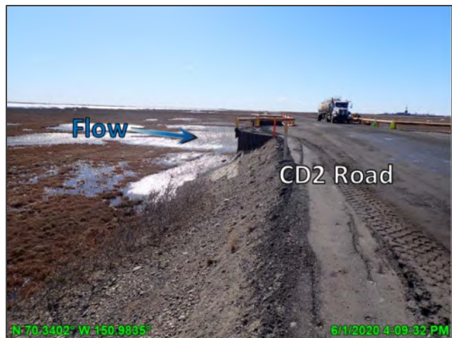
Photo D.4: CD2 road short swale bridge SW abutment, looking east; June 1, 2020
