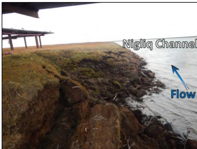
Photo 6-5: West bank of the Nigliq Channel near the Nigliq Bridge, looking north; September 7, 2020
