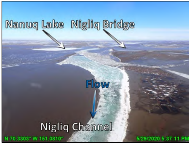
Photo 4-49: Widespread floodwater inundation downstream of Nigliq Bridge crossing, looking south (upstream); May 29, 2020
