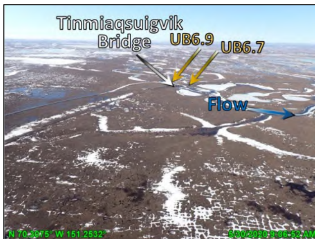
Photo 4-65: Tinmiaqsiugvik Bridge prior to peak stage, looking south (upstream); May 30, 2020
