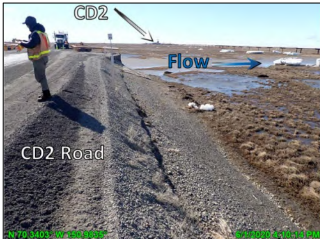
Photo 5-3: CD2 road near Short Swale Bridge post-breakup, looking west; June 1, 2020
