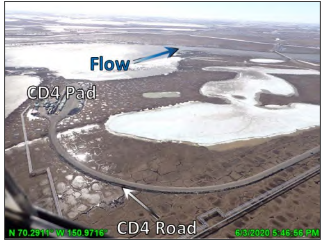
Photo D.14: CD4 road in vicinity of G18 culverts post-breakup, looking northeast; June 3, 2020
