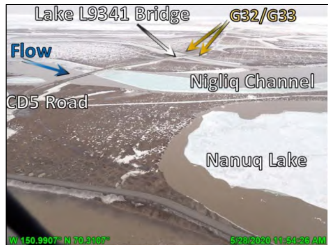
Photo 4-54: Lake L9341 hydraulically connected to Nigliq Channel on north end, looking southwest; May 28, 2020
