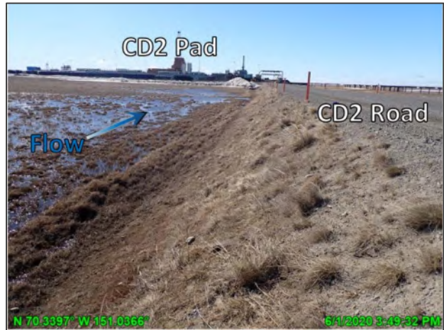
Photo D.12: Road in vicinity of culvert CD2-1S post-breakup, looking east; June 1, 2020
