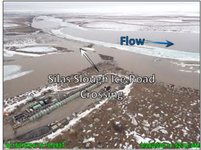
Photo D.43: Peak stage near the slotted Silas Slough ice road crossing, looking southwest; May 28, 2020
