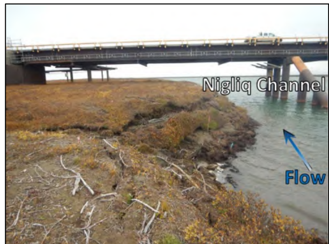
Photo 6-6: West bank of the Nigliq Channel south of the Nigliq Bridge, looking north; September 7, 2020
