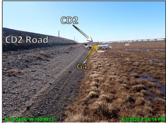
Photo 5-2: CD2 road post-breakup, looking northwest; June 1, 2020
