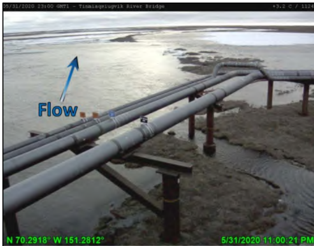
Photo 4-67: RTFM photo from directly downstream of Tinmiaqsuigvik Bridge at peak stage, looking north (downstream); May 31, 2020
