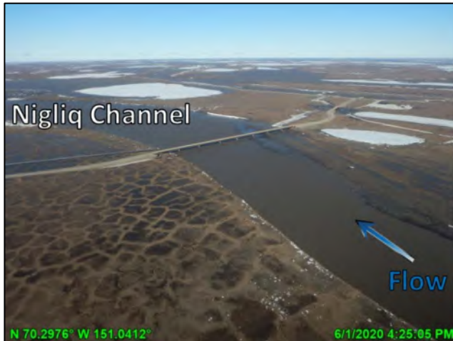
Photo 6-3: Nigliq channel post breakup showing no channel migration, looking northeast; June 1, 2020
