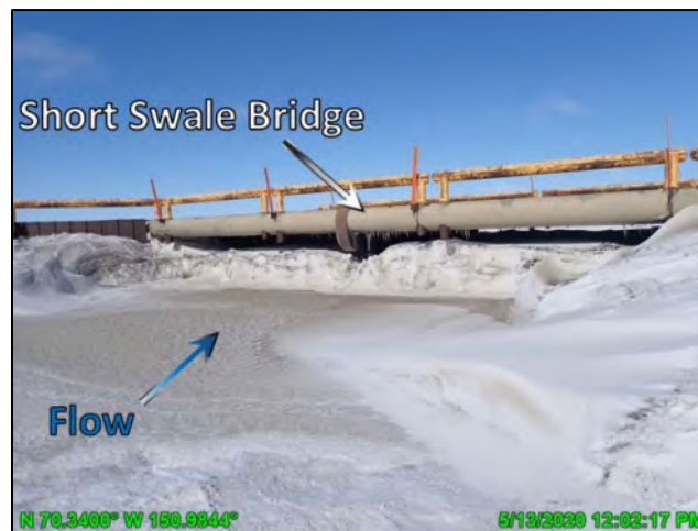
Photo 4-21: Snow cleared from the south side of the short swale bridge. Note drifted snow still present directly underneath bridge deck
