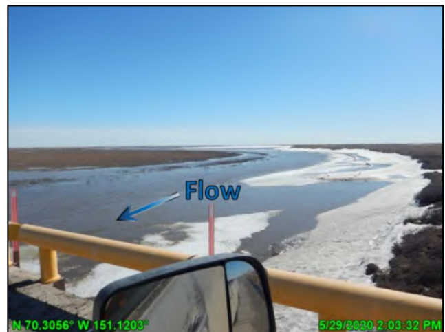
Photo 4-60: Nigliagvik Bridge near peak stage, looking southeast; May 29, 2020
