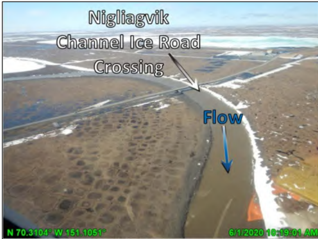
Photo D.36: Post-breakup conditions at the Nigliagvik ice road crossing, looking southwest (upstream); June 1, 2020
