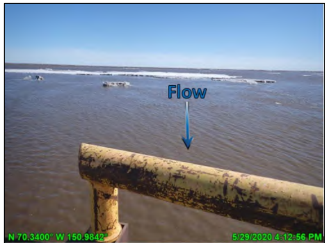
Photo 4-31: Ice present south of Short Swale Bridge during discharge measurement, looking south (upstream); May 29, 2020
