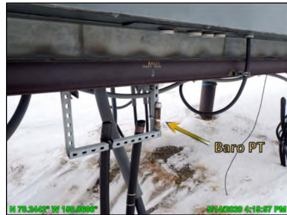
Photo 2-7: Baro at MON9/East Channel HDD; May 14, 2020
