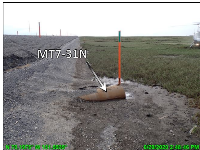
Photo F.18: Sloughed gravel near culvert MT7-31 and S12, looking west; July 2, 2020
