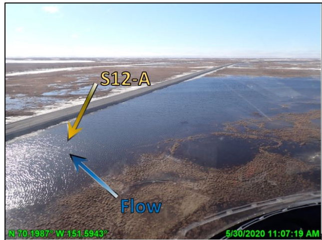
Photo F.16: Ponded water on the upstream side of the road near S12, looking southwest; May 30, 2020
