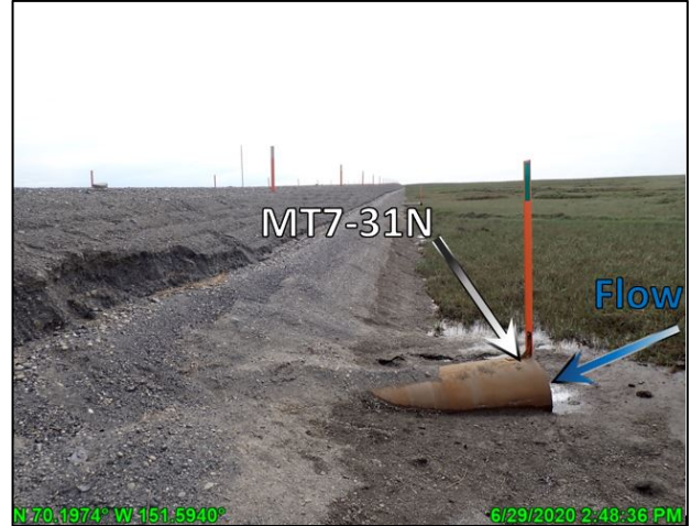
Photo 3.7: Sloughing along the north embankment near MT7-31, looking west; June 29, 2020
