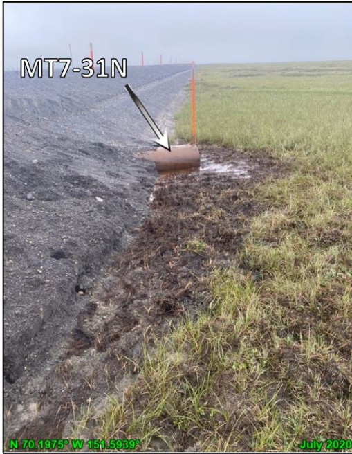
Photo F.19: Culvert MT7-31 after sloughed gravel replaced on embankment; July, 2020
