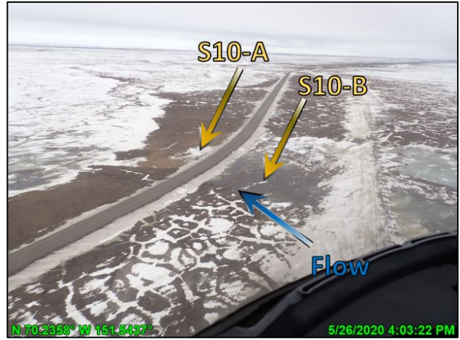
Photo F.6: Increasing meltwater on the upstream (south) side of road, looking northeast; May 26, 2020
