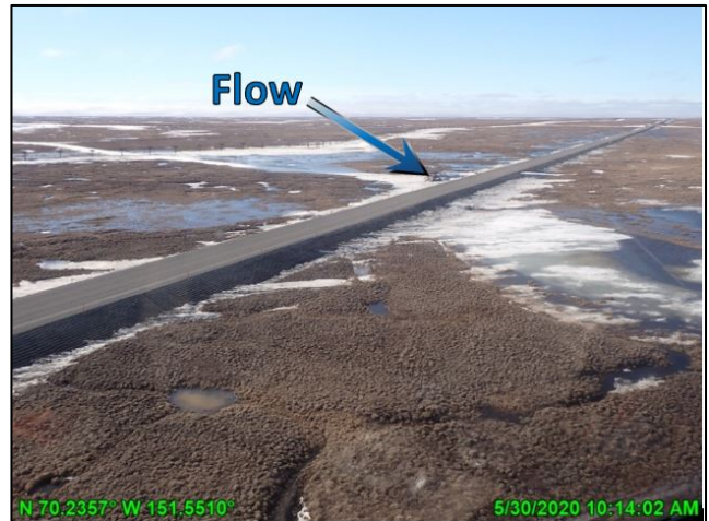
Photo 3.5: Drifted snow along GMT2/MT7 road embankments, looking southwest; May 30, 2020
