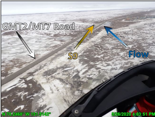
Photo F.1: Meltwater accumulation near S9, looking northeast; May 26, 2020
