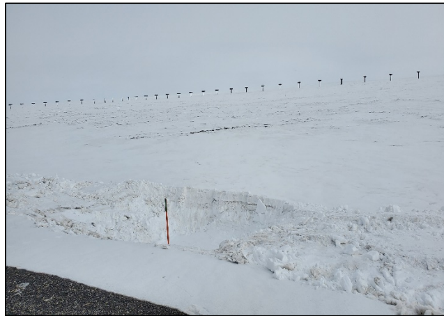
Photo 3.1: Snow cleared from a culvert on the GMT2/MT7 road, looking south; early May, 2020
