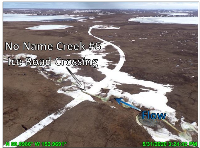
Photo D.23: Breakup conditions at the No Name Creek #6 ice road crossing, looking east; May 31, 2020
