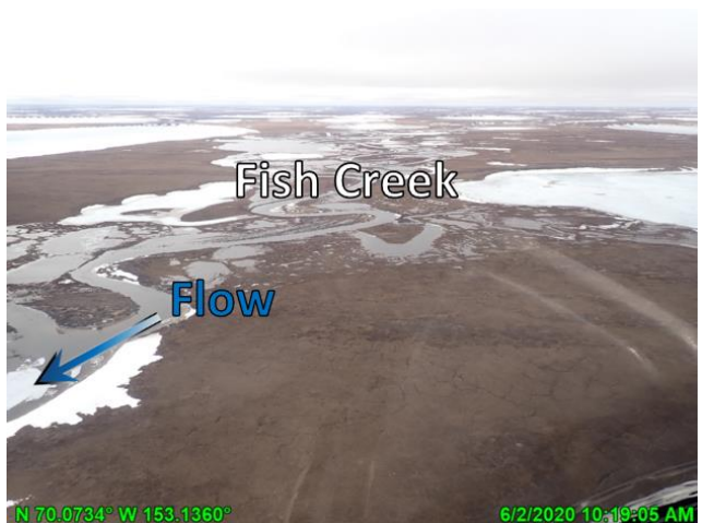
Photo 4.6: Minor overbank flooding near the headwaters of Fish Creek, looking west (upstream); June 2, 2020
