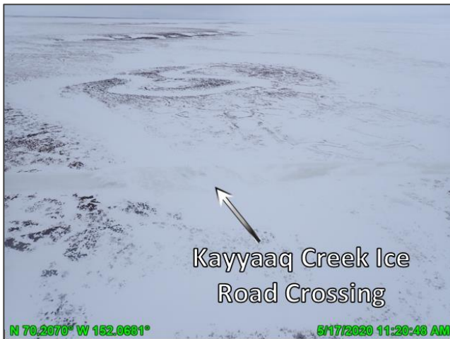
Photo D.7: Pre-breakup conditions at the slotted Kayyaaq Creek ice road crossing, looking southwest; May 17, 2020
