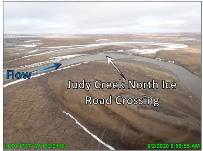
Photo D.2: Post-breakup conditions at the Judy Creek North ice road crossing, looking west; June 2, 2020
