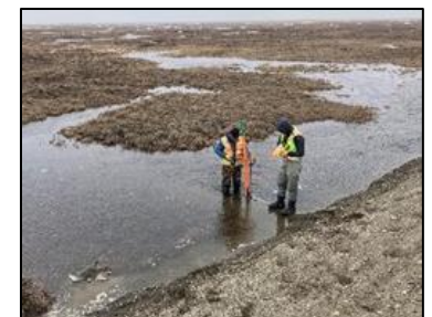
Measuring flow at culvert along the GMT2/MT7 road.
