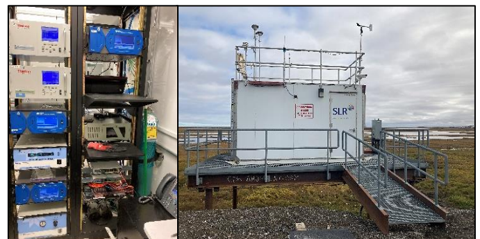
Interior and exterior photographs of CD5 Air Monitoring Station.
