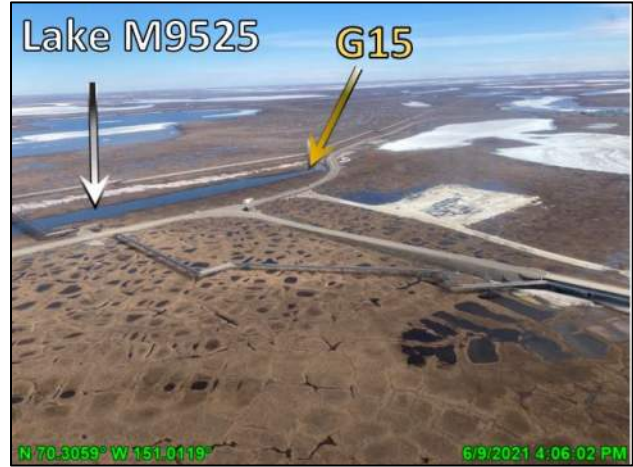
Photo 4.41: CD4 and CD5 intersection near G15/G16 culvert battery after peak stage, looking southeast; June 9, 2021
