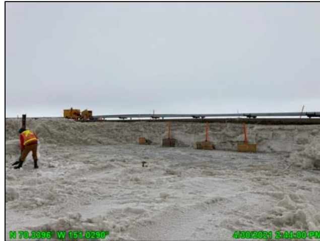
Photo 4.25: Snow cleared from the south side of the culvert battery between G6 & G7.
