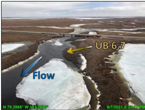
Photo 4.66: Tinmiaqsiugvik Bridge with persisting snow approximately 11 days after peak, looking south (upstream); June 7, 2021
