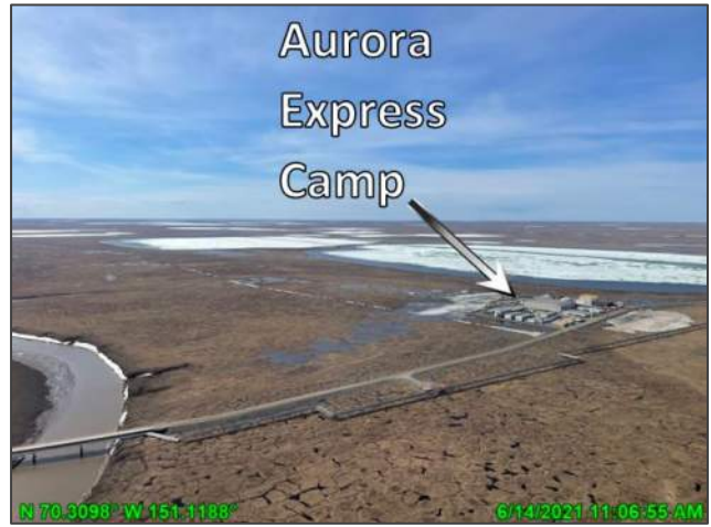
Photo D.22: CD5 road west of the Nigliagvik bridge, looking southwest; June 14, 2021
