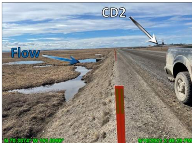
Photo D.3: CD2 road embankment in the vicinity of culvert CD2-16, looking northwest; June 10, 2021
