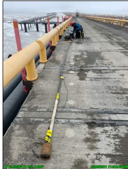
Photo 2.13: Pier scour sonar equipment on the Nigliagvik; May 20, 2021
