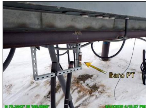
Photo 2.7: Baro at MON9/East Channel HDD
