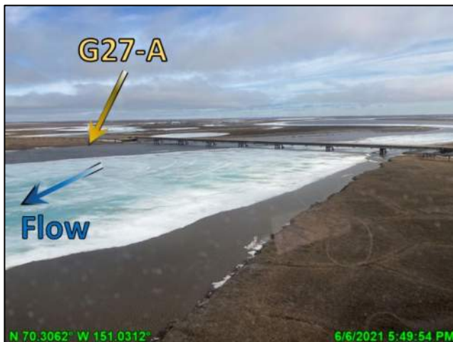
Photo 4.48: Rising stage with channel ice persisting at the Nigliq bridge, looking southeast (upstream); June 6, 2021
