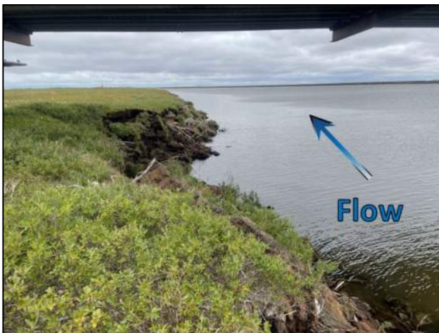
Photo 6.5: West bank of the Nigliq Channel near the Nigliq Bridge, looking north; August 12, 2021
