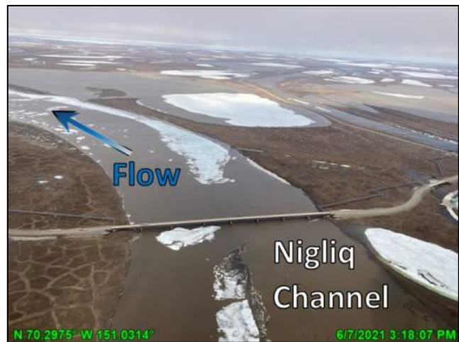
Photo 3.10: CD5 Bridge across the Nigliq Channel near peak conditions showing no floodplain inundation or overbank flooding, looking north (downstream); June 7, 2021
