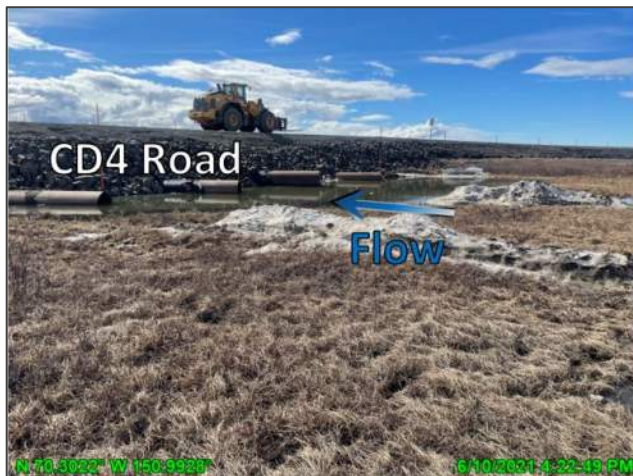
Photo D.15: CD4 road in vicinity of G15 culverts post-breakup, looking west; June 10, 2021
