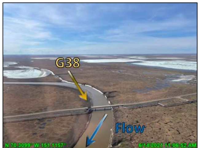
Photo 4.59: Stage below bankfull in the Nigliagvik Channel, looking south (upstream); June 14, 2021
