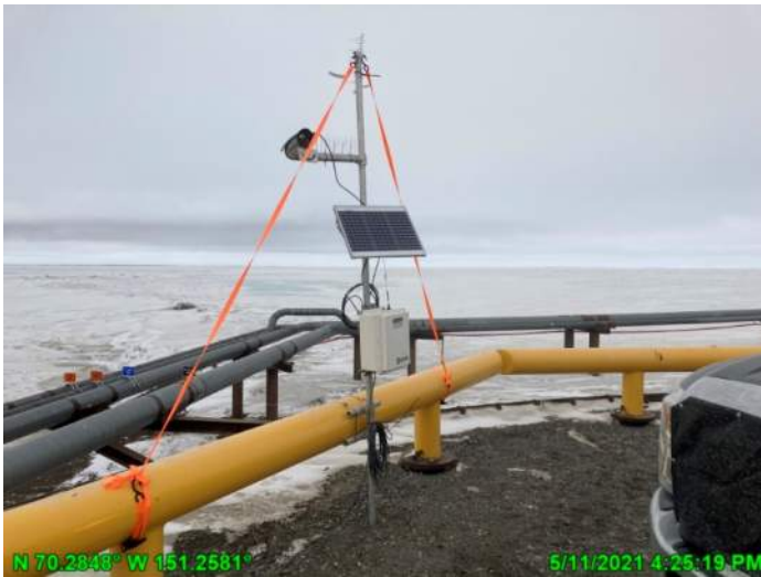
Photo 2.14: Installation of telemetry and solar/battery RTFM equipment at the Tinmiaqsiugvik Bridge; May 11, 2021
