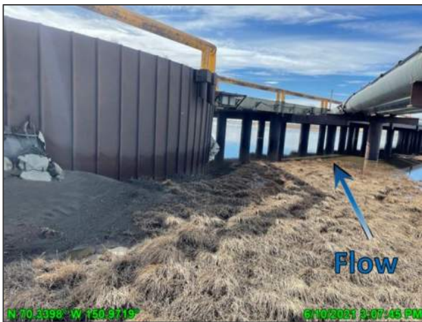
Photo D.11: CD2 long swale SW abutment, looking north; June 10, 2021
