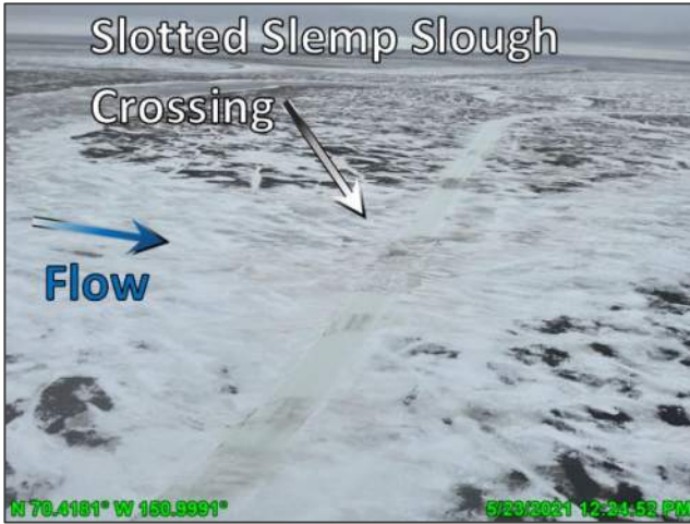
Photo D.37: Pre-breakup conditions at the slotted Slemph Slough ice road crossing, looking south; May 23, 2021
