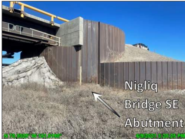
Photo D.19: Nigliq SE abutment post-breakup, looking northeast; June 9, 2021
