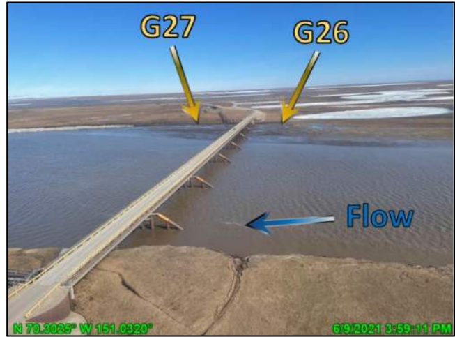
Photo 4.51: Open water conditions at the Nigliq bridge with receding stage, looking east; June 9, 2021
