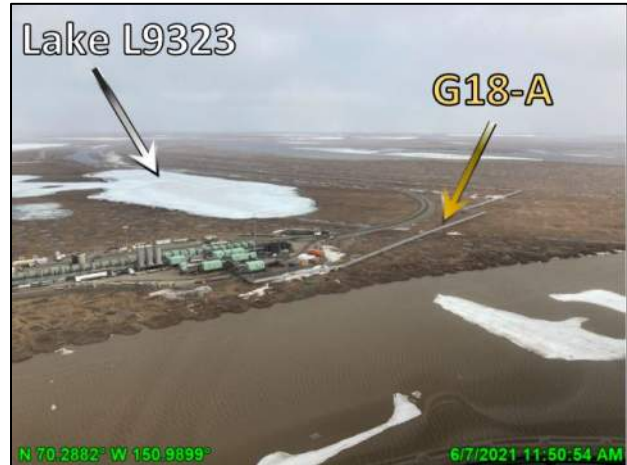
Photo 4.37: Conditions at CD4 pad near peak stage, looking north; June 7, 2021
