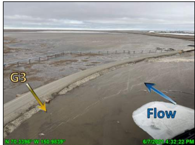
Photo 4.30: Floodwater passing through culverts near peak stage; looking northeast (downstream) June 7, 2021
