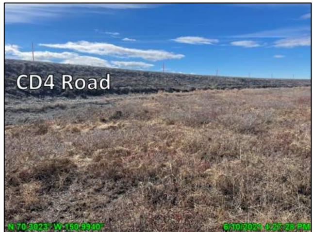
Photo 5.4: CD4 road post breakup near Gage G16, looking northwest; June 10, 2021
