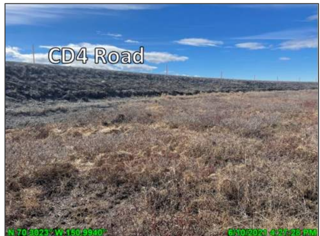
Photo D.16: CD4 road embankment in the vicinity of G15 post-breakup, looking north; June 10, 2021
