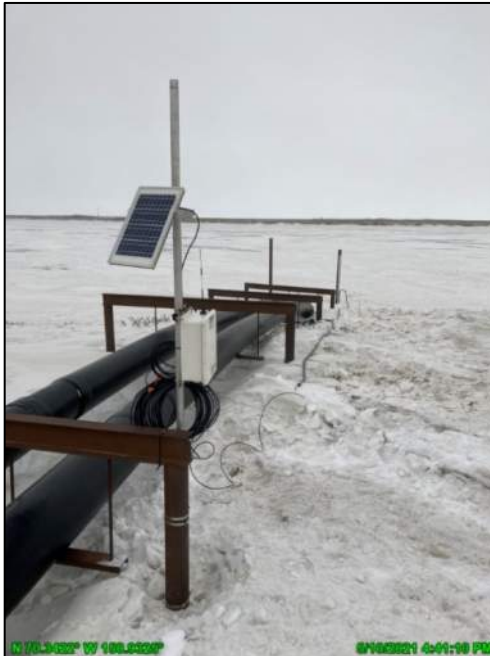
Photo 2.12: Remote stage monitoring equipment at Lake L9313 (G10); May 10, 2021
