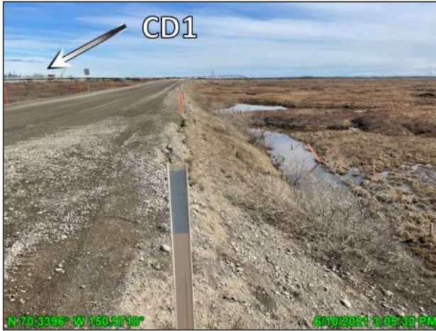
Photo D.9: CD2 road embankment in the vicinity of the long swale bridge, looking south east; June 10, 2021
