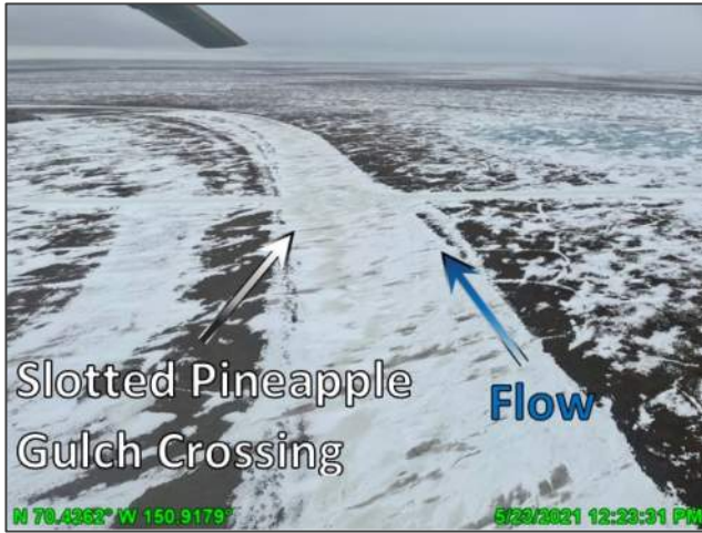
Photo D.41: Pre-breakup conditions at the slotted Pineapple Gulch (West Ulamniaq Channel) ice road crossing, looking north (downstream); May 23, 2021
