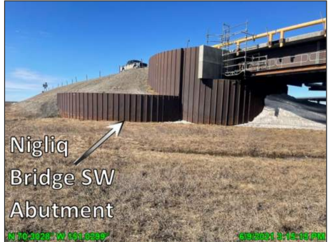
Photo D.18: Nigliq SW abutment post-breakup, looking north; June 9, 2021
