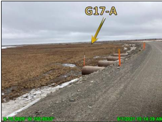
Photo 4.36: Local melt at CD4 road south culvert battery near G17/G18, looking northeast; June 1, 2021
