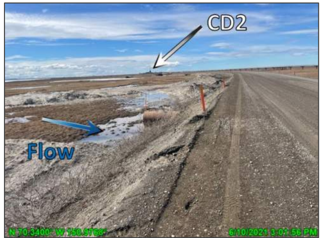
Photo D.8: Road in vicinity of culvert CD2-23 post-breakup, looking northwest, 2021
