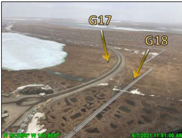
Photo 4.38: Conditions prior to peak on CD4 road near Gage G17/G18, looking northeast; June 7, 2021
