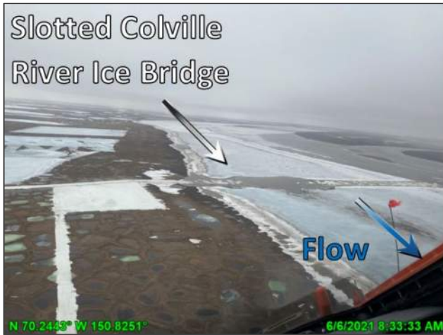
Photo D.27: Meltwater progression through the slotted Colville River Ice Bridge, looking south (upstream); June 6, 2021
