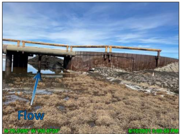
Photo D.12: CD2 long swale SE abutment, looking north; June 10, 2021
