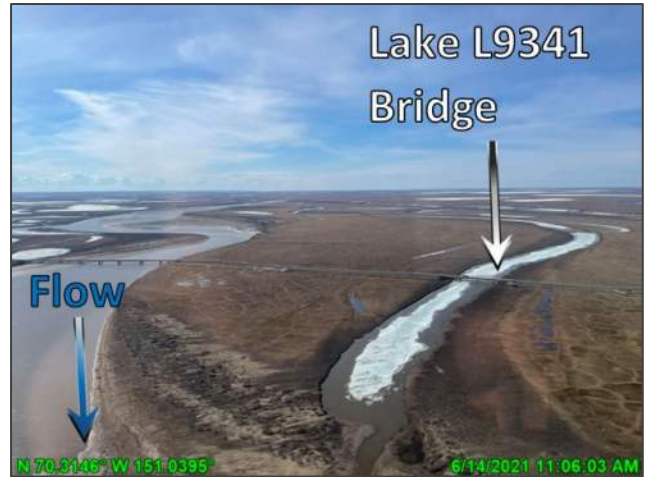
Photo D.20: CD5 road in between Lake L9341 and Nigliq Channel post-breakup, looking south; June 14, 2021
