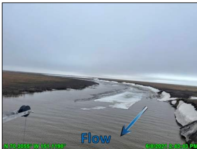
Photo 4.58: Conditions at the Nigliagvik Bridge during discharge measurement one day after peak stage, looking southwest (upstream); June 8, 2021
