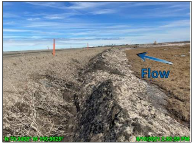
Photo D.6: CD2 road embankment in between the long swale and short swale bridge post-breakup, looking east; June 10, 2021
