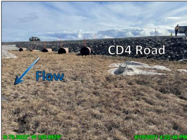
Photo D.13: CD4 road in vicinity of G15 culverts post-breakup, looking southwest; June 10, 2021
