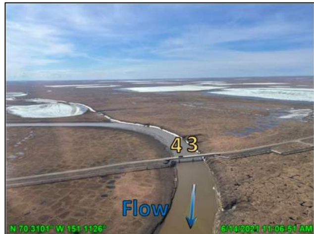
Photo 6.2: Pier numbers on the Nigliagvik Bridge, looking south (upstream); June 14, 2021
