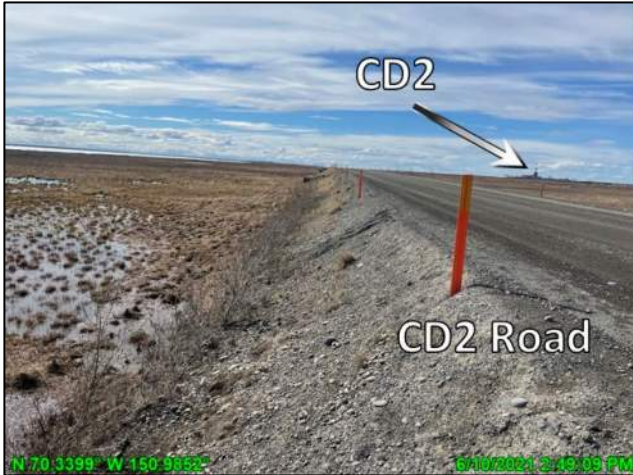
Photo 5.1: CD2 road post-breakup, looking northwest; June 10, 2021
