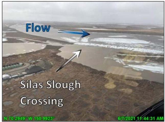
Photo D.36: Peak stage near the slotted Silas Slough ice road crossing, looking southwest; June 7, 2021
