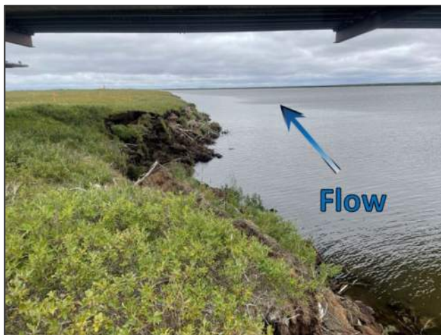
Photo D.23: West bank of Nigliq Channel south of CD5 road during bank erosion survey, looking north; August 12, 2021
