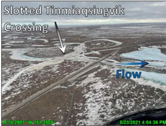
Photo D.44: Pre-breakup conditions at the slotted Tinmiaqsiugvik Bypass ice road crossing, looking southwest; May 23, 2021
