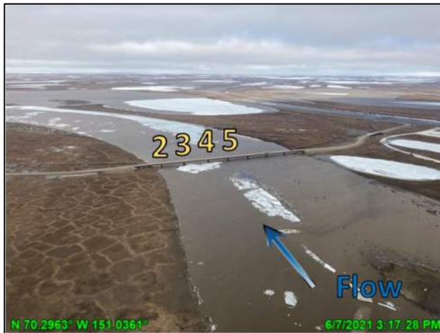
Photo 6.1: Pier numbers on the Nigliq Bridge, looking northeast (downstream); June 7, 2021
