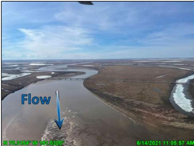
Photo 6.3: Nigliq Channel post breakup showing no channel migration, looking south; June 14, 2021
