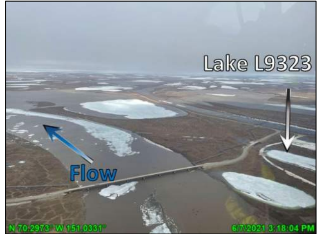
Photo 4.43: Nigliq Channel and Lake L9323 bridge near peak stage showing no overbank flooding, looking northeast; June 7, 2021
