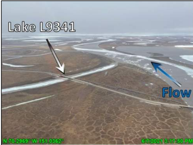
Photo 4.60: CD5 road near Lake L9341 with no overbank flooding, looking north; June 7, 2021
