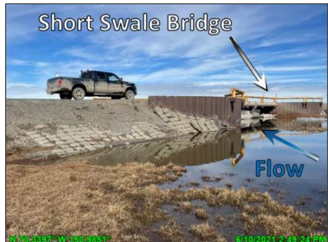
Photo D.4: CD2 road short swale bridge SW abutment, looking northeast; June 10, 2021
