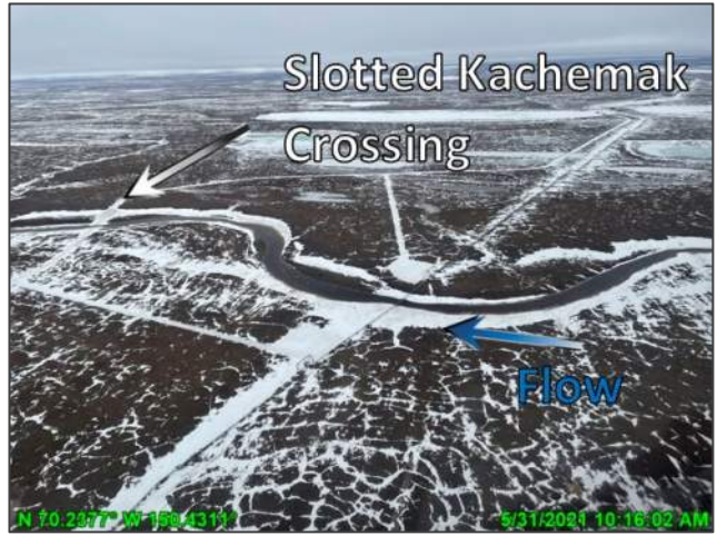
Photo D.34: Pre-breakup conditions near the slotted Kachemach ice road crossing, looking northeast (downstream); May 31, 2021
