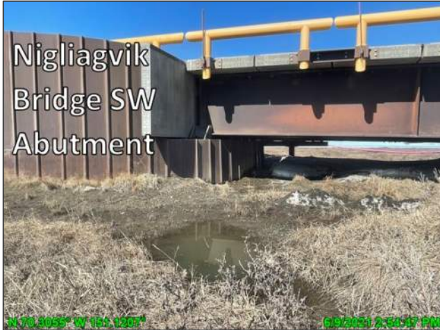
Photo D.17: Nigliagvik SW abutment post-breakup, looking north; June 9, 2021
