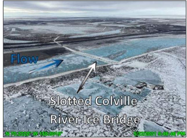
Photo D.26: Local melt near the slotted Colville River Ice Bridge, looking northwest; May 2, 2021
