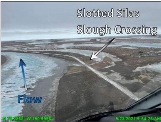
Photo D.35: Pre-breakup conditions at the slotted Silas Slough ice road crossing, looking north; May 23, 2021
