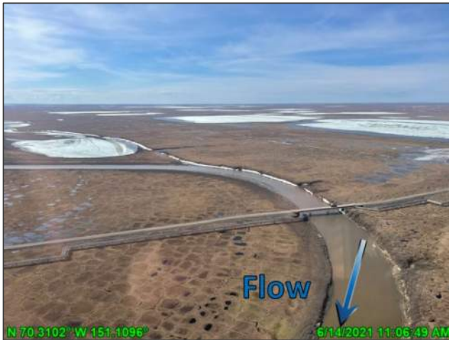
Photo D.21: CD5 road near Nigliagvik Bridge post-breakup, looking south; June 14, 2021
