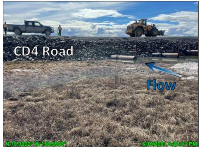
Photo D.14: CD4 road in vicinity of G15 culverts post-breakup, looking west; June 10, 2021
