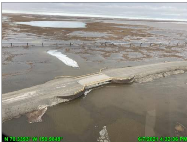
Photo 4.31: Drifted snow and ice underneath the short swale bridge, looking north; June 7, 2021
