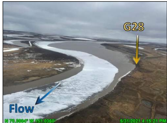
Photo 4.47: Channel ice persisting upstream of the bridge, looking southeast (upstream); May 31, 2021
