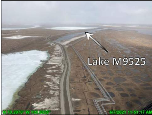
Photo 4.40: Conditions prior to peak at the CD4 road near G15/G16 culvert battery, looking north; June 7, 2021
