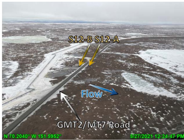
Photo 3.5: Drifted snow blocking flow near S12 gages, looking southwest; May 27, 2021
