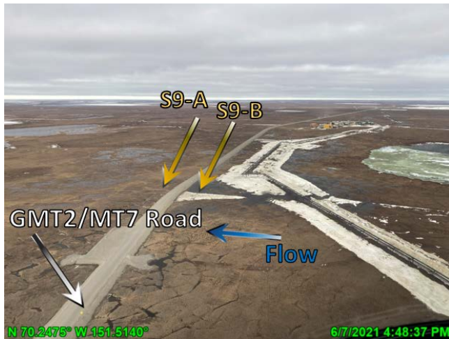
Photo F.3: Near peak stage at S9-B, looking northeast; June 7, 2021
