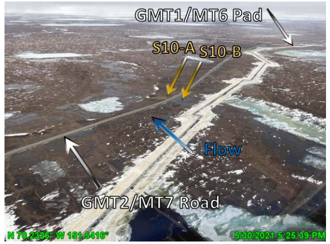
Photo F.6: Increasing meltwater on the upstream (south) side of road, looking northeast; May 30, 2021
