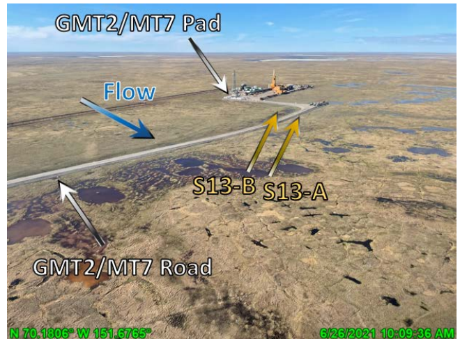
Photo F.20: Summer conditions near S13, looking south (upstream); June 26, 2021
