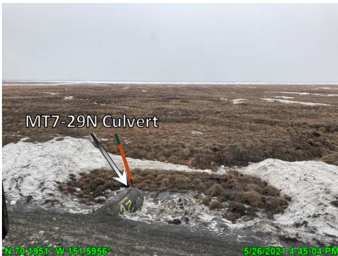
Photo 3.1: Culvert MT7-29 outlet after mechanical clearing of snow, looking north; May 26, 2021
