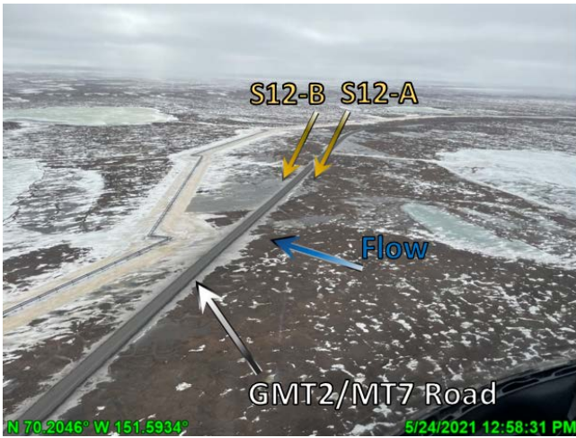
Photo F.13: Ponded water on the upstream side of the road near S12, looking south; May 24, 2021
