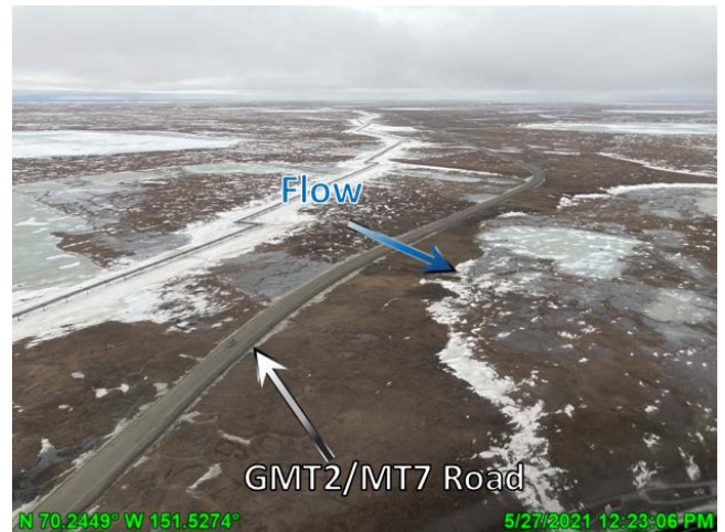
Photo 3.6: Drifted snow along GMT2/MT7 road embankments, looking southwest; May 27, 2021
