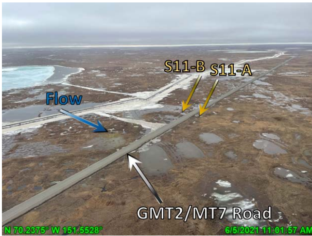
Photo F.11: Receding stage near S11, looking south; June 5, 2021
