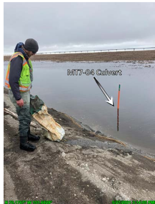
Photo 3.2: Bladder after being removed from culvert MT7-04 still blocked with ice; May 27, 2021
