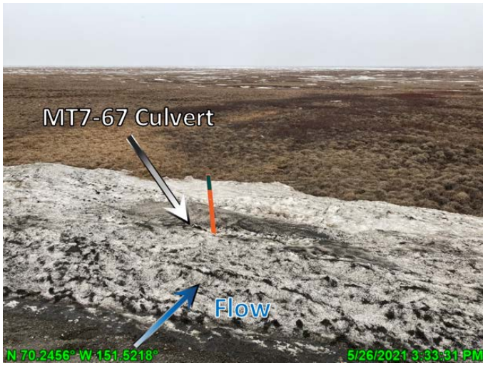
Photo 3.3: Culvert MT7-67 outlet partially buried with snow, looking north; May 26, 2021
