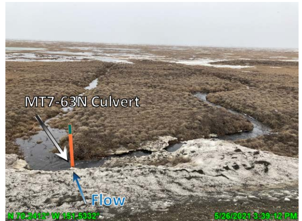
Photo 3.8: Flow through culvert MT7-63 showing natural drainage pattern cutting through snow, looking north; May 26, 2021
