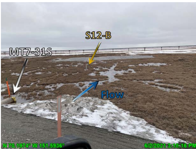
Photo F.15: Minimal ponding along road embankments at S12, looking east (downstream); June 2, 2021
