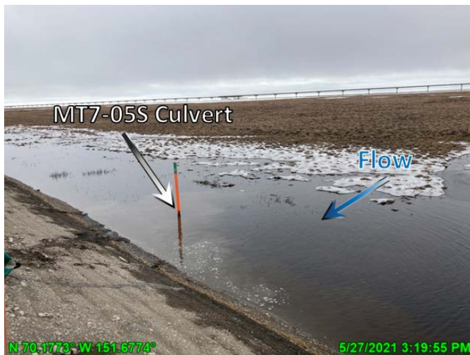
Photo 3.9: Wash line with no sloughing along the south embankment near MT7-05, looking east; May 27, 2021
