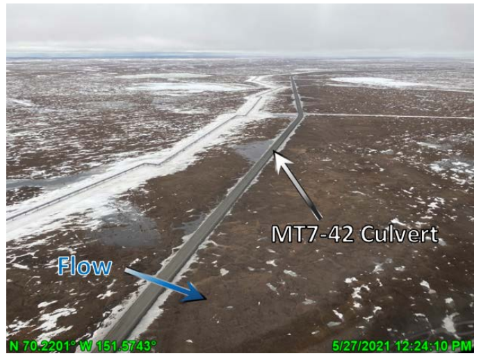
Photo 3.4: Ponding near culvert MT7-42 looking southwest; May 27, 2021
