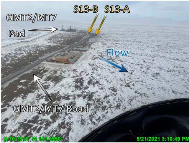
Photo F.17: Ponded meltwater on the upstream side of the road near S13, looking southwest; May 21, 2021
