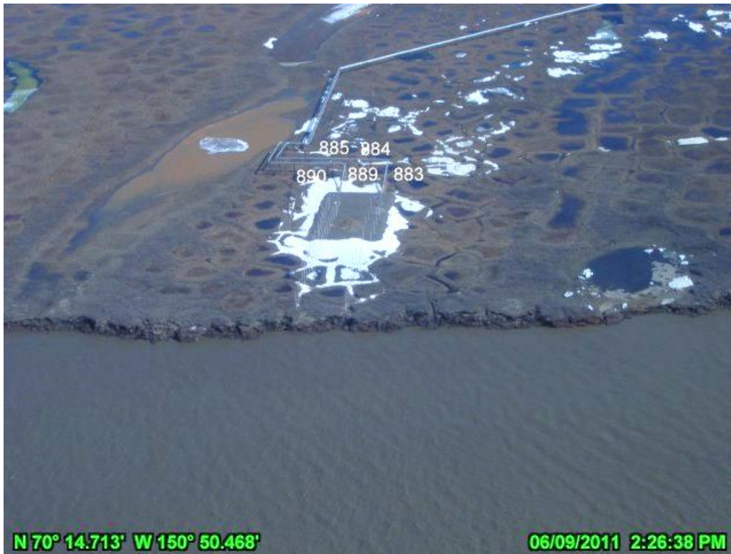
PHOTO A.11 HDD EAST, JUNE 9, 2011: AERIAL PHOTO OF EAST BANK, LOOKING EAST
