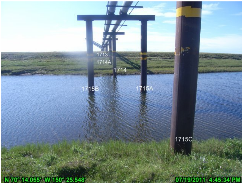
PHOTO A.22 KACHEMACH RIVER CROSSING, JULY 19, 2011: EAST BANK, LOOKING WEST
