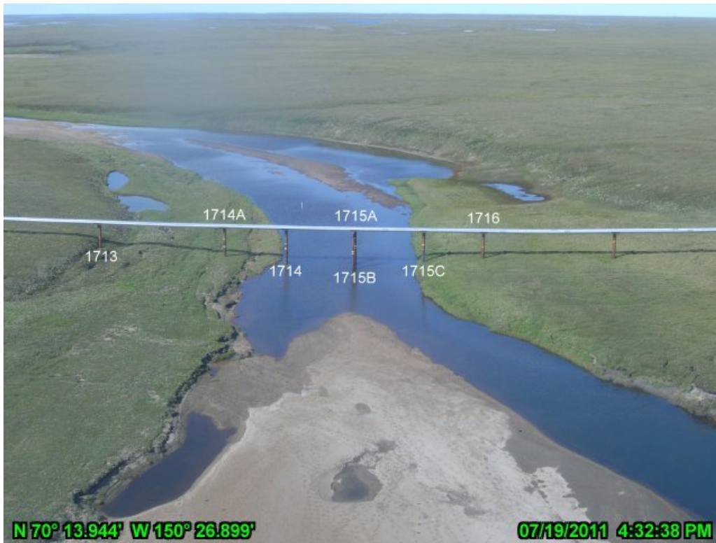
PHOTO A.19 KACHEMACH RIVER CROSSING, JULY 19, 2011: AERIAL PHOTO, LOOKING NORTH
