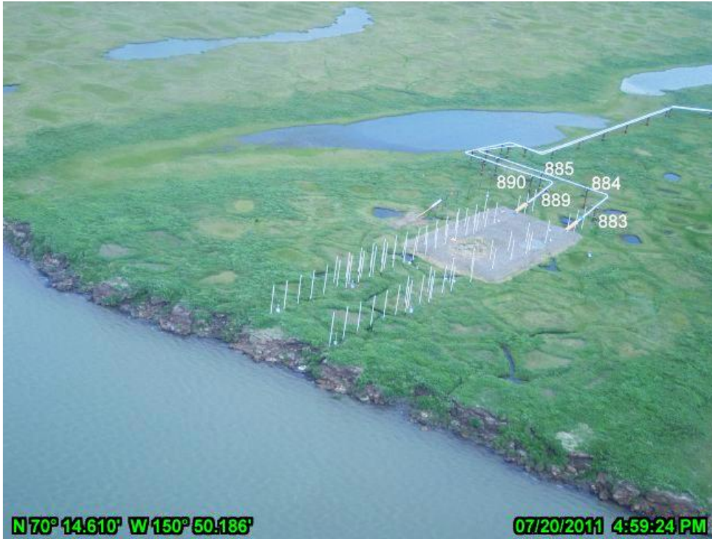
PHOTO A.13 HDD EAST, JULY 20, 2011: AERIAL VIEW OF TROUGH FROM WATER, LOOKING NORTHEAST
