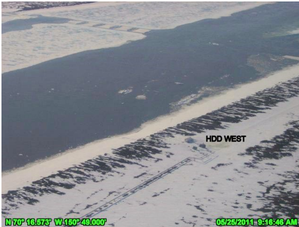
PHOTO A.1 HDD WEST, MAY 25, 2011: FIVE DAYS BEFORE PEAK STAGE, LOOKING SOUTHEAST
