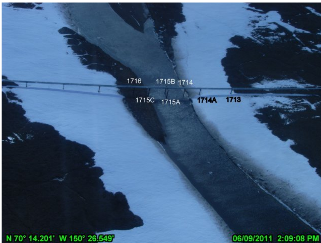
PHOTO A.18 KACHEMACH RIVER CROSSING, JUNE 9, 2011: AERIAL PHOTO, LOOKING SOUTHWEST
