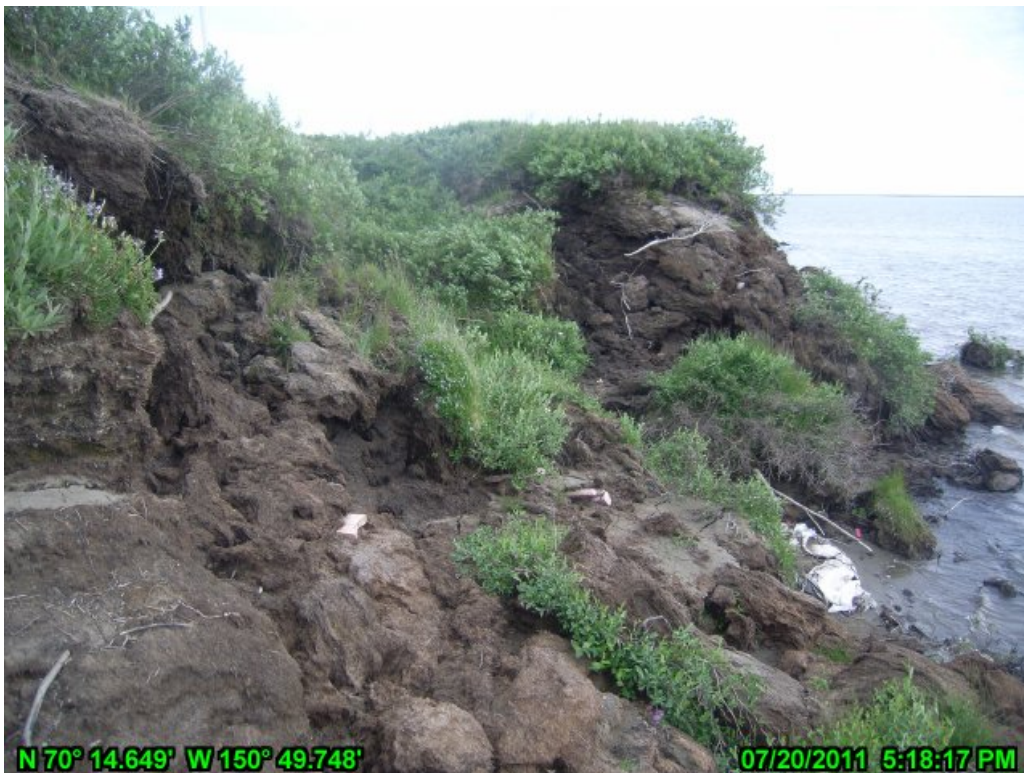
PHOTO A.14 HDD EAST, JULY 20, 2011: TROUGH FROM TOE OF BANK, LOOKING SOUTHEAST
