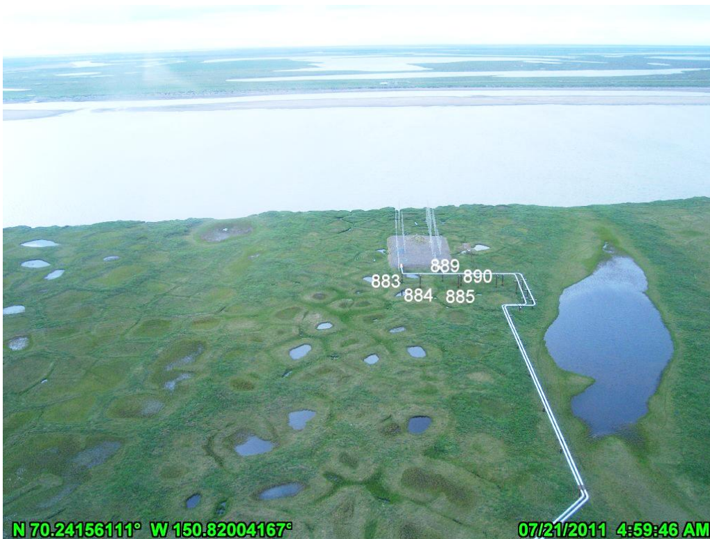
PHOTO A.12 HDD EAST, JULY 21, 2011: AERIAL PHOTO OF EAST BANK, LOOKING WEST
