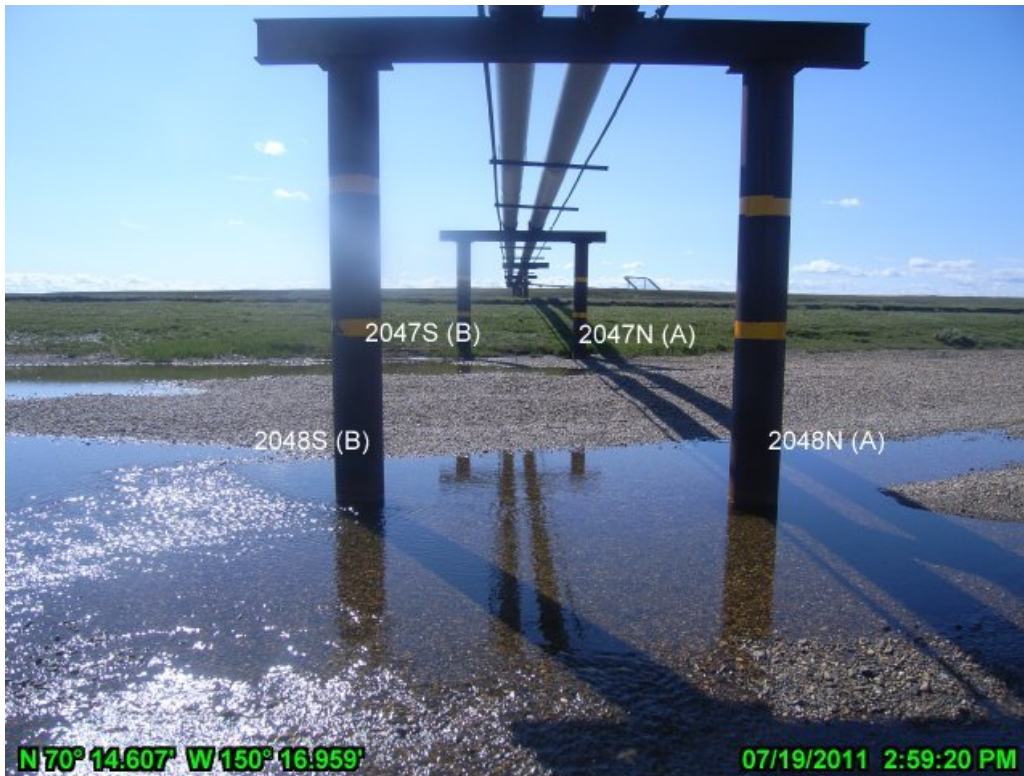
PHOTO A.29 MILUVEACH RIVER CROSSING, JULY 19, 2011: EAST BANK, LOOKING WEST
