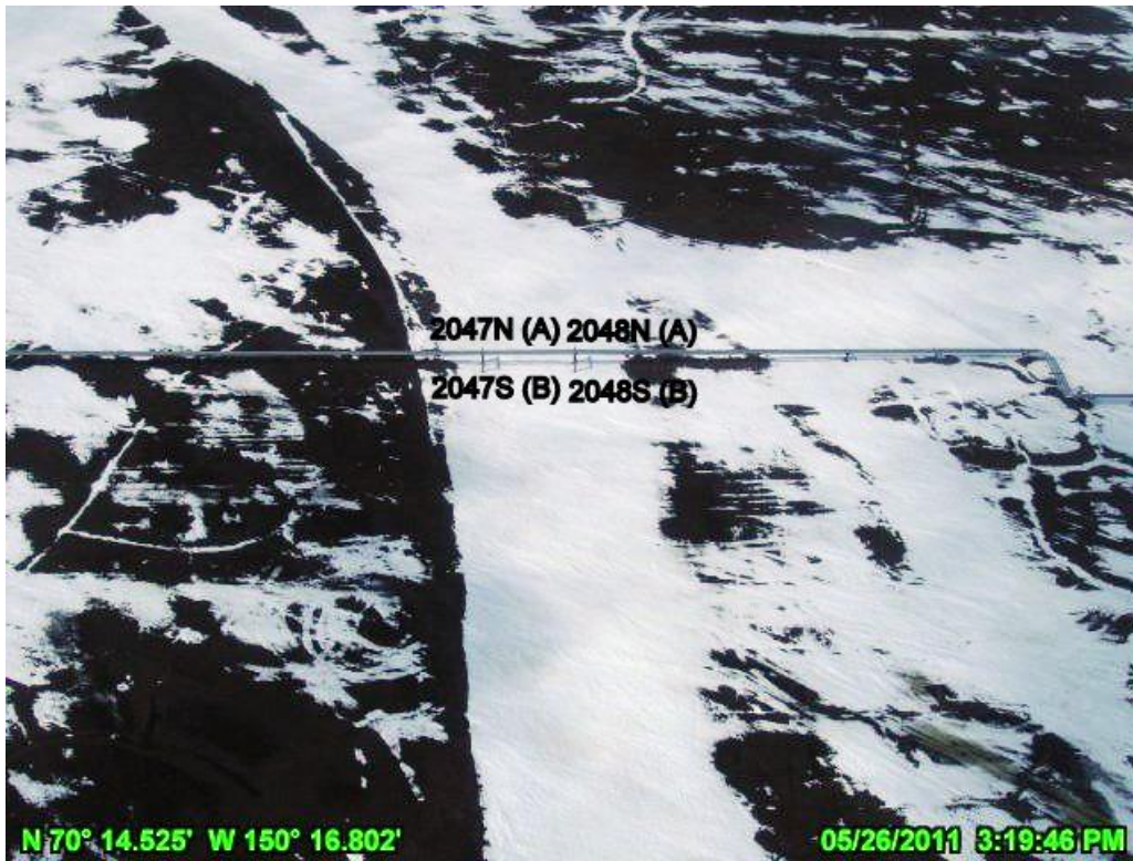
PHOTO A.25 MILUVEACH RIVER CROSSING, MAY 26, 2011: FOUR DAYS BEFORE PEAK STAGE, LOOKING NORTH
