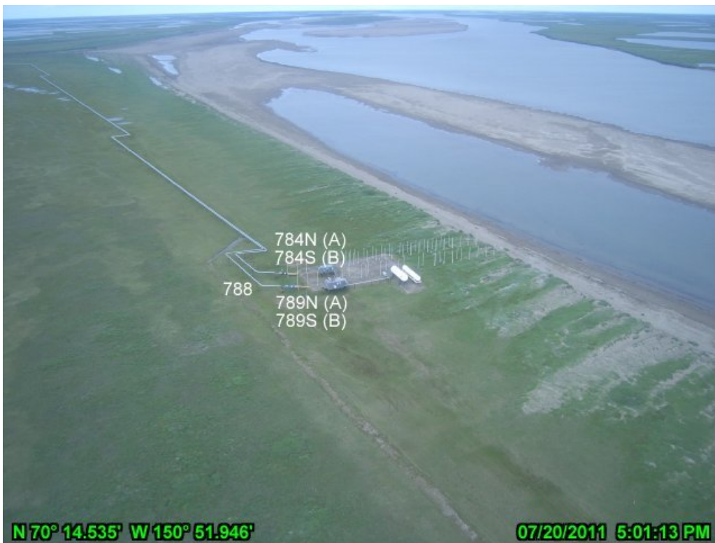
PHOTO A.6 HDD WEST, JULY 20, 2011: WEST BANK, LOOKING NORTHEAST
