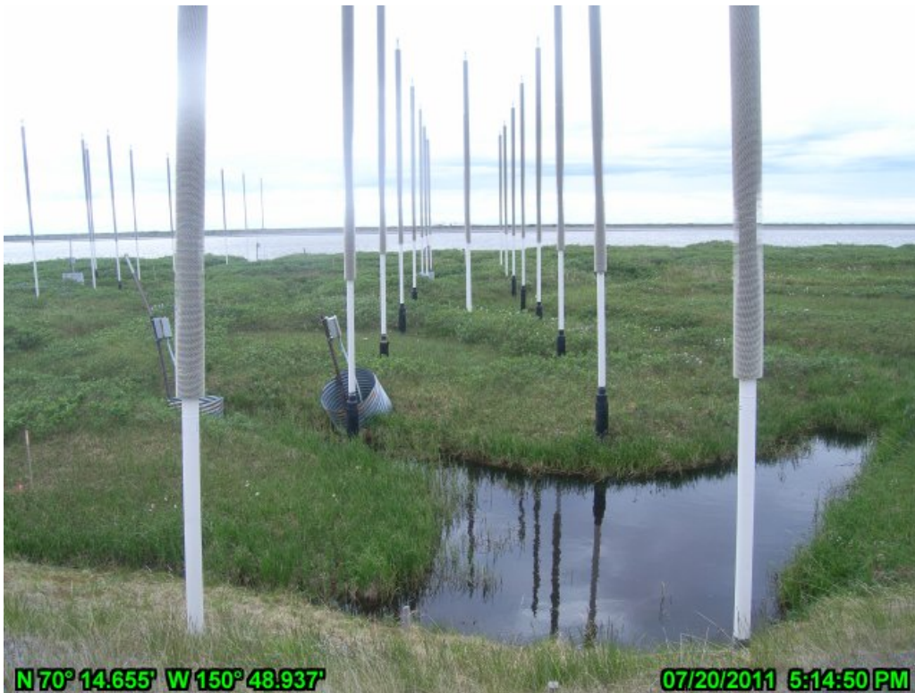
PHOTO A.16 HDD EAST, JULY 20, 2011: LOOKING WEST THROUGH THERMOSIPHONS WITH TROUGH IN FOREGROUND
