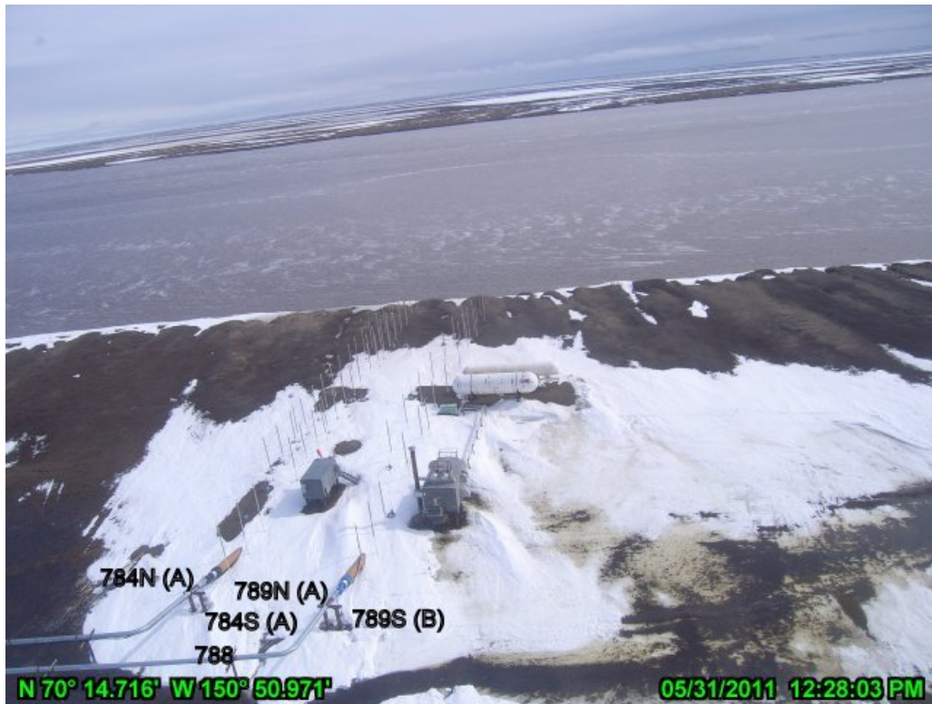
PHOTO A.3 HDD WEST, MAY 31, 2011: ONE DAY AFTER PEAK STAGE, LOOKING EAST
