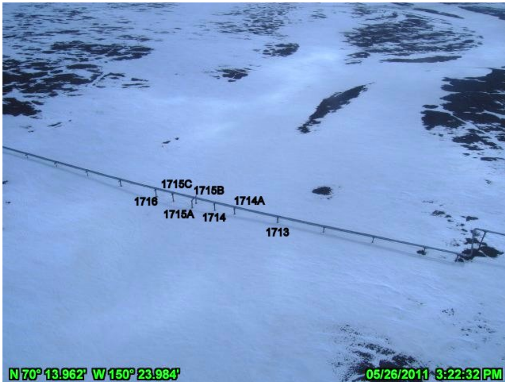
PHOTO A.17 KACHEMACH RIVER CROSSING, MAY 26, 2011: FOUR DAYS BEFORE PEAK STAGE, LOOKING SOUTHEAST
