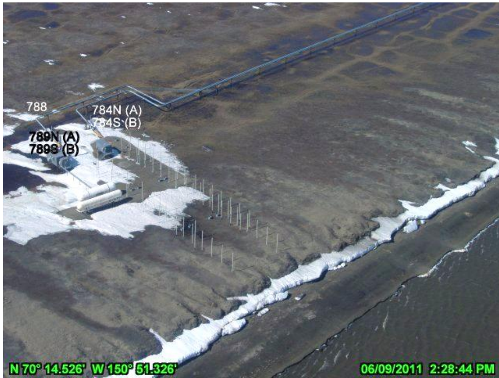
PHOTO A.5 HDD WEST, JUNE 9, 2011: AERIAL PHOTO, LOOKING NORTHWEST
