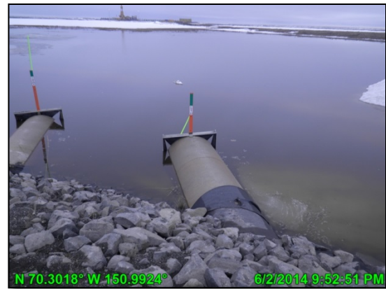
Photo 11: Flow through CD4 Road culverts; June 2, 2014
