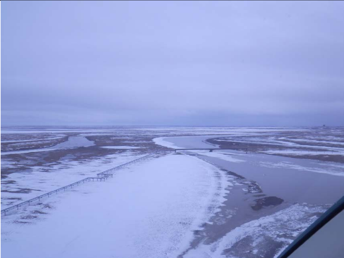
Photo 2: Ulamnigiaq pipeline crossing; June 2, 2014
