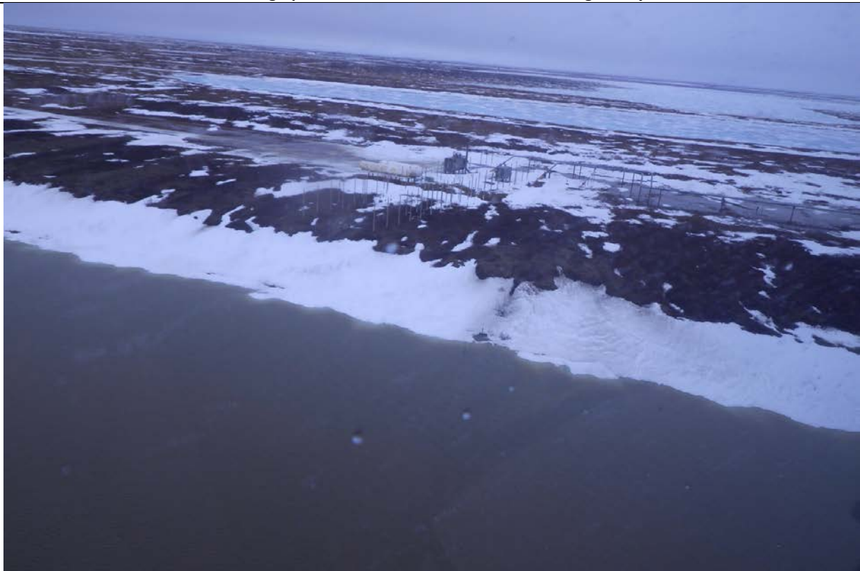
Photo 2: Gages at MON9 near the HDD crossing; May 16, 2014
