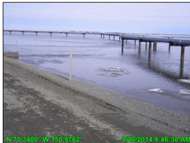
Photo 5: CD2 road culvert conveying water; May 20, 2014
