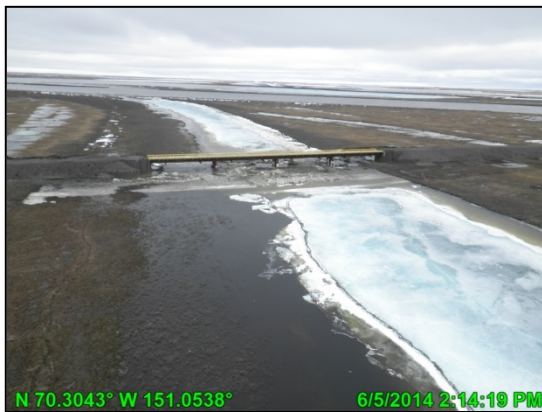
Photo 15: Lake L9341 Bridge; June 5, 2014
