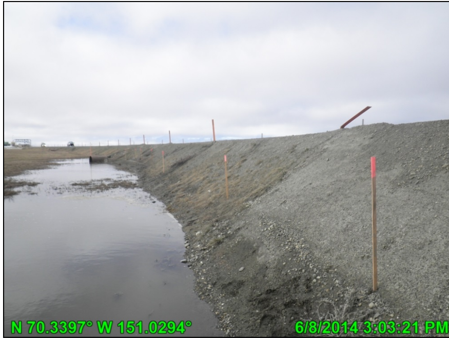
Photo 13: Stakes placed to illustrate minor high water scarp; June 8, 2014
