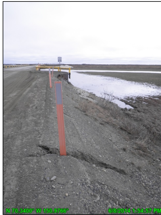
Photo 14: Minor erosion around road delineator; June 8, 2014
