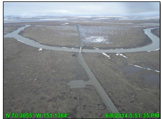
Photo 24: Nigliagvik Bridge looking east; June 8, 2014
