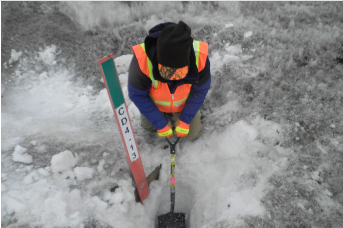
Photo 2: Shoveling out culvert at G40; May 9, 2014
