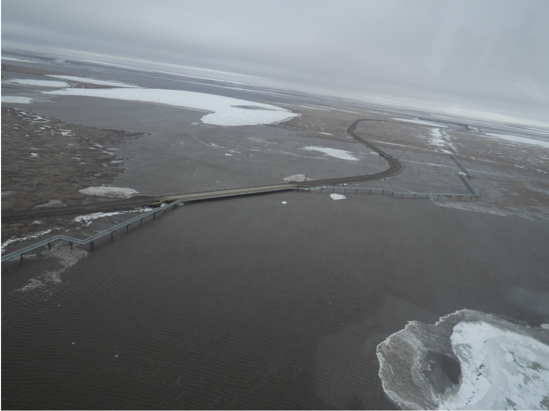
Photo 1: Flow through CD2 swale bridges; May 30, 2014
