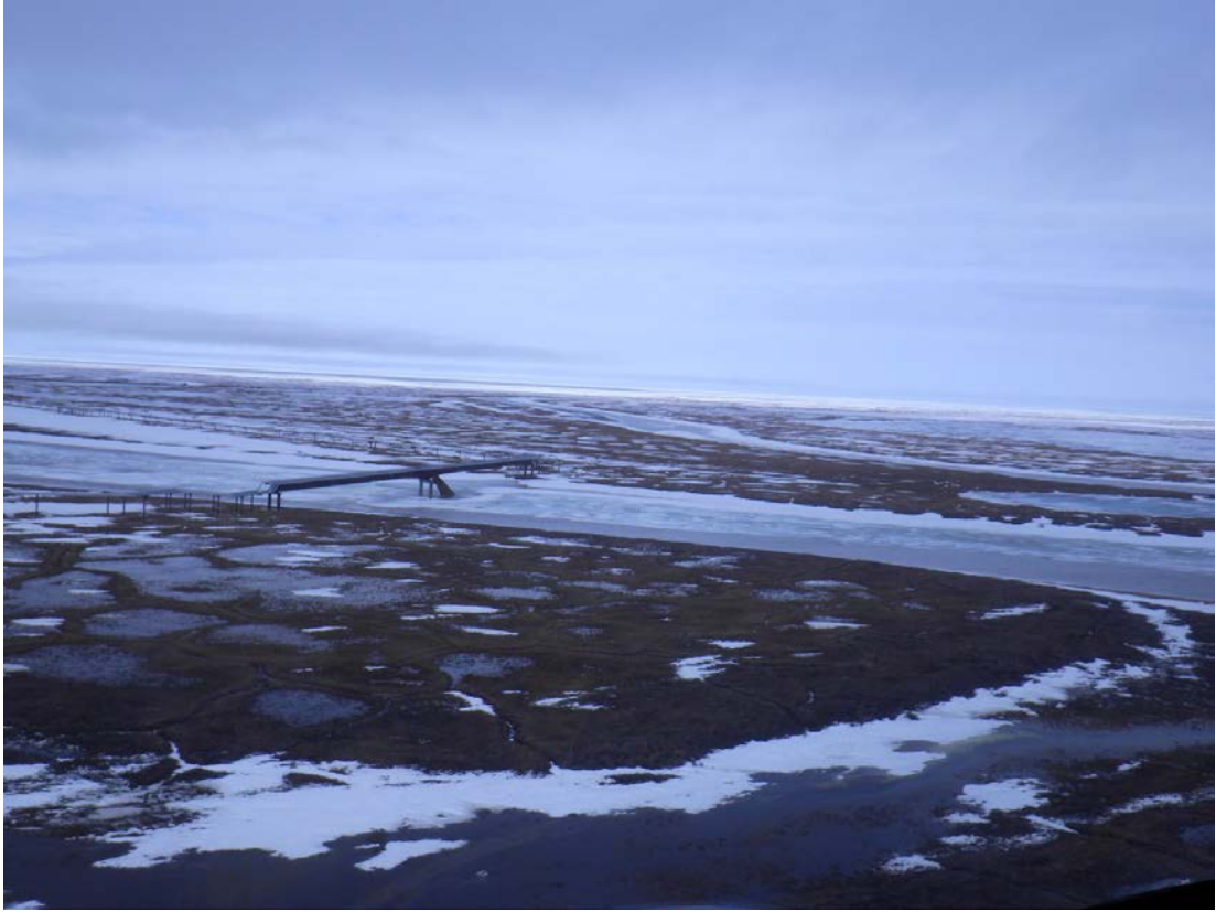
Photo 6: Pipeline crossing at the Ulamnigiaq Channel; May 17, 2014
