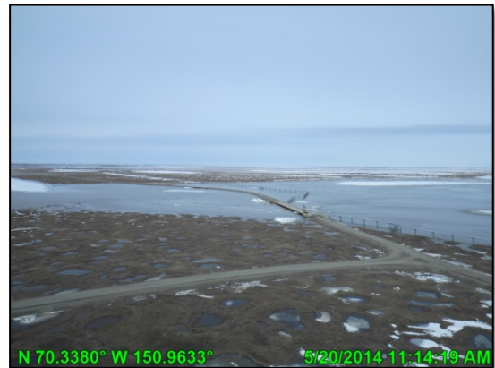
Photo 4: Swale bridges conveying water; May 20, 2014
