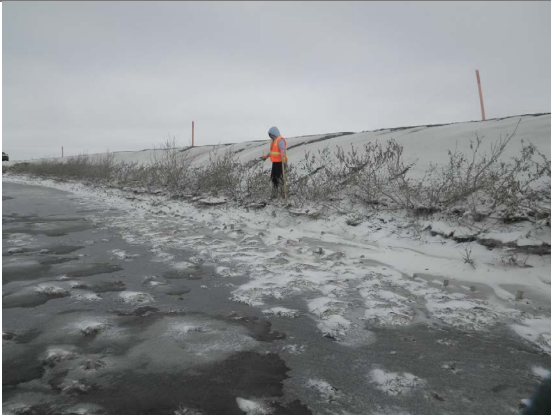
Photo 1: Erosion Survey on the CD2 Road; May 25, 2014
