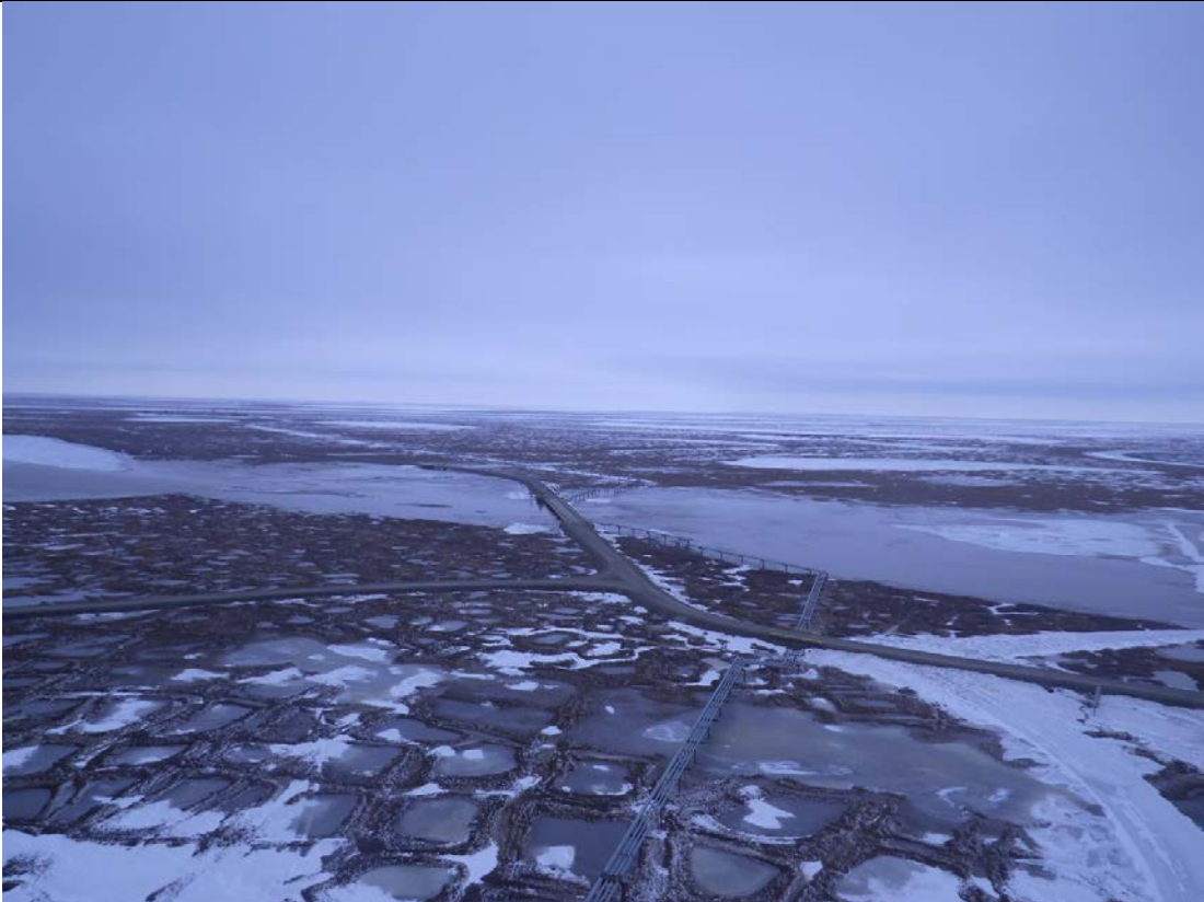
Photo 3: Long swale bridge on CD2 Road conveying water; May 19, 2014
