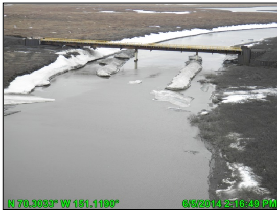
Photo 23: Nigliagvik Bridge looking downstream; June 5, 2014
