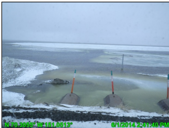
Photo 8: CD2 Road culverts at Gage G6; June 1, 2014
