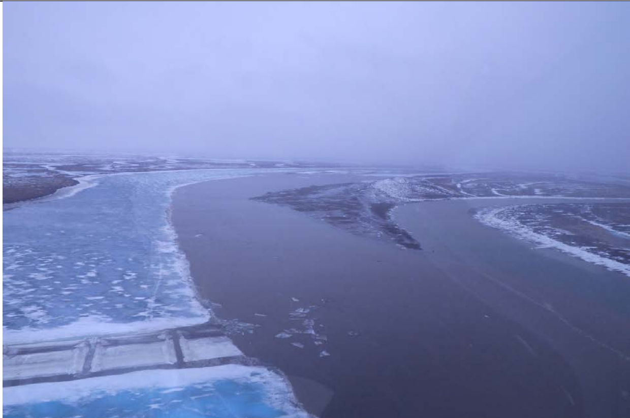
Photo 1: Looking upstream at the slotted Colville Ice Bridge; May 16, 2014
