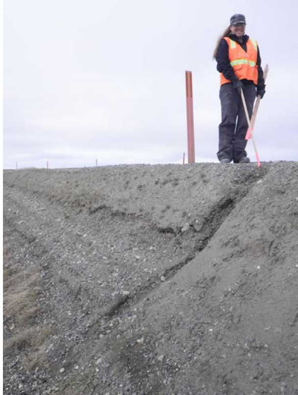
Photo 2: Minor runoff erosion effects on CD2 Road; June 8, 2014
