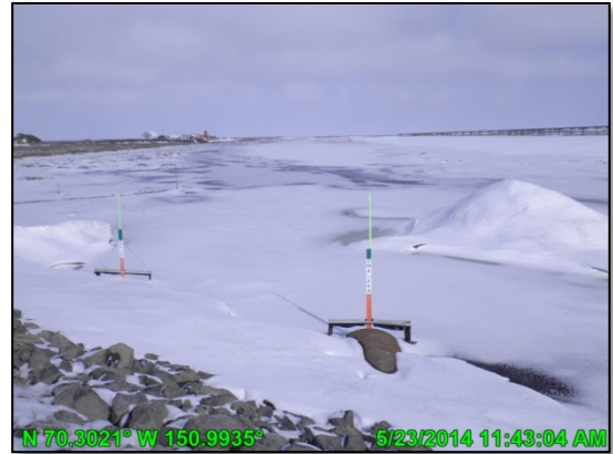
Photo 7: CD4 Road culverts; May 23, 2014
