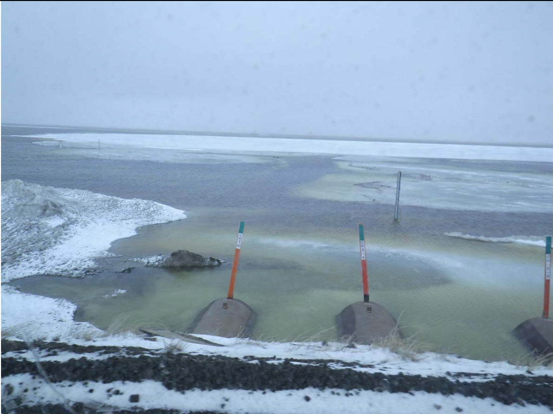
Photo 4: Culvert battery at G6 near the CD2 pad; June 1, 2014
