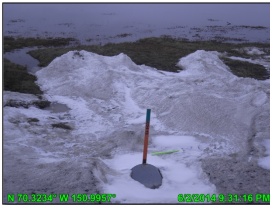
Photo 10: Minimal flow through CD4 Road culvert; June 2, 2014
