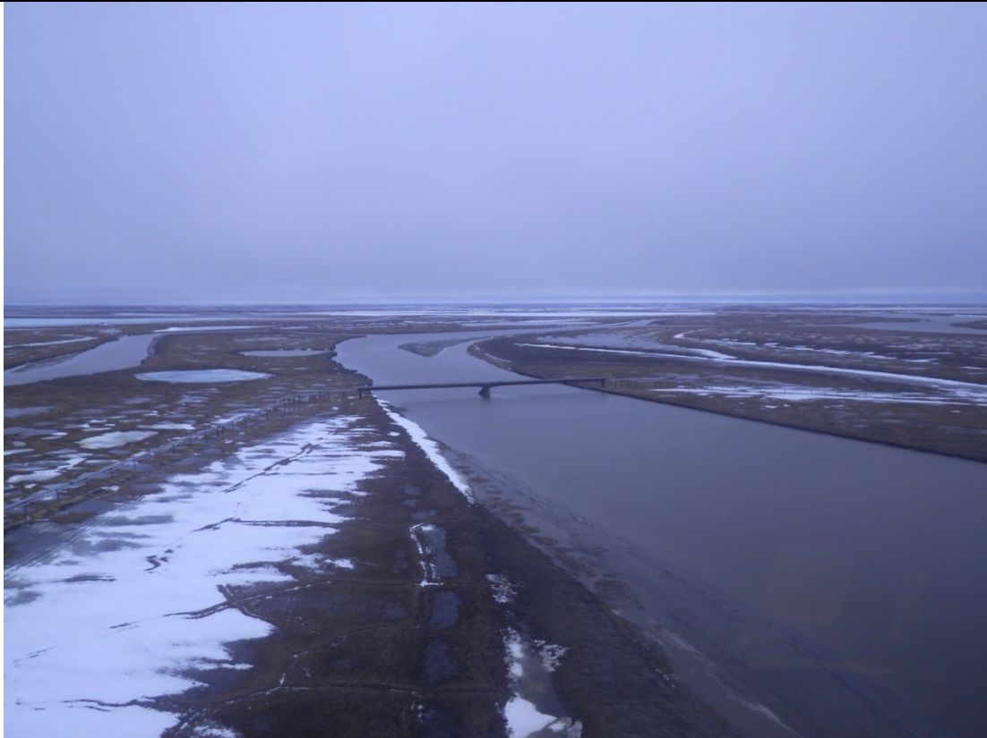
Photo 6: Pipeline crossing on the Ulamniaq Channel; June 6, 2014
