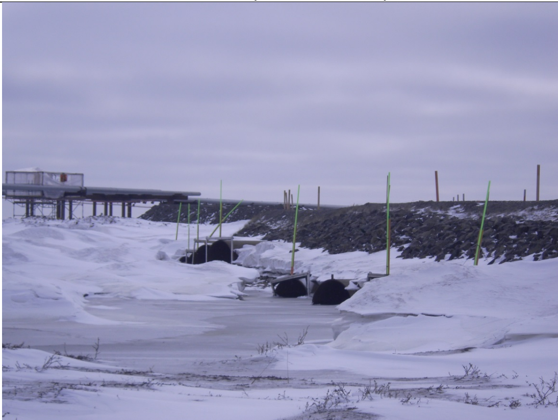
Photo 2: Culvert battery on the CD4 Road; May 25, 2014
