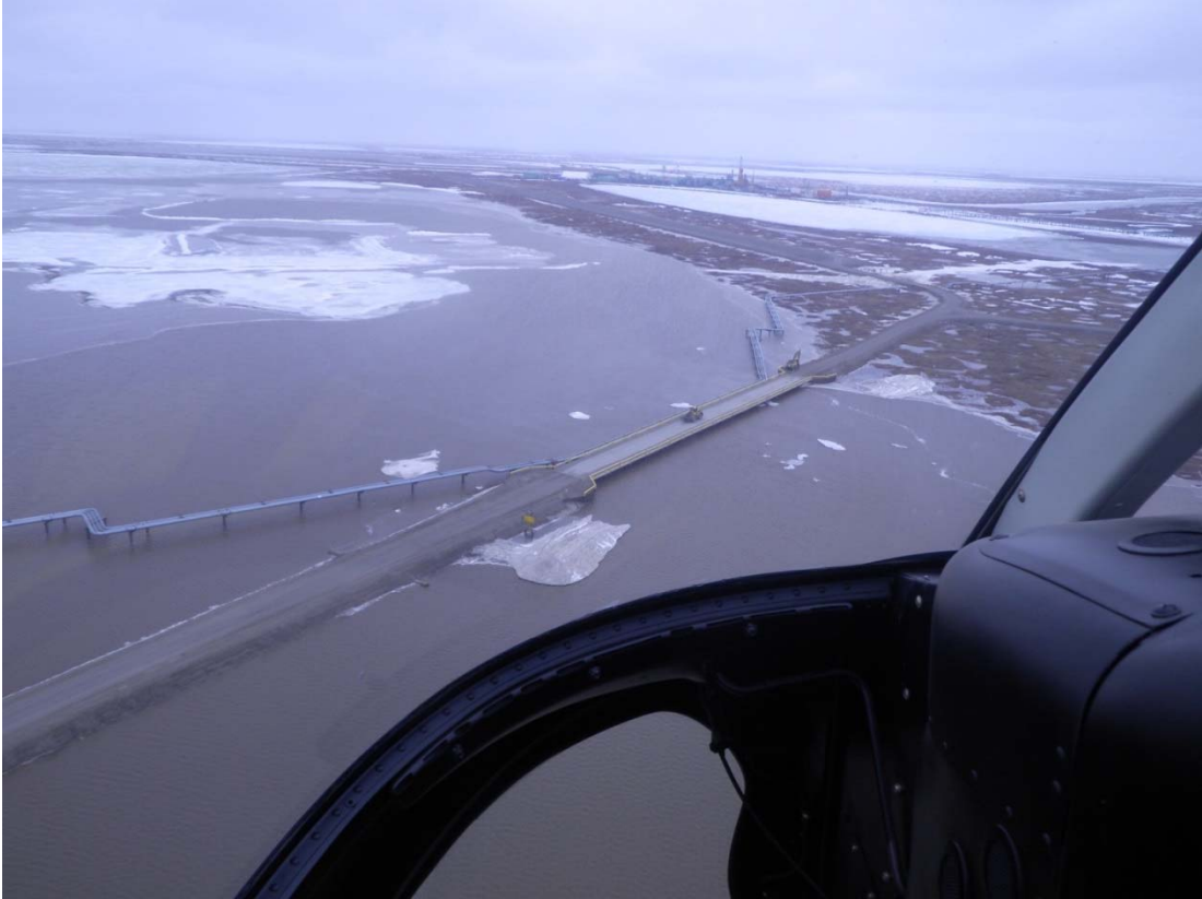
Photo 5: Long swale bridge on CD2 Road; May 21, 2014
