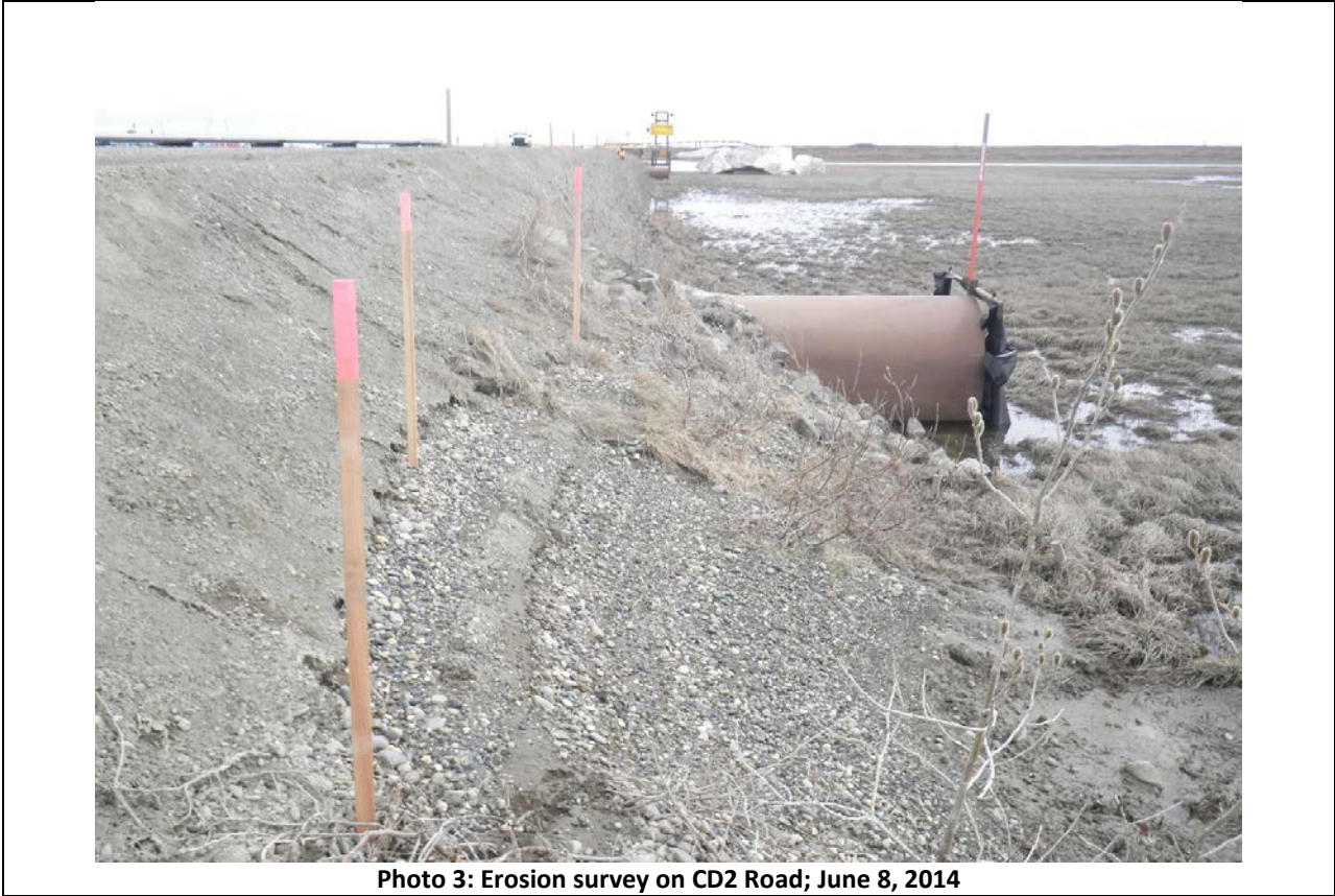
Photo 3: Erosion survey on CD2 Road; June 8, 2014
