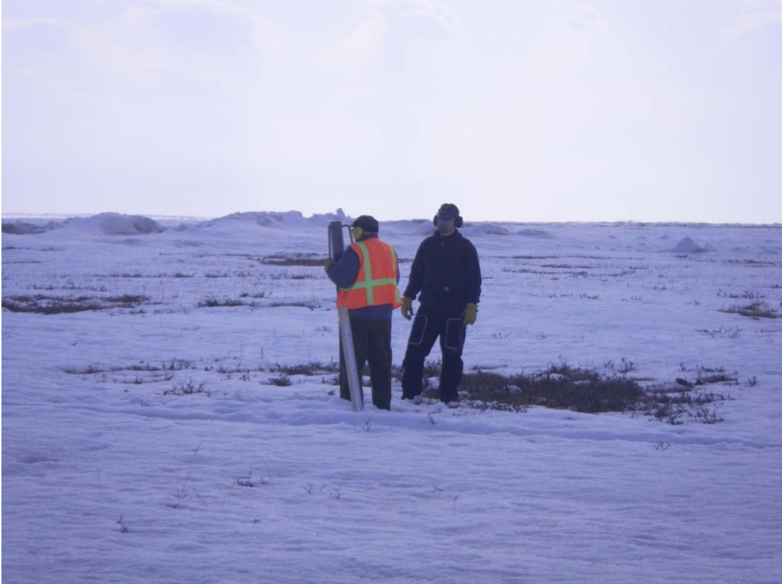
Photo 1: Installing gages at G38; May 4, 2014
