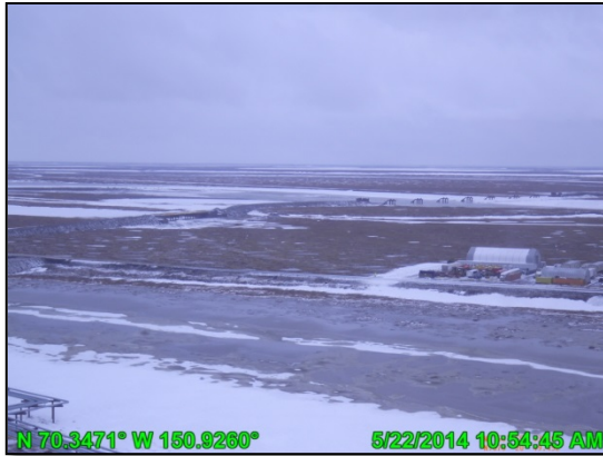
Photo 6: CD4 and CD5 roads, looking southwest, May 22, 2014
