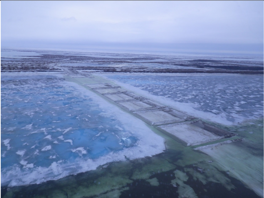
Photo 1: Slotted Colville Ice Bridge near the HDD crossing; May 15, 2014
