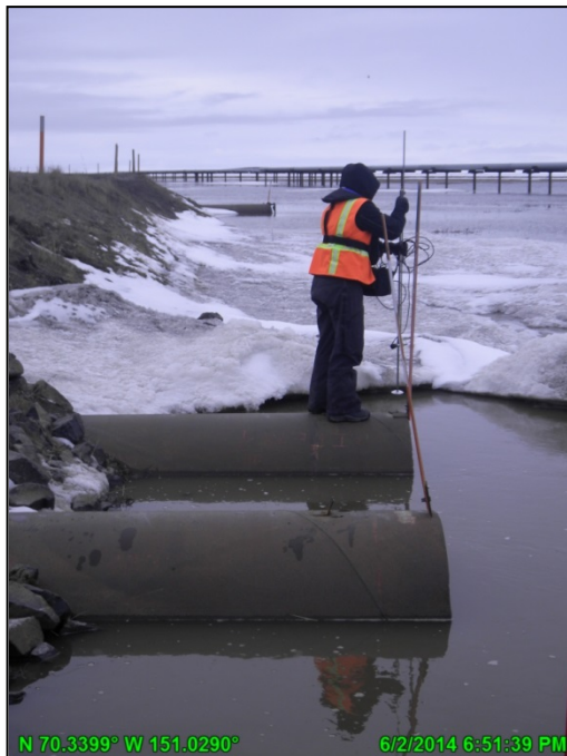
Photo 12: Discharge measurement at CD2 road culvert; June 2, 2014
