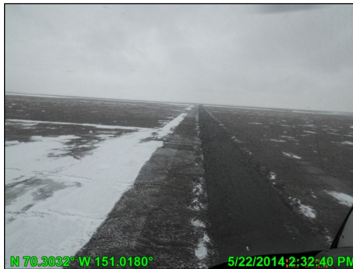
Photo 17: CD5 Road between Lake L9341 and Nigliagvik Channel; May 22, 2014
