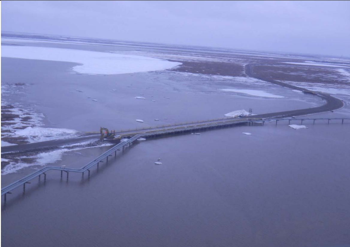
Photo 3: Long swale bridge on CD2 Road; May 22, 2014
