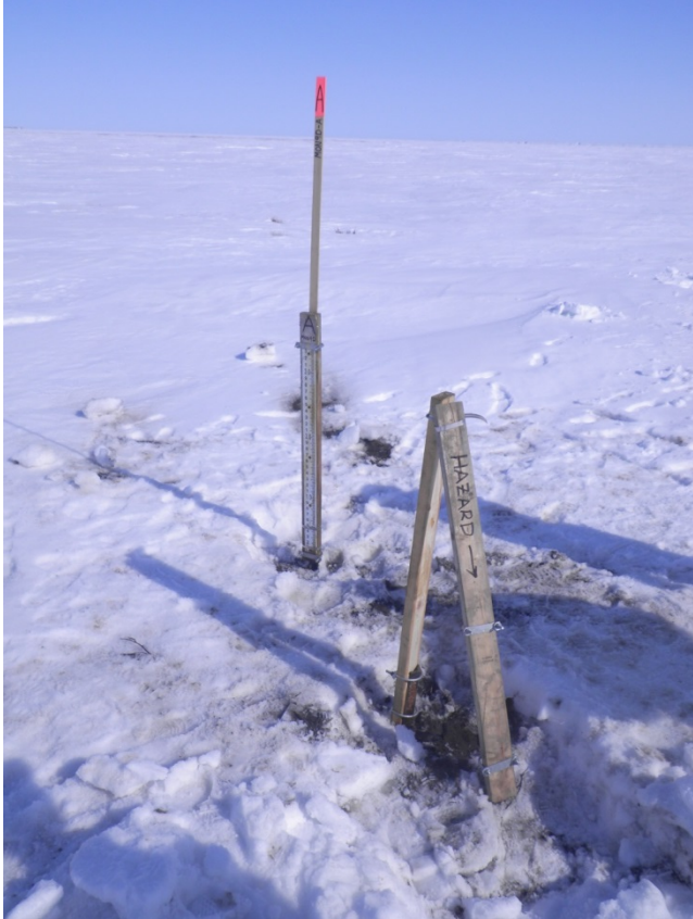
Photo 2: Hazardous exposed steel at MON9D marked; May 2, 2014
