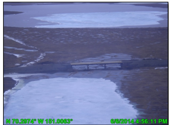
Photo 16: Lake L9323 Bridge and CD5 access road culvert; June 6, 2014
