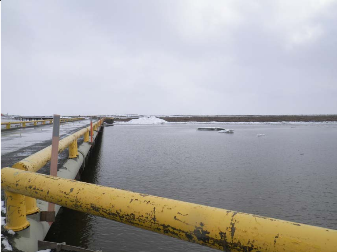
Photo 5: Upstream side of long swale bridge; May 23, 2014
