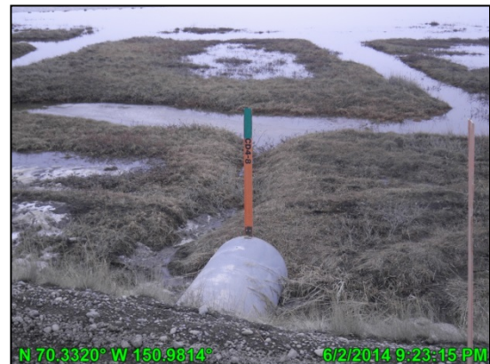
Photo 9: CD4 Road culvert with no flow present; June 2, 2014
