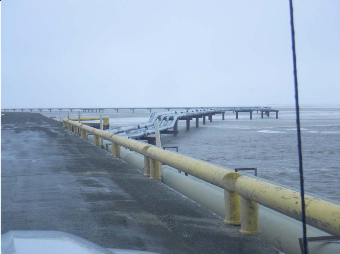
Photo 3: Water flowing through the long swale bridge; June 1, 2014
