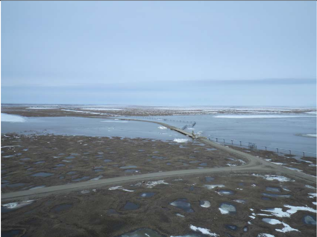
Photo 1: Long swale bridge on CD2 Road; May 20, 2014
