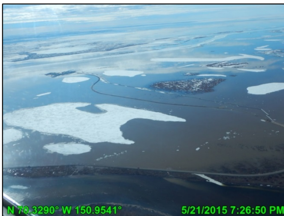
Photo 3.4: Extent of inundation near peak flooding around the CD2 road and pad, looking northwest; May 21, 2015
