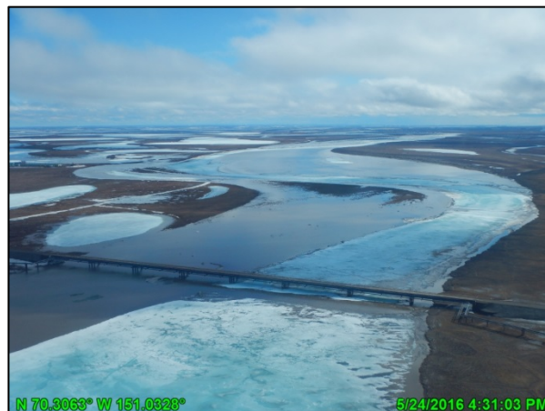
Photo 3.5: Intact channel ice starting to deteriorate near the Nigliq Bridge, looking south; May 24, 2016
