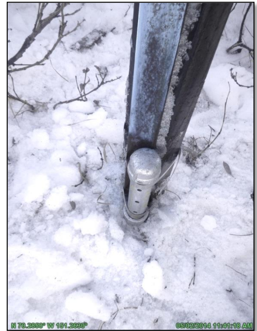
Photo 2.3: Pressure transducer setup; May 2, 2014
