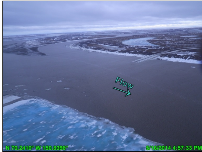
Photo C.13: Colville East Channel ice road crossing ramps, looking southwest; May 16, 2014
