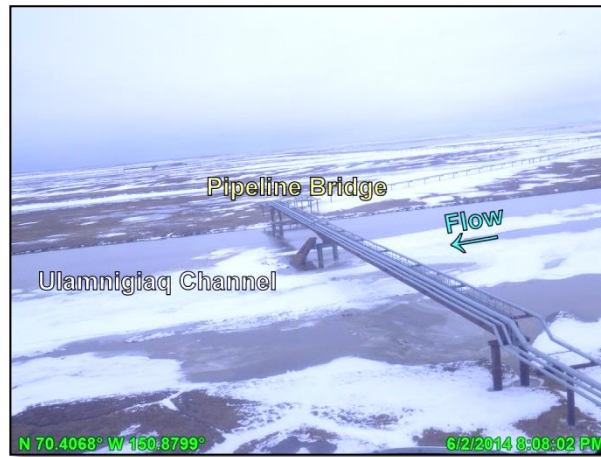
Photo 3.20: Ulamnigiq Channel pipeline crossing at peak stage, looking north; June 2, 2014
