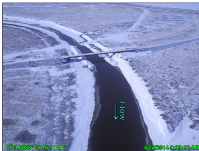
Photo C.27: Degradation of Nigliagvik Channel Bridge construction ice pad, looking south; May 24, 2014
