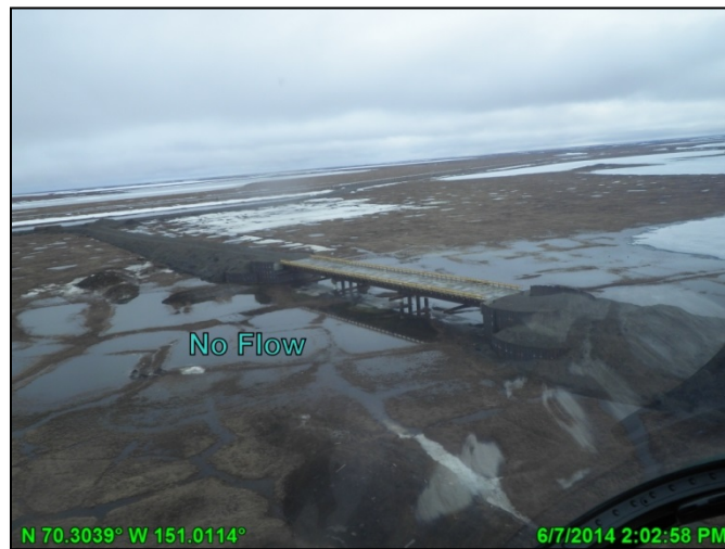
Photo C.32: Lake L9323 Bridge crossing open water, looking southeast; June 7, 2014
