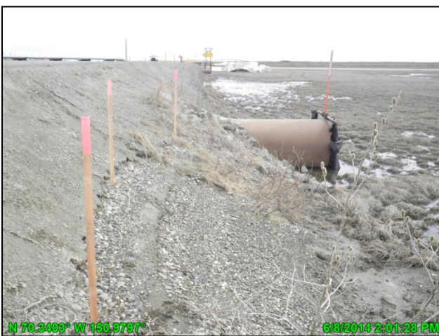
Photo 5.2: CD2 Road Erosion Survey, looking north; June 8, 2014
