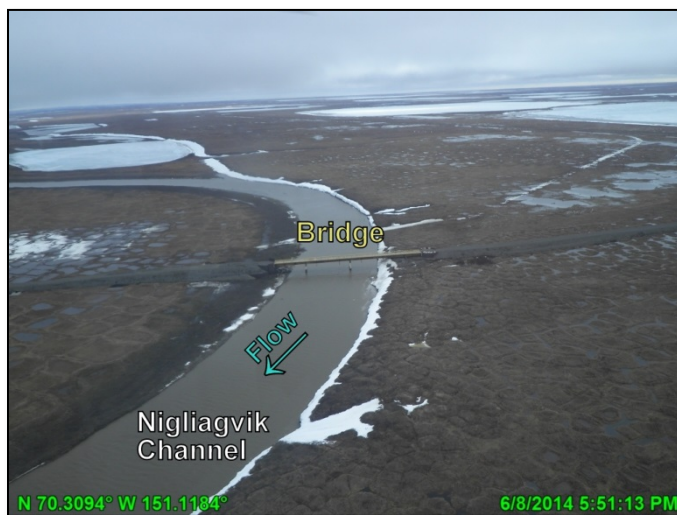
Photo 3.17: Nigliagvik Channel Bridge, looking south, June 8, 2014
