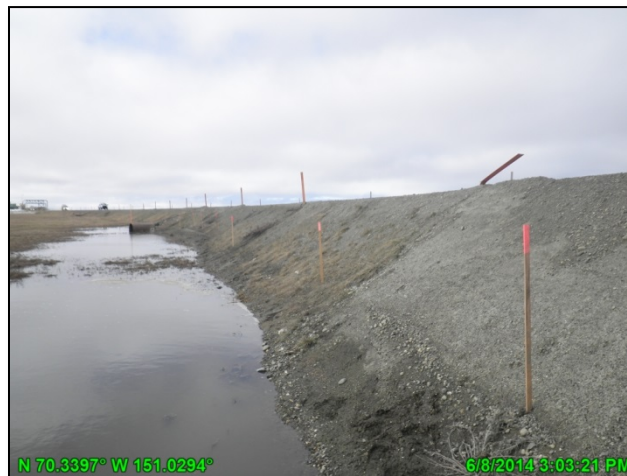
Photo C.6: CD2 Road Erosion Survey, looking north; June 8, 2014
