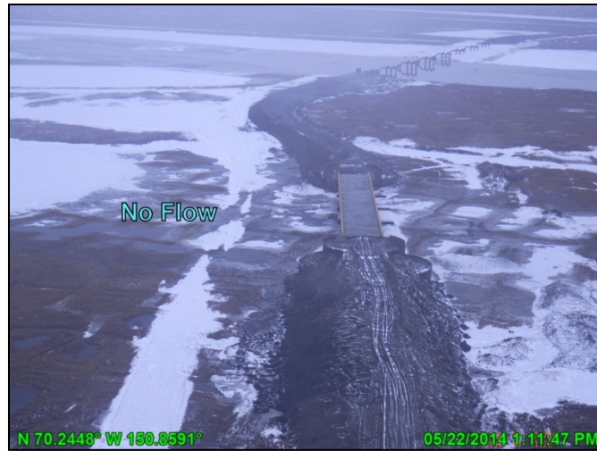
Photo C.31: Lake L9323 Bridge and construction ice pad, looking west, May 22, 2014
