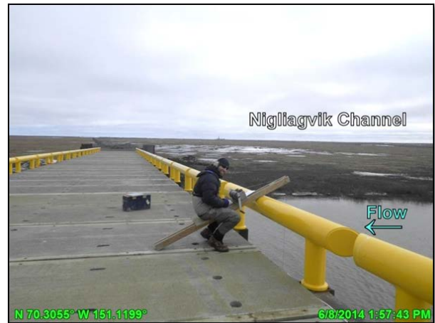
Photo 2.5: Nigliagvik Channel Bridge direct discharge measurement collection, looking east; June 8, 2014
