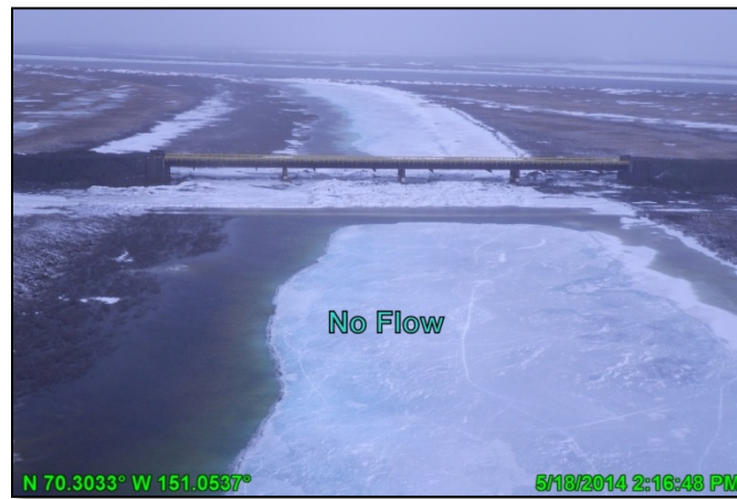
Photo C.29: Lake L9341 Bridge and construction ice pad, looking northeast; May 18, 2014
