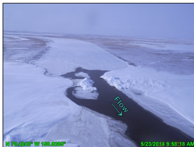
Photo C.18: Flow through slotted Pineapple Gulch ice road crossing, looking southwest; May 23, 2014
