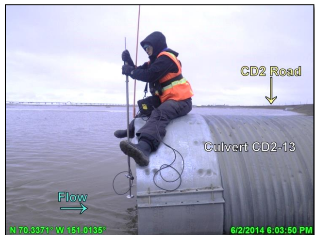
Photo 3.11: Collecting a discharge measurement at CD2 Road culvert during peak stage, looking northwest; June 2, 2014
