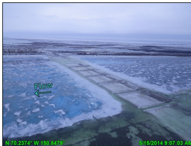
Photo C.12: Colville East Channel ice road crossing slotted, looking east; May 15, 2014
