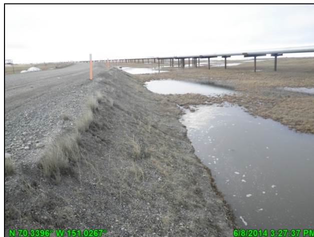
Photo C.7: CD2 Road Erosion Survey, looking north; June 8, 2014
