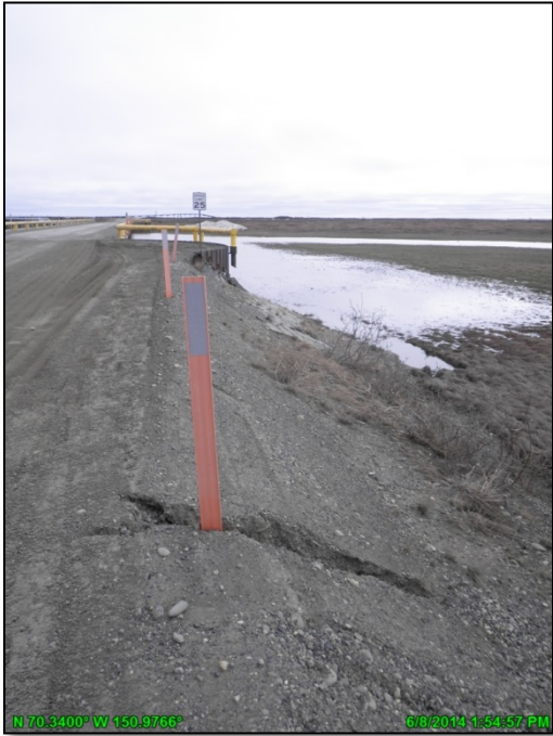
Photo C.9: CD2 Road Erosion Survey, looking north; June 8, 2014
