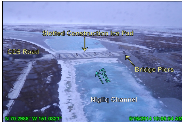
Photo 6.1: Nigliq Channel Bridge pilings at slotted construction ice pad, looking north; May 16, 2014
