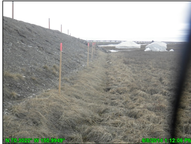
Photo C.10: CD4 Road Erosion Survey; June 8, 2014
