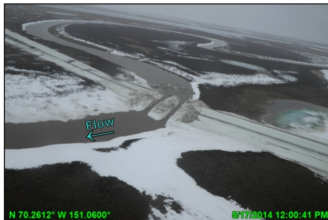
Photo C.15: Flow through slotted sections of the Nigliagvik exploration ice road crossing, looking southeast; May 17, 2014
