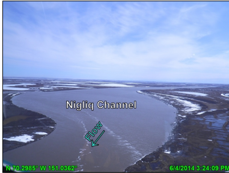
Photo 3.8: Nigliq Channel upstream of the bridge crossing, looking south; June 4, 2014
