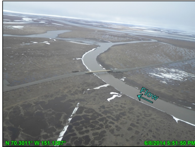
Photo C.28: Open channel at Nigliagvik Bridge crossing, looking north; June 8, 2014
