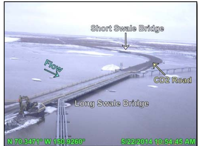
Photo 3.2: CD2 Road swale bridges conveying water, looking west; May 22, 2014
