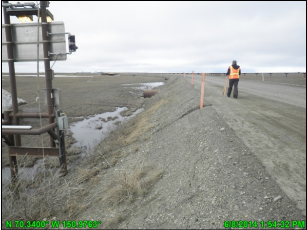
Photo C.8: CD2 Road Erosion Survey, looking north; June 8, 2014
