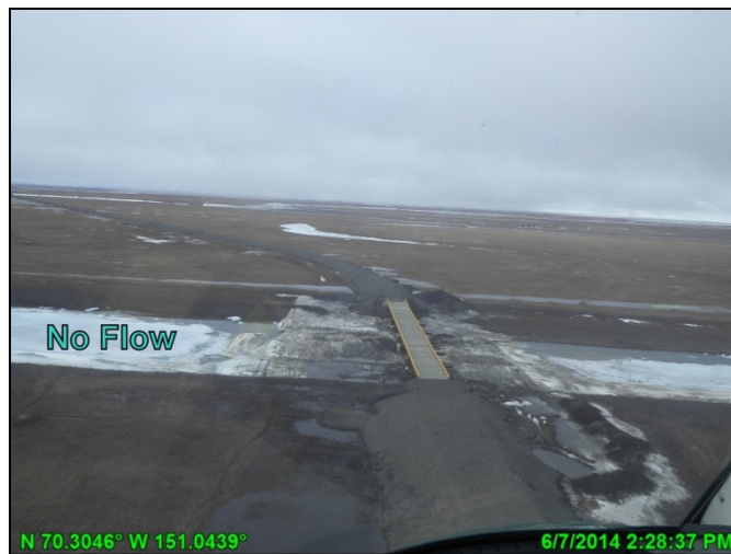
Photo C.30: Lake L9341 Bridge and construction ice pad, looking west; June 7, 2014
