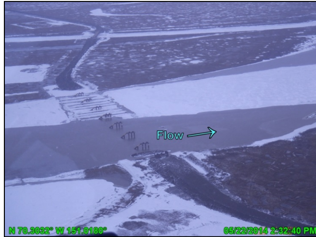
Photo C.25: Degradation of construction ice pad at Nigliq Channel Bridge crossing, looking west;
