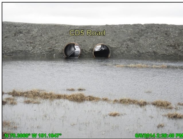
Photo 5.1: CD5 Road culverts adjacent to Gage S1, ponded local melt water with no observed flow, looking north; June 5, 2014
