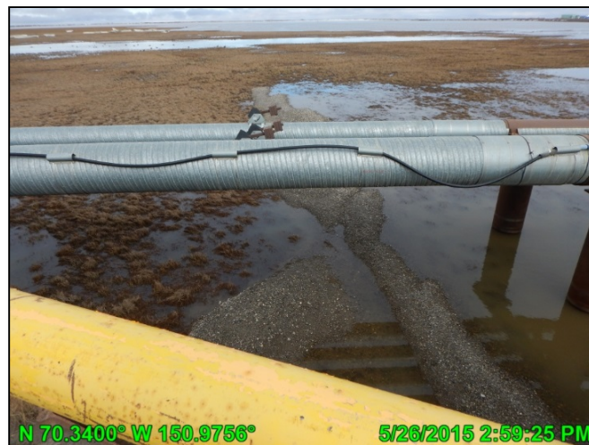
Photo C.10: Gravel outwash deposited on the north side of the Long Swale Bridge, looking north; May 26, 2015
