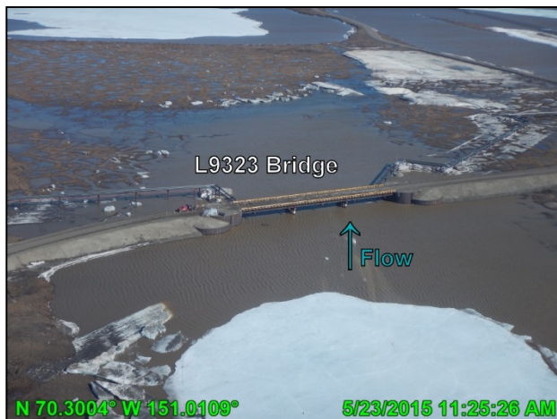
Photo 3.25: Lake L9323 Bridge following peak flooding, looking north toward connection with Nanuq Lake; May 23, 2015
