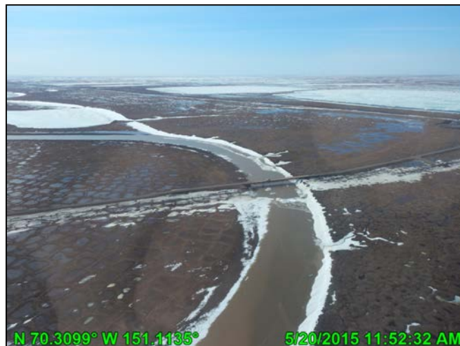
Photo C.41: Nigliagvik ice road crossing at CD5 road during breakup, looking south; May 20, 2015
