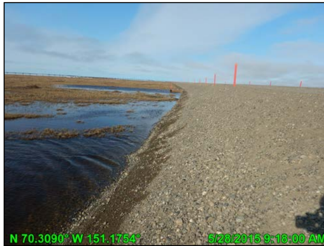
Photo C.21: CD5 road between gage S1 and the Nuiqsut Road intersection, looking west at culvert CD5-13; May 28, 2015
