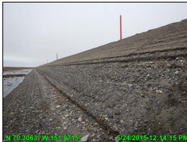
Photo C.25: Wash lines on the south side of the CD5 road between the Nigliagvik and L9341 bridges, looking west; May 24, 2015
