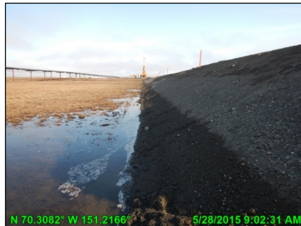
Photo C.18: CD5 road near the CD5 pad showing water saturated embankment on the west side of the road, looking north toward CD5 pad; May 28, 2015
