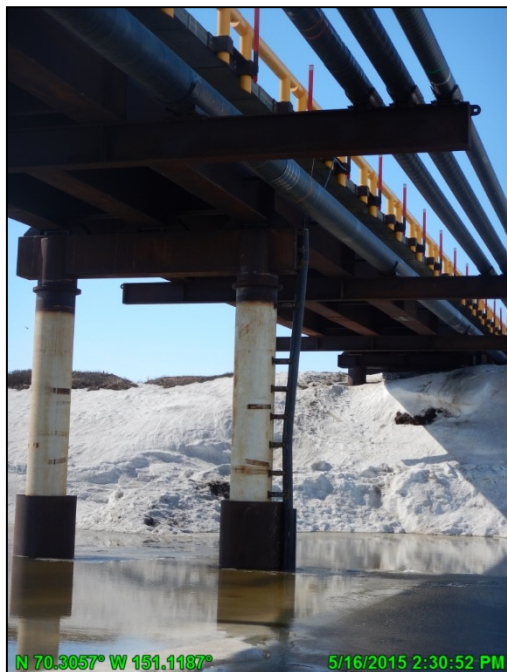
Photo 2.9: Steel pipe casing on Nigliagvik Bridge containing sonar for real-time scour monitoring; May 6, 2015
