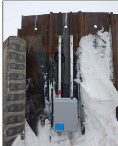
Photo 4: Nigliagvik Bridge fiberglass electronics enclosure hanging from the west abutment sheet pile; May 2015
