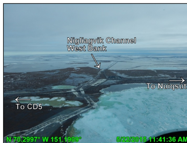
Photo 3.29: CD5 road looking east, flooding is contained by the Nigliagvik Channel and Lake M0356; May 22, 2015
