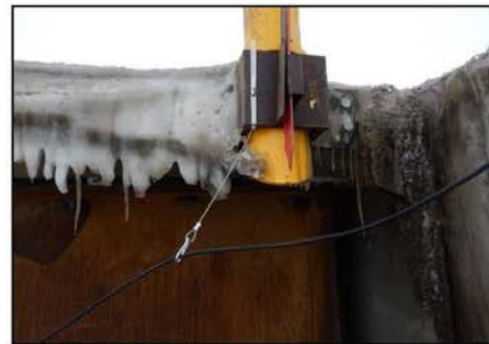
Photo 6: Nigliagvik Bridge sonar transducer cable hanger detail; May 2015
