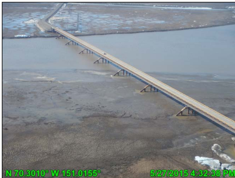
Photo 6.1: Nigliq Bridge Piers Post-Breakup; May 27, 2015
