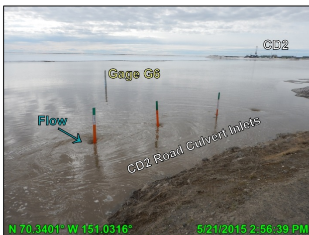
Photo 3.13: CD2 road culvert battery inlets inundated prior to peak WSE, looking west; May 21, 2015
