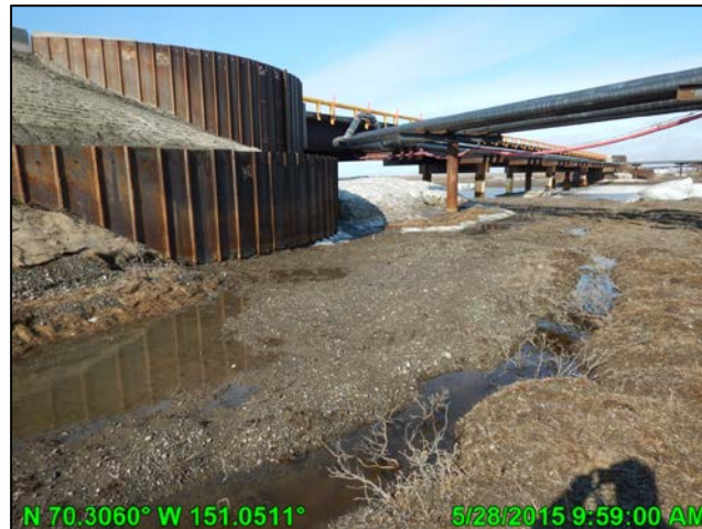
Photo C.26: Wash line and deposition at the north side of the L9341 Bridge east abutment, looking west; May 28, 2015
