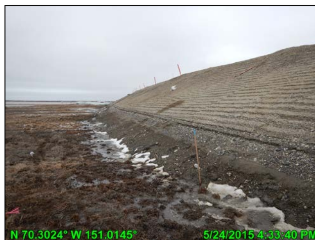
Photo C.28: Wash lines east of the Nigliq Bridge, looking west at south side of road; May 24, 2015
