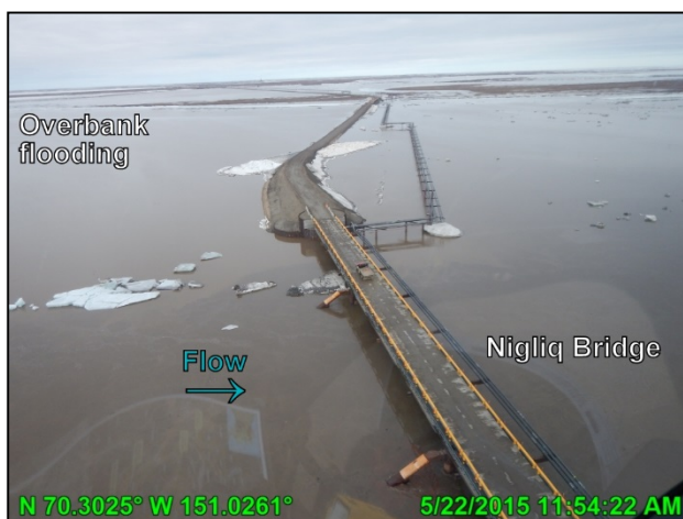
Photo 3.28: Inundation around the eastern half of the CD5 road, looking west after peak stage; May 22, 2015
