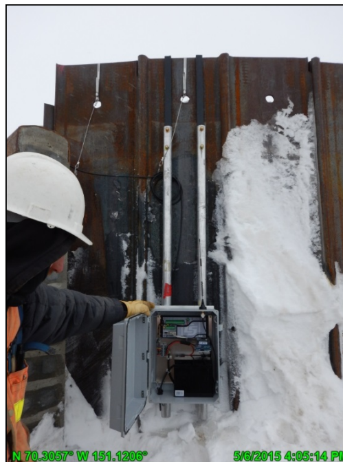
Photo 2.10: On-site data logger for Nigliagvik Bridge real-time scour sonar; May 6, 2015
