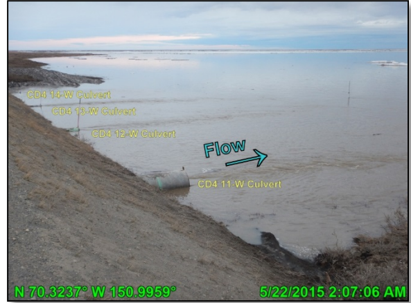
Photo 4.3: CD4 road north battery conveying flowing during peak conditions, looking north; May 22, 2015
