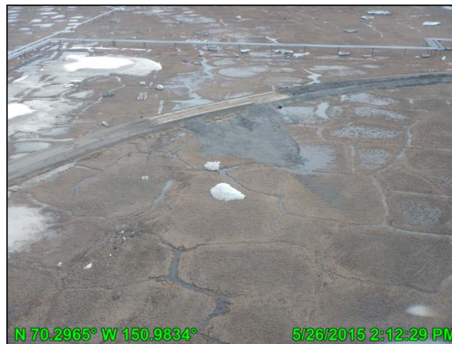
Photo C.13: Aerial view of the CD4 road washout showing the material deposit following initial clean up and road repair, looking southeast; May 26, 2015
