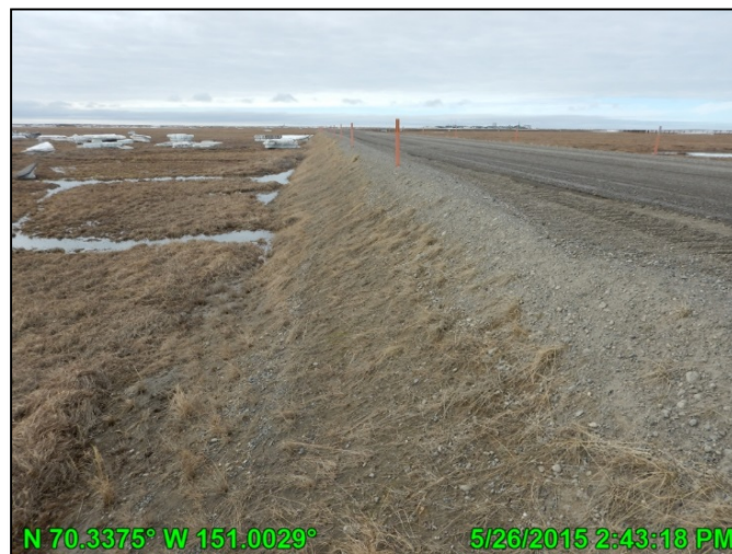
Photo C.2: Section of CD2 road near CD2 pad showing vegetation cover where no erosion occurred, looking east at the north side of the road; May 26, 2015
