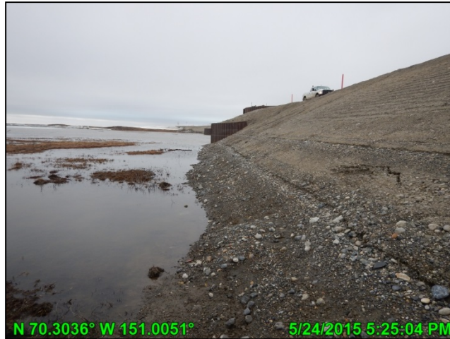
Photo C.29: Wash lines along the CD5 road east of the L9323 Bridge, looking west at south side of the road; May 24, 2015
