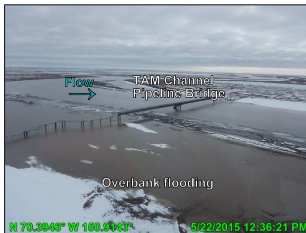
Photo 3.17: Tamayayak Channel at the CD3 pipeline crossing near the time of peak flooding, looking southeast; May 22, 2015
