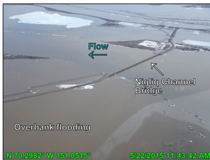
Photo 3.24: Inundation around the Nigliq Bridge 10 hours after peak stage, looking northeast; May 22, 2015
