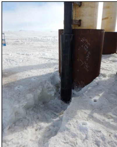
Photo 2: Bottom of the protective steel casing after ice removal; May 2015
