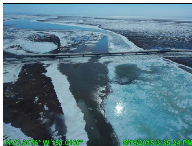
Photo C.45: Nigliq Channel ice road crossing at CD5 road during initial breakup, looking south; May 18, 2015
