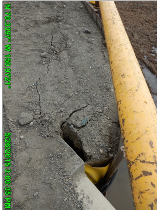
Photo C.12: Cracks in the Long Swale Bridge abutment fill, southeast abutment; May 26, 2015
