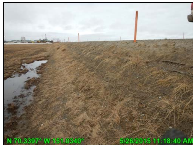
Photo C.4: HWMs along the south side of CD2 road near CD2 pad, looking west; May 26, 2015
