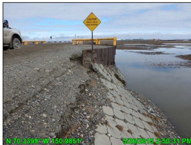
Photo C.8: Wash line at the Short Swale Bridge on the south side of the road showing scour at the sheet pile abutment, looking east; May 26, 2015
