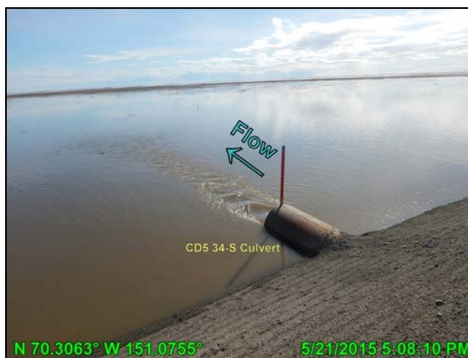
Photo 4.4: CD5 road culvert conveying flow during peak conditions; May 21, 2015
