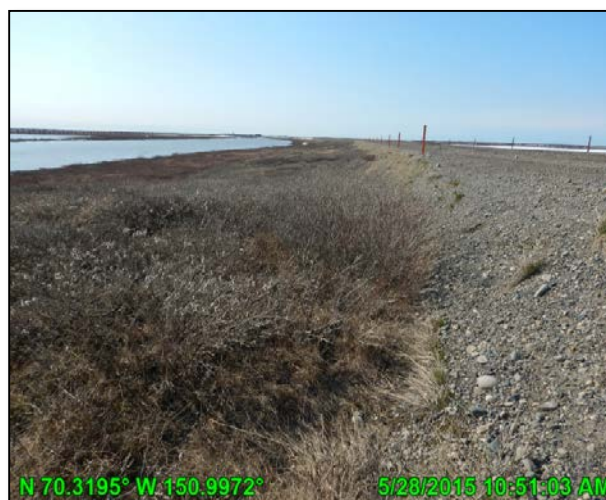
Photo C.16: Section of the CD4 road north of the CD5 road intersection unaffected by flooding, looking south; May 28, 2015
