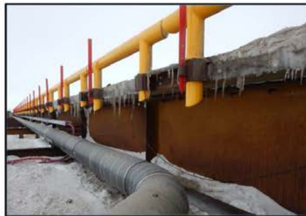
Photo 5: Nigliagvik Bridge sonar transducer cable routed through hangers from pier 3 to the west abutment; May 2015
