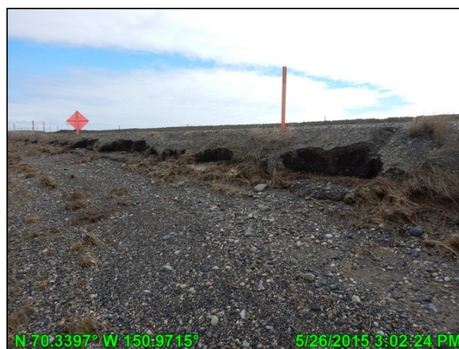
Photo C.11: Scour and deposition along the north side road embankment east of the Long Swale Bridge, looking south east; May 26, 2015
