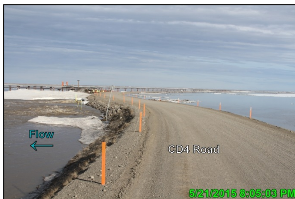
Photo 3.21: CD4 road looking southeast at north culvert battery at the time of the 5.74 foot WSE differential; May 21, 2015
