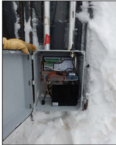
Photo 1: Electronics including the datalogger, cellular modem, and battery; May 2015
