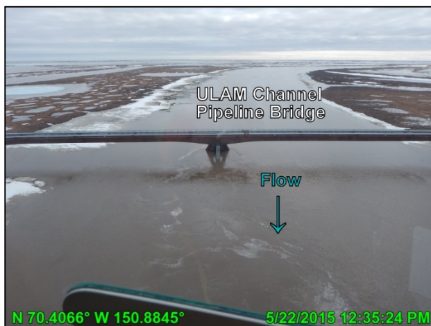
Photo 3.16: Ulamnigiq Channel at the CD3 pipeline crossing near the time of peak flooding, looking southeast; May 22, 2015
