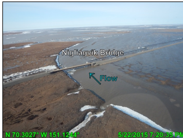
Photo 3.27 Nigliagvik Bridge following peak stage, looking north east; May 22, 2015
