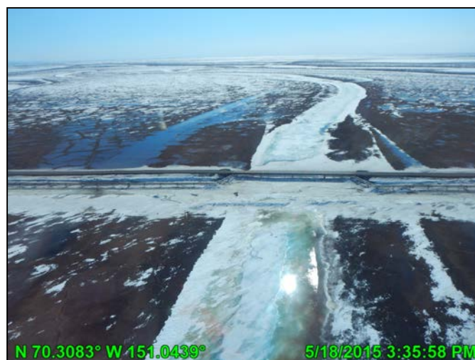
Photo C.36: Lake L9341 ice road crossing at CD5 road prior to breakup, looking south; May 18, 2015
