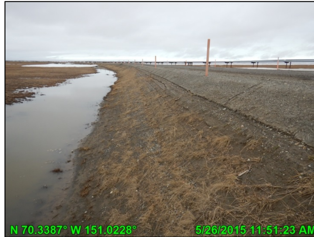
Photo C.3: Wash line on the south side of the western section of CD2 road, looking west between gages G6 and G12; May 26, 2015
