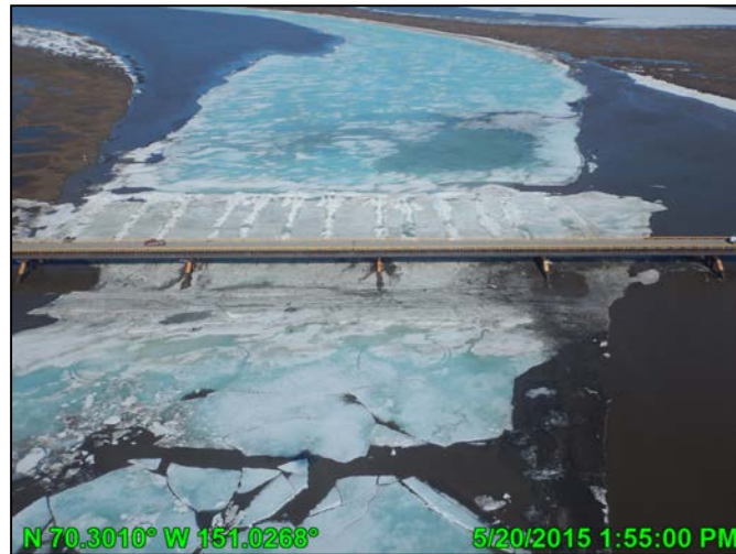
Photo C.46: Nigliq Channel ice road crossing at CD5 road during breakup, looking north; May 20, 2015
