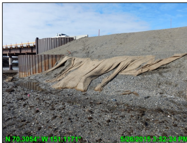
Photo C.22: Nigliagvik Bridge east abutment showing scour line and damaged erosion control material, looking west; May 28, 2015
