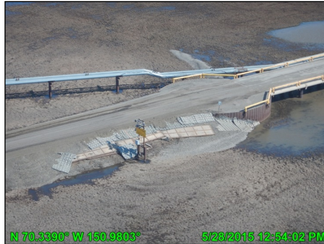
Photo C.9: Scour and deposition at the Long Swale Bridge west abutment, looking northeast; May 26, 2015
