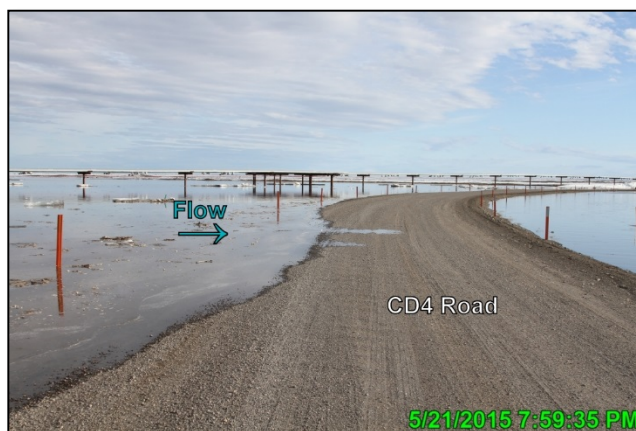
Photo 3.20: Floodwater overtopping the road near gage G18 prior to peak stage, looking south; May 21, 2015
