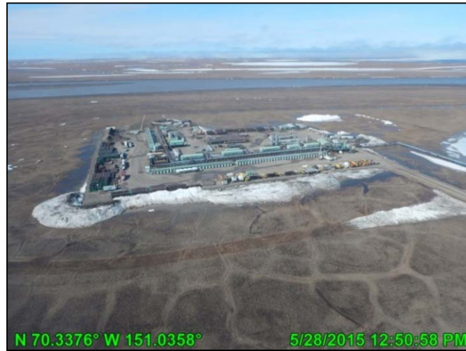
Photo C.1: CD2 pad showing snow coverage and ice road approach ramp remaining following flooding, looking west toward Nigliq Channel; May 28, 2015
