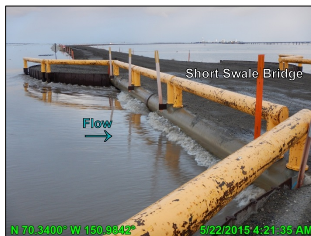
Photo 3.14: Flow through the CD2 road Short Swale Bridge following peak WSE, looking west, May 22, 2015
