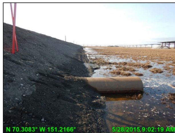
Photo C.19: CD5 road showing water saturated embankment and cracking, looking south on the west side of the road at culvert CD5-02; May 28, 2015
