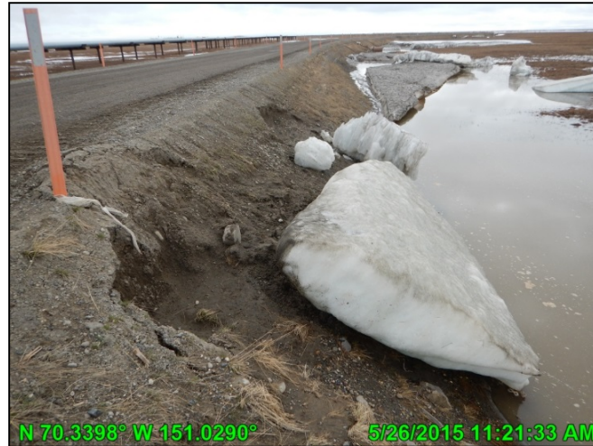
Photo C.6: Scarp from ice on the south side of CD2 road at gage G6, looking east; May 26, 2015
