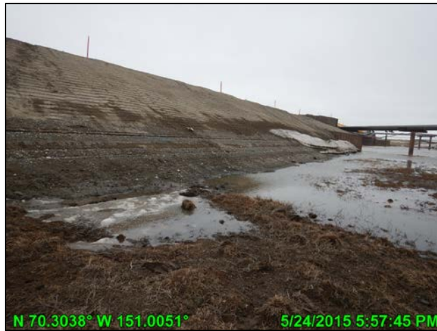
Photo C.30: Wash lines along the CD5 road east of the L9323 Bridge, looking west at north side of road; May 24, 2015
