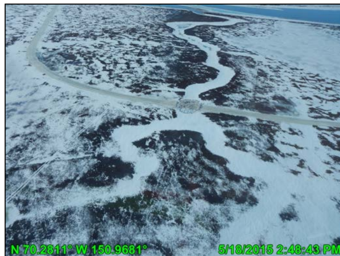
Photo C.62: Toolbox Creek ice road crossing prior to breakup, looking west; May 18, 2015
