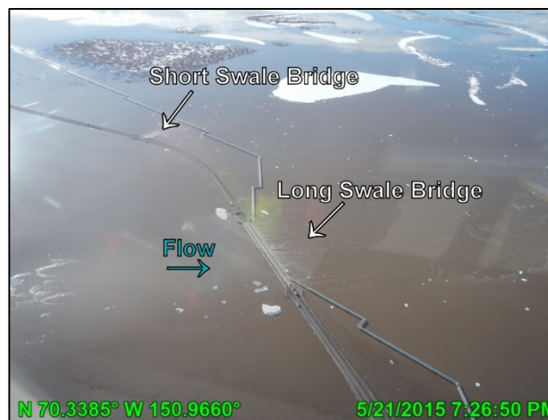
Photo 3.15: CD2 road swale bridges near the time of peak WSE, looking northwest; May 21, 2015
