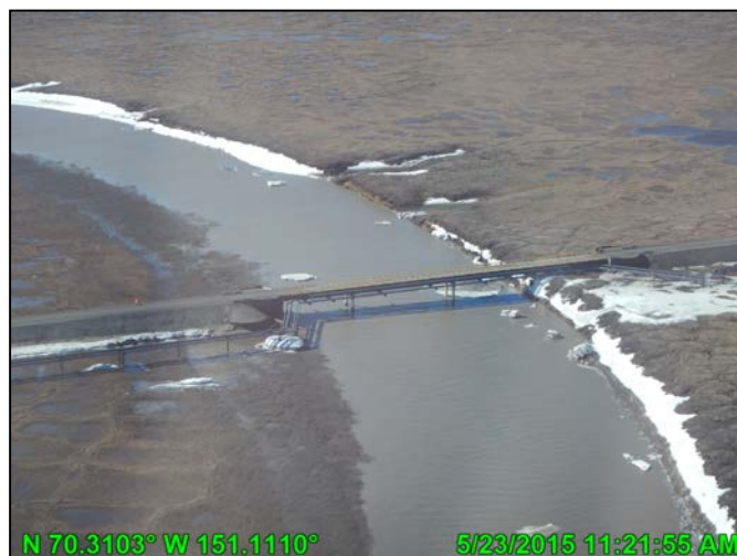
Photo C.42: Nigliagvik ice road crossing at CD5 road following breakup, looking south; May 23, 2015
