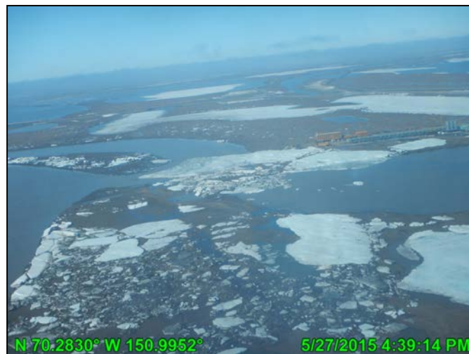
Photo C.56: Silas Slough ice road crossing following breakup, looking north; May 27, 2015
