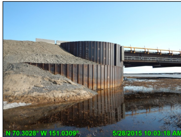
Photo C.27: Nigliq Bridge west abutment wash line and erosion control material, looking north east; May 25, 2015
