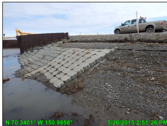
Photo C.7: Wash line at the Short Swale Bridge on the north side of the road, looking east; May 26, 2015
