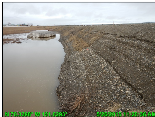
Photo C.5: Wash lines and vegetation scour around culvert CD2-4 on the western section of CD2 road, looking west at the south side of the road toward culvert CD2-3; May 26, 2015
