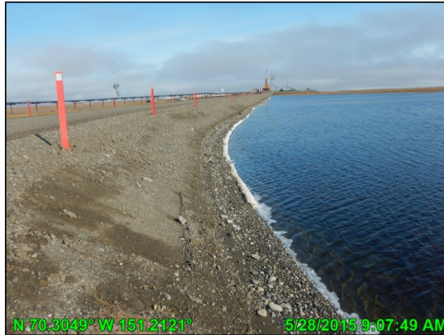
Photo C.20: CD5 road near the CD5 pad showing wash line on the east side of the road, looking north at Lake MB0301 toward CD5 pad; May 28, 2015
