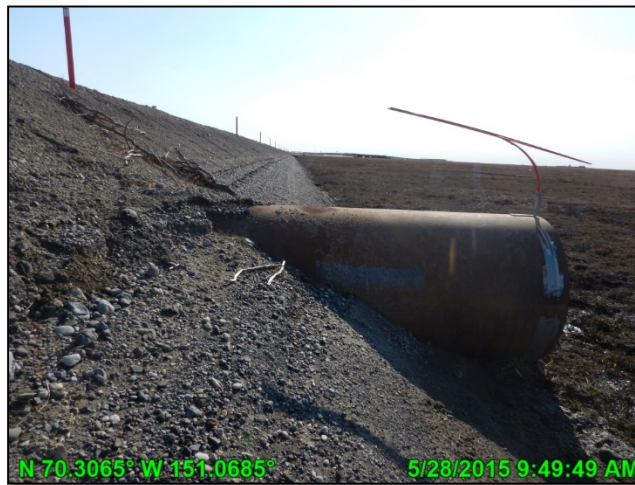
Photo C.24: Wash line on the south side of the CD5 road between the Nigliagvik and L9341 bridges, looking east at culvert CD5-35; May 28, 2015
