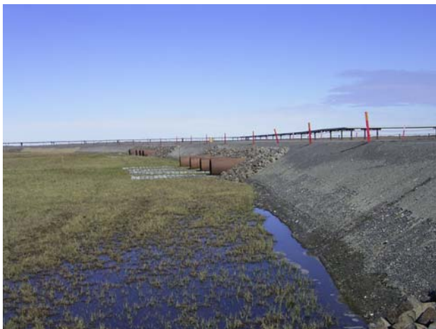
Photo 4-21 Northern Side of CD4 Access Road Erosion after Breakup at STA 200+00, June 15, 2006.
