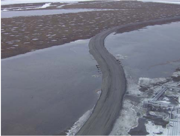
Photo 4-16 Northern CD4 Culvert Battery, May 30, 2006.
