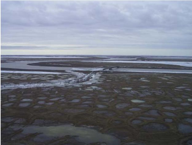
Photo 4-7 Tamayagiaq Channel Pipeline Bridge, June 2, 2006.
