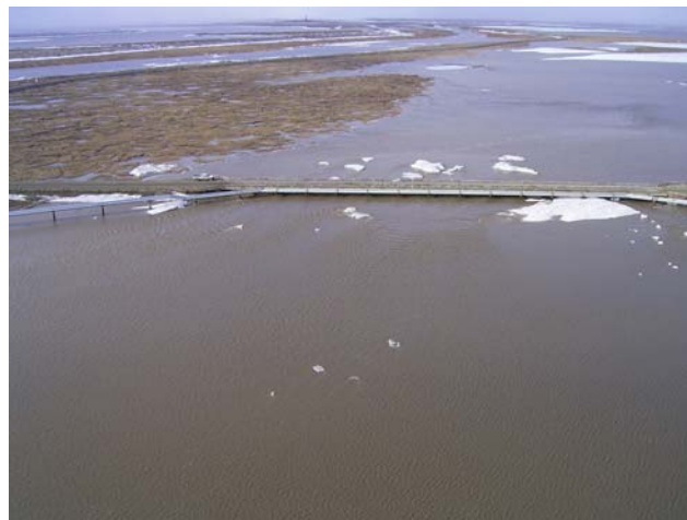
Photo 4-15 452-foot Swale Bridge, May 29, 2006.
