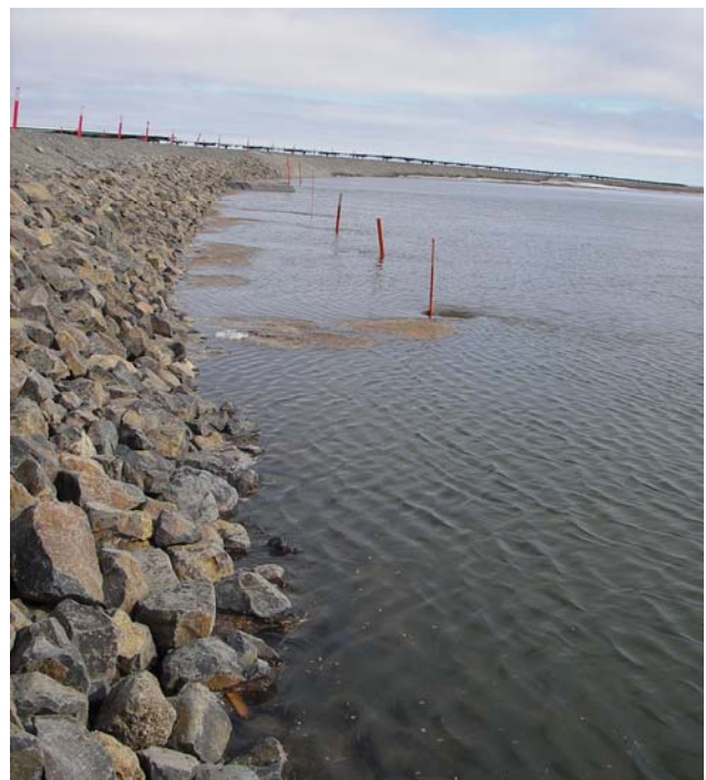
Photo 4-18 Peak Headwater at Northern CD4 Culvert Battery, May 30, 2006.
