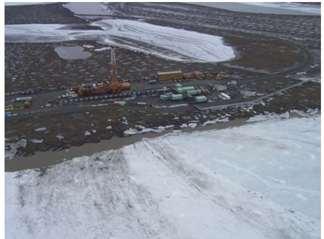
Photo 4-5 Stranded Ice next to CD4, June 1, 2006.
