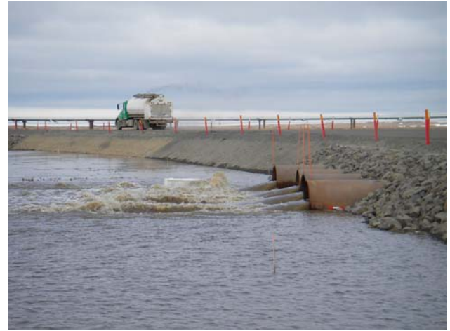
Photo 4-17 Southern CD4 Culvert Battery, May 30, 2006.
