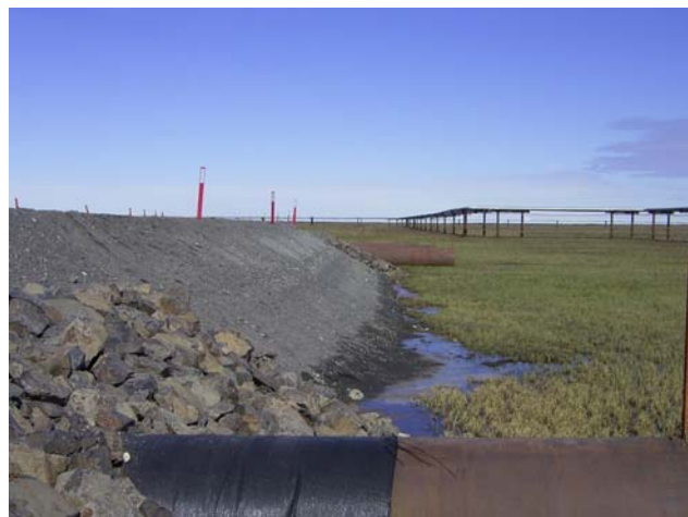
Photo 4-22 Southern Side of CD4 Access Road Erosion after Breakup at STA 200+00, June 15, 2006.
