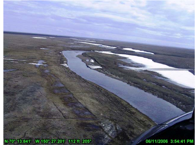
Photo 4-26 Kachemach River Ice Bridge after Breakup with Ice Road Remnants, June 11, 2006.
