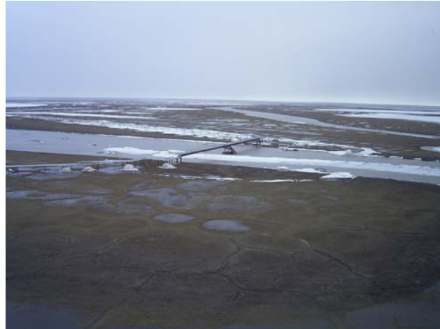
Photo 4-8 Ulamnigiaq Pipeline Bridge, June 2, 2006.
