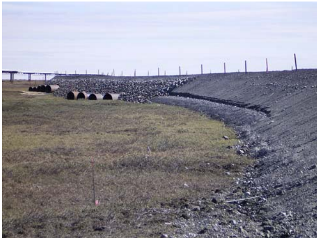
Photo 4-19 Fine Grained Sediment Settlement on Eastern Side of CD4 Road at STA 160+00, June 15, 2006.
