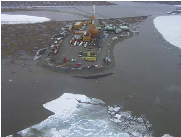
Photo 4-4 CD4 with Floodwater, May 30, 2006.
