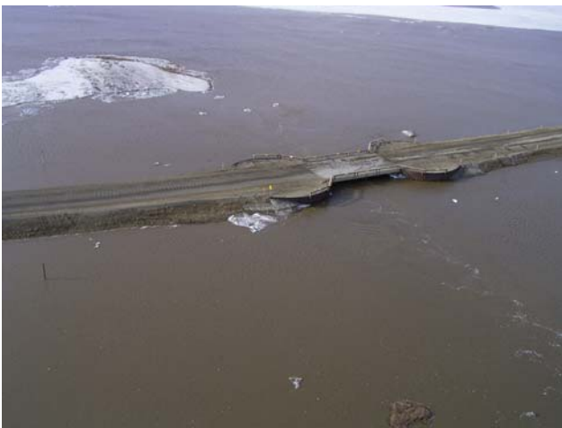
Photo 4-14 62-foot Swale Bridge, May 29, 2006.
