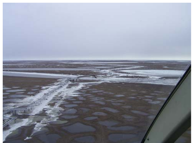
Photo 4-6 Sakoonang Channel Pipeline Bridge, June 2, 2006.
