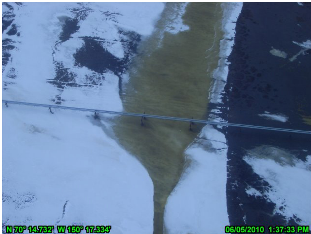
PHOTO A.22 MILUVEACH RIVER CROSSING, JUNE 5, 2010: PRE-BREAKUP, LOOKING SOUTH
