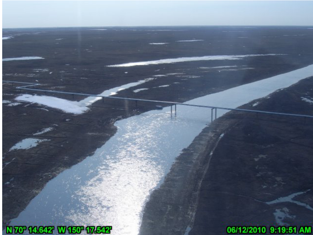
PHOTO A.24 MILUVEACH RIVER CROSSING, JUNE 12, 2010: LOOKING SOUTHEAST
