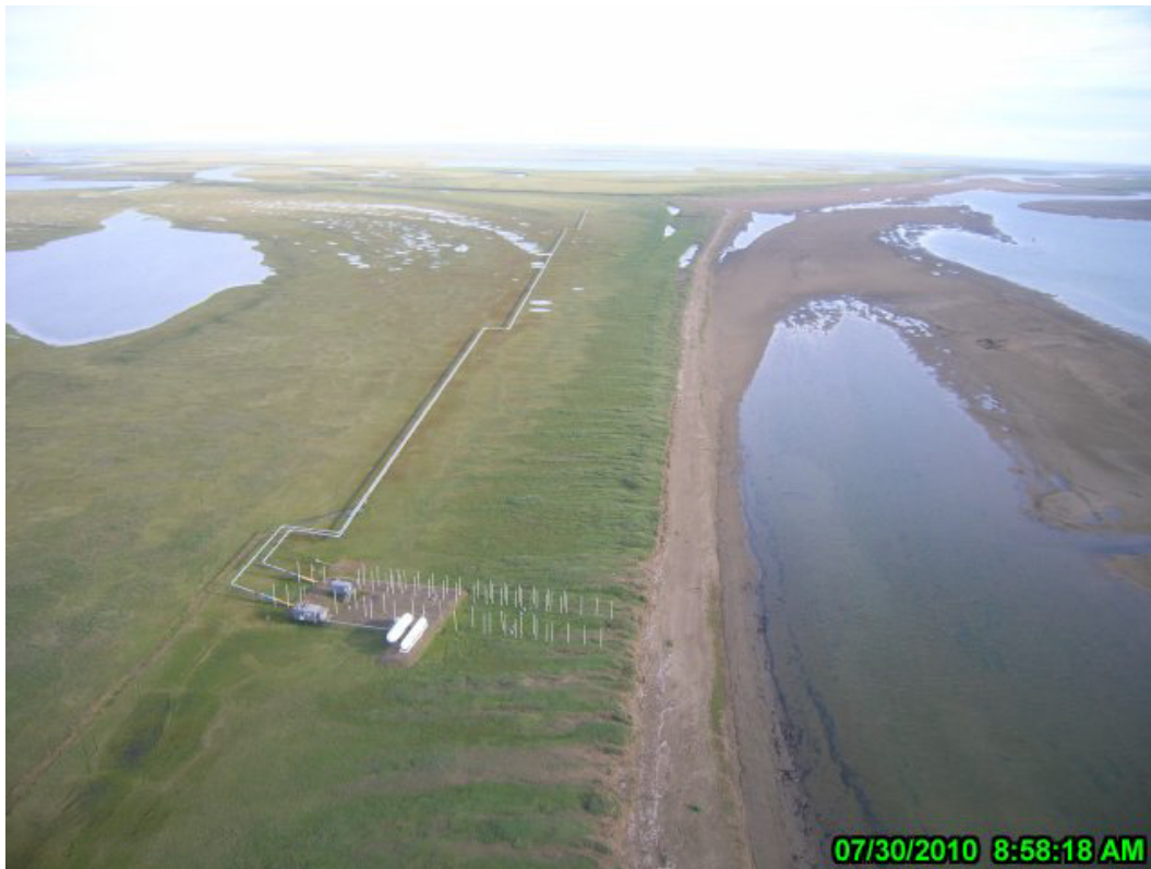
PHOTO A.3 HDD WEST, JULY 30, 2010: WEST BANK, LOOKING NORTH
