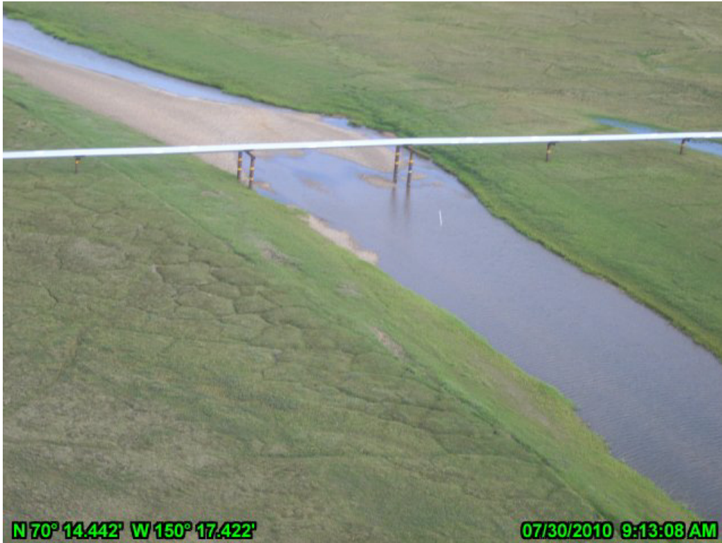
PHOTO A.25 MILUVEACH RIVER CROSSING, JULY 30, 2010: LOOKING NORTHEAST
