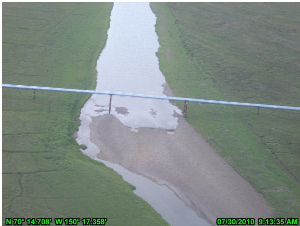
PHOTO A.26 MILUVEACH RIVER CROSSING, JULY 30, 2010: LOOKING SOUTH
